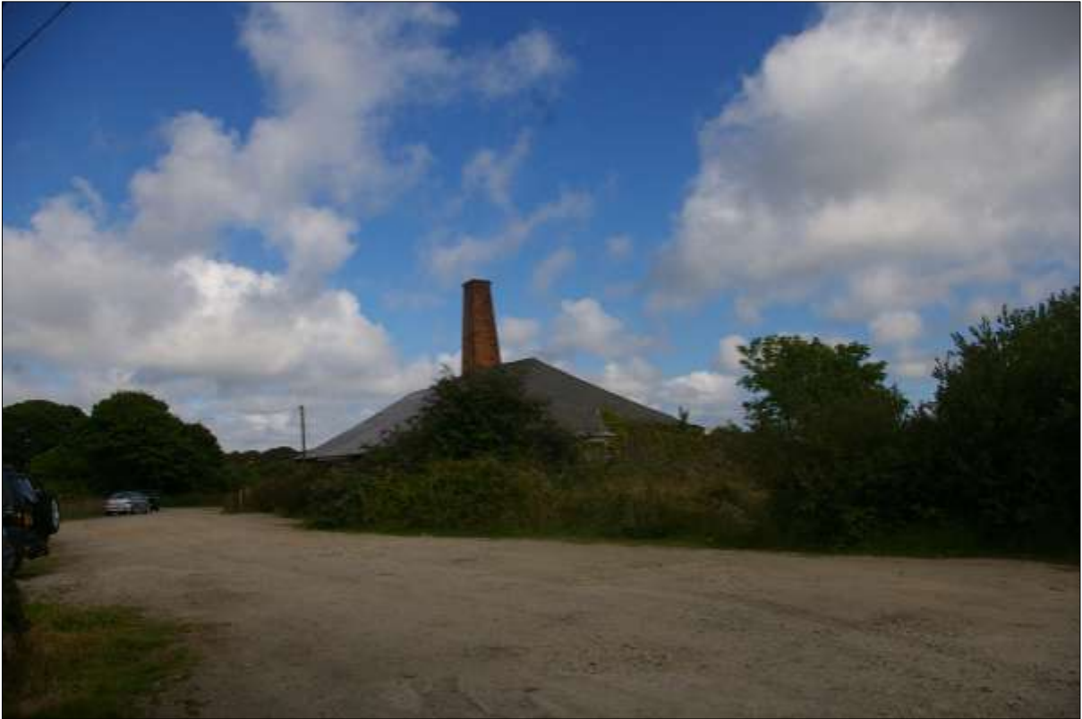
Mine buildings near Chacewater, Wheal Busy; from the north-west.
