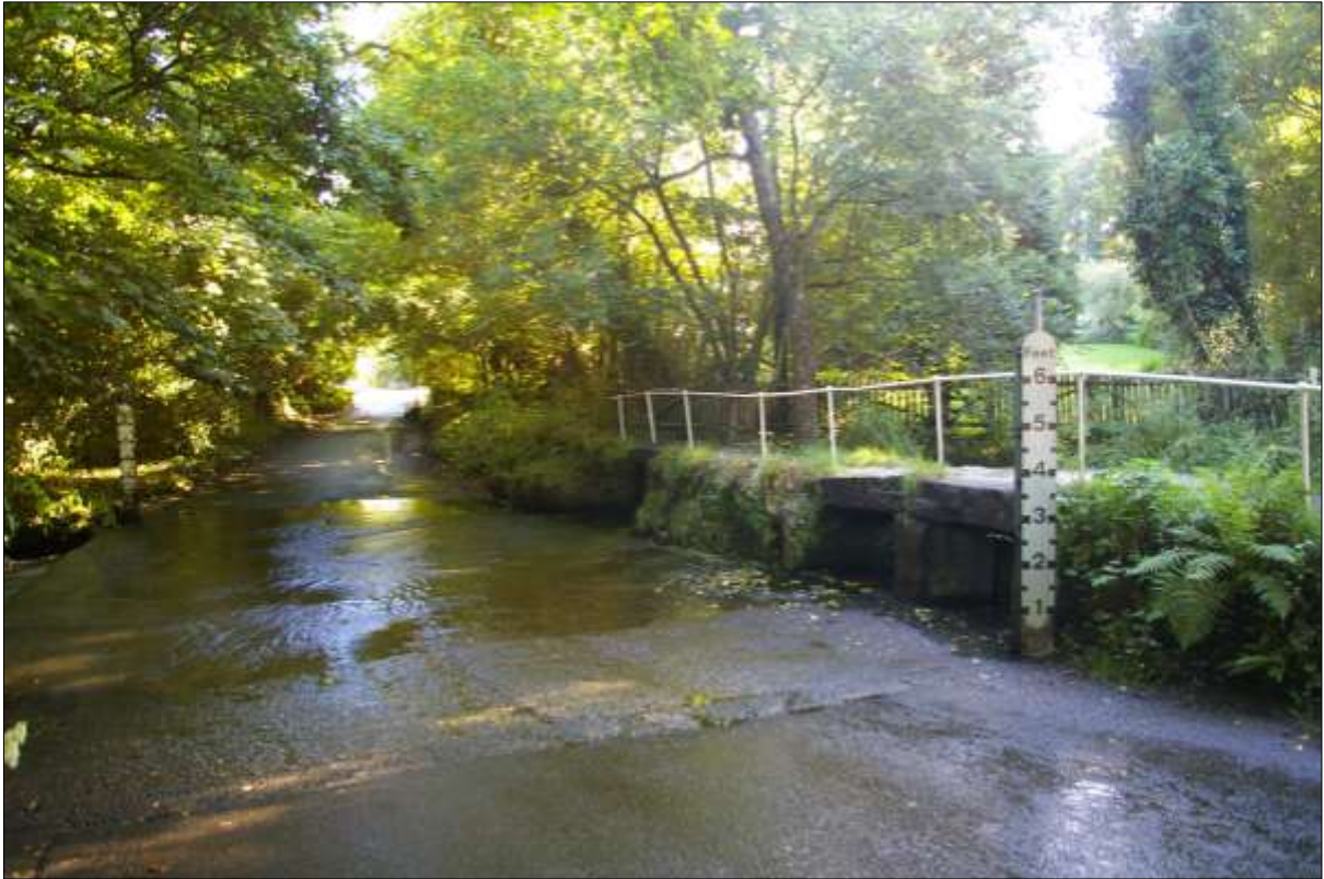
Footbridges over the River Kenwyn at Newmills; from the north.
