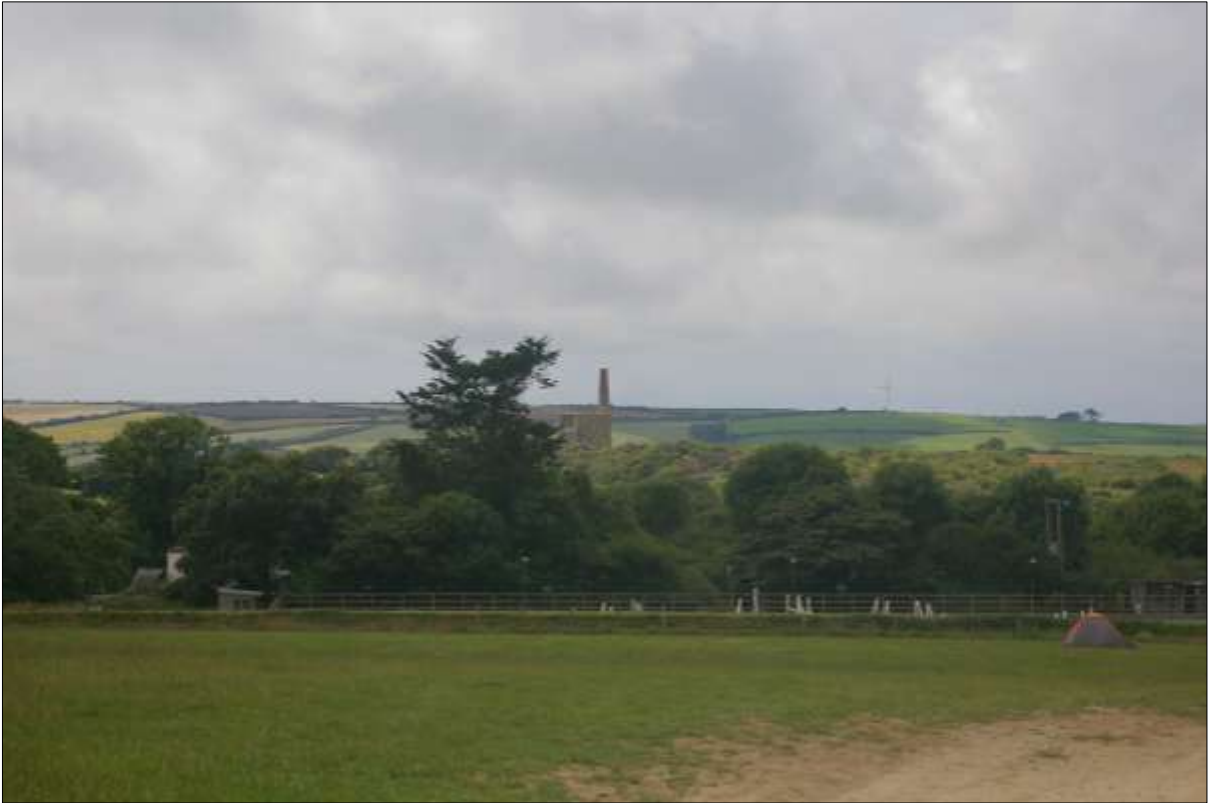
More engine houses and mine buildings near Ventongimps; from the north-east.
