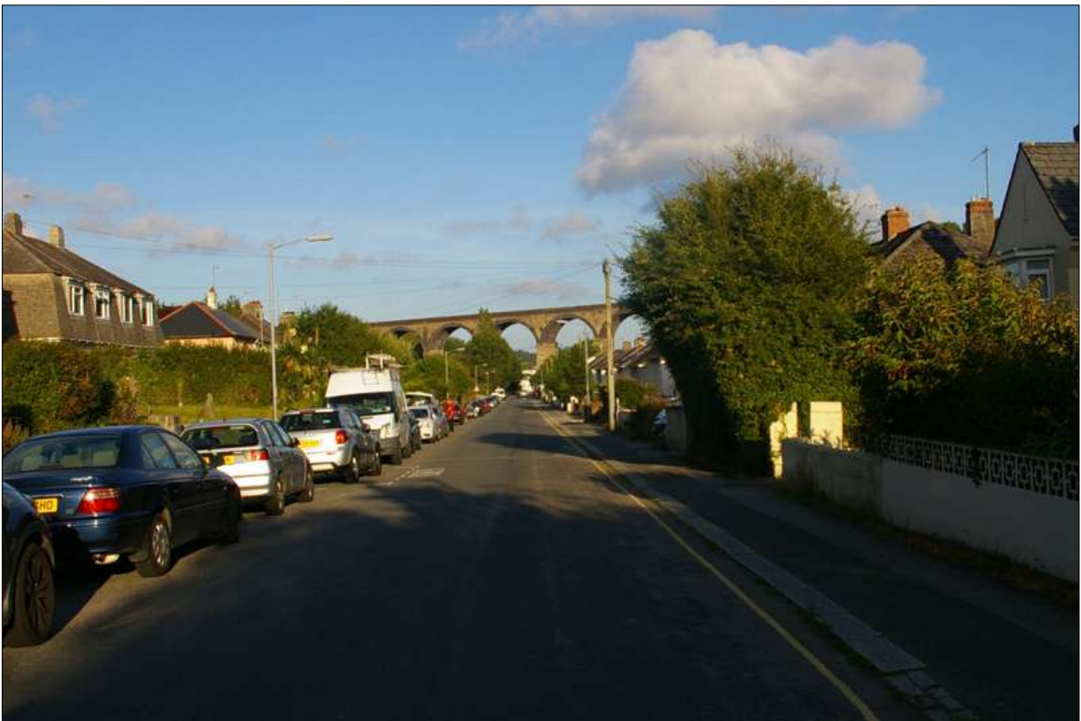
Truro viaduct; from the north.
