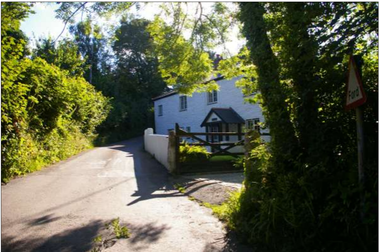
Cottages in Newmills, shielded by the trees and valley topography; from the east.
