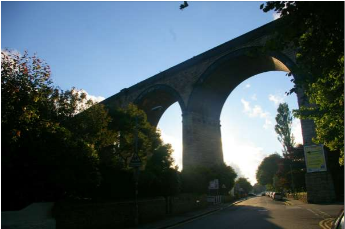
The viaduct; from the south-east.
