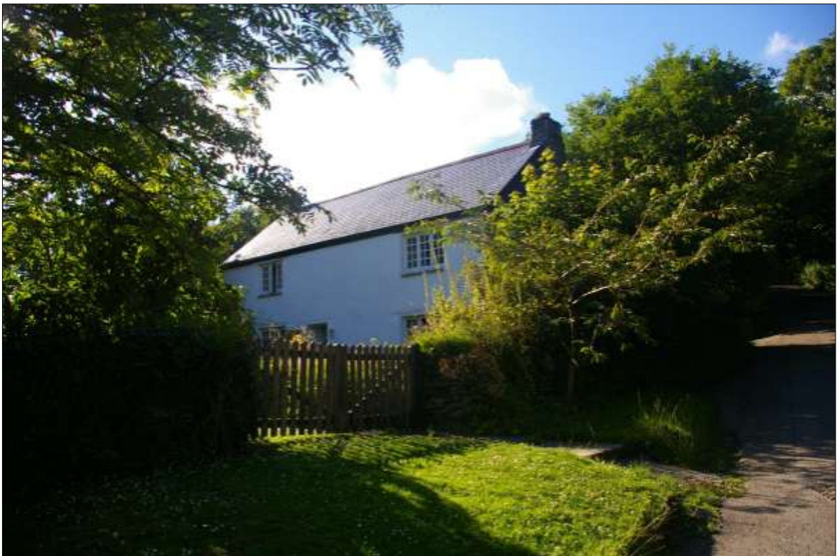
New Mill cottage; from the south-east.
