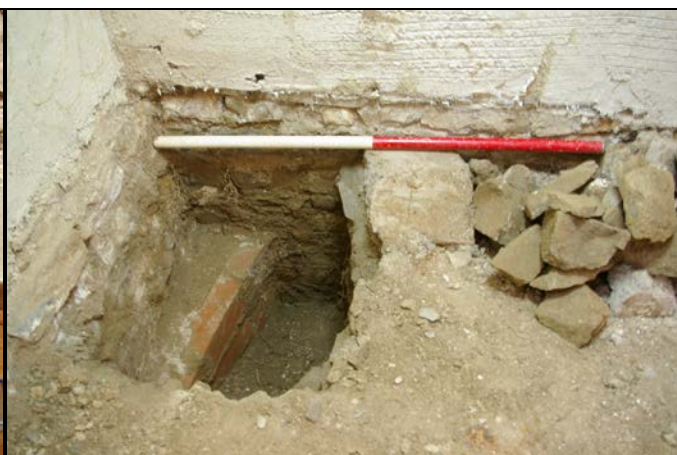
Figure 10: Test pit in south west corner, showing the brick foundations (1m scale).
