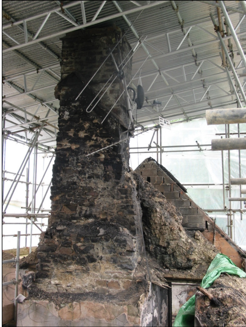
Figure 12: The eastern stack with surviving flashing, viewed from the west.
