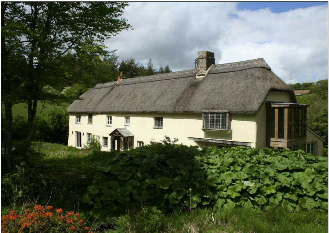
Figure 10: The renovated south elevation of Knowstone Mill, viewed from the south.
