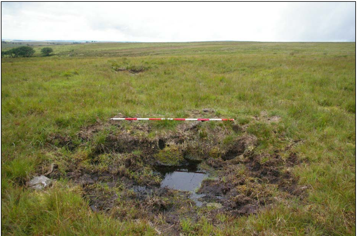
Figure 4: View of cutting 597 showing its condition, viewed from the east (2m scale).
