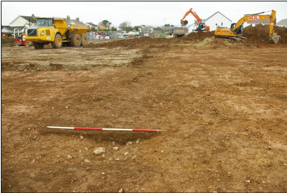
Figure 4: View along Ditch [102], viewed from the west (2m scale).
