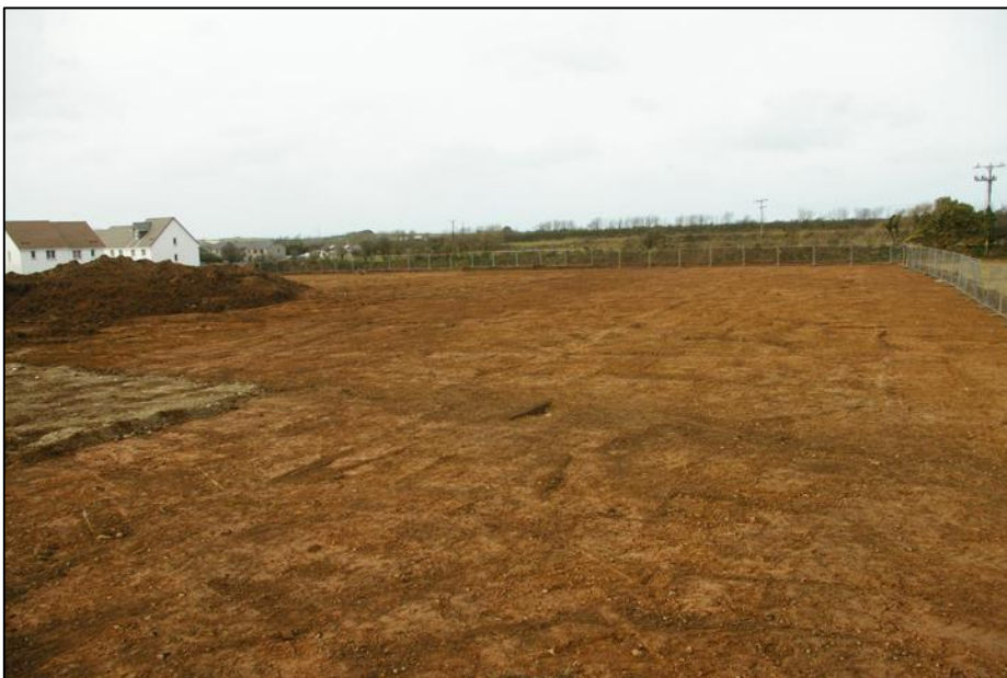
Figure 5: Site shot, post-excitation, viewed from the north-west (no scale).
