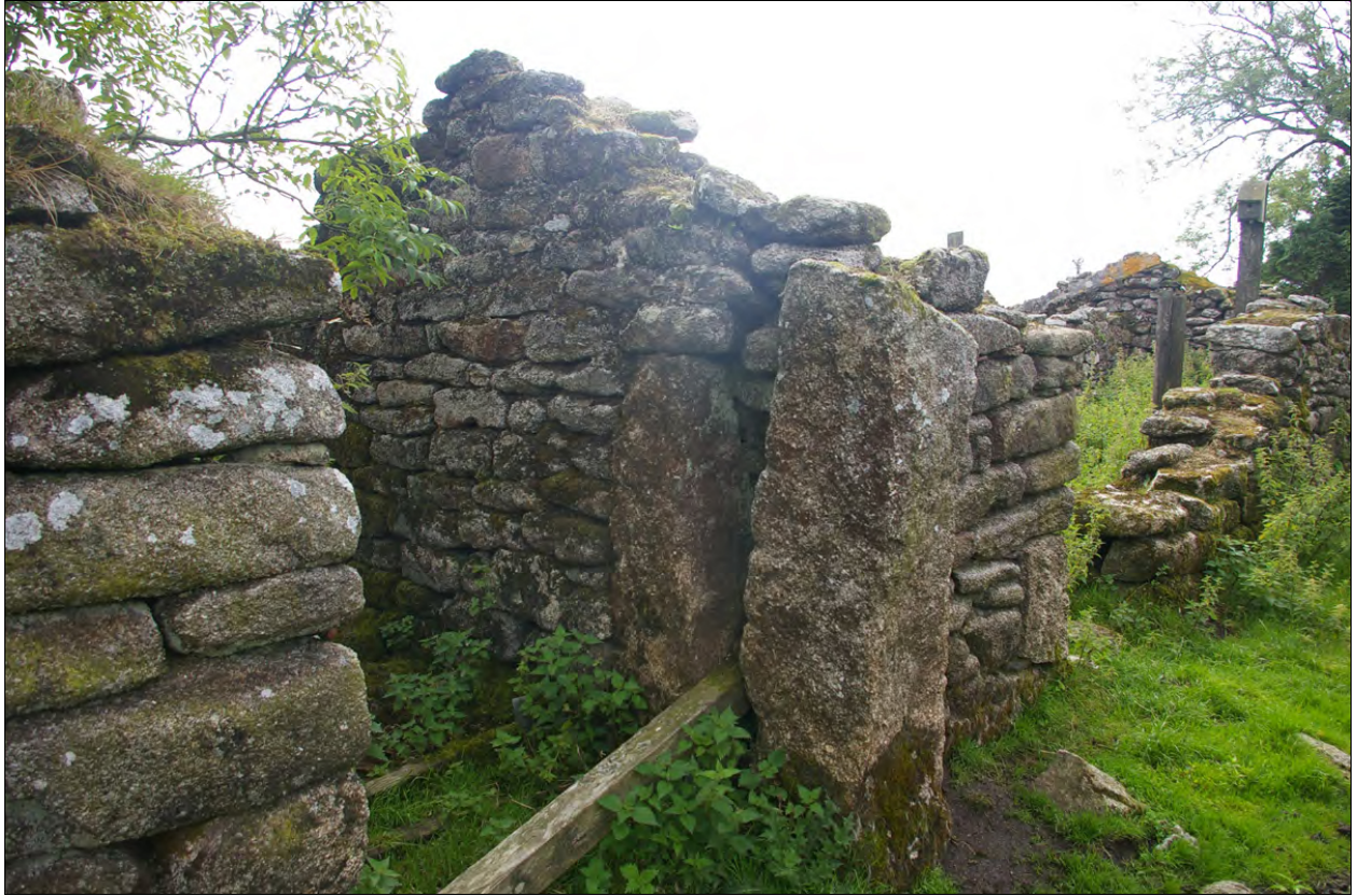
Detailed view of the doorway into Building 3d; from the north-east.
