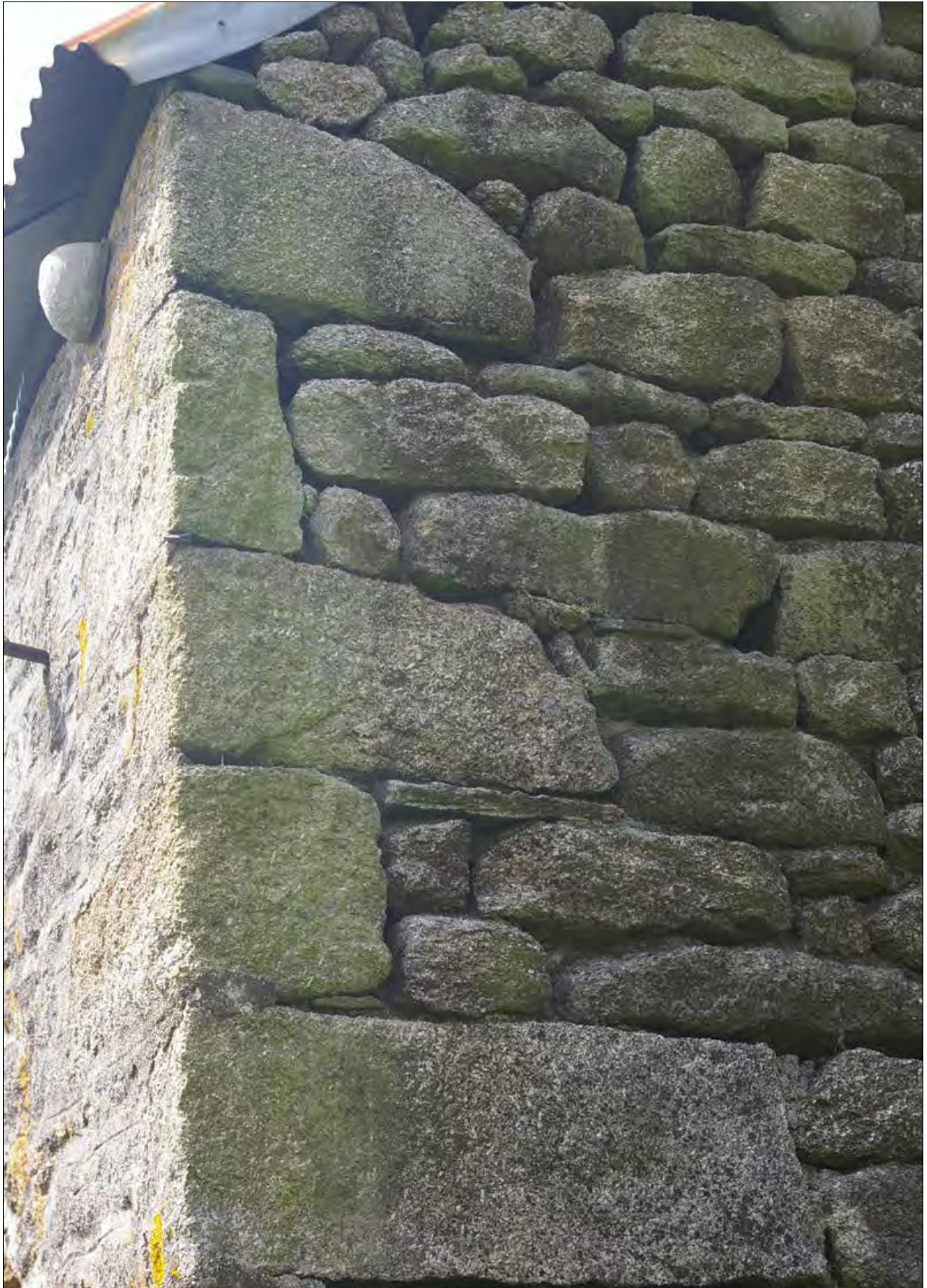
The quoins to the south-east corner of Building 1; from the south-east.
