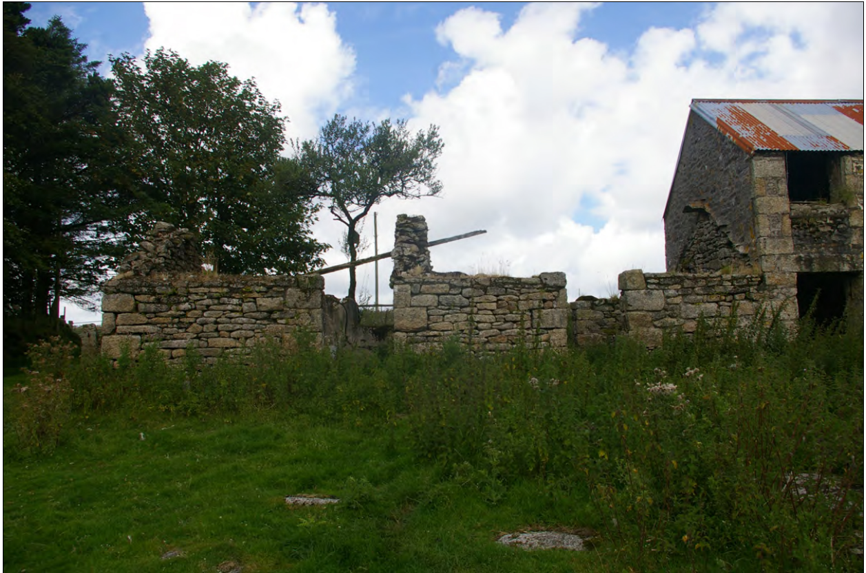
The south elevation of Building 1a; from the south.
