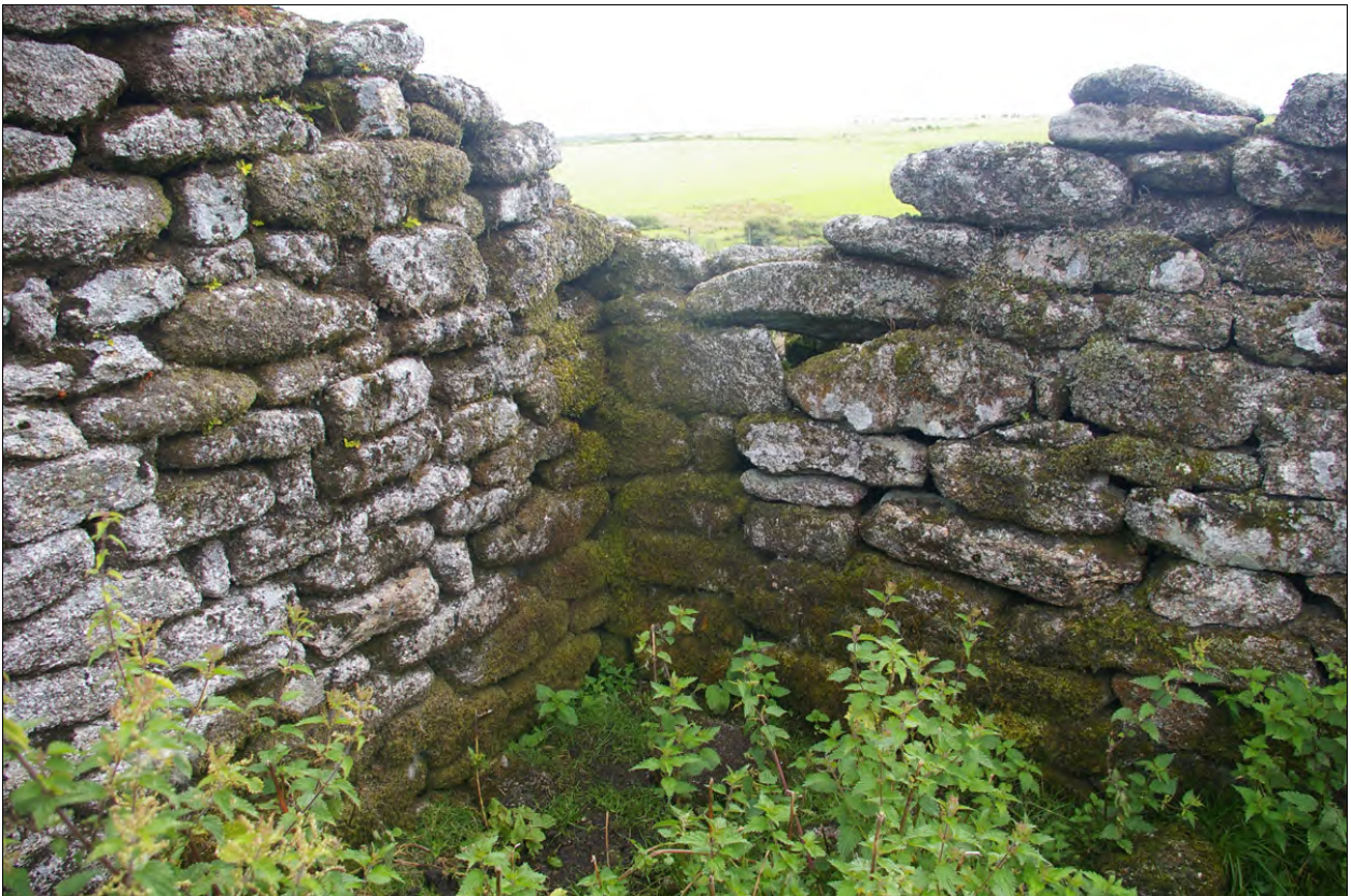
The south-east corner of Building 3d; from the north-west.
