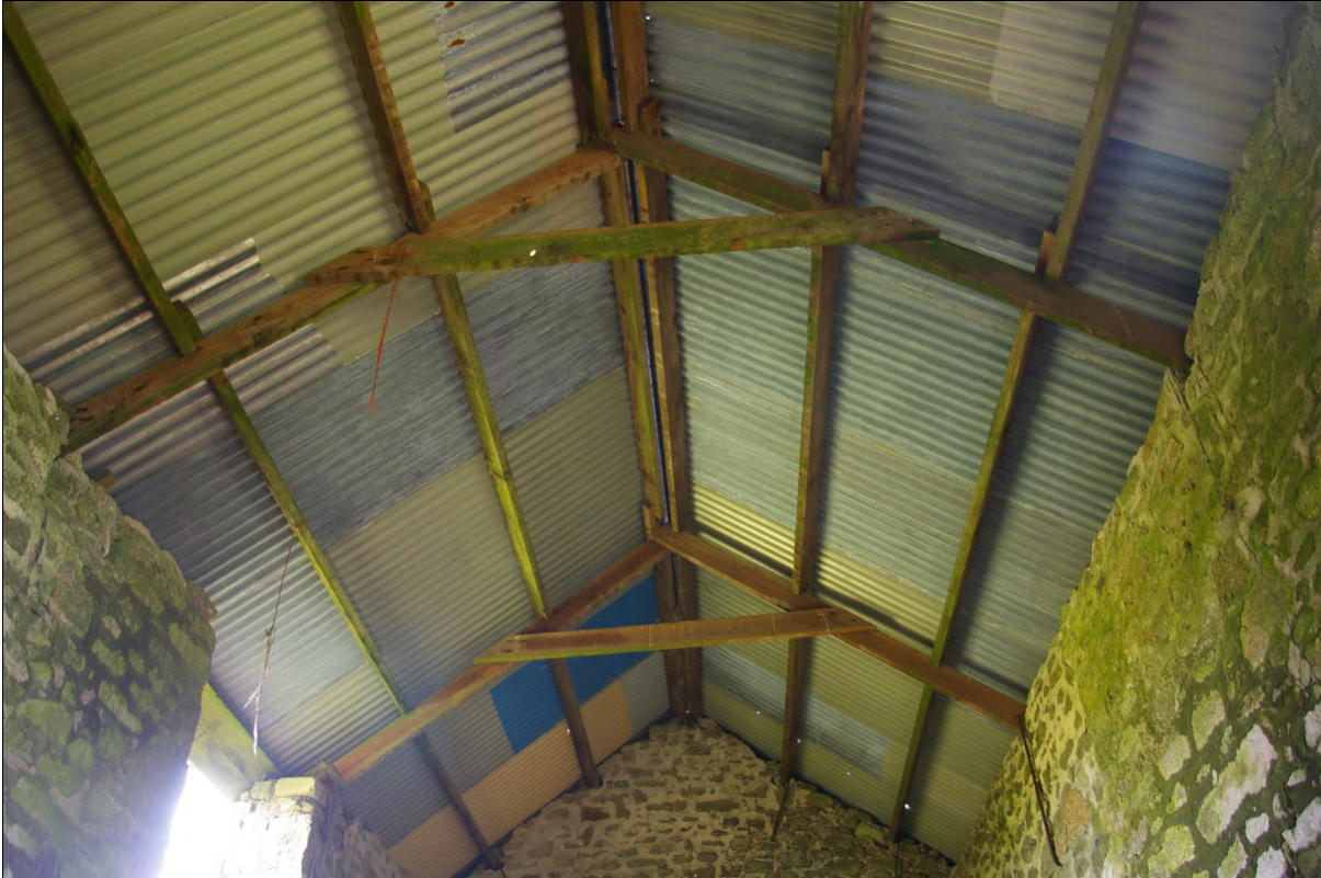
The modern timber trusses of the roof structure
