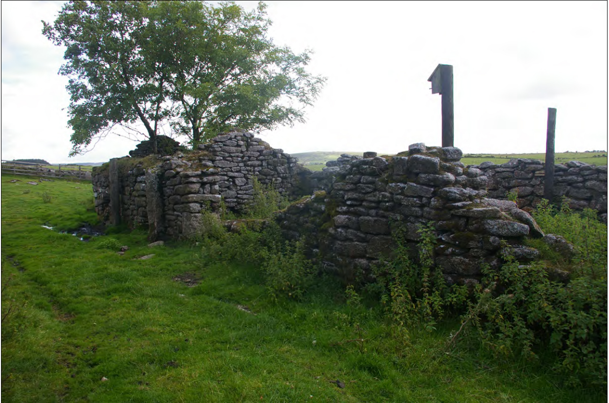
Building 3, sections B3c and B3d, at the eastern end of the building range; from the north-west.
