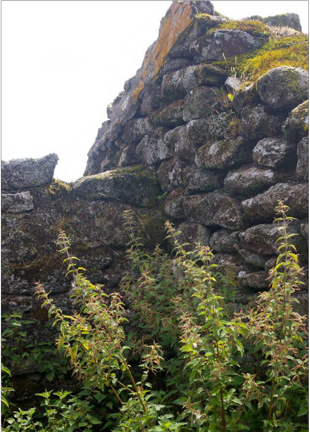
Detailed view of where Building 3c abuts the east wall of the earlier building, Building 3b; from the north, north-east.
