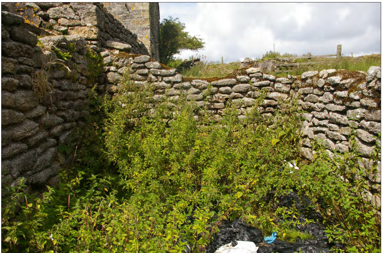
View into building abutting 2b; from the south.
