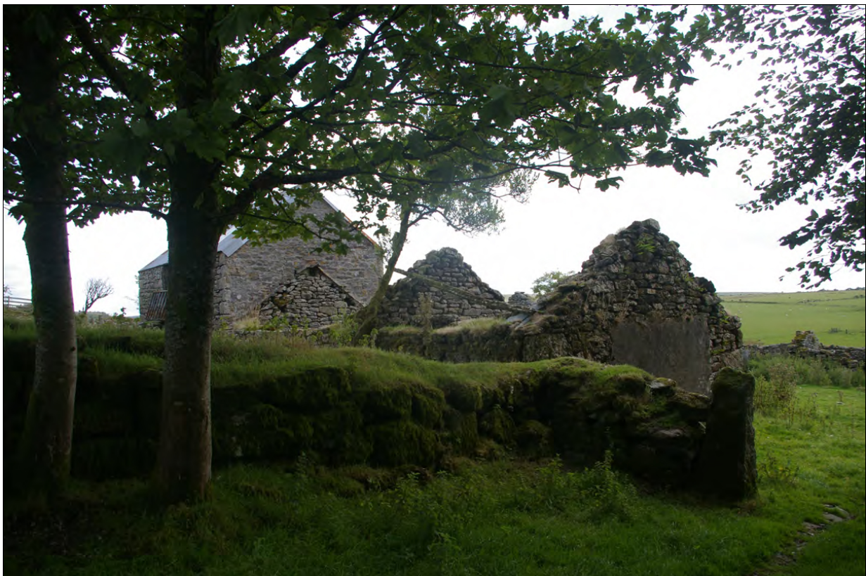
The north side of the farmyard, from the entrance; from the north-west.
