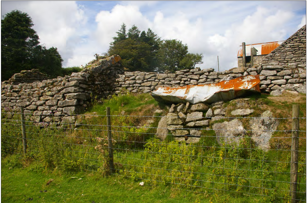
Section of further built wall, ruined and backfilled now part of the field bank; from the south-east.
