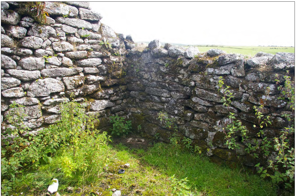
The south-east corner of Building 2b; from the north-west.
