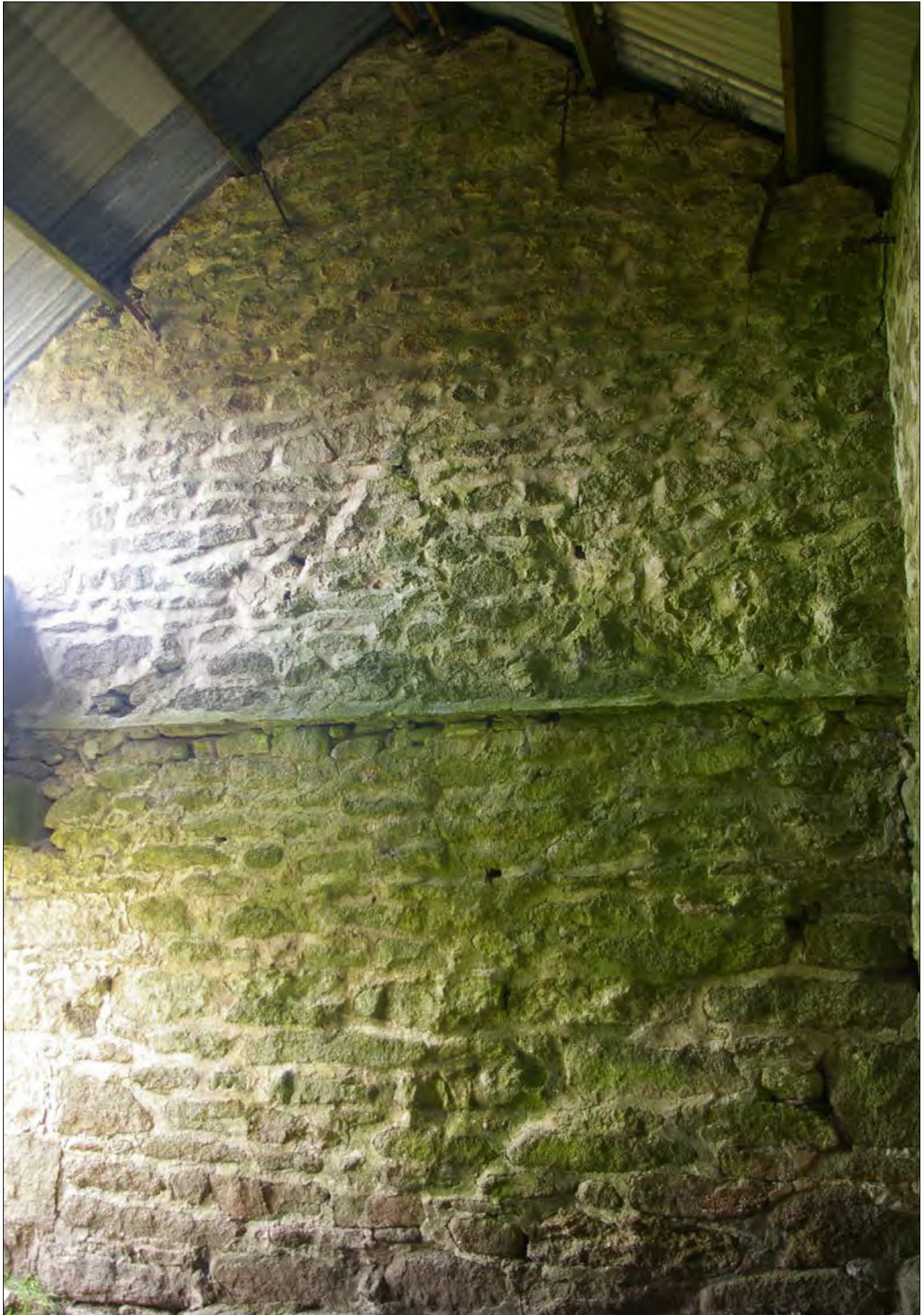
The west wall of Building 1; from the east.
