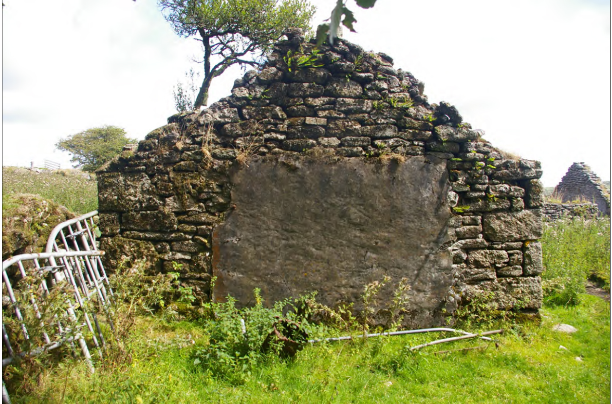
The west elevation of Building 1a; from the west.
