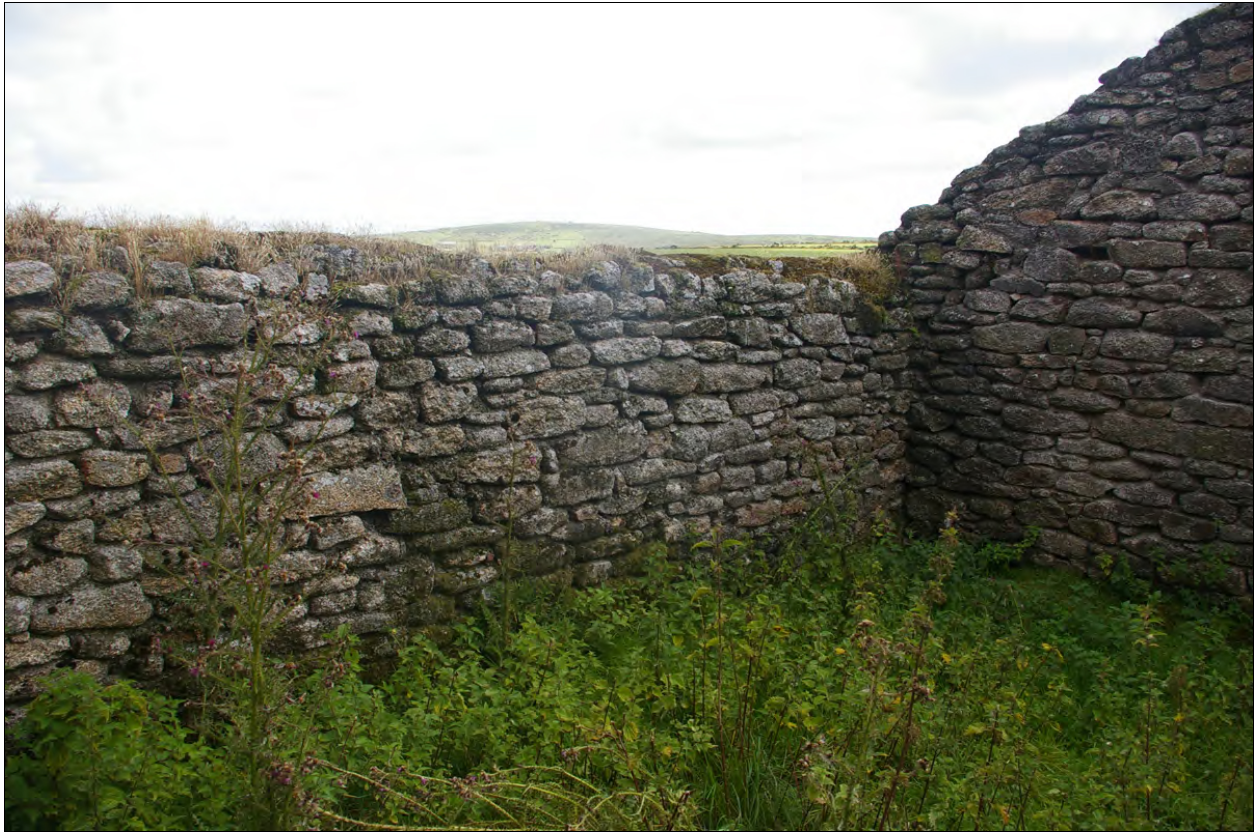
The interior face of the east wall within Building 2c; from the north-west.
