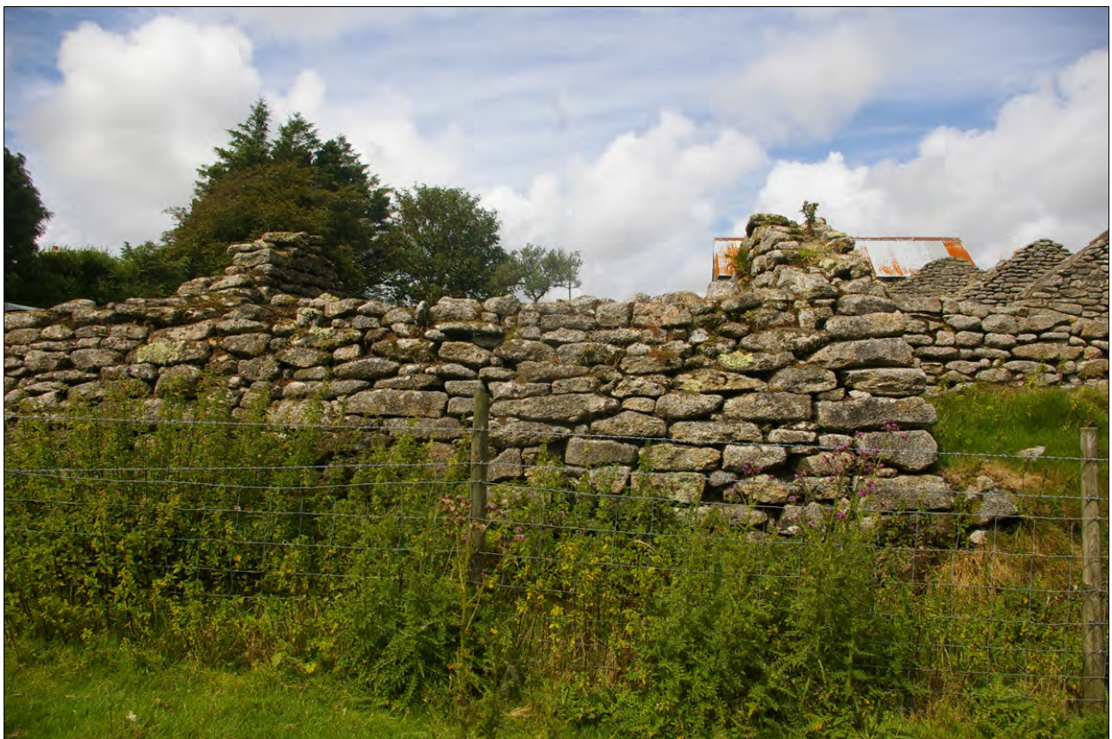
The south elevation of Building 3b; from the south-east.
