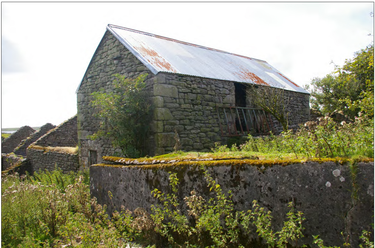
Building 1 and Building 2; from the north, north-east.
