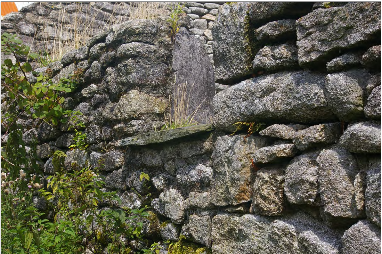
Detailed view of the window in the west wall of Building 2b; from the south-west.
