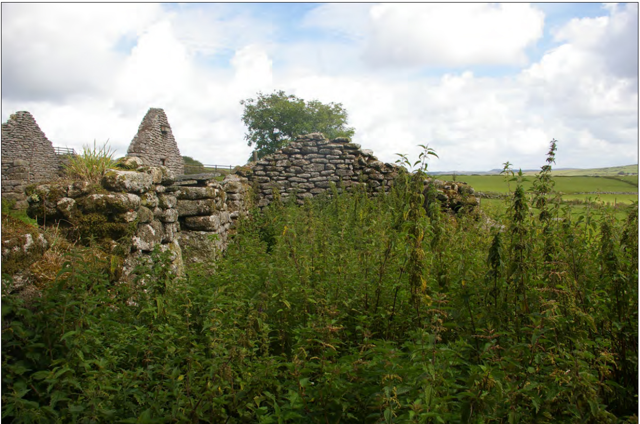
View along the interior of Building 3a; from the west.
