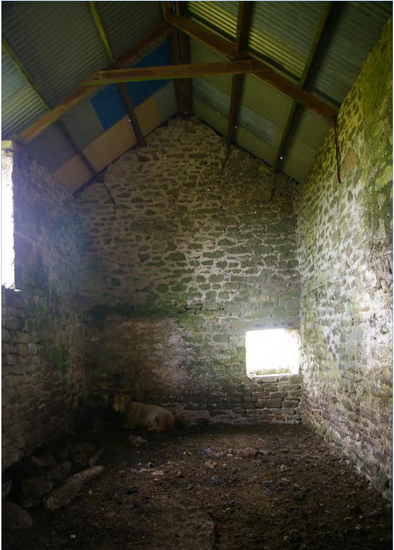
The interior of Building 1, the eastern end; from the west.
