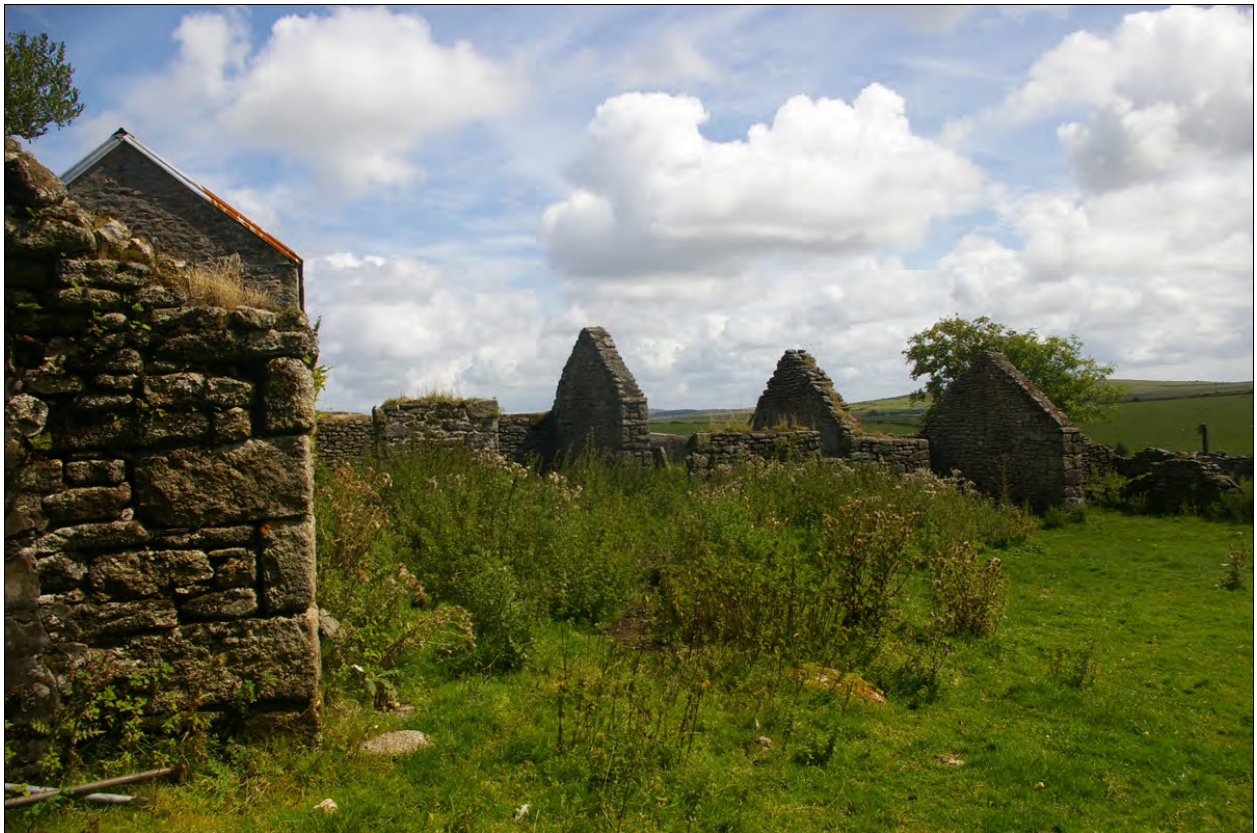
View across the north side of the farmyard, showing Building 1a and Building 2; from the west, north-west.
