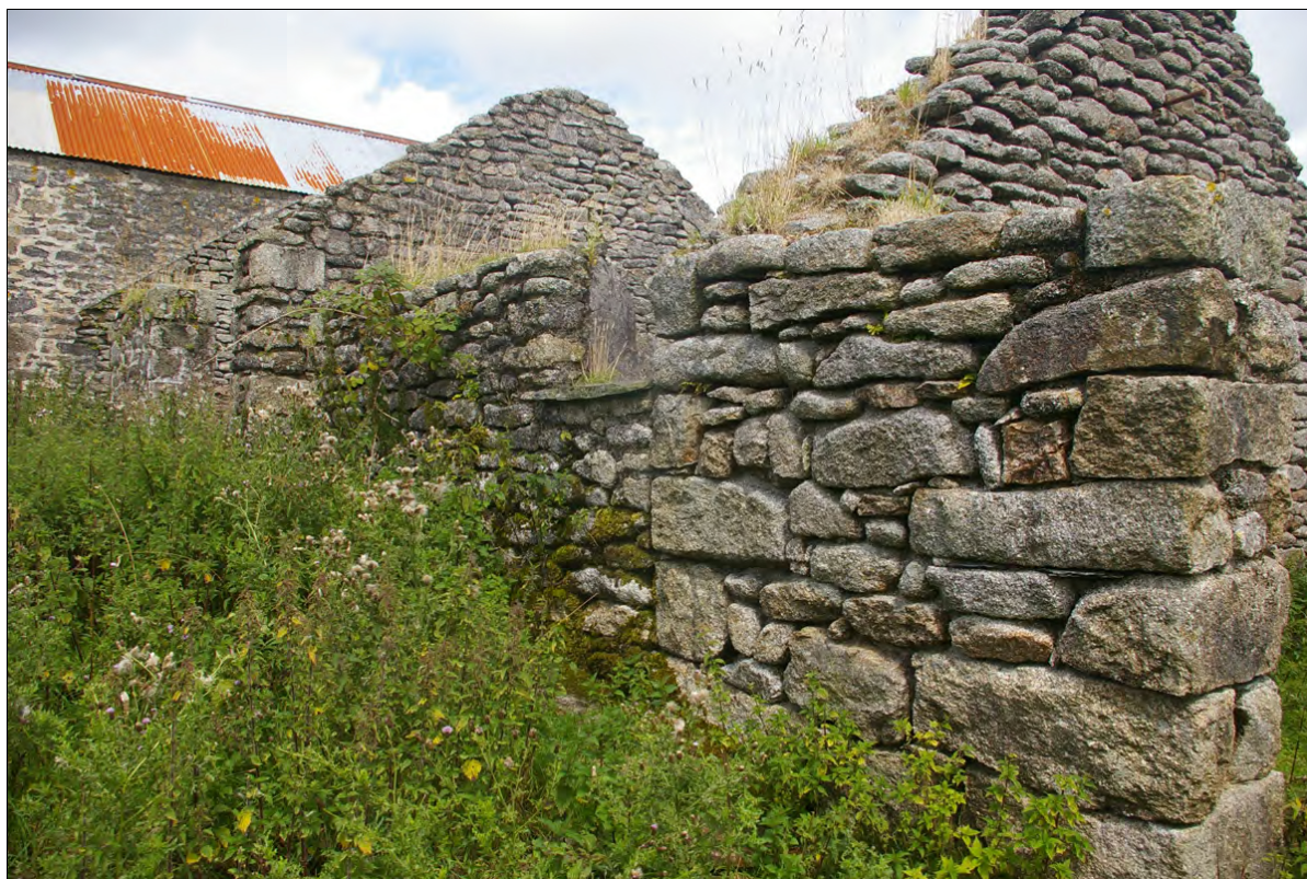
Figure 11: Shot of the west wall of Building 2b, showing how it is built up against the north gable of Building 2a; viewed from the south-west.
