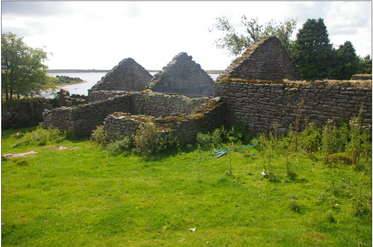
Building 2 viewed from the north-east.
