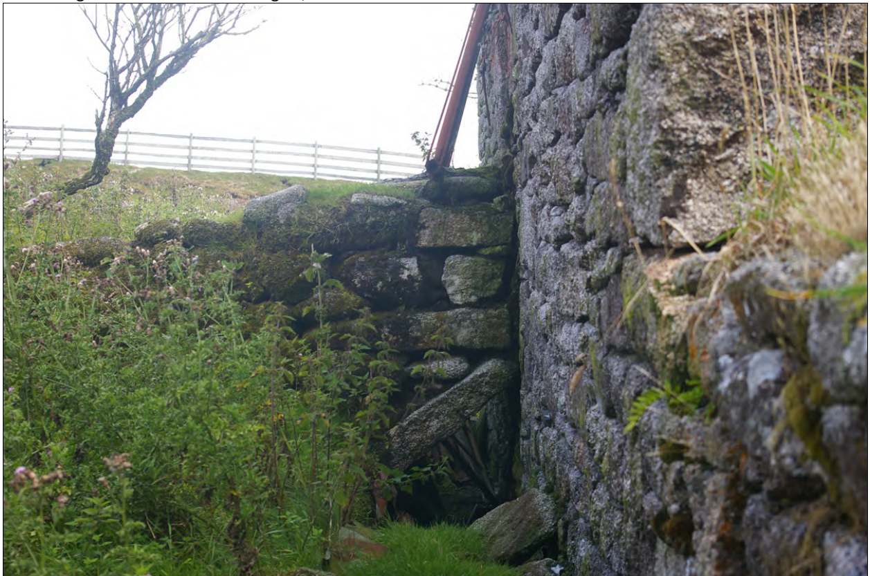
View of the granite slab 'bridge' across to the loading door in the north elevation of Building 1; from the west.
