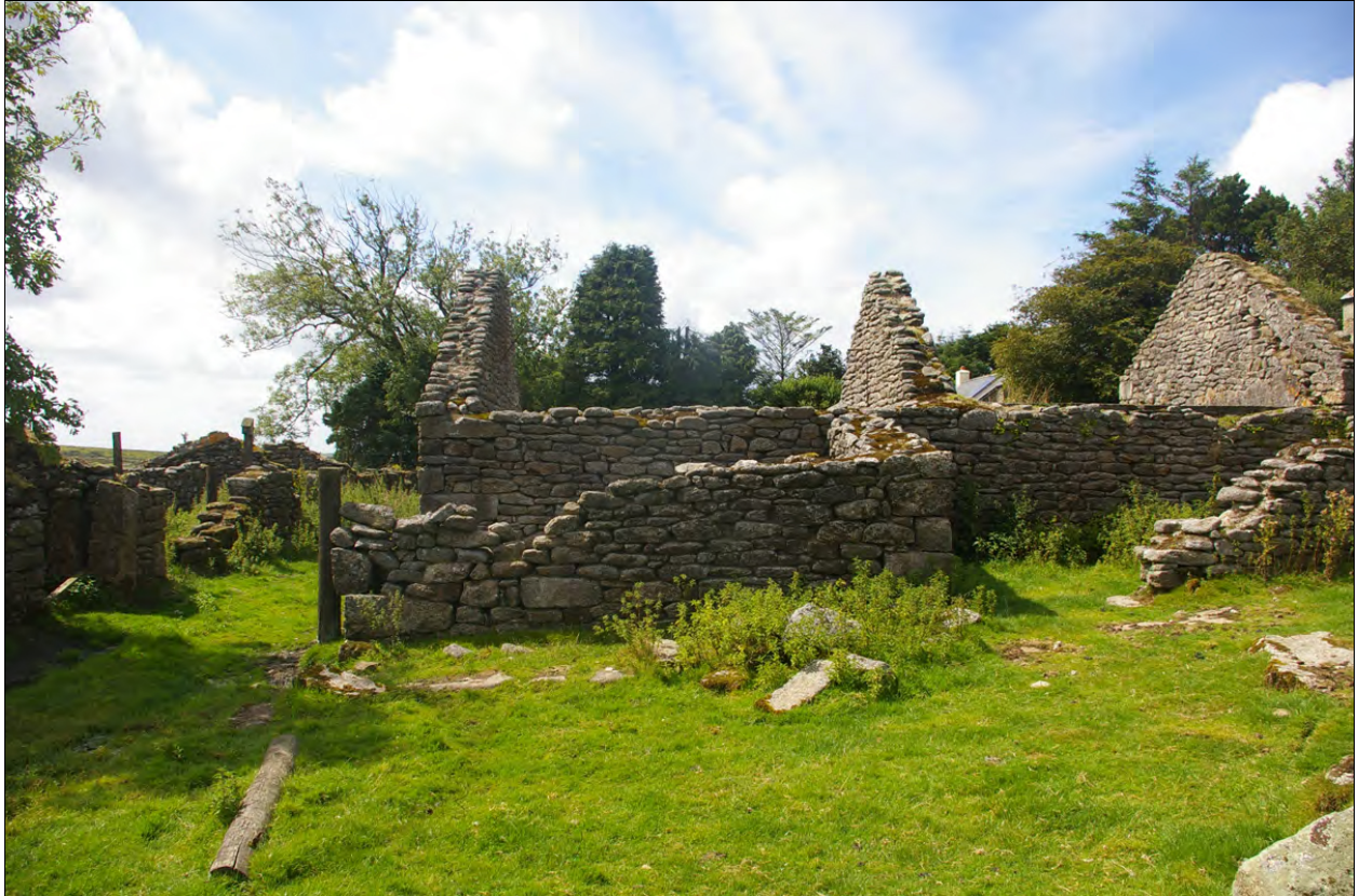
The east elevations of structures east of Building 2; viewed from the east.
