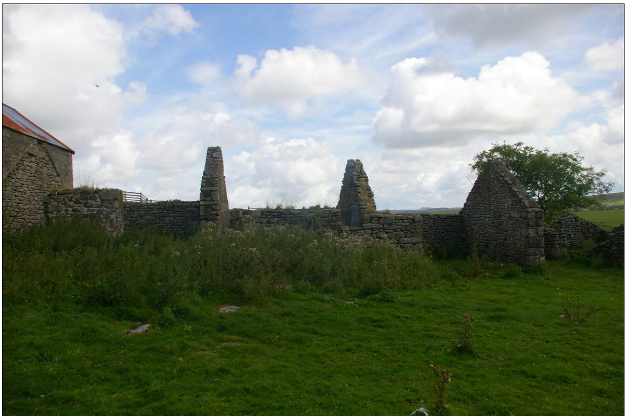
The west elevation of Building 2; from the west.
