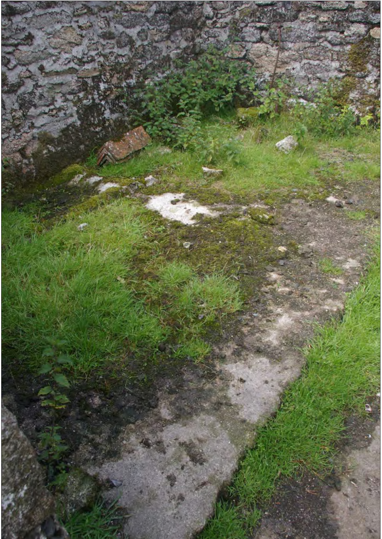
The remains of shallow concrete pens in the eastern compartment of Building 1a; from the south-east.
