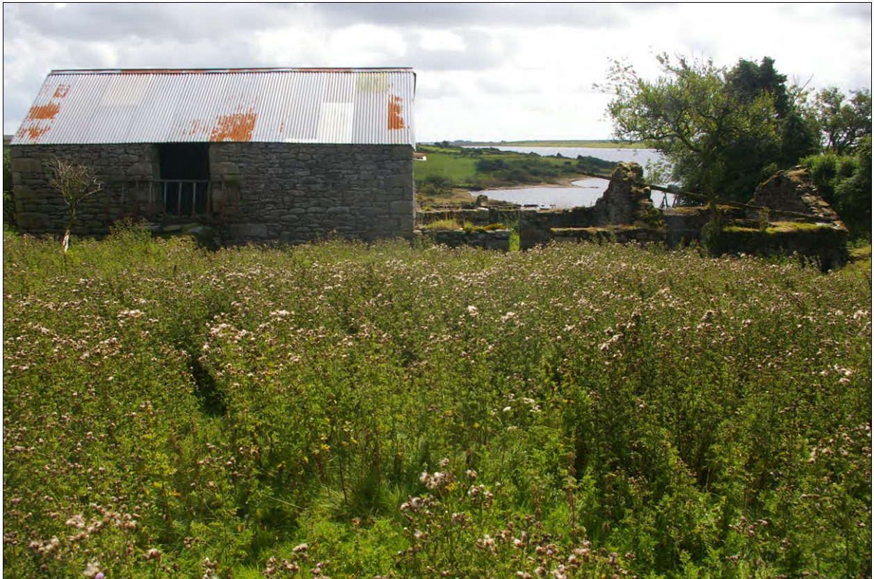
Building 1a and Building 1b; from the north.
