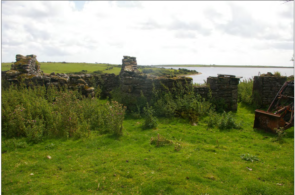
Figure 13: The north elevation of Buildings 3a and Building 3b; viewed from the north.
