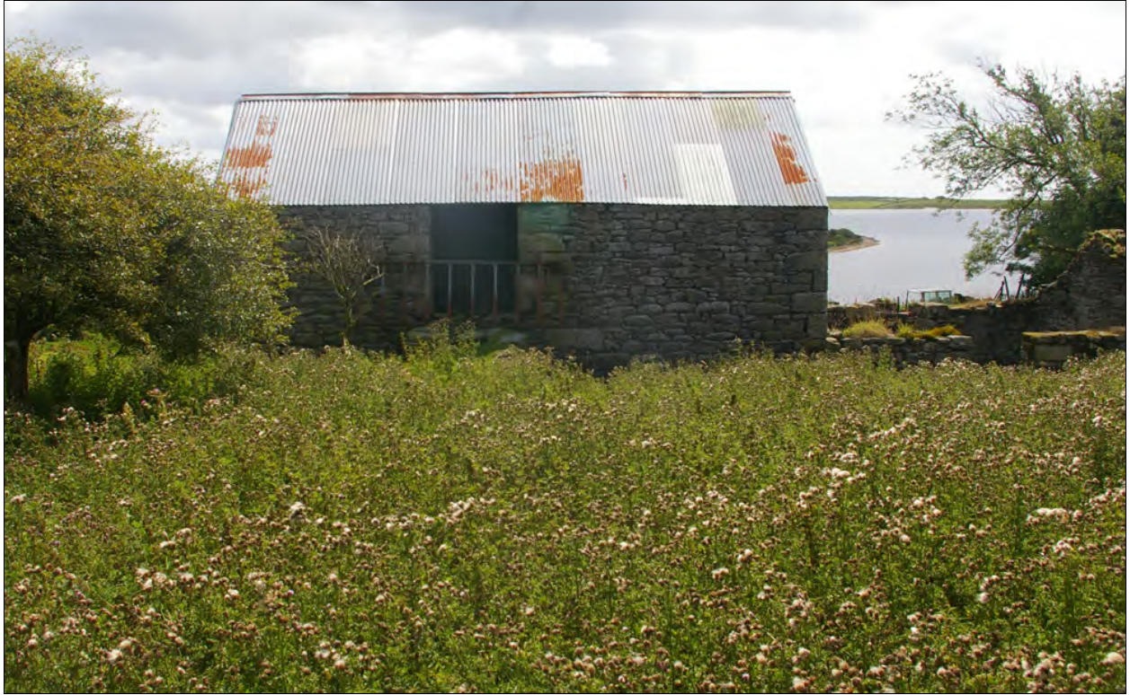
Building 1 from the north.
