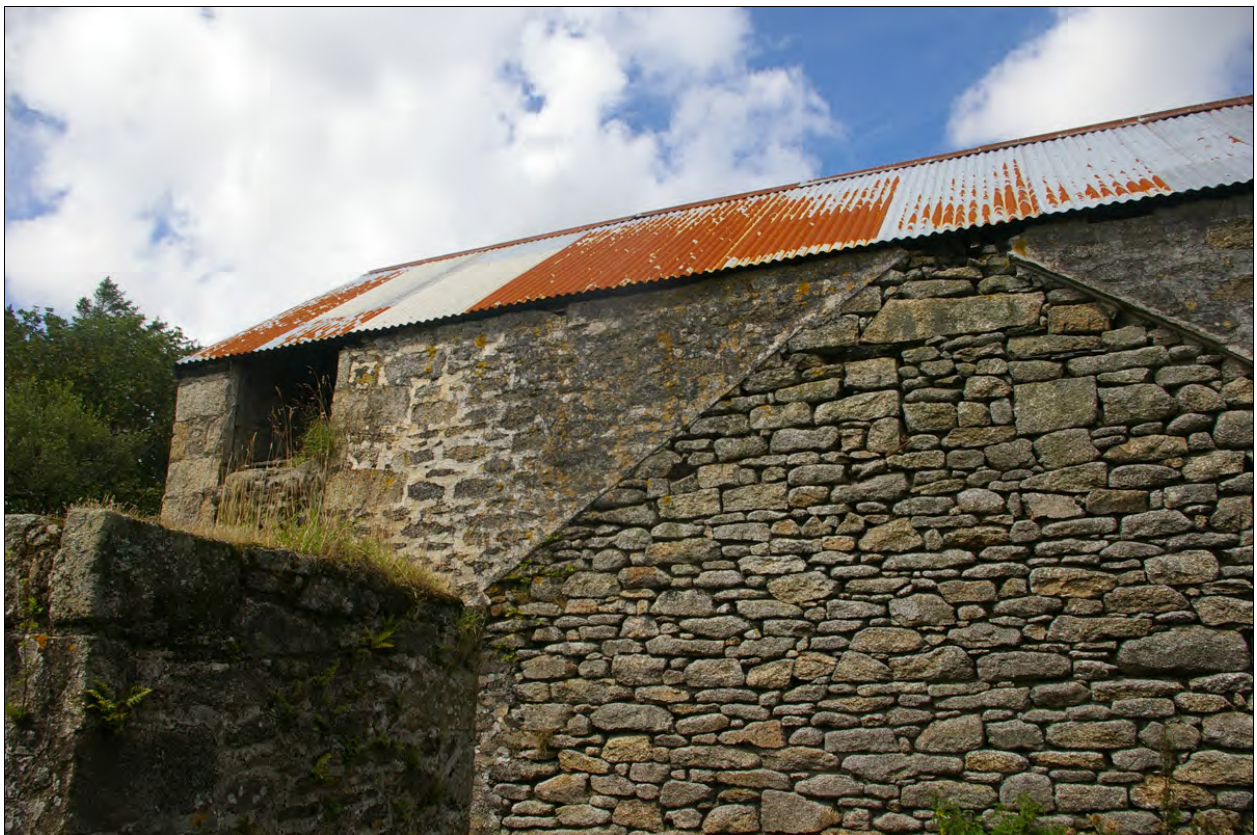
View across the south elevation of Building 1; from the south-east.
