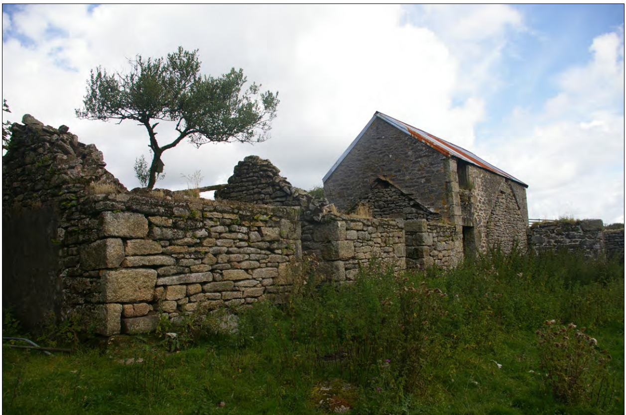
Building 1 and Building 1a, the south elevations; from the south-west.
