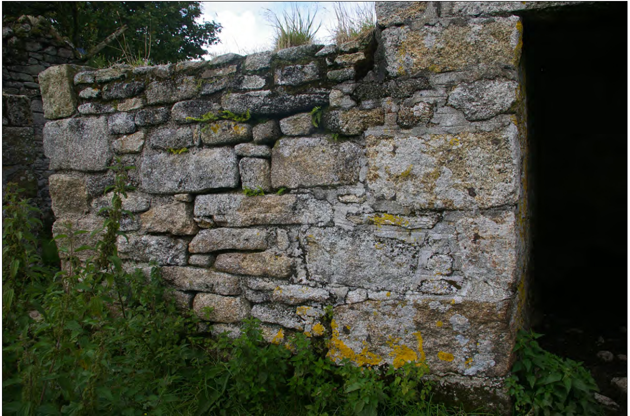
The adjoining buildings, Building 1 and Building 1a; from the south-east.
