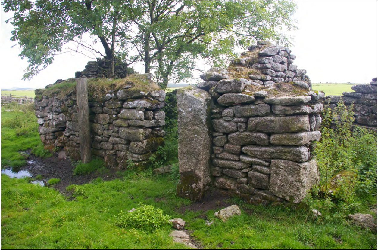
The north elevation of Building 3d; from the west, north-west.
