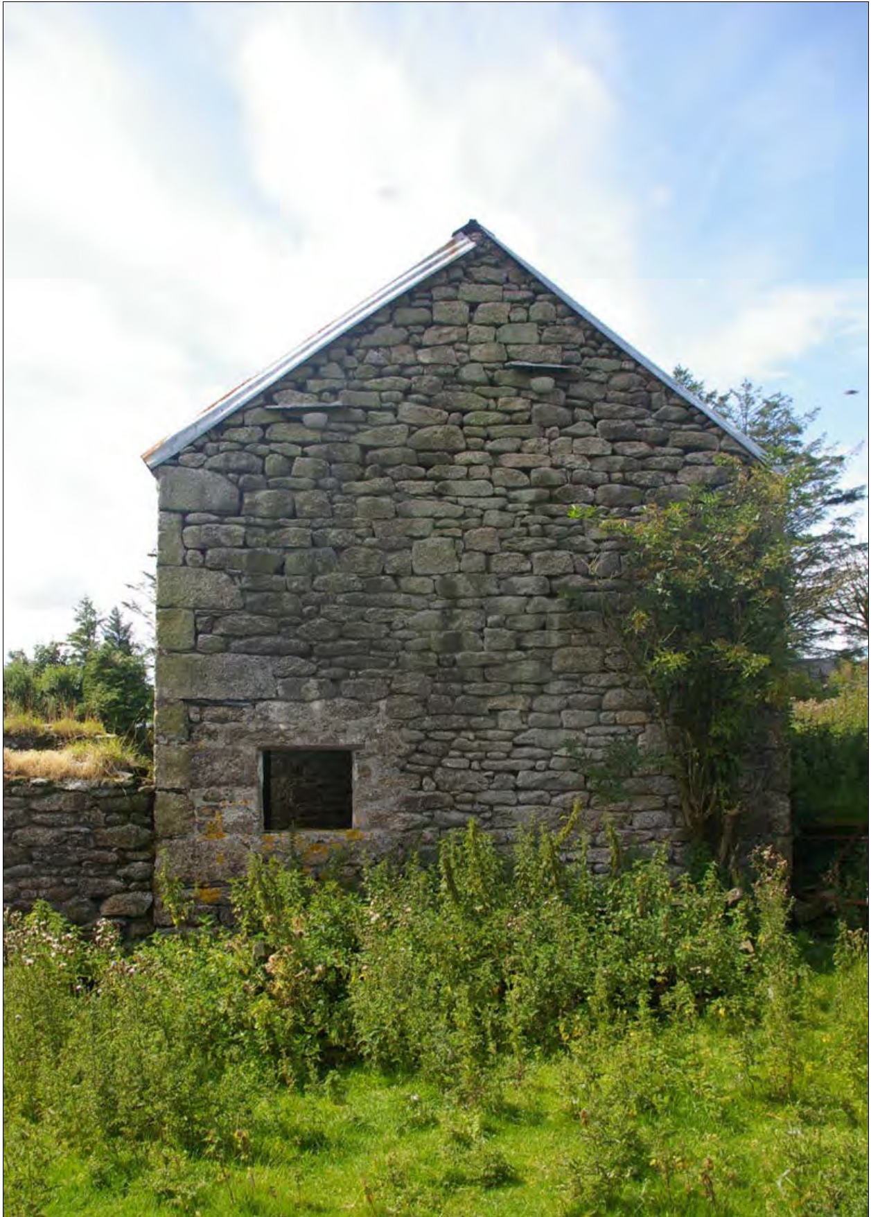
The east elevation of Building 1; from the east.
