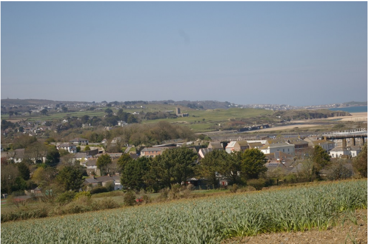
Detailed view across to the church of Lelant and towards St Ives; from the south-east.
