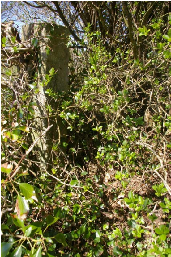
View of a granite gate pier, leading into the eastern of the two plots, from the field to the south; from the north-east.
