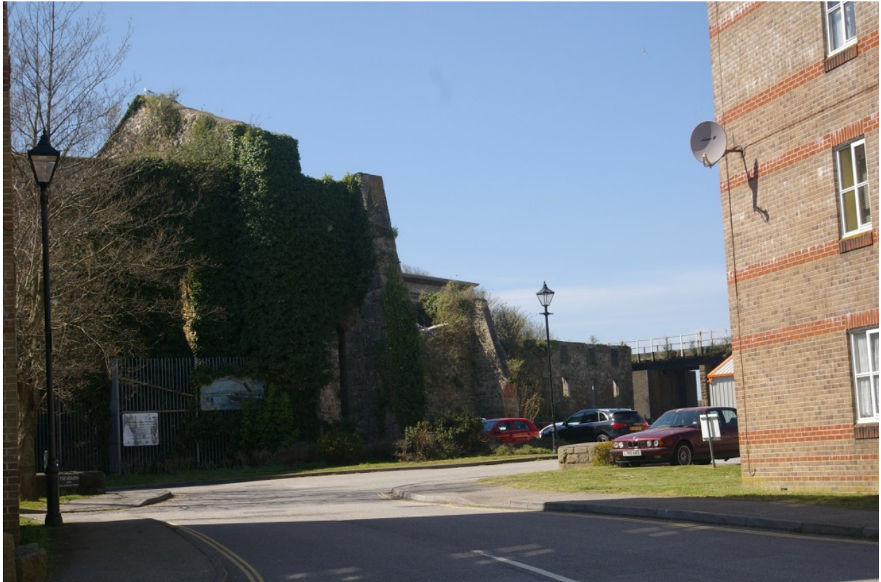
More stone industrial buildings to the north, behind Foundry square; from the south-east.
