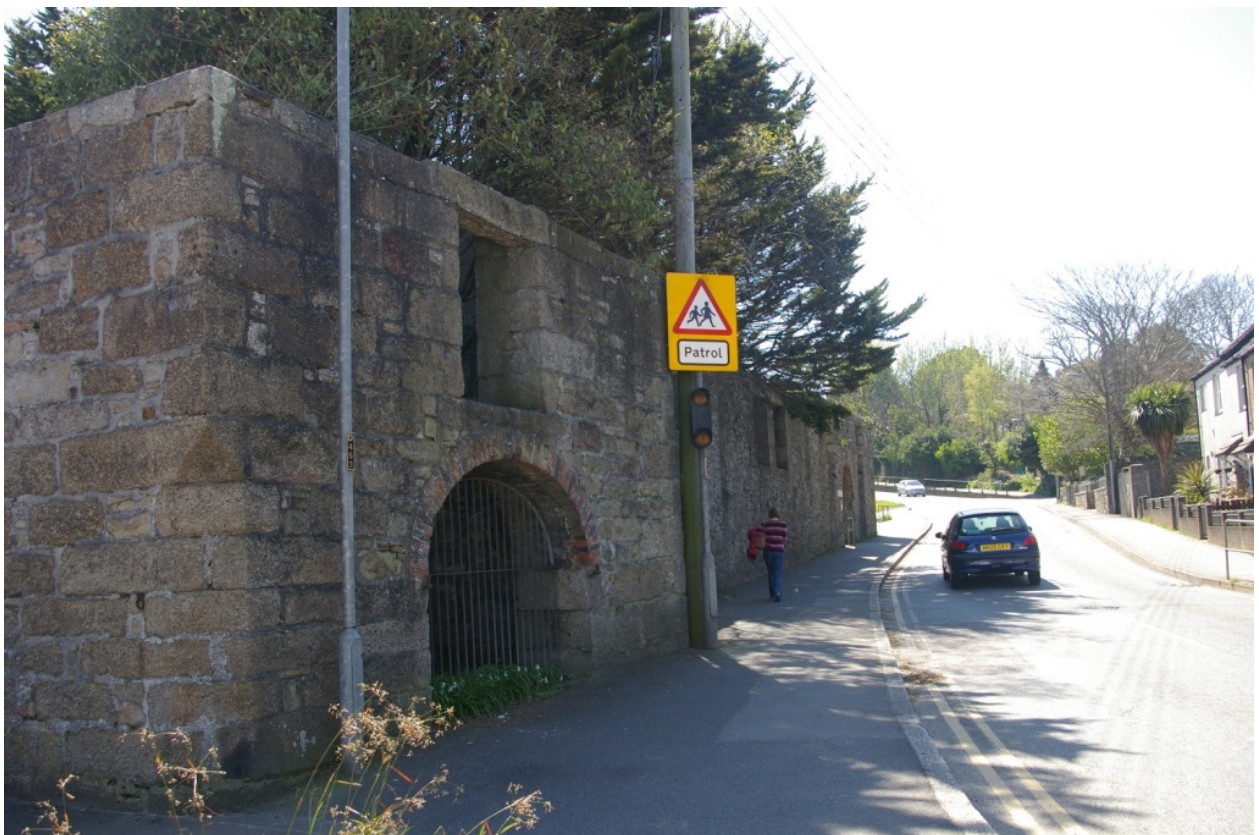
The frontage of the former mill building as it faces onto Foundry square and Foundry Hill; from the north-east.
