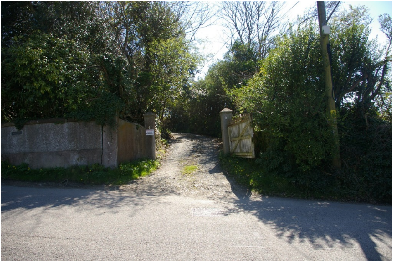
Gates leading onto St George's Road with curving flanking walls; from the north.
