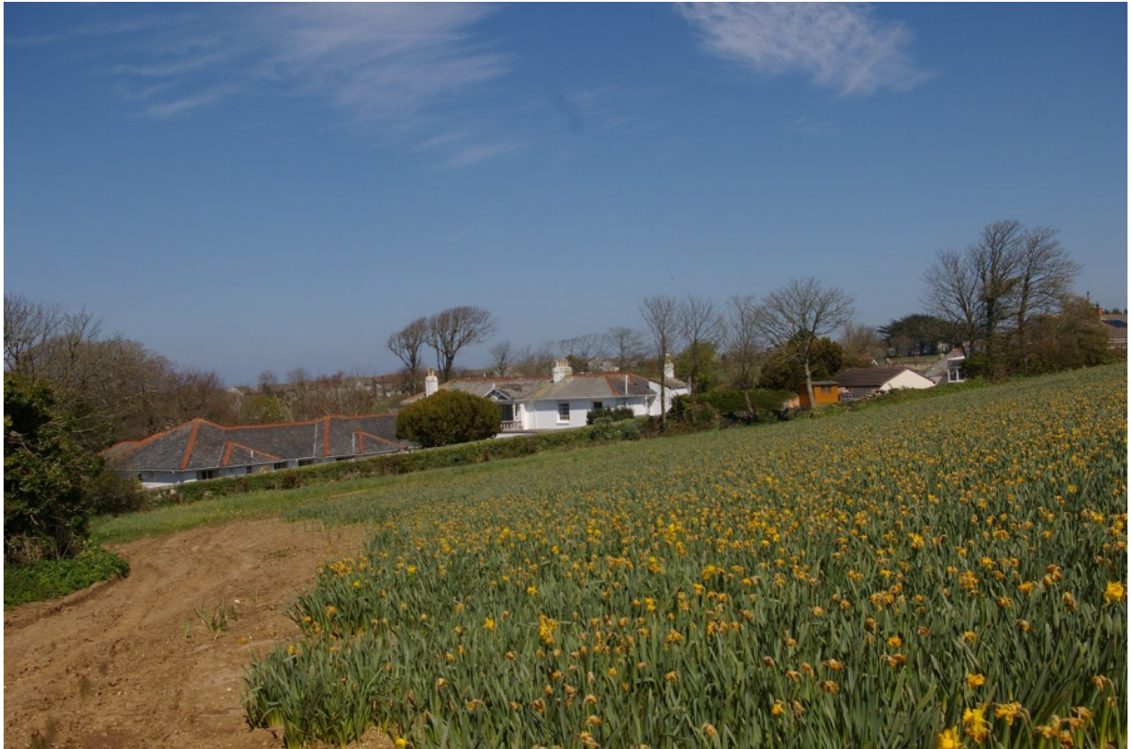
View to The Beeches and its single storey service wing; from the south-west.
