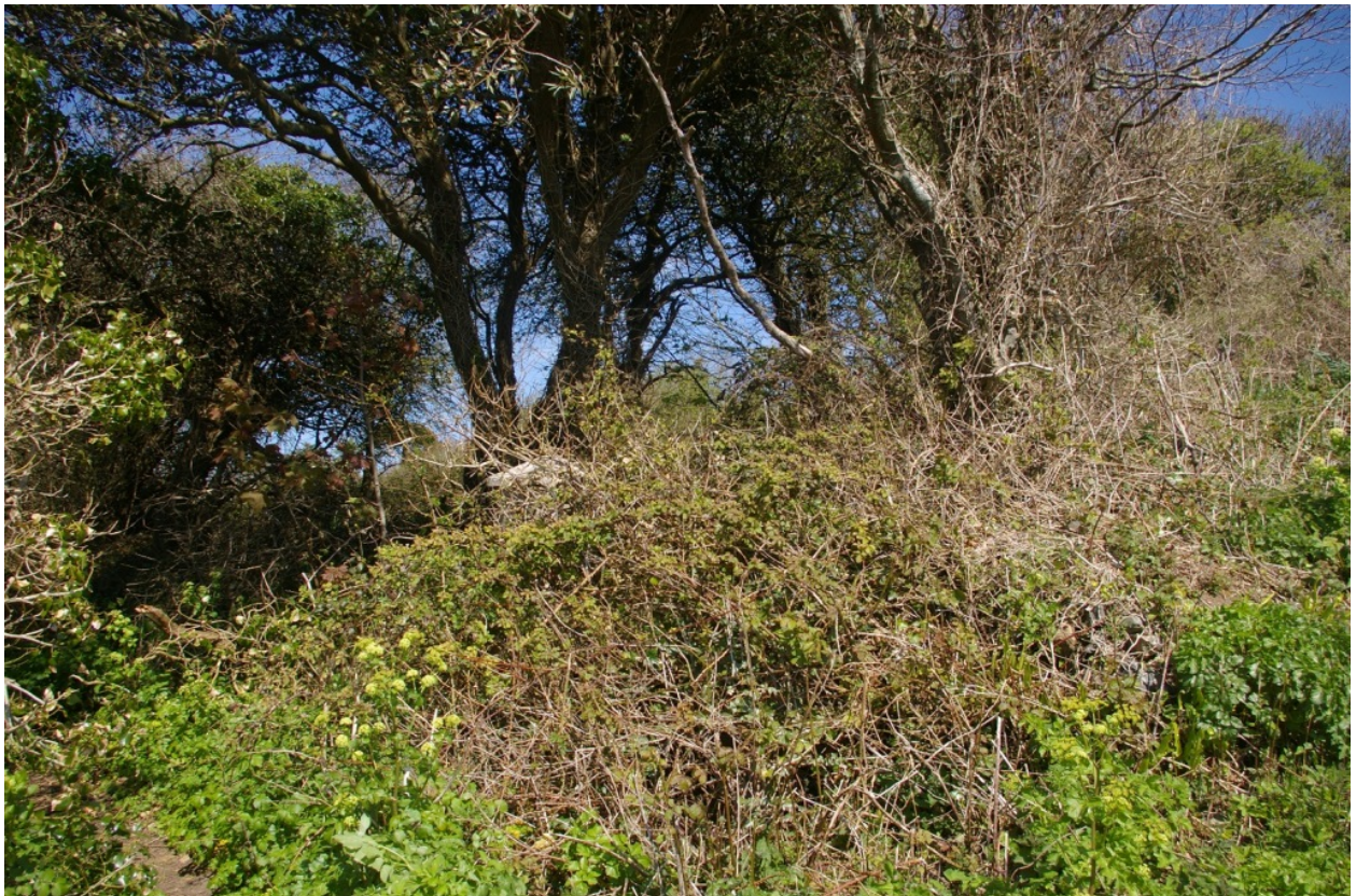
View of the entrance with gate piers into the eastern of the two overgrown plots; from the south-west.
