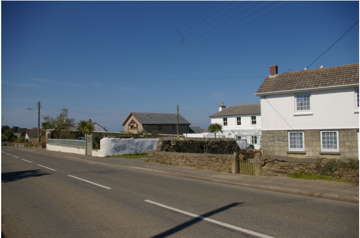
Views of the walls and houses associated with Wheal Alfred or Mellanear workings; from the south-west.
