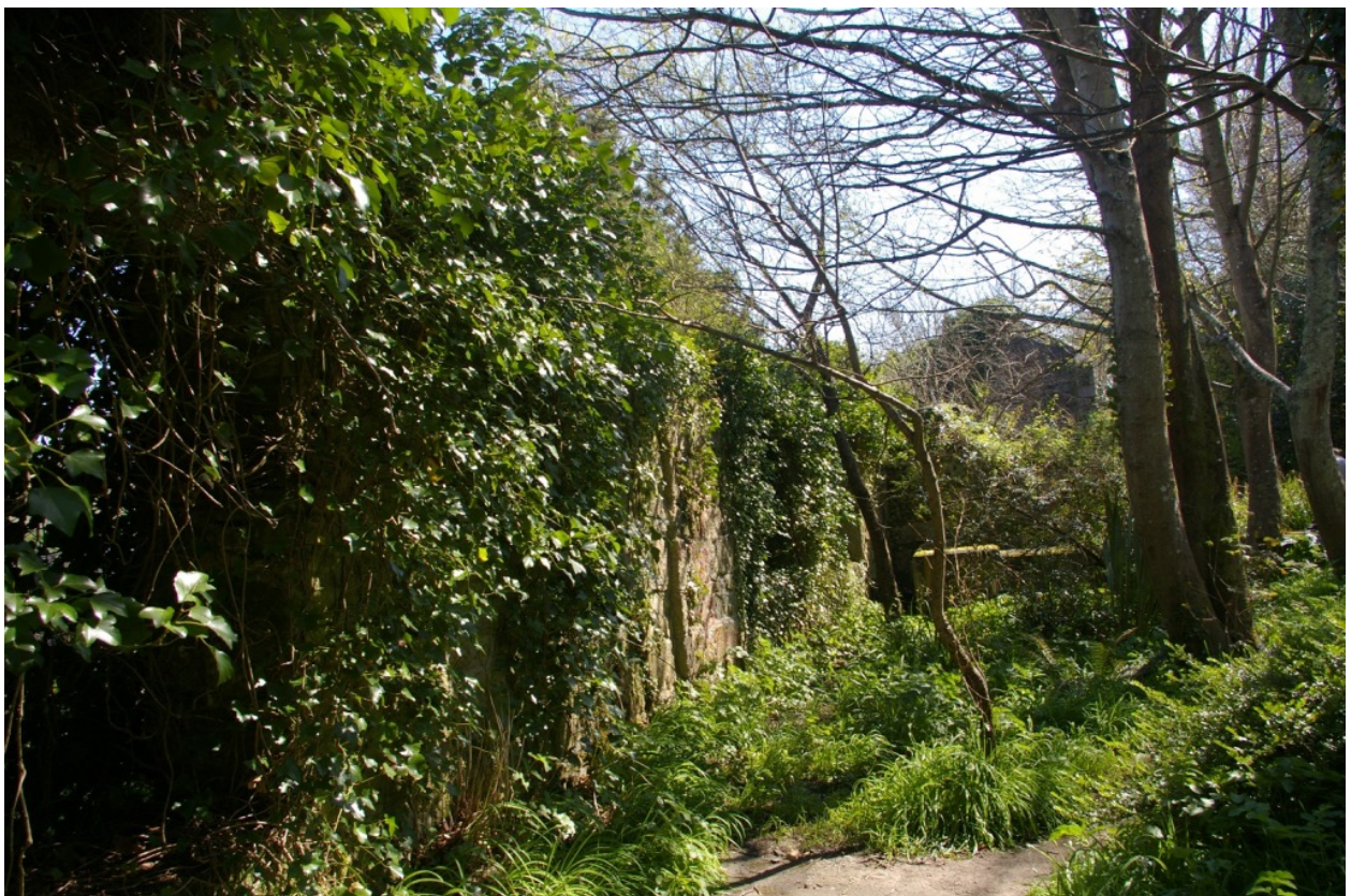
View of the long east walls of the ropeworks; from the north-west.
