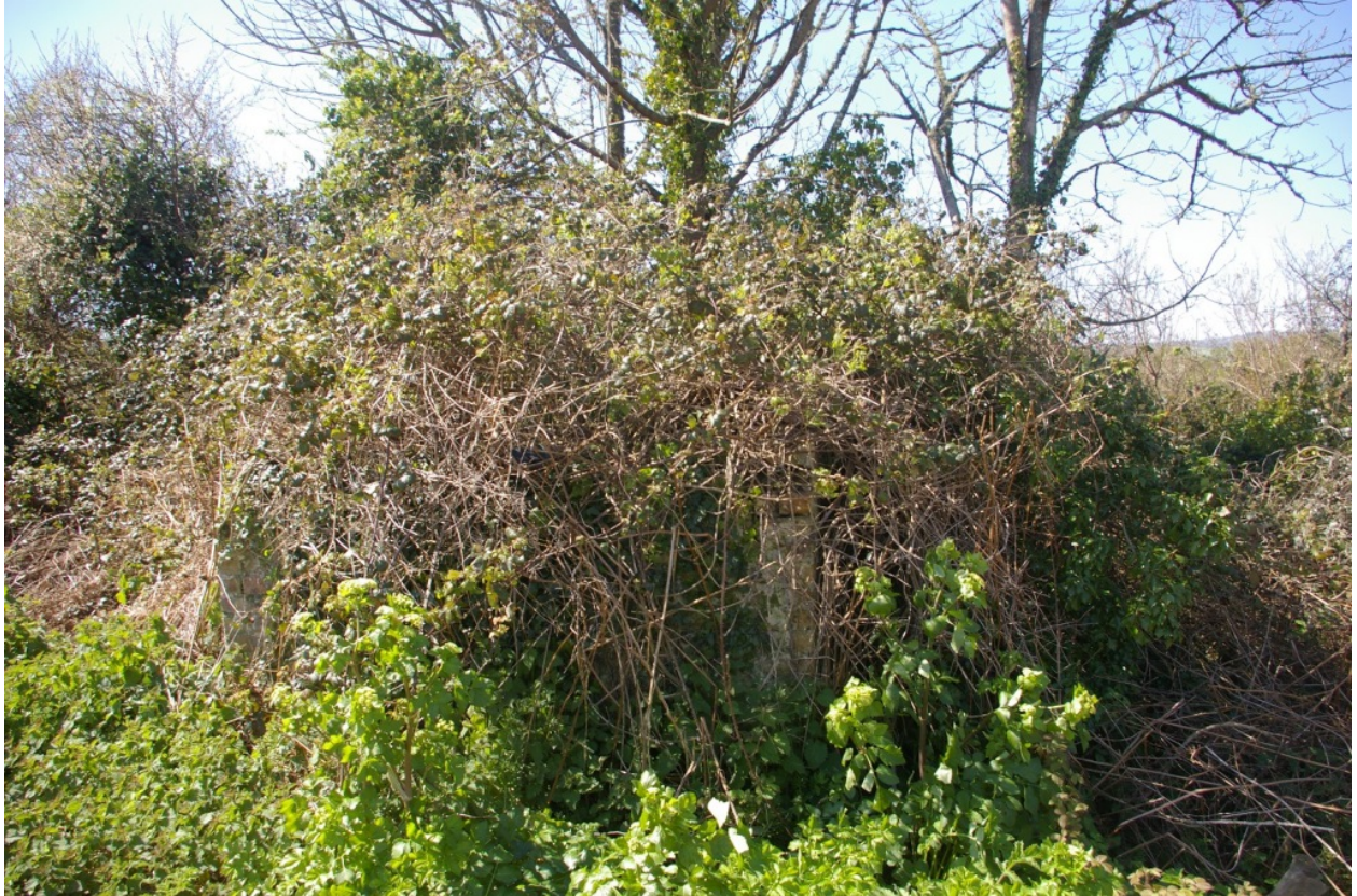
View of the enclosed northern section of the building range; from the north-east.
