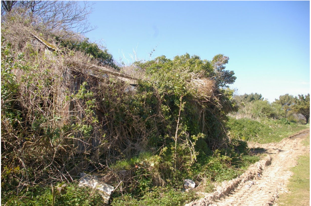
The upstanding timber and corrugated iron building; from the south-east.
