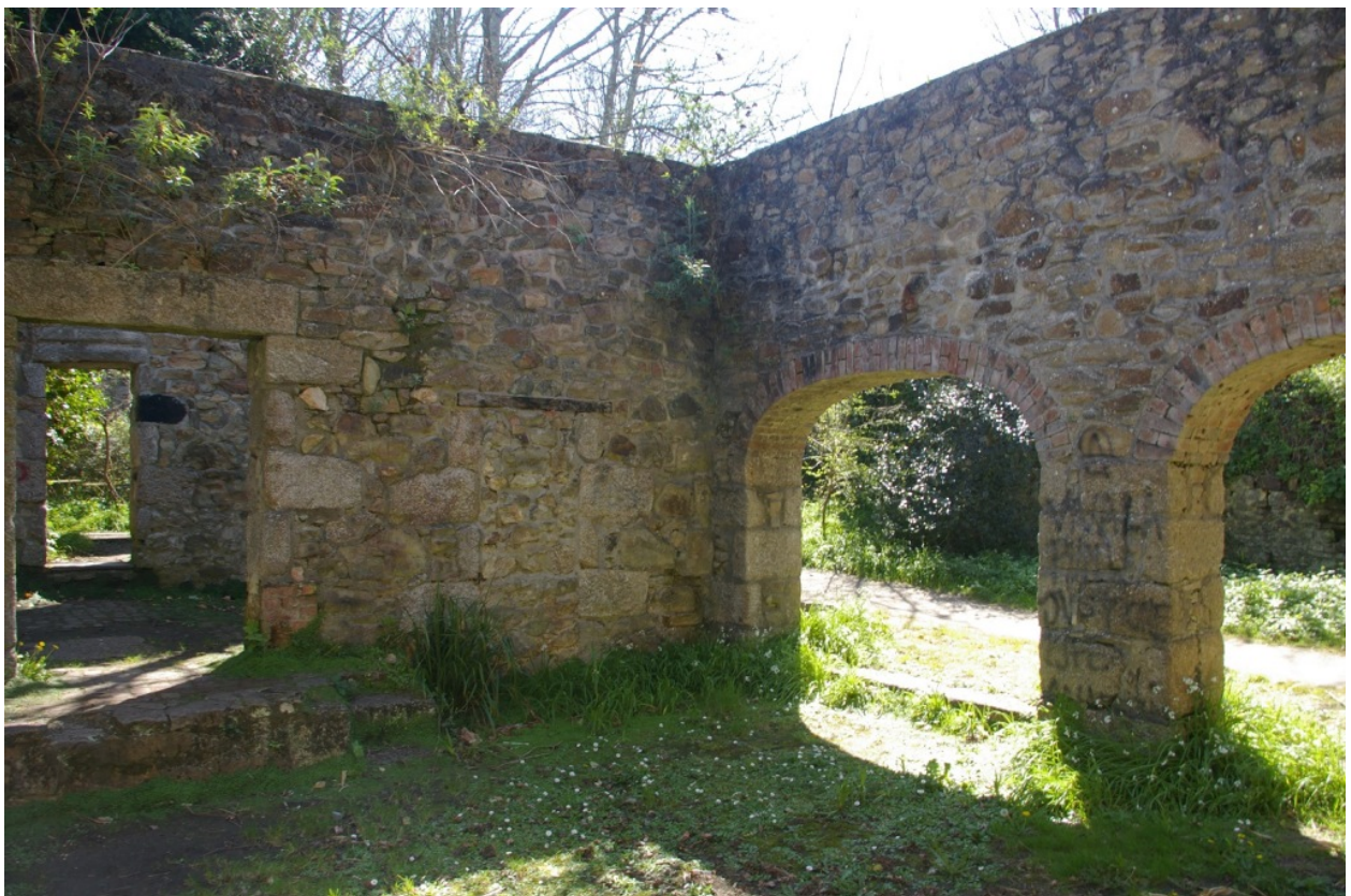
The west side of the rope works; from the north-east.
