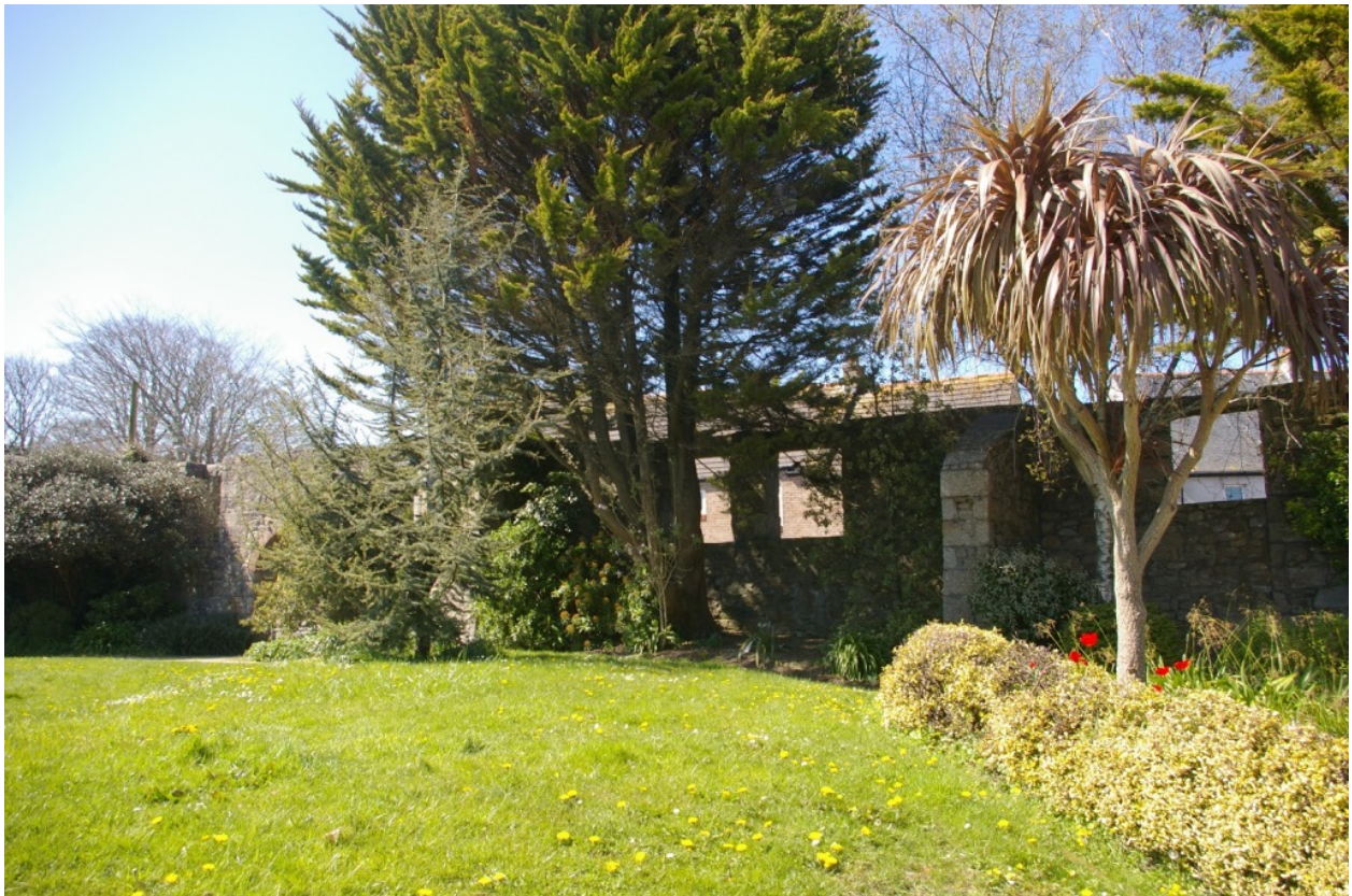
View of the west side of the mill building; from the north-east.
