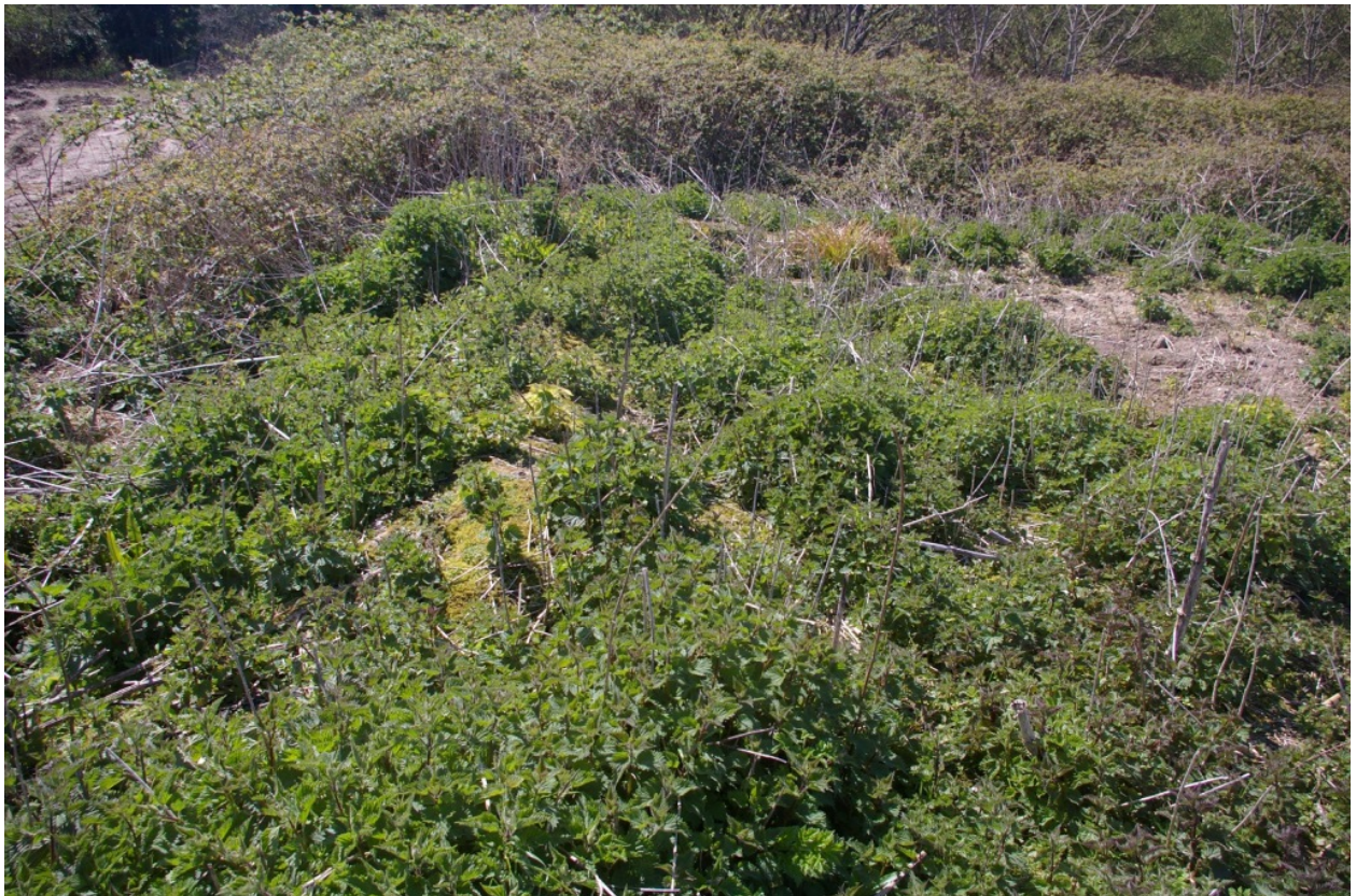
L-shaped structure which may be the foundations of a building; from the east, north-east.
