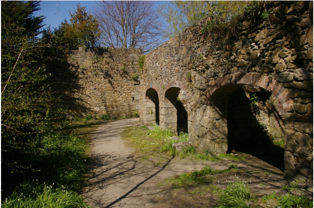
View of the northern end of the ropeworks; from the south-west.
