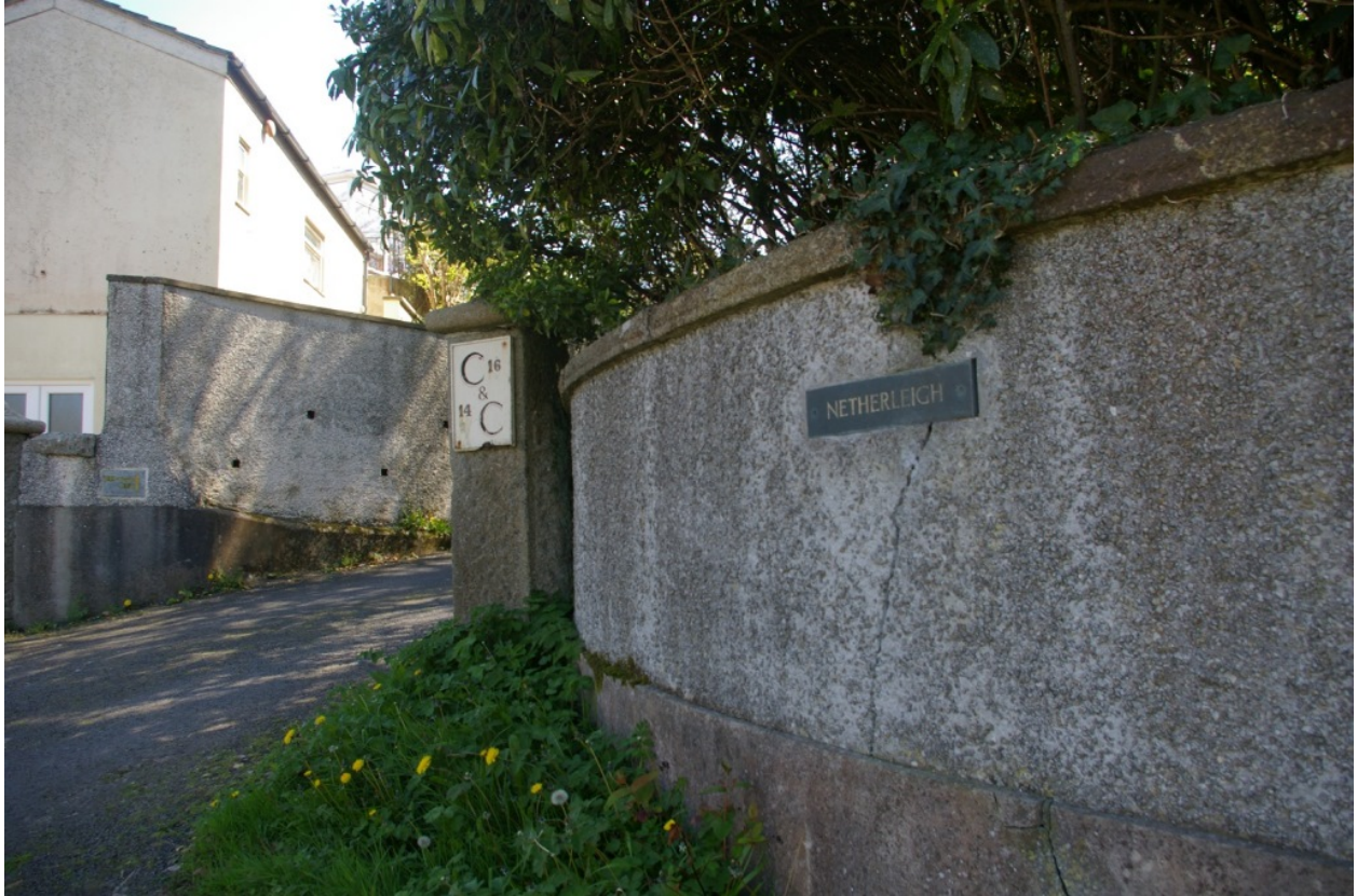
Detail of entrance to Netherleigh; from the north-west.
