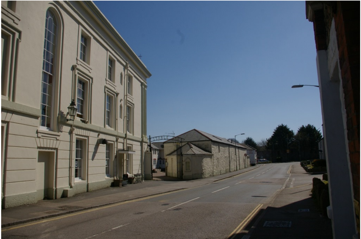
The stables and service courtyards behind the White Hart Hotel; from the north-west.
