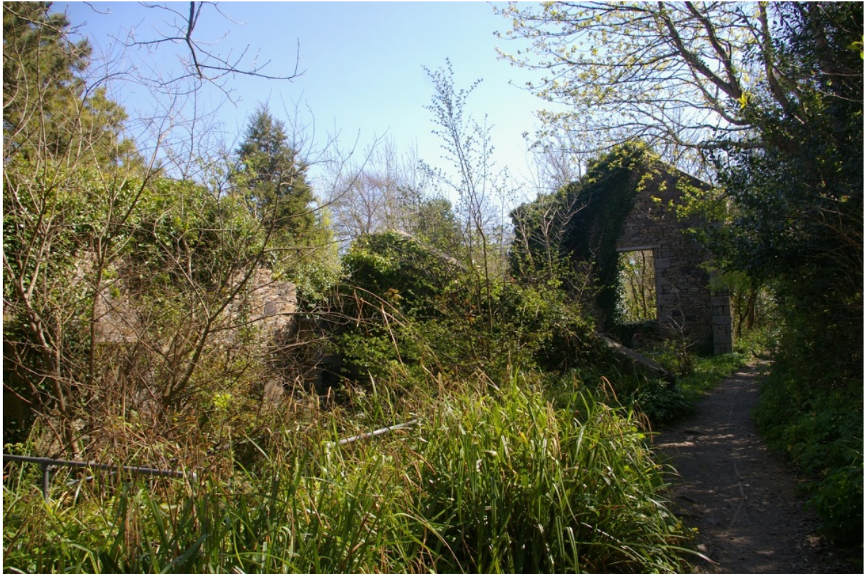
View down the ropeworks, to the southern gable; from the north-west.
