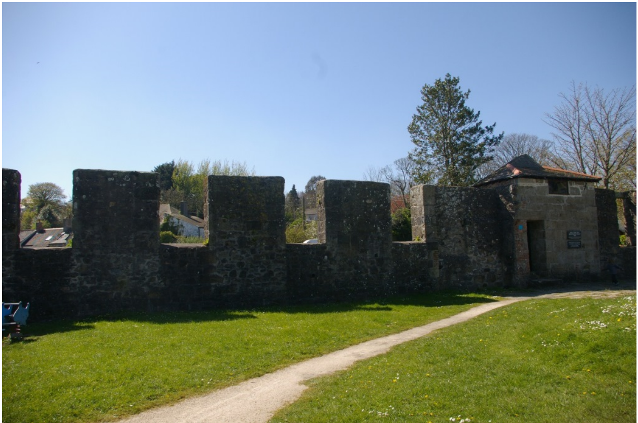
The west walls of the mill building; from the south-east.
