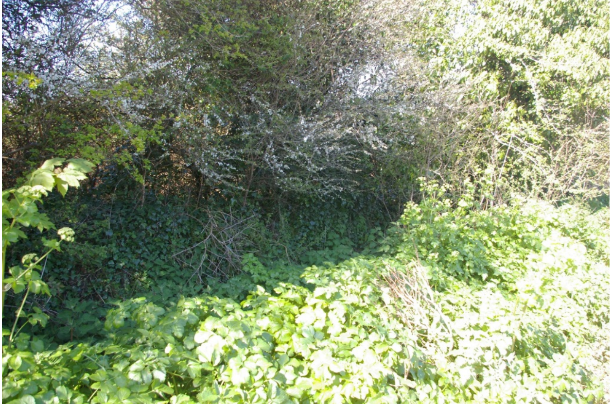
View to the overgrown hedgebank which forms the western boundary of this building, up against which the buildings are built; from the south-east.
