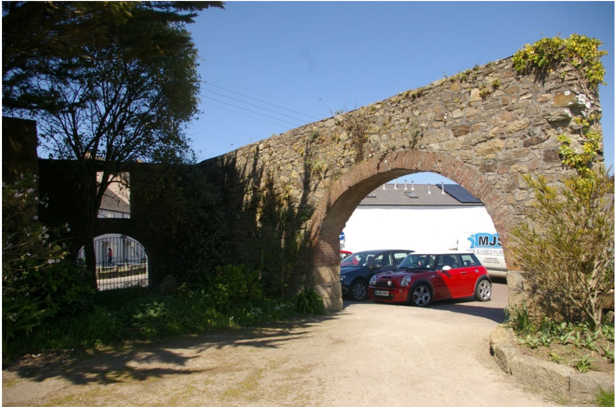
View of the south side of the mill frontage; from the south-west.
