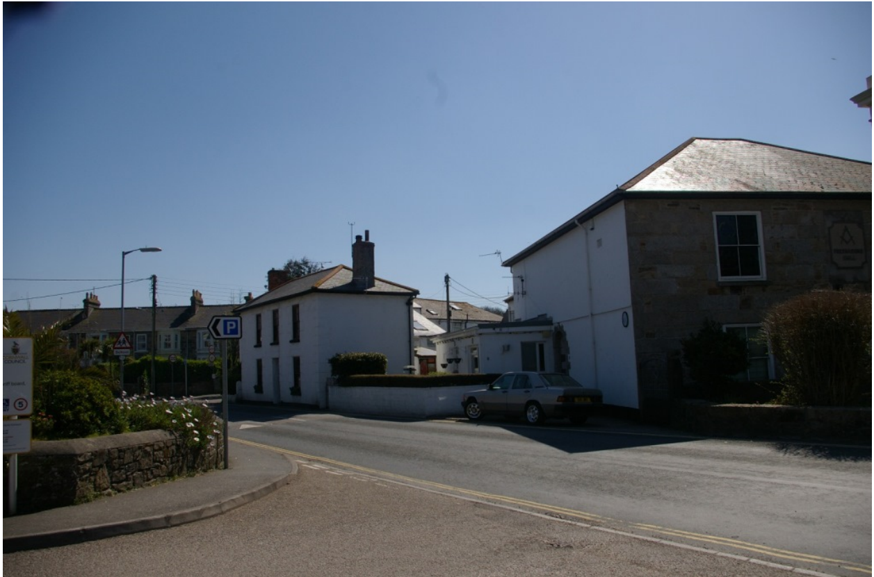
Showing the local blocking to the Freemasons Hall, which backs onto the service courtyards; from the north-east.
