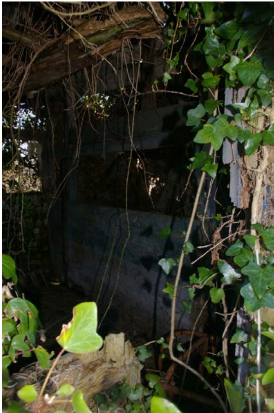
View into the building; from the south-east.
