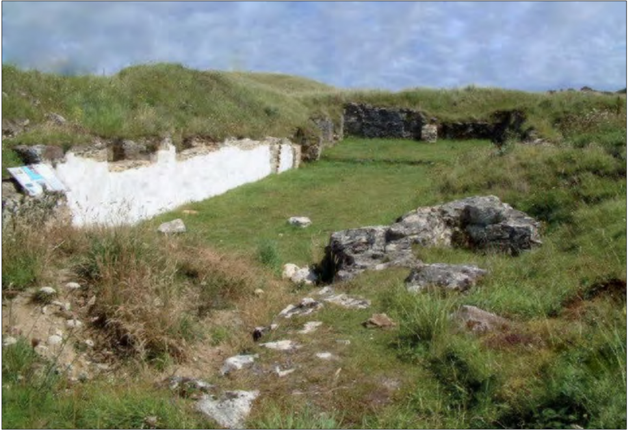
St Piran's Church within the sand dunes; from the south-west.
