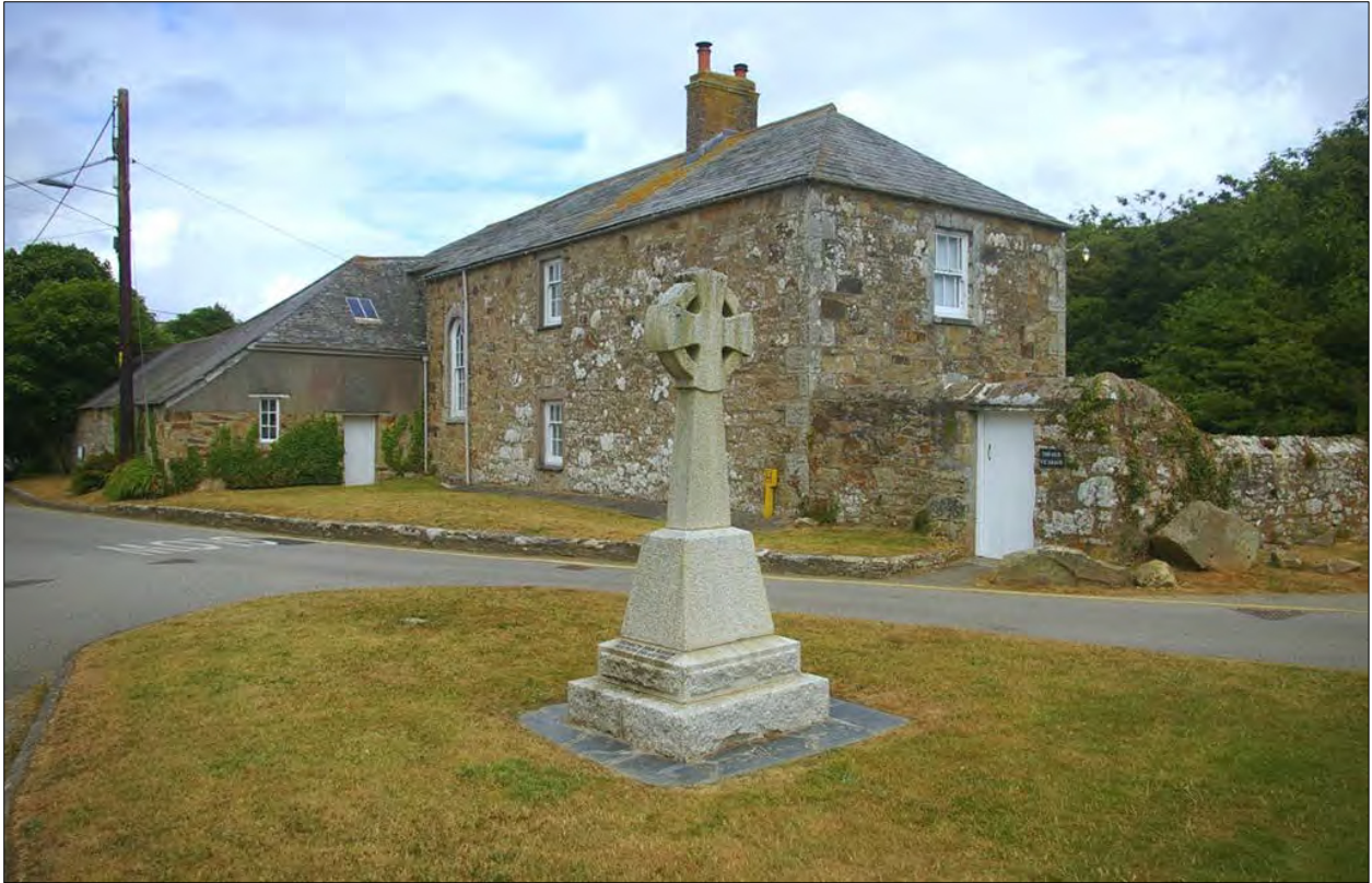
The Old Vicarage and walled gardens and war memorial on the small village green in Cubert; form the south-west.
