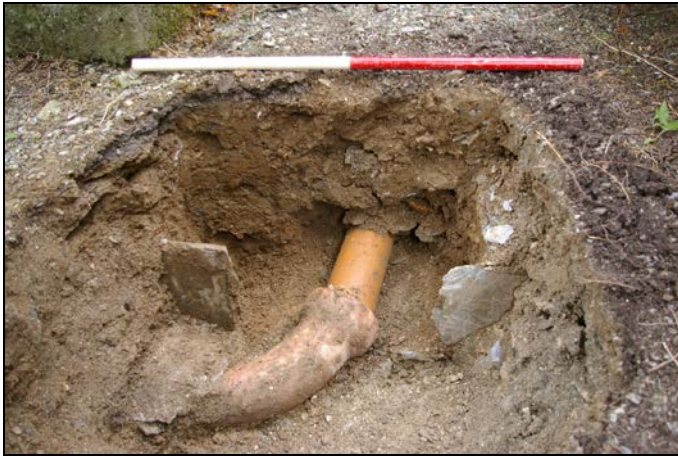
Figure 1: Test Pit 1; viewed from the south (1m scale).
