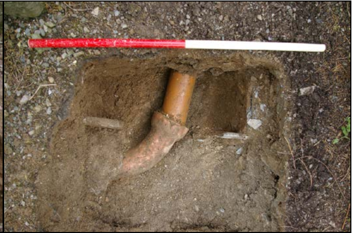
Figure 4: Test Pit 1; viewed from above (1m scale).
