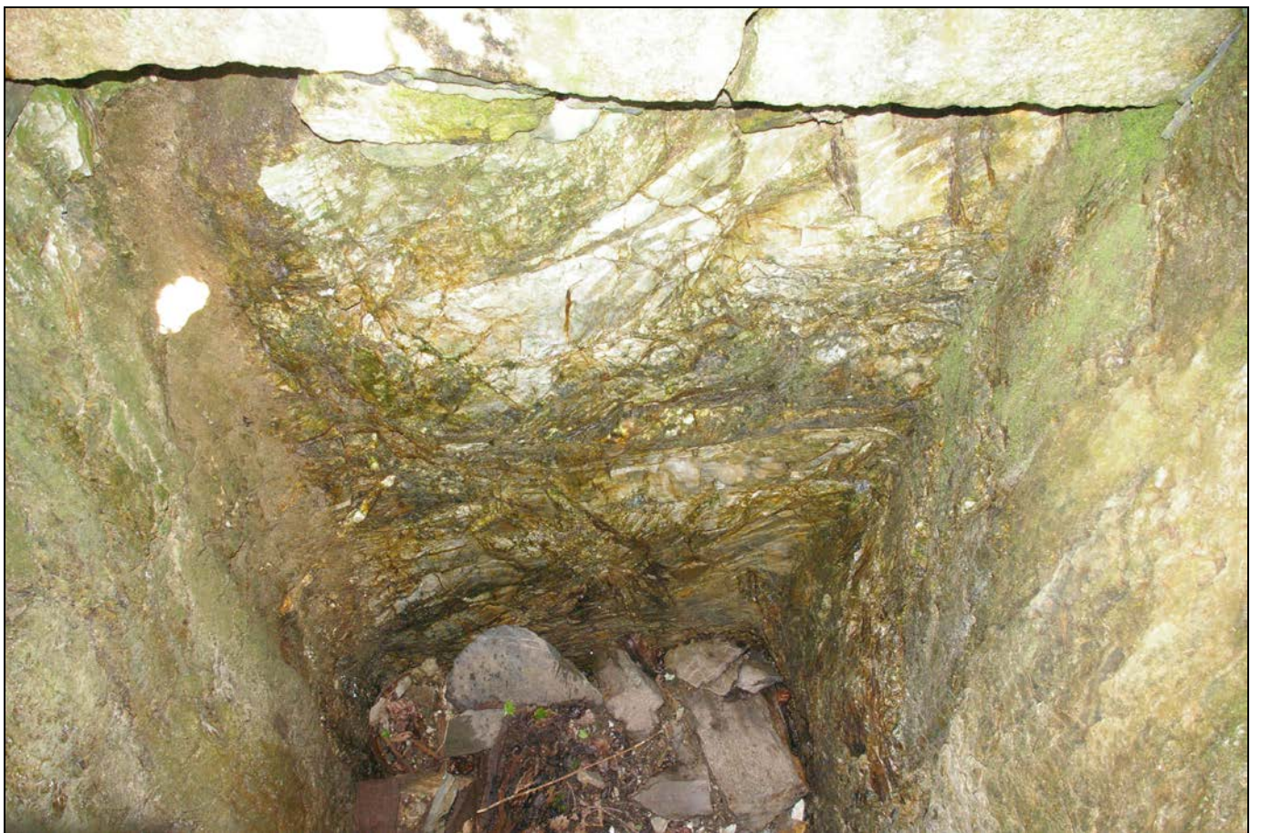
Figure 9: View down into the well; viewed from the south-west.
