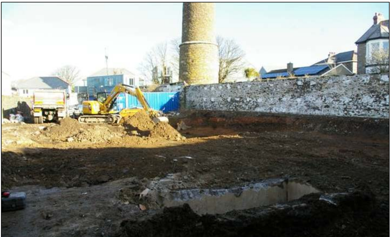
Figure 4: Site post-excavation, viewed from the south-west corner; looking north-east (no scale).
