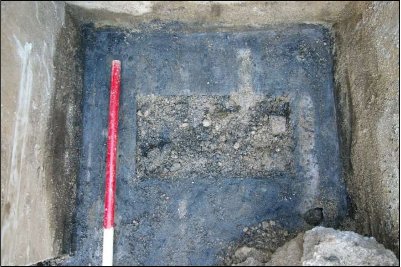
Figure 13: Drain at the west end of the concrete structure; viewed from above and to the east (partial 1m scale).
