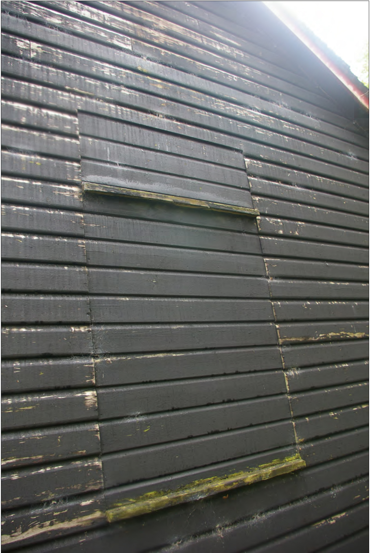
Detail of the blocked window opening in the north-east elevation; from the east.
