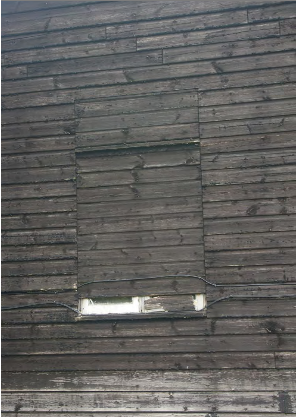
Detail of the blocked window opening in the south-west elevation; from the south-south-west.
