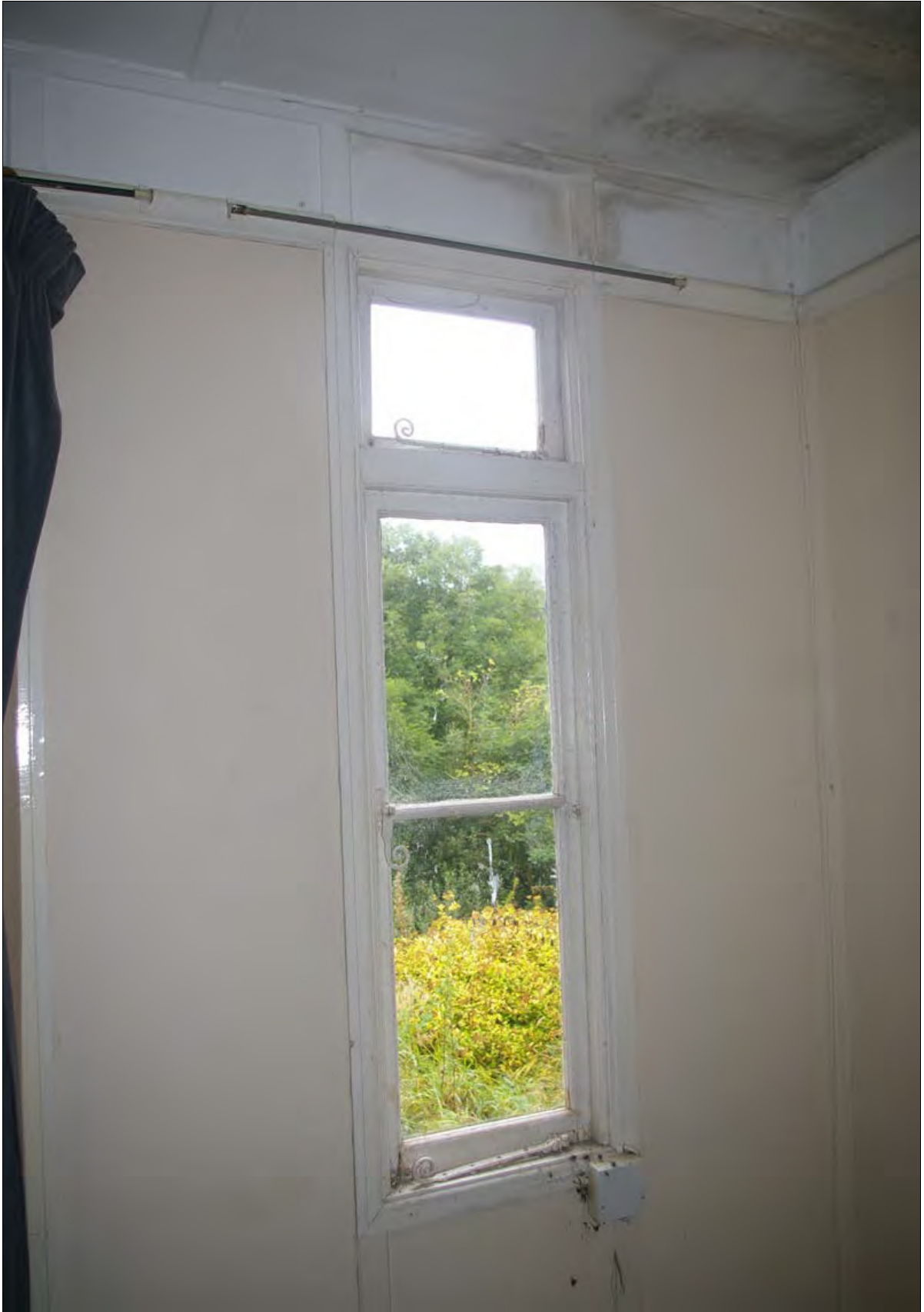
Detail of the narrow window, south of the front door, showing a two pane casement and upper hopper single pane casement, with scroll detail latches; from the north, north-east.
