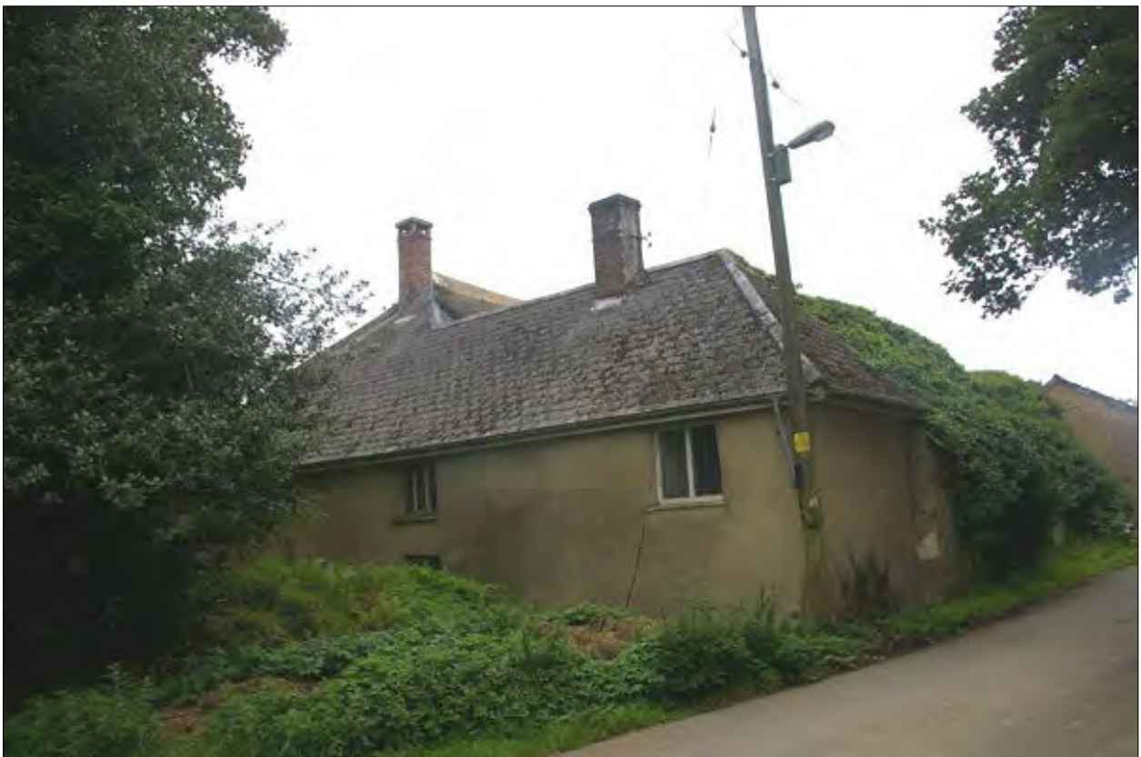
The Barton in Spreyton; from the north-east.
