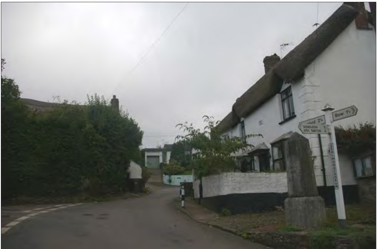
Cottages within Zeal Monachorum, of typical Devon vernacular; from the south, south-west.
