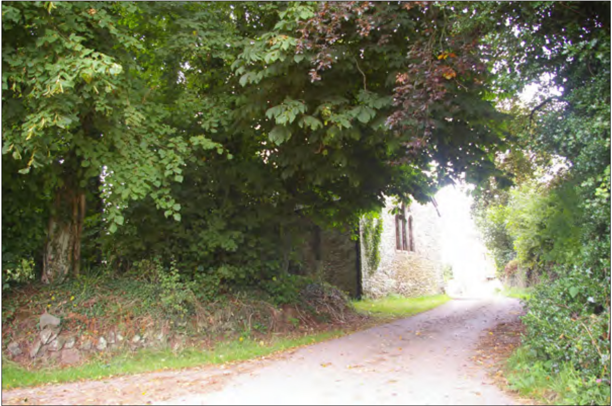
The former chapel at Hampson; from the south-east.
