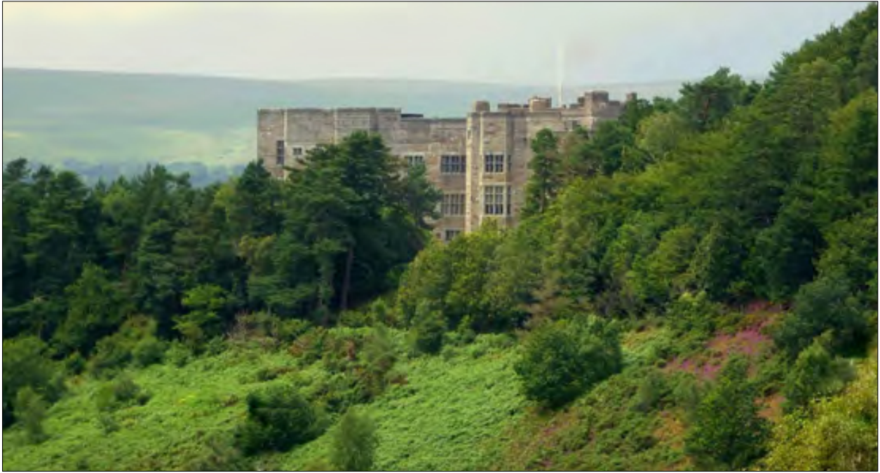
View along the gorge to Castle Drogo; from the north.
