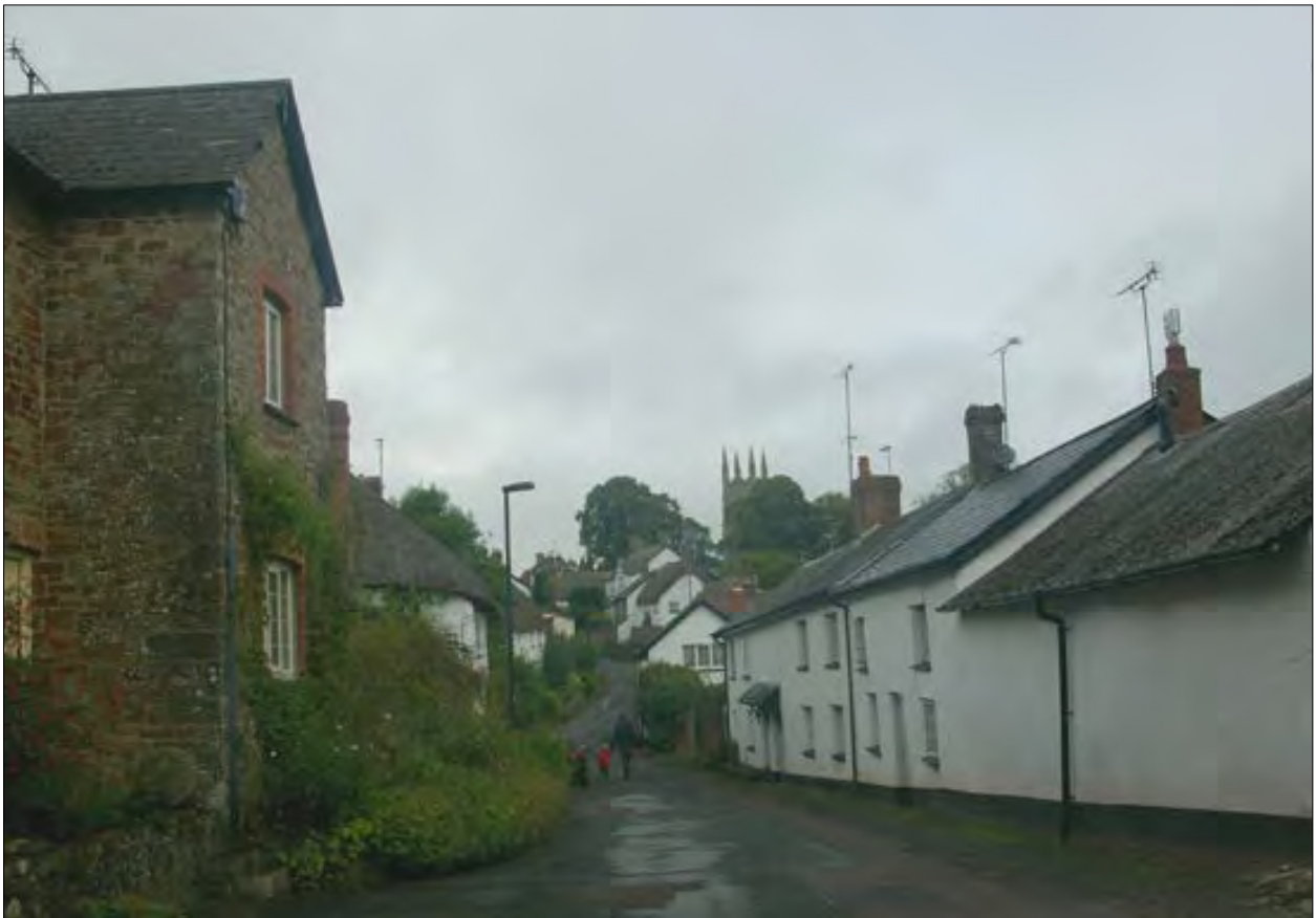
View up the main street in the conservation area of Sampford Courtenay; from the south.
