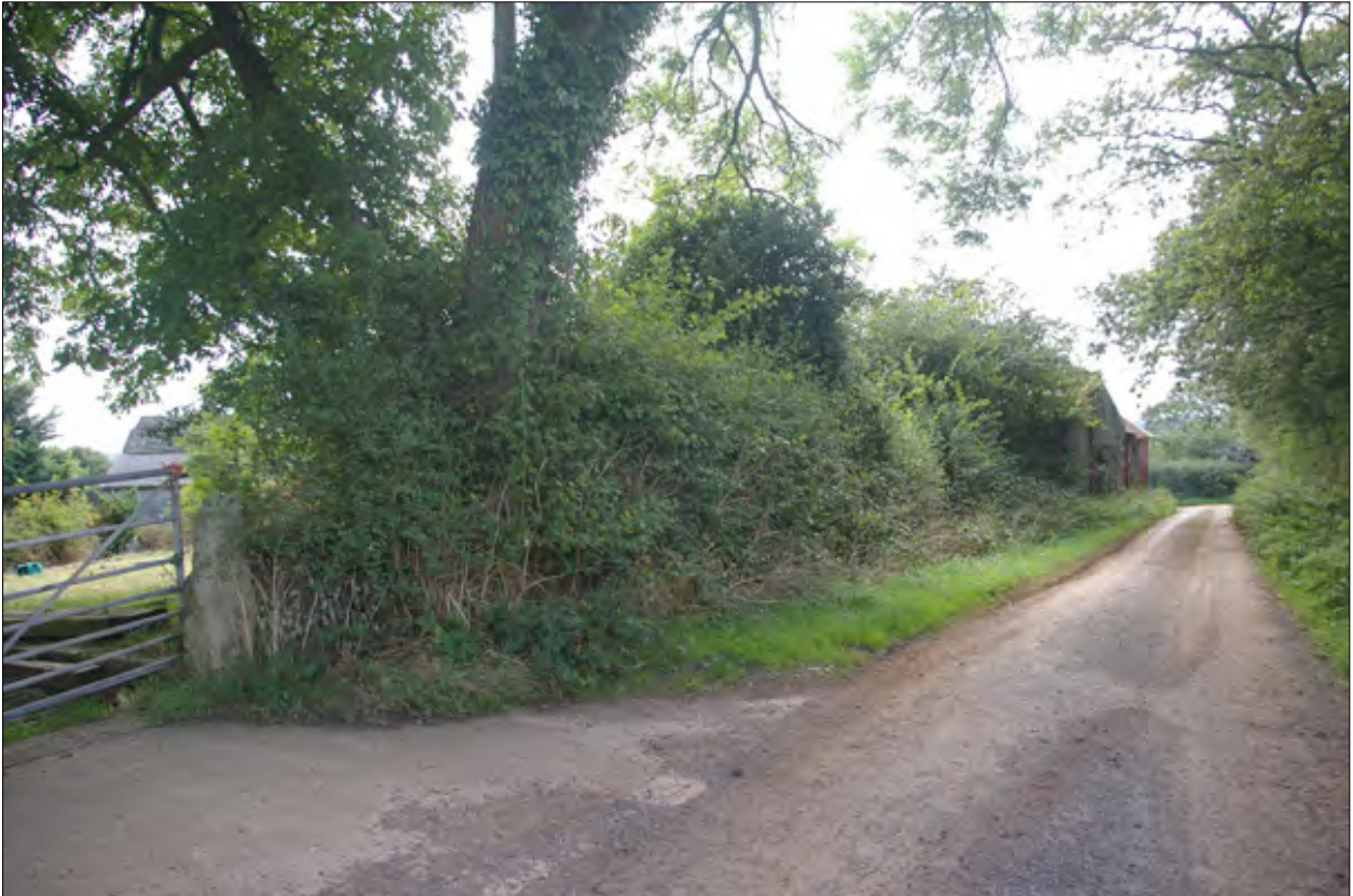
Barns at Upcott Farmhouse; from the west, south-west.
