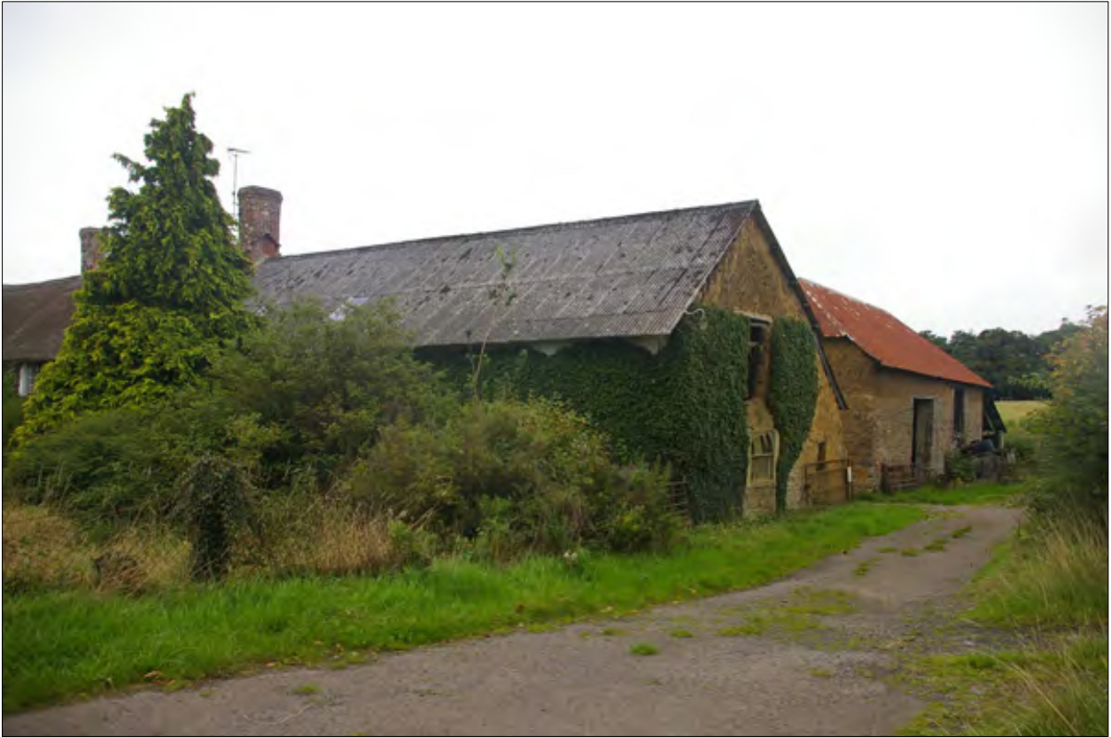
View of the barns at Heath Farmhouse; from the east, north-east.
