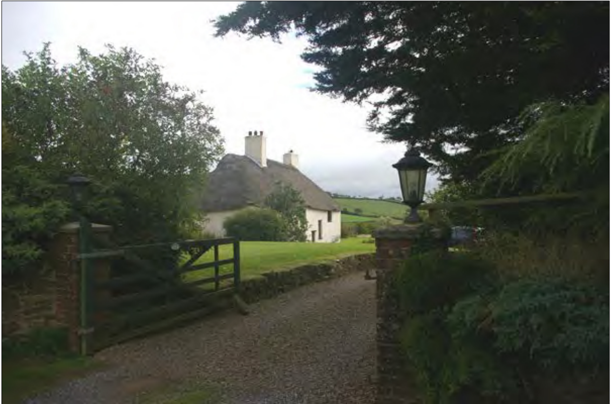
View of Higher Nicol Nymet farmhouse; from the west, south-west.
