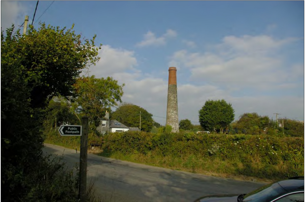
The Listed chimney at Honey Wheel; viewed from the west, looking east.
