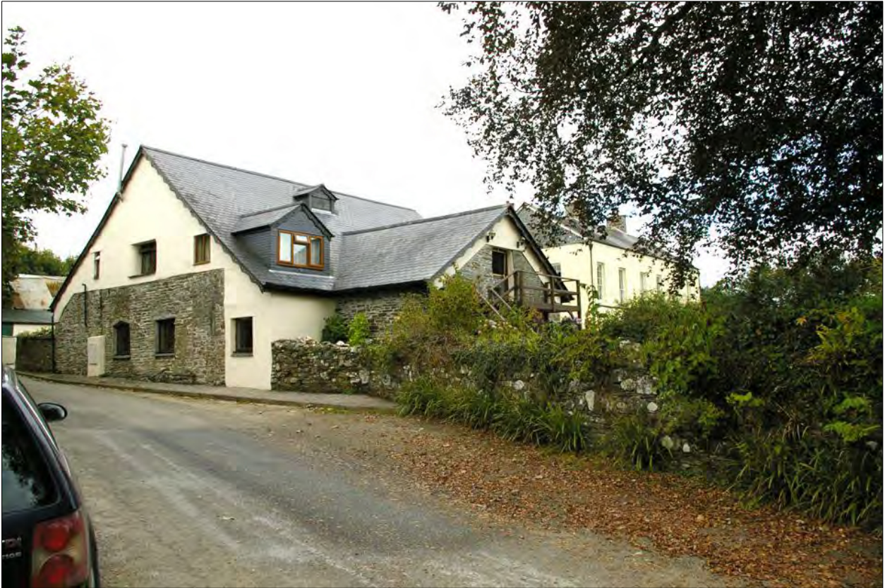
The converted farm building at Trengrove, with the Listed farmhouse in the background; viewed from the south-west, looking north-east.
