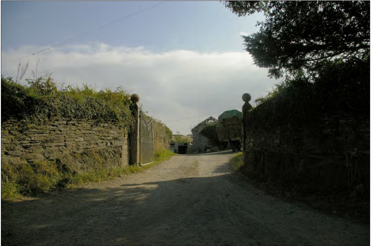
The Listed gate piers and barn at Trehawke; viewed from the north, looking south.
