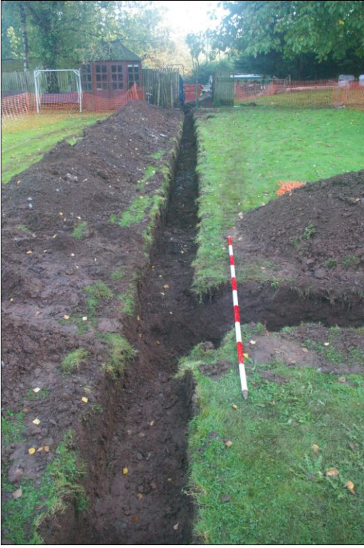
Figure 4: North end of trench #1; viewed from the north-west (2m scale).
