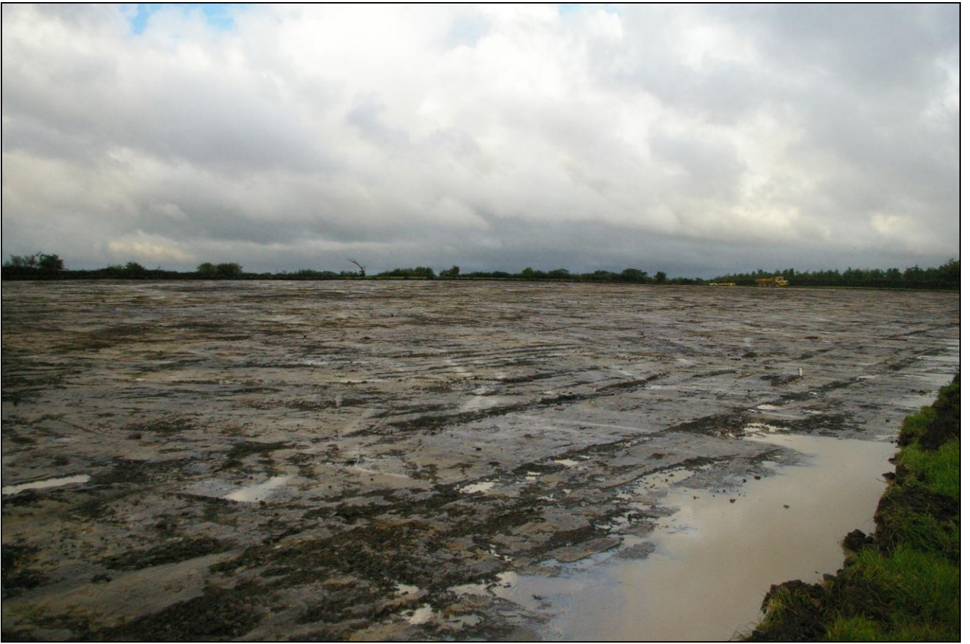
The whole area stripped, viewed from the north-east corner (no scale).
