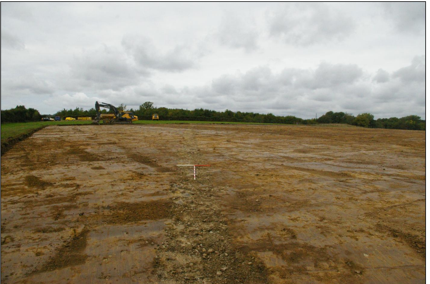
The south-west corner of the site, showing land drain [107]; viewed from the south-south-east (scales 1m & 2m).
