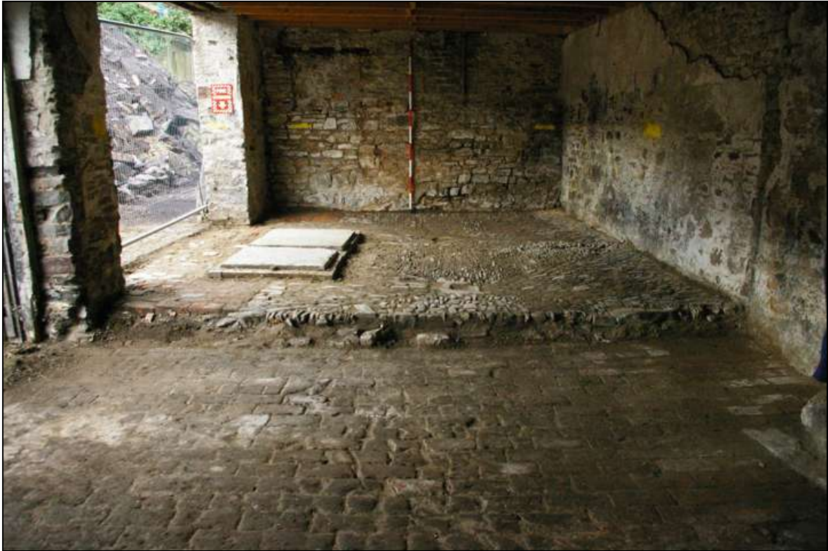
Interior of building on site, pre-excitation; looking west (2m scale).
