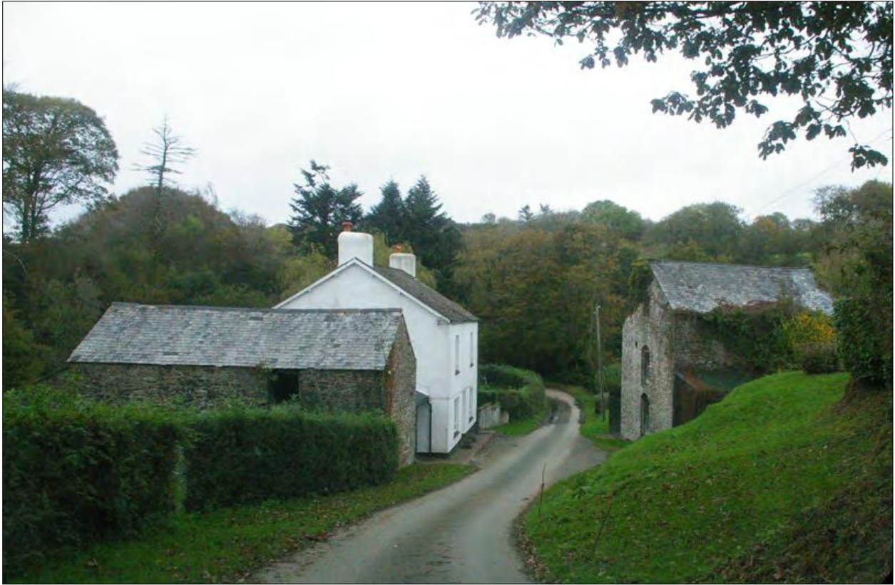
Former Mill at Buckland Brewer, within a steep wooded valley; from the south.
