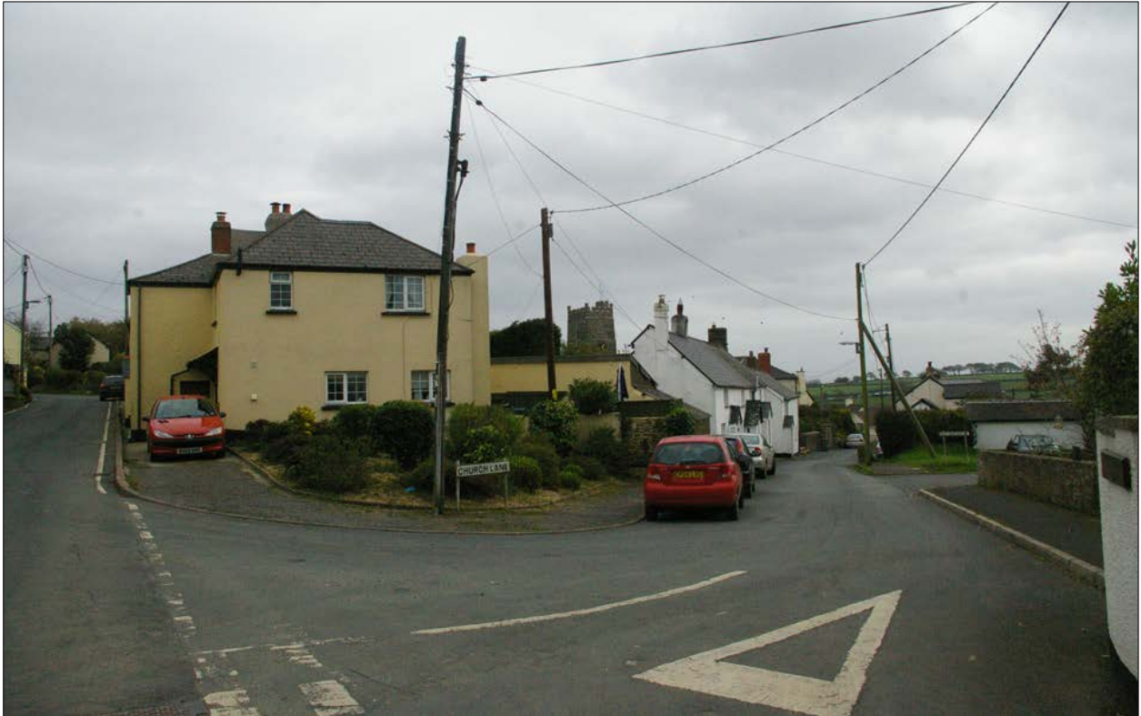
The church in Langtree, within the setting of the village settlement; from the north-west.
