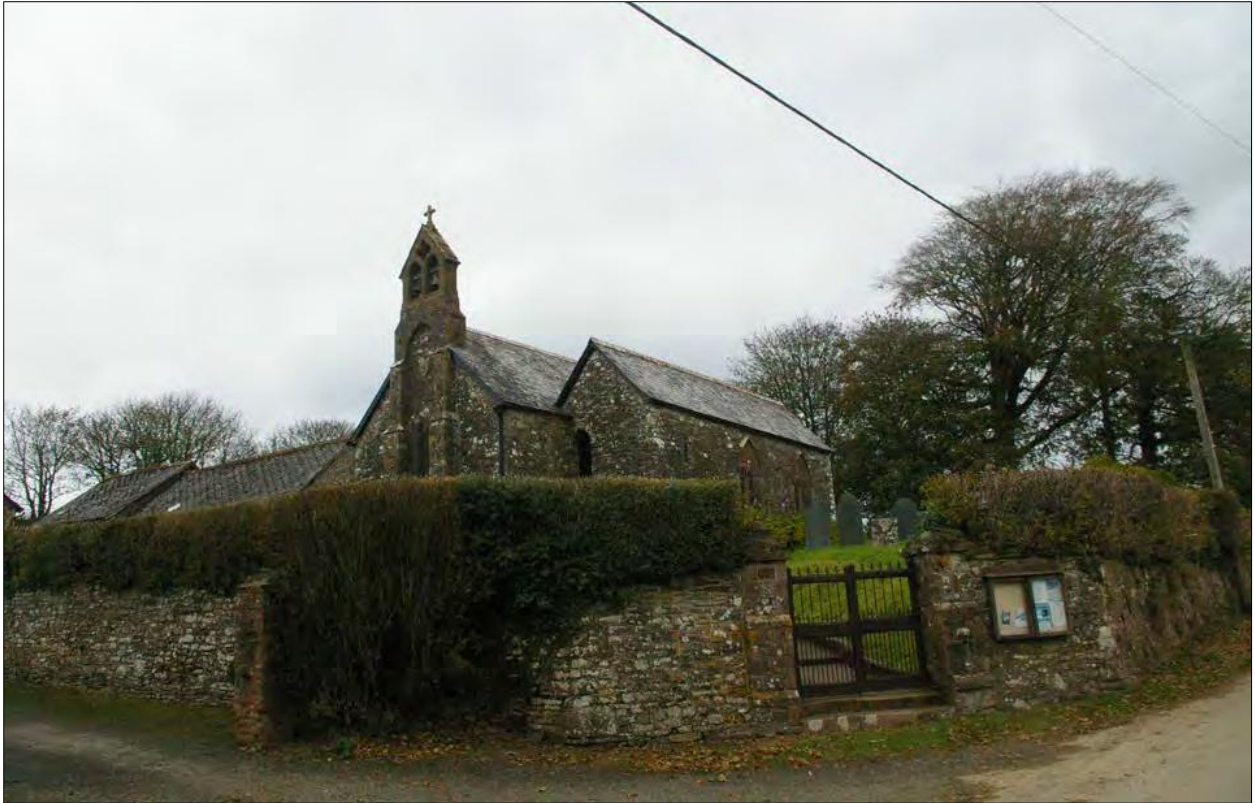
Bulkworthy Church, within its walled churchyard, with the buildings of the adjacent farmyard behind; from the south-west.
