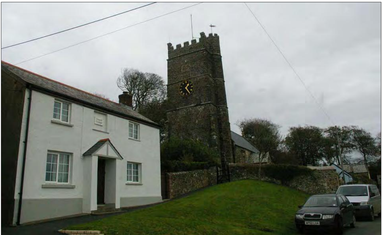
Detailed view of Langtree Church; from the west, south-west.
