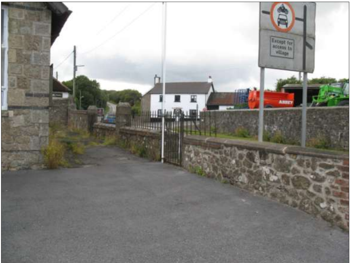
As above, showing the roadside wall, from the east.
