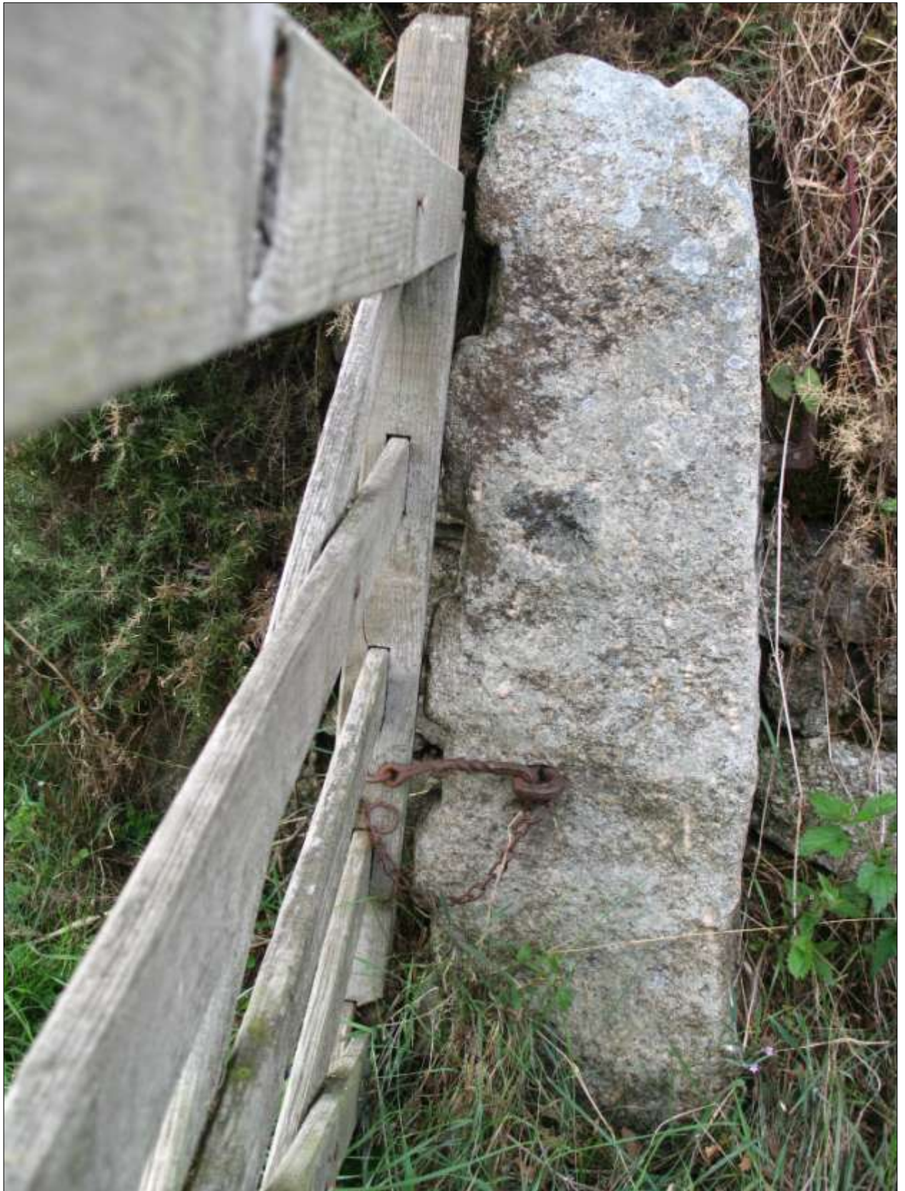
As above, showing the regular grooves in the post (slammer), from the east.
