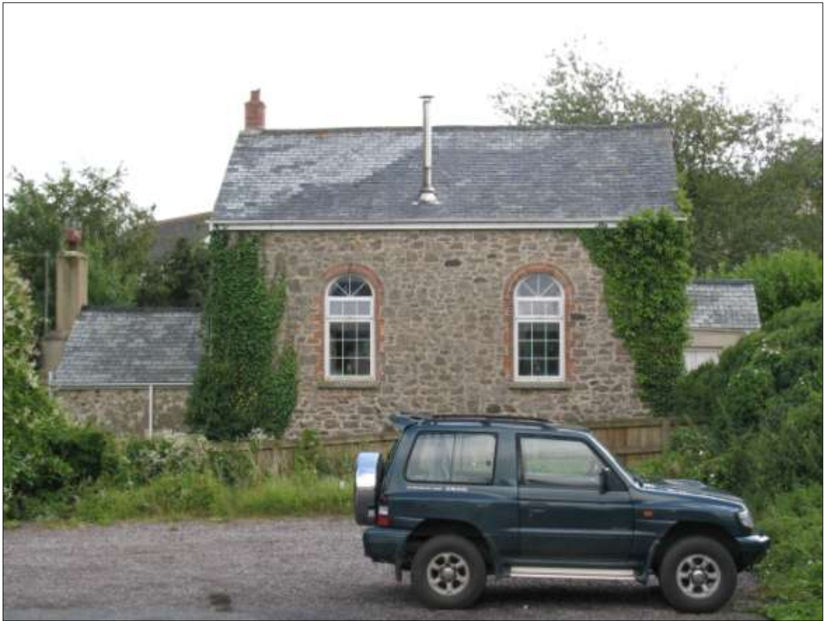
The north elevation of the Old Chapel at Whiddon Down, from the north.
