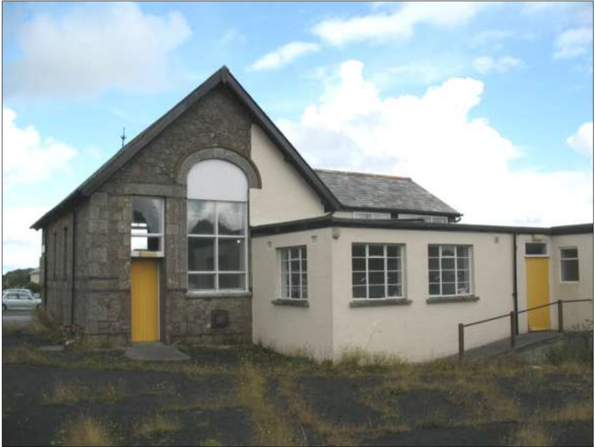
The western elevation of the Village Hall in Whiddon Down, from the west.
