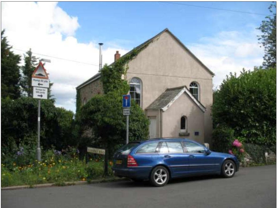
As above, the western elevation, from the north-west.
