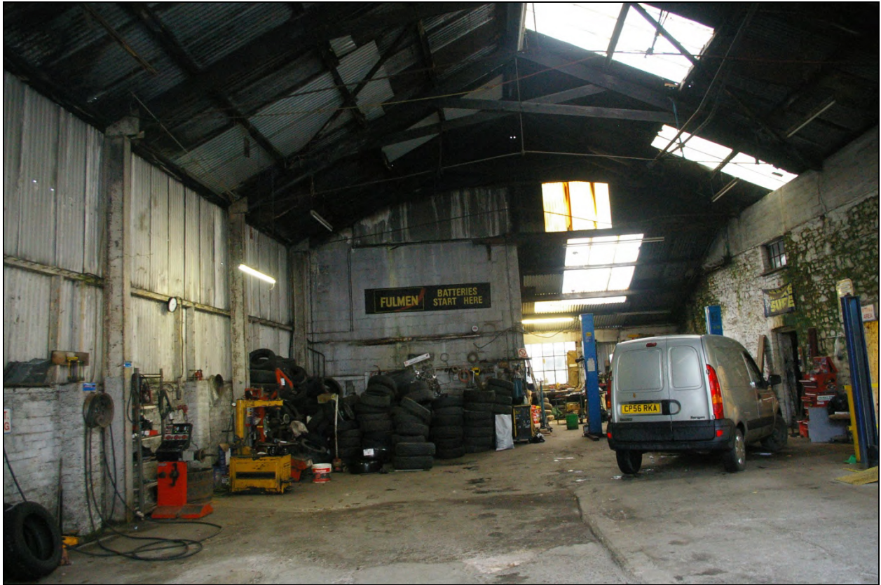
View of open span building from the main doors onto Park Row; from the east.
