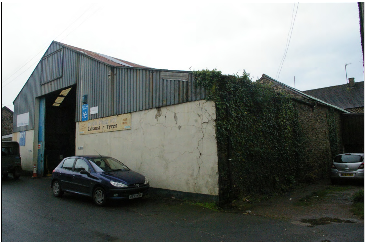
The north and east elevations, showing the stonework of the outbuilding and the flanking walls; from the north-east.
