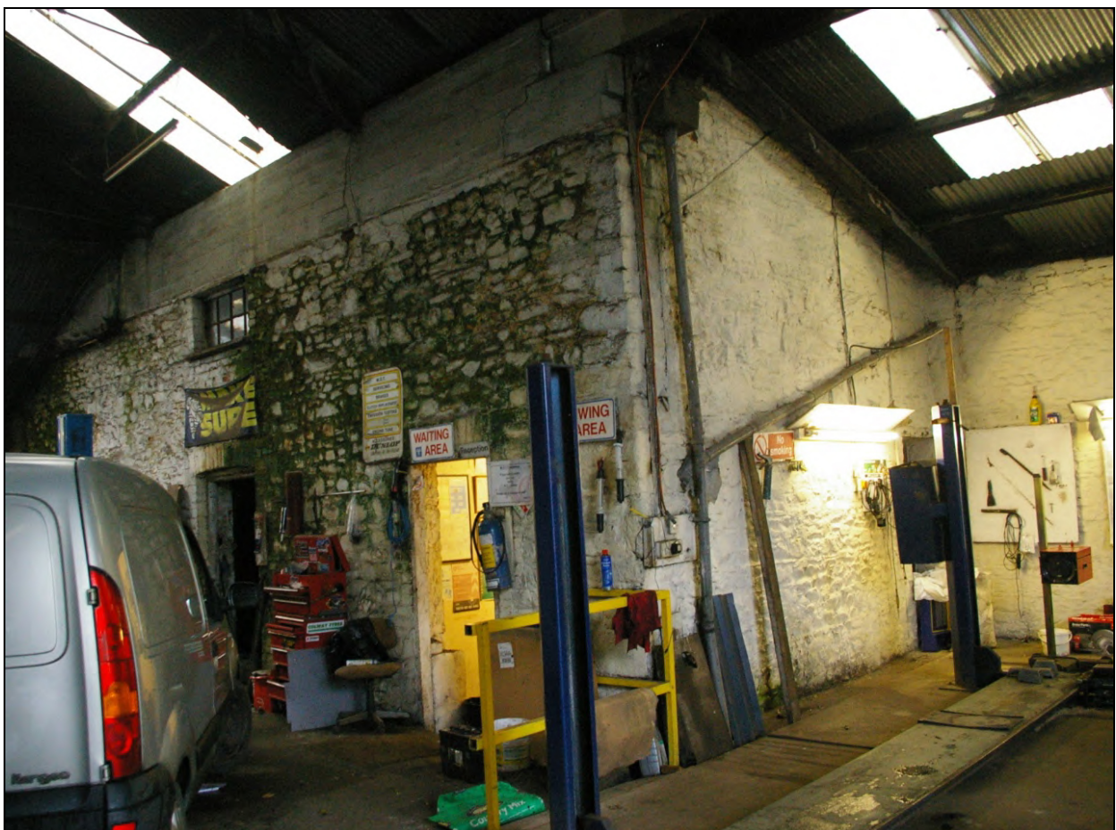
The stone outbuilding within the open span building; from the south-east.
