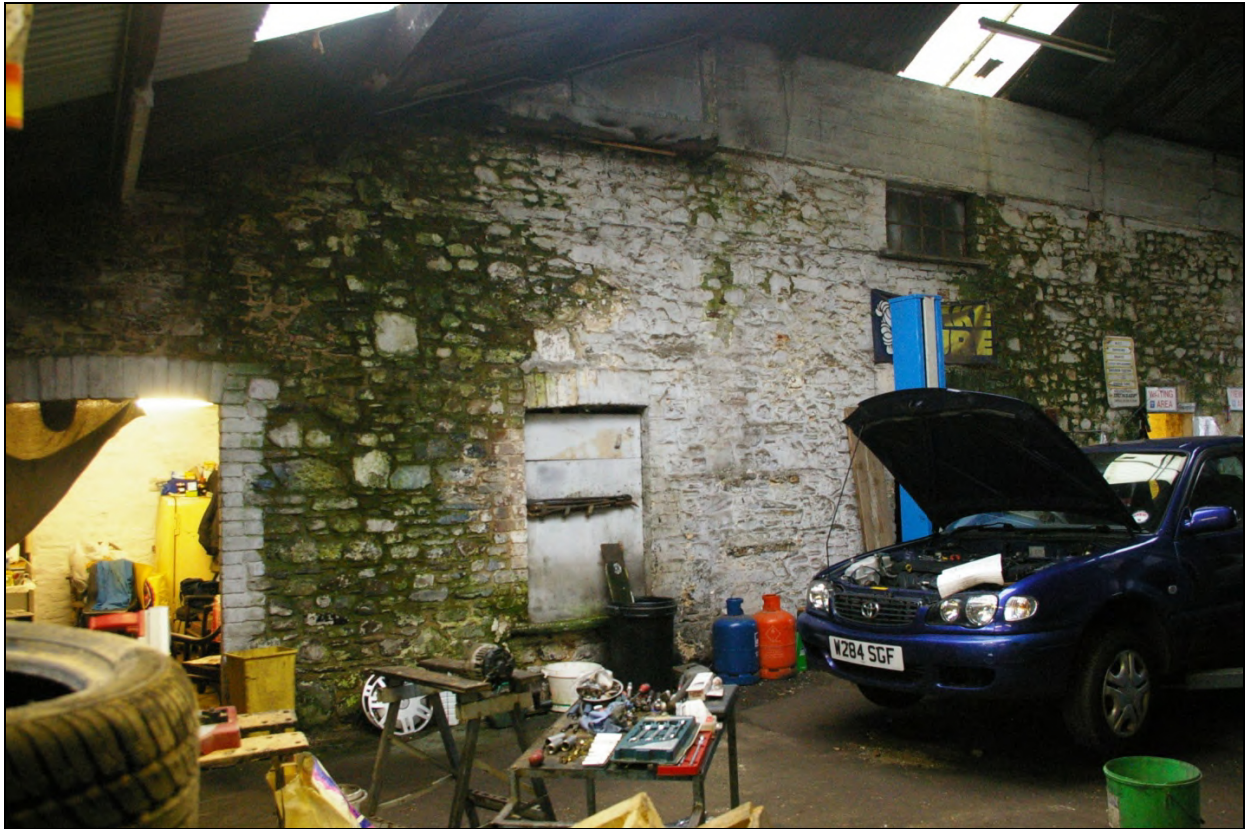
The stone outbuilding, within the open span building; from the south-east.
