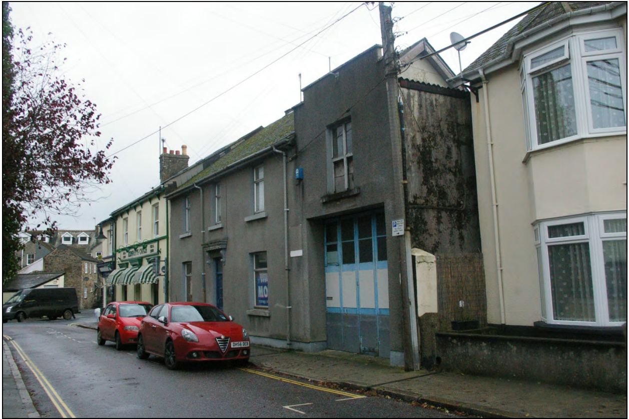
View of the street frontage and garage from the south-west.
