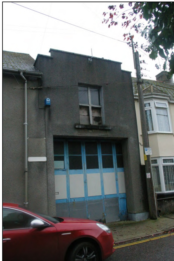
The Kempley Road frontage of the garage building; from the west-north-west.
