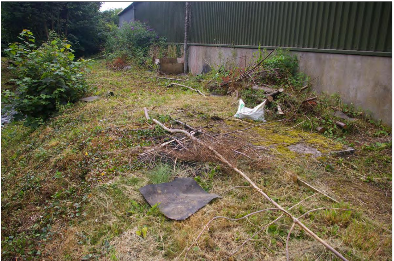
View of some of the concrete pads which line the river bank behind the main range of buildings; from the north-east.
