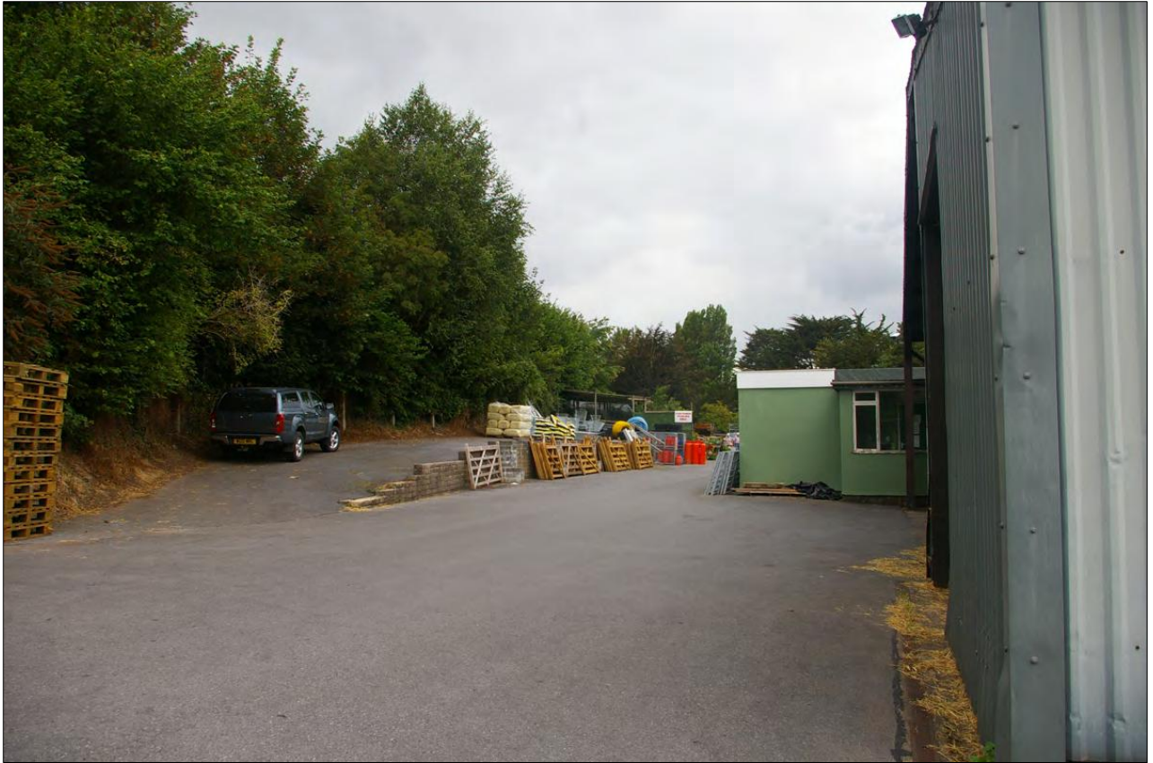
View along the raised western part of the site which is now retained by modern concrete block walls; from the south-east.
