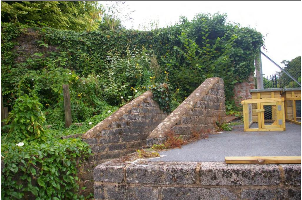
Figure 10: View of the steps leading up to the raised area along the western boundary and the 20 th century brick-blocked opening seen in the stone wall; from the east-north-east.
