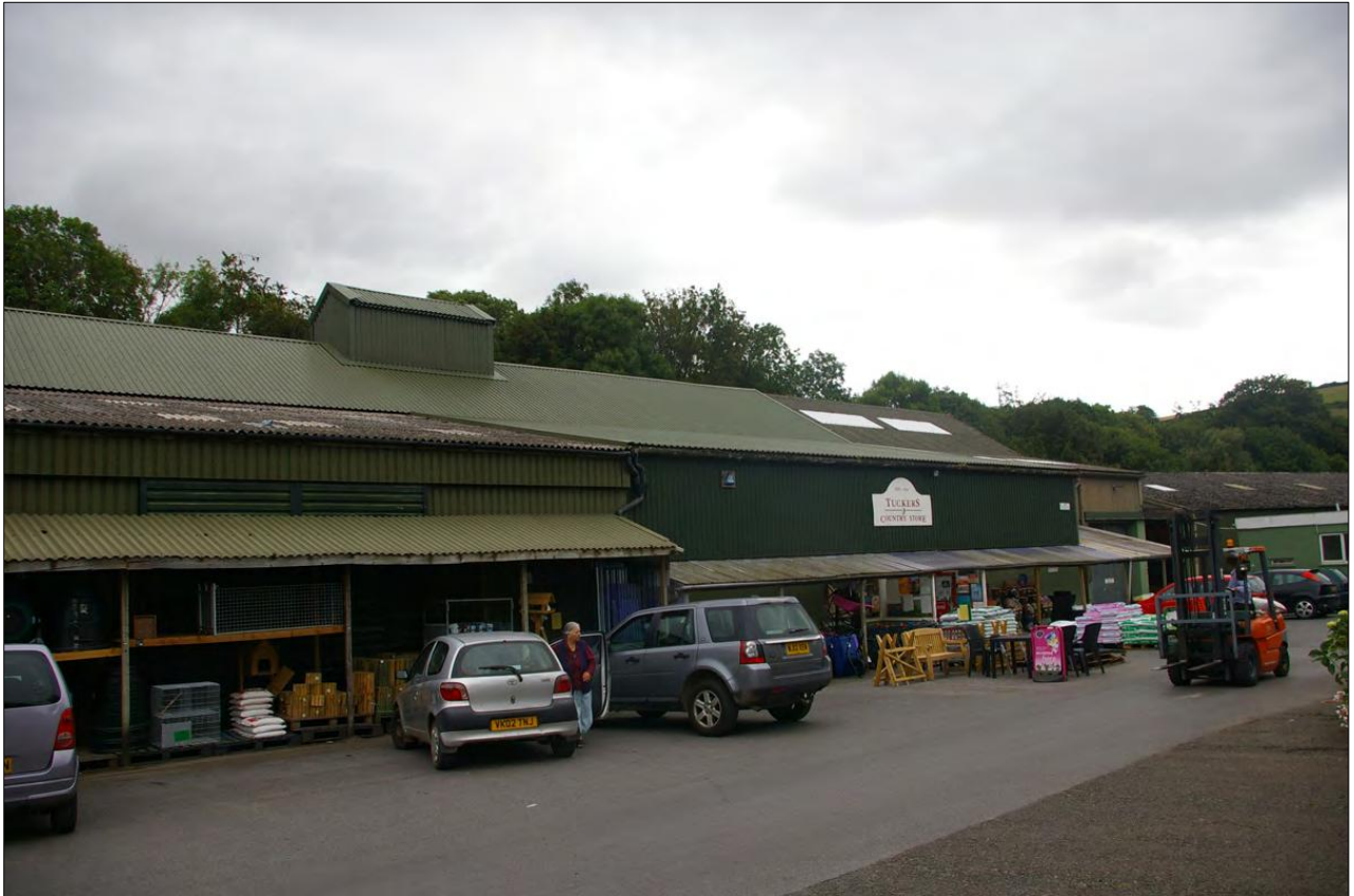
View down the long main range of buildings; from the west-north-west.
