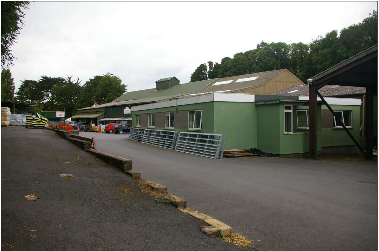
The office building and main range of buildings behind; from the west-south-west.
