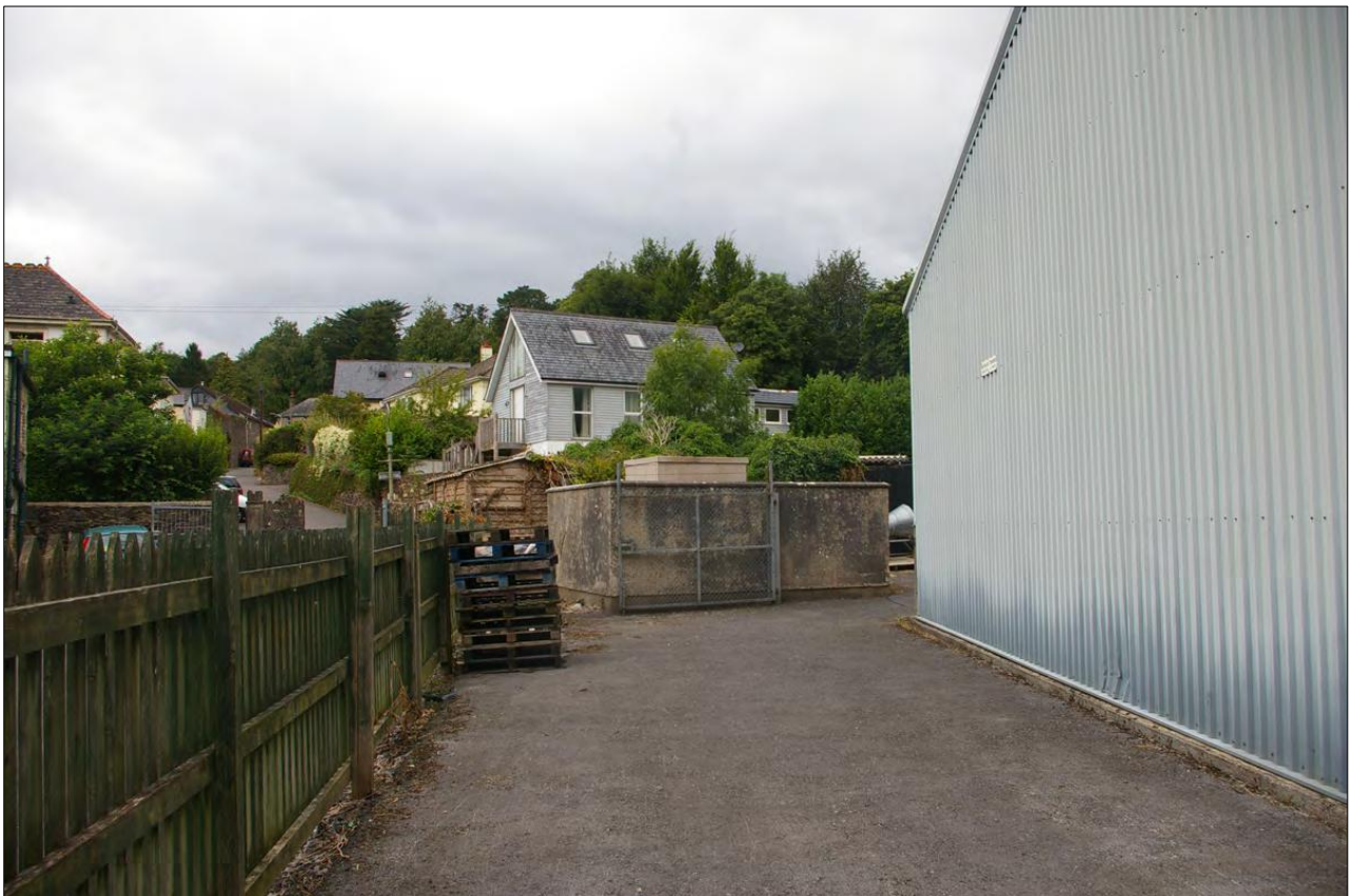
View back along the southern boundary of the site, looking to Stonepark Road which rises to the west and uphill towards Ashburton; from the east.
