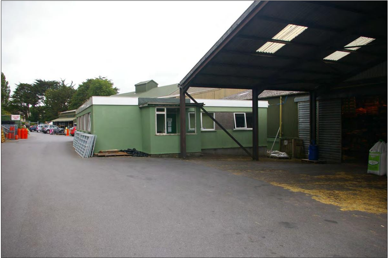
The flat-roofed office building; from the south-west.
