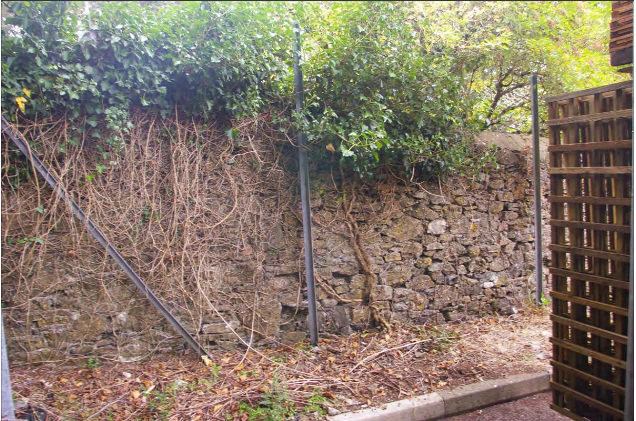
The north stone boundary wall of the site; from the south.
