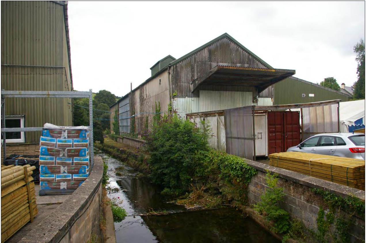
View down the main range of buildings from the bridge over the river; from the north-east.
