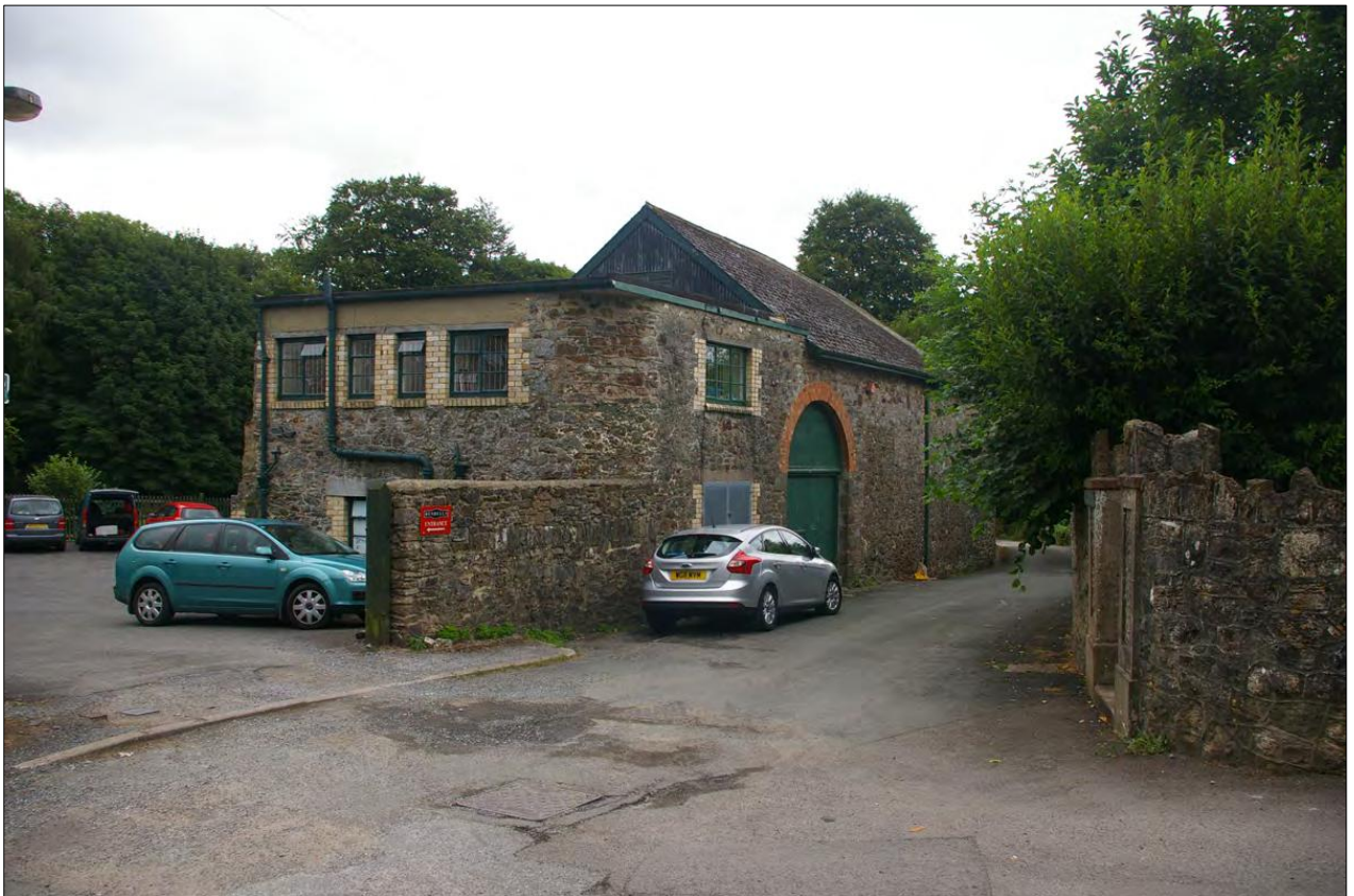
The auction rooms building, formerly a 19 th century building associated with the railway station; from the north.
