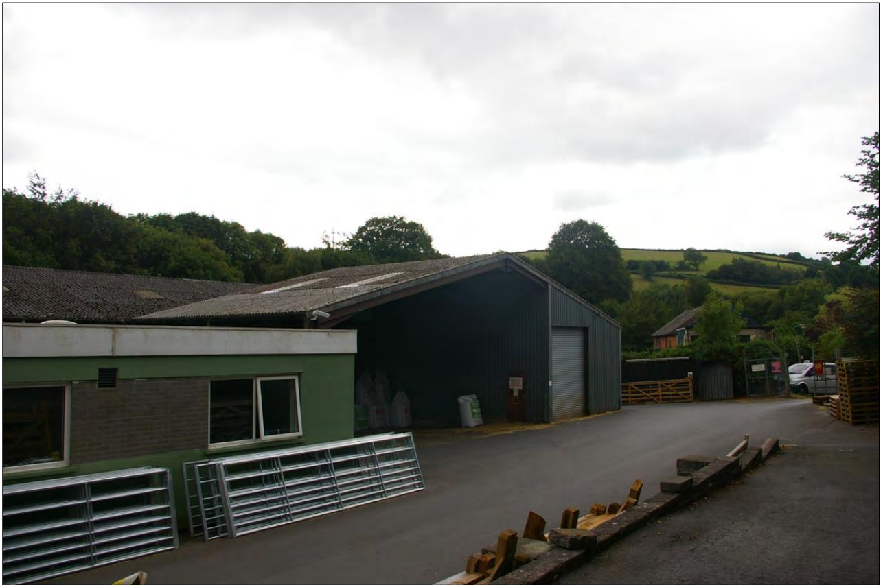
The open shed to the south of the site; from the west-north-west.
