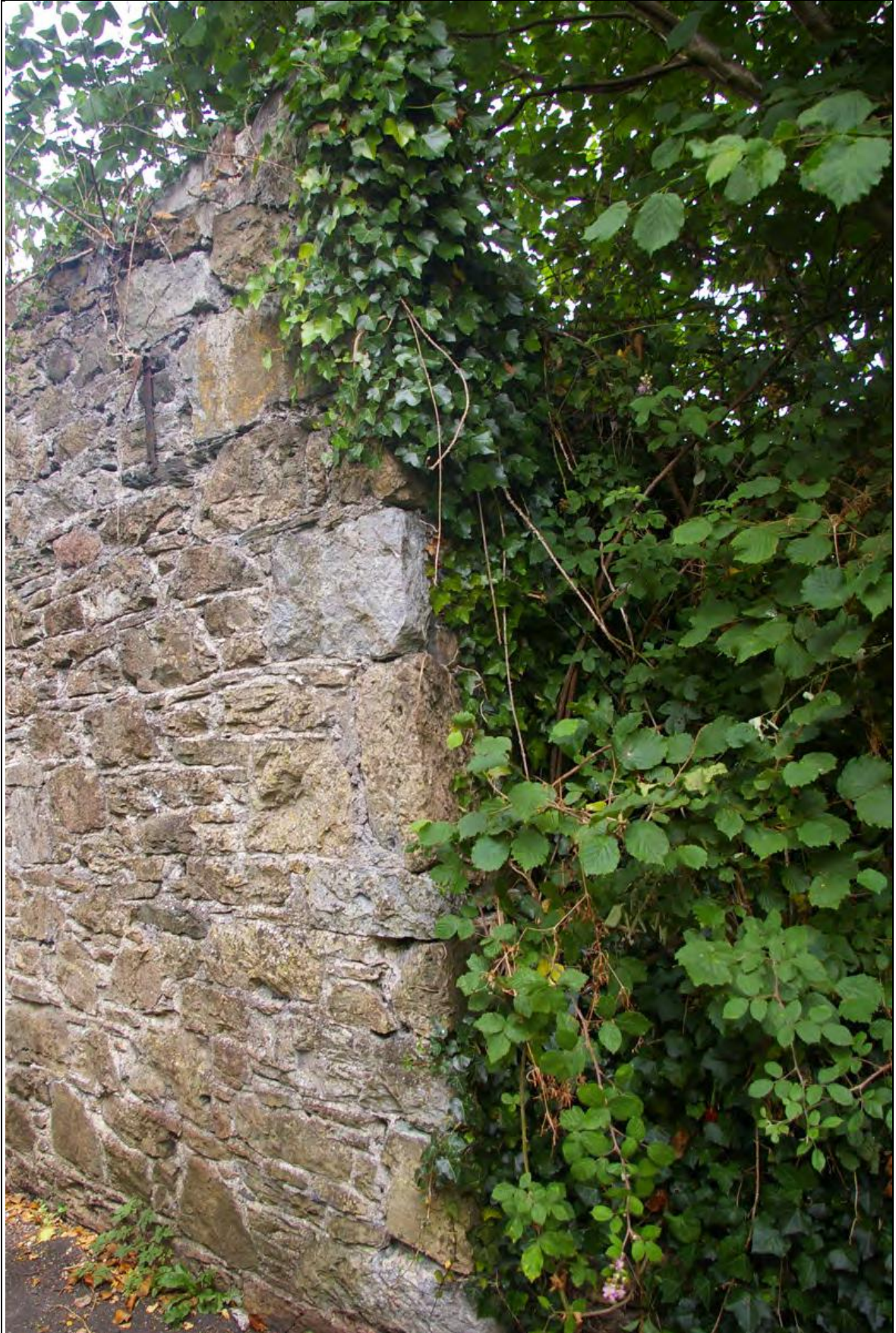
The southern end of the wall showing the roughly dressed stone quoins, where it meets the historic hedgebank; from the south-west.
