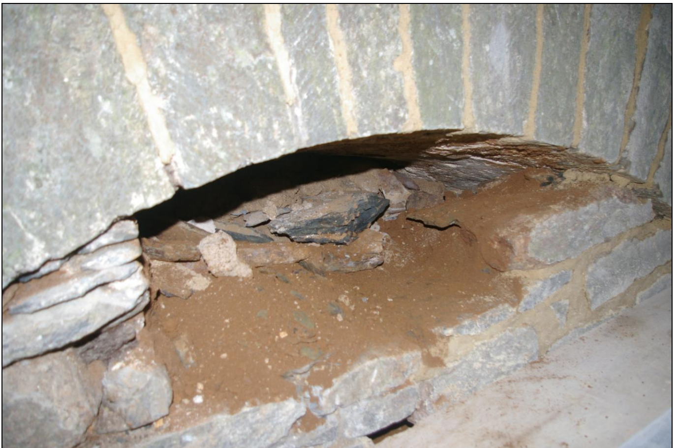
Figure 2: The blocked doorway formerly leading to the south transept; from the south west.
