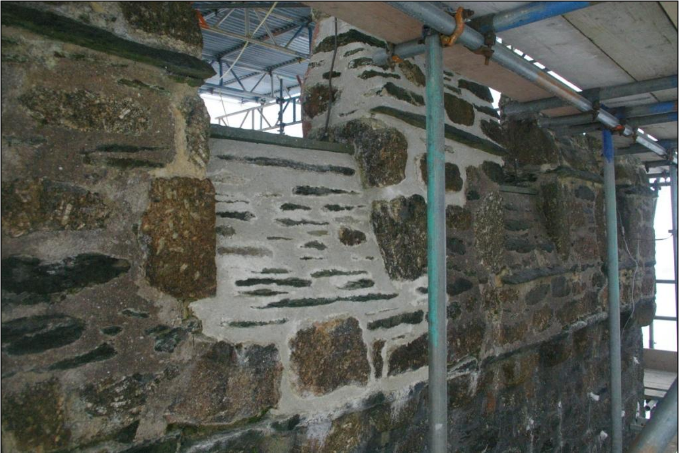
Figure 1: The top of the tower during consolidation works.
