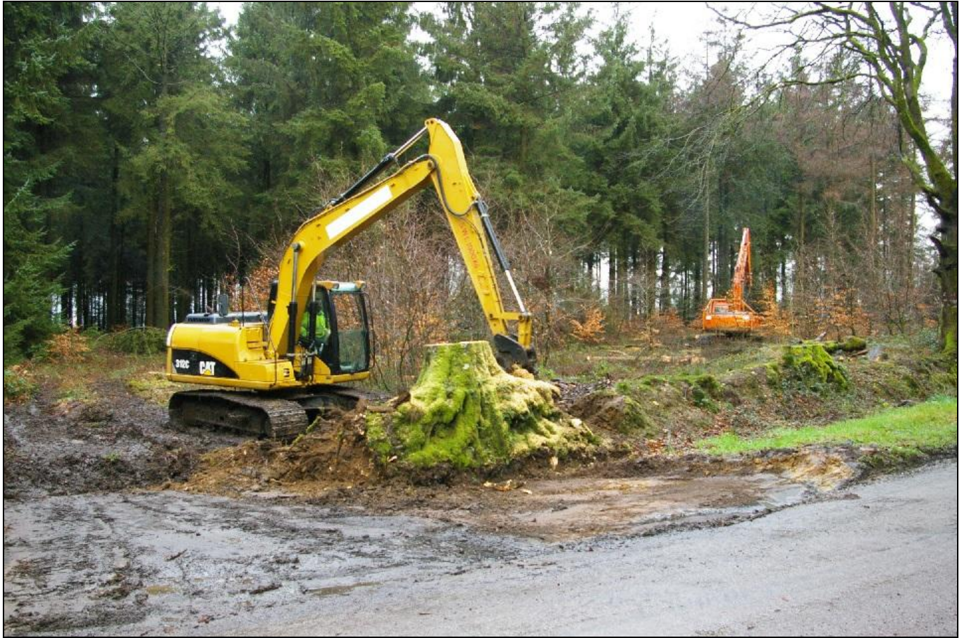
Figure 3: The excavator removing the beech tree stump; viewed from the south-south-east.
