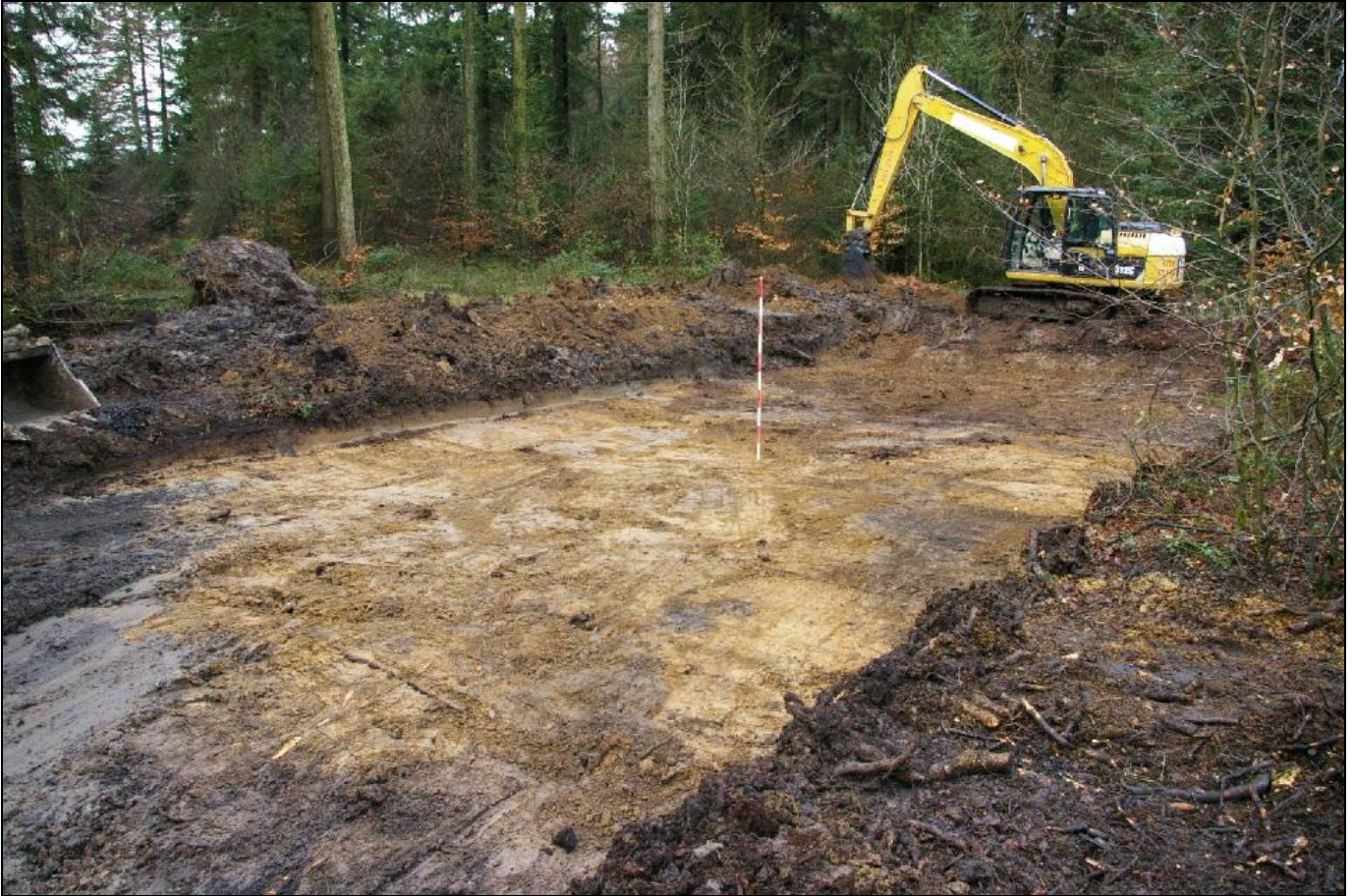
Figure 5: The completed strip; viewed from the east (scale 2m).
