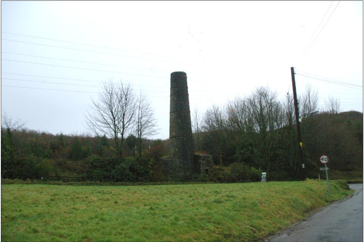
Chimney in the St Austell River valley; from the west.
