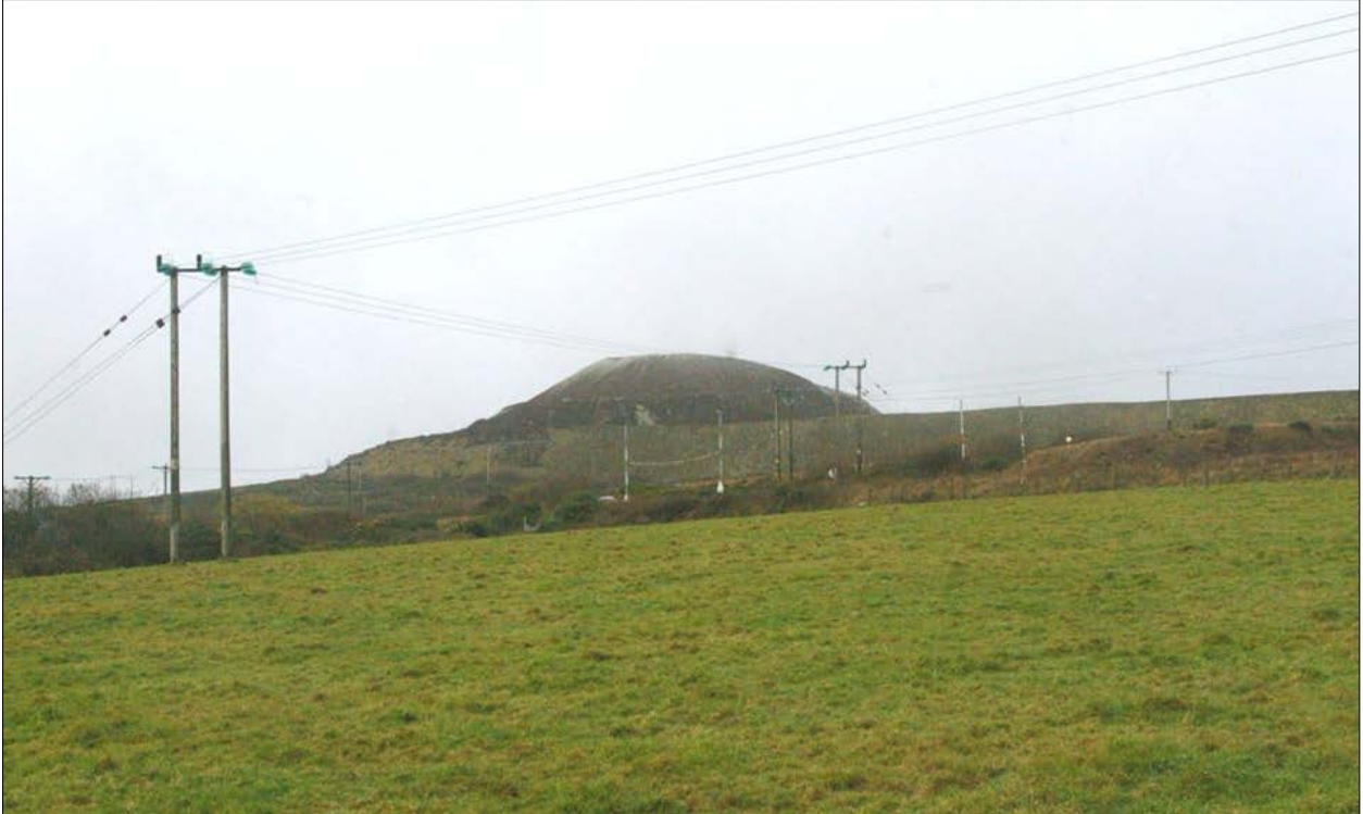
View towards St Stephen beacon; from the south-east.
