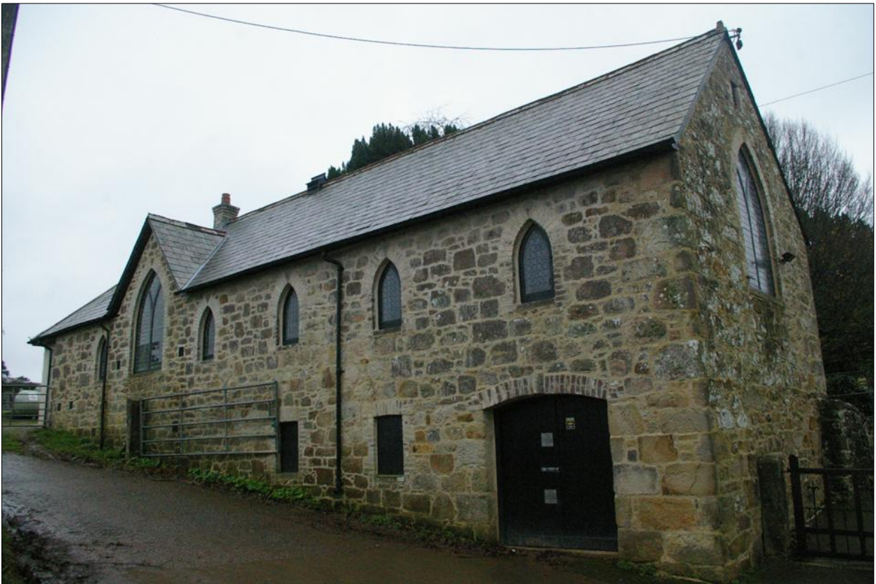
St Mewan Sunday School; from the west-north-west.
