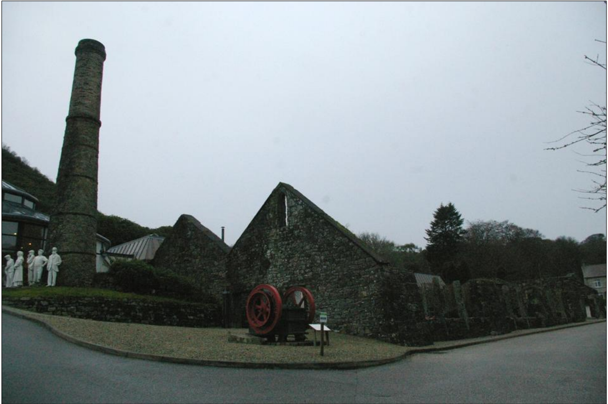
Wheal Martyn, main buildings; from the south-east.
