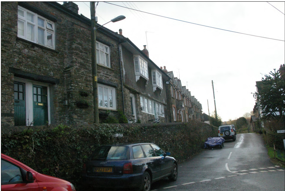
Eliot Terrace, almshouses, in St Germans, within the conservation area; from the east.
