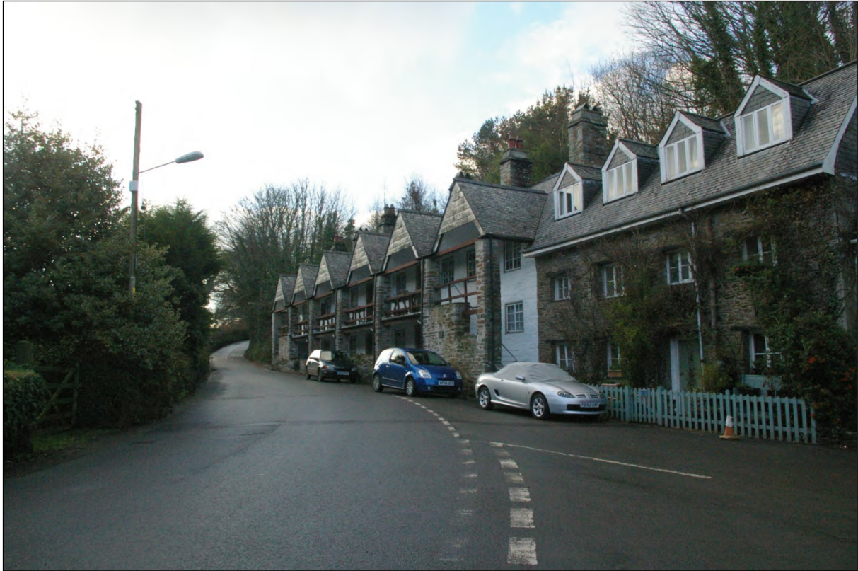
The Sir William Moyles Almshouses in St Germans, set down in the valley, on the north side of the stream; from the south, south-east.
