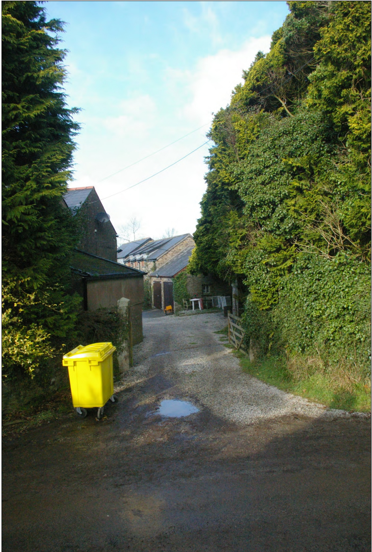
View of the listed outbuildings at St Erney House; from the east.
