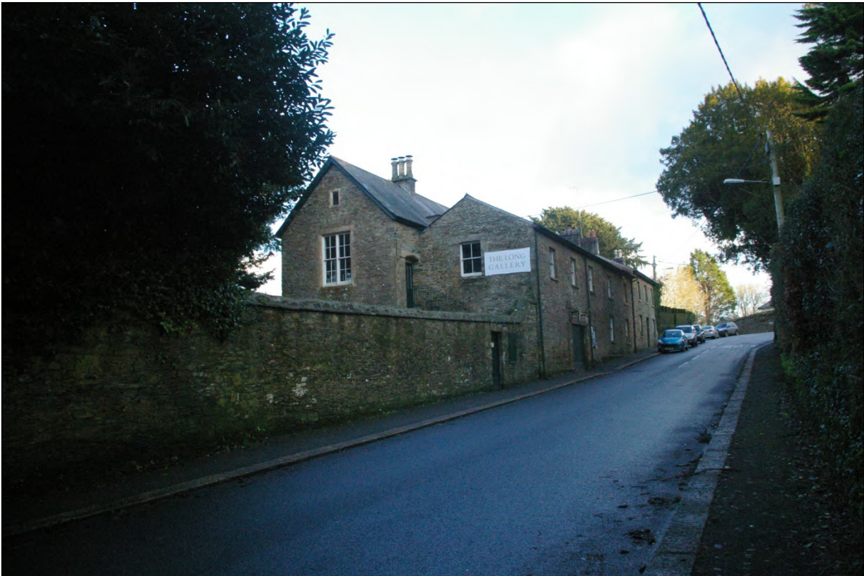
Views along Church Road, within St Germans, within the conservation area; from the north-west.
