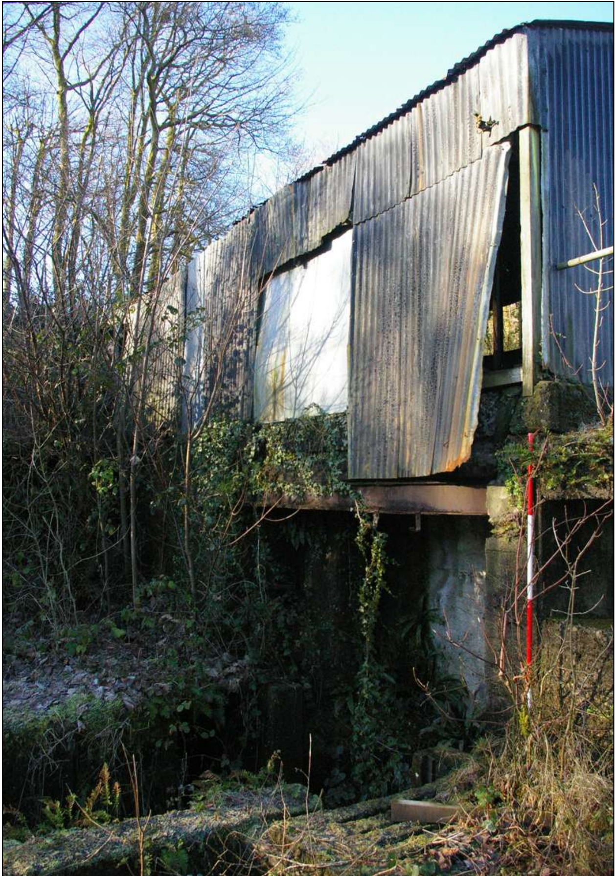
Figure 74: As above, viewed from the south-east (scale 2m).
