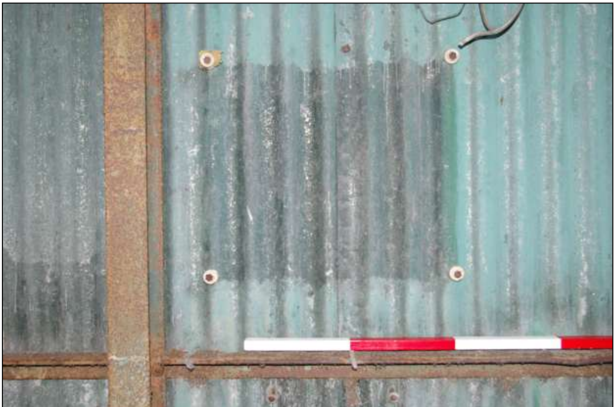
Figure 127: Detail of one of the paint scars on the north wall of B1; viewed from the south (scale 1m).
