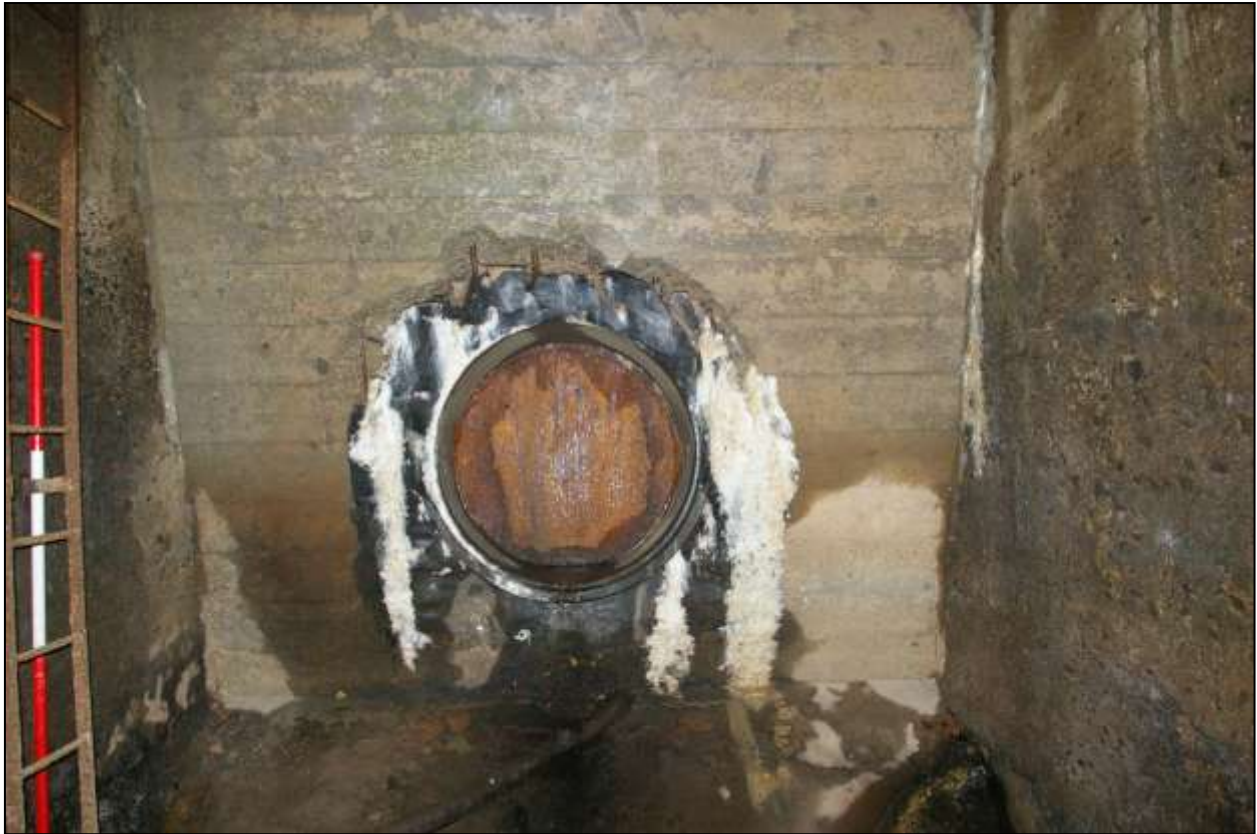
Figure 85: The 1950s sluice gate, viewed from the south (scale 2m).
