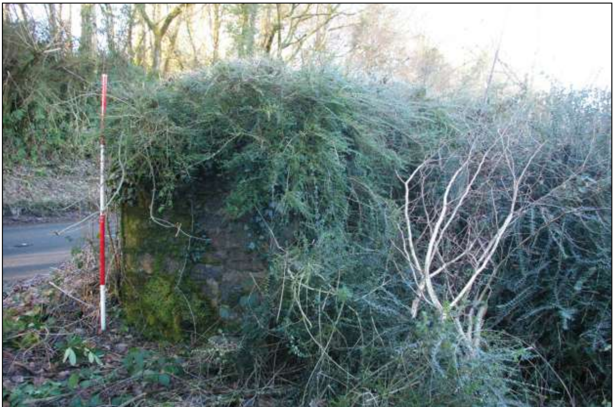
Figure 23: As above, viewed from the south-east (scale 2m).
