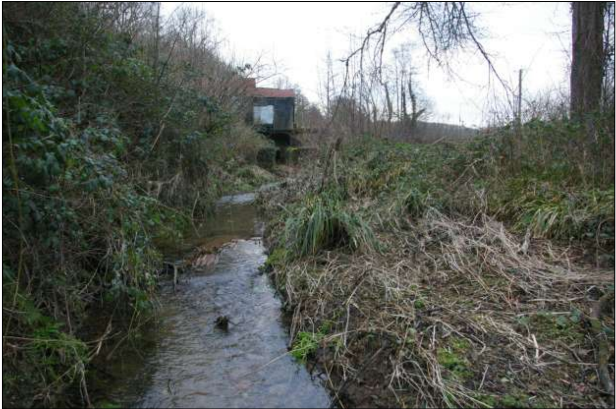
Figure 106: View back along Leat 3 to Building #2; viewed from the south (no scale).
