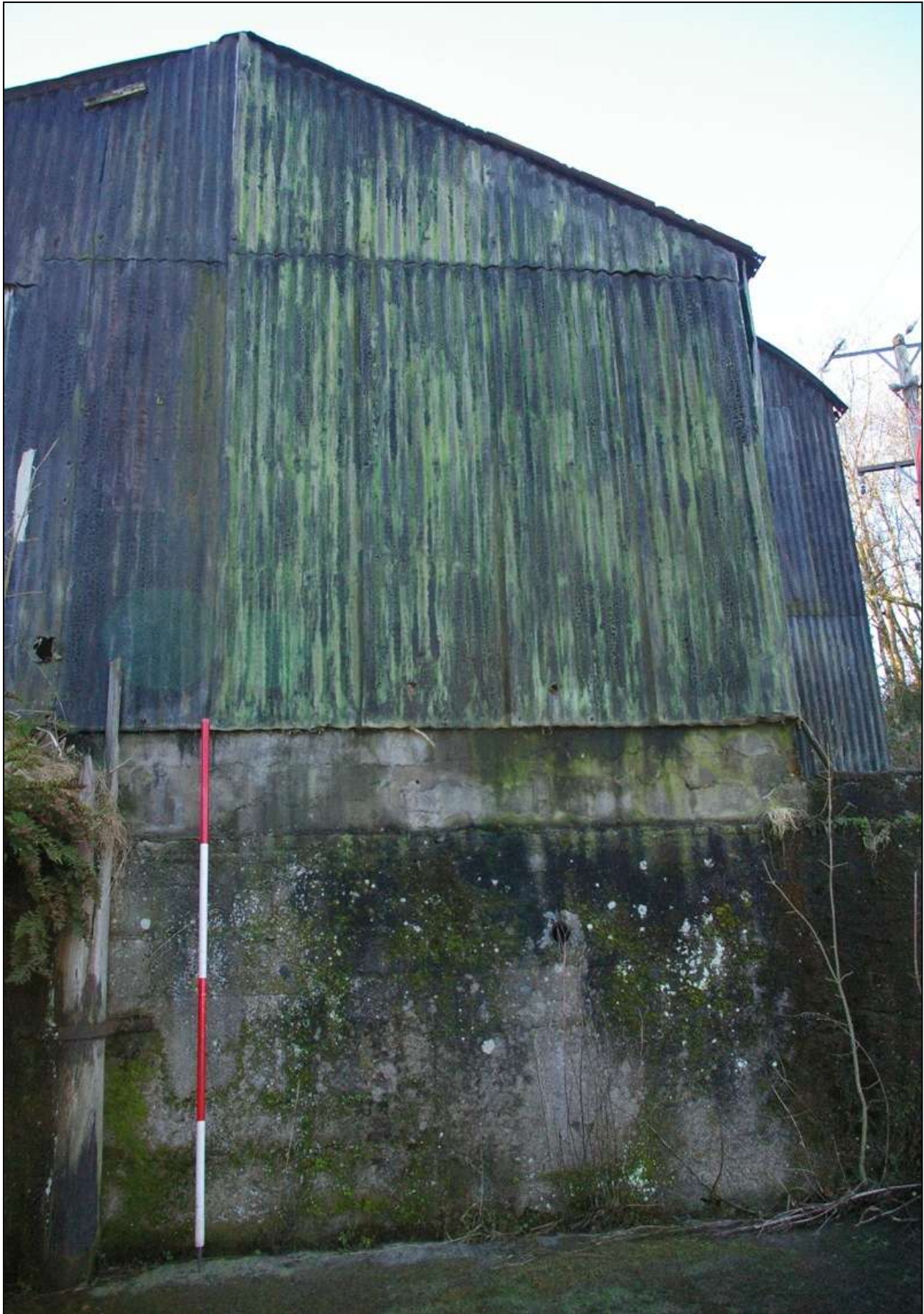
Figure 50: The eastern elevation of B2, viewed from the east (scale 2m).
