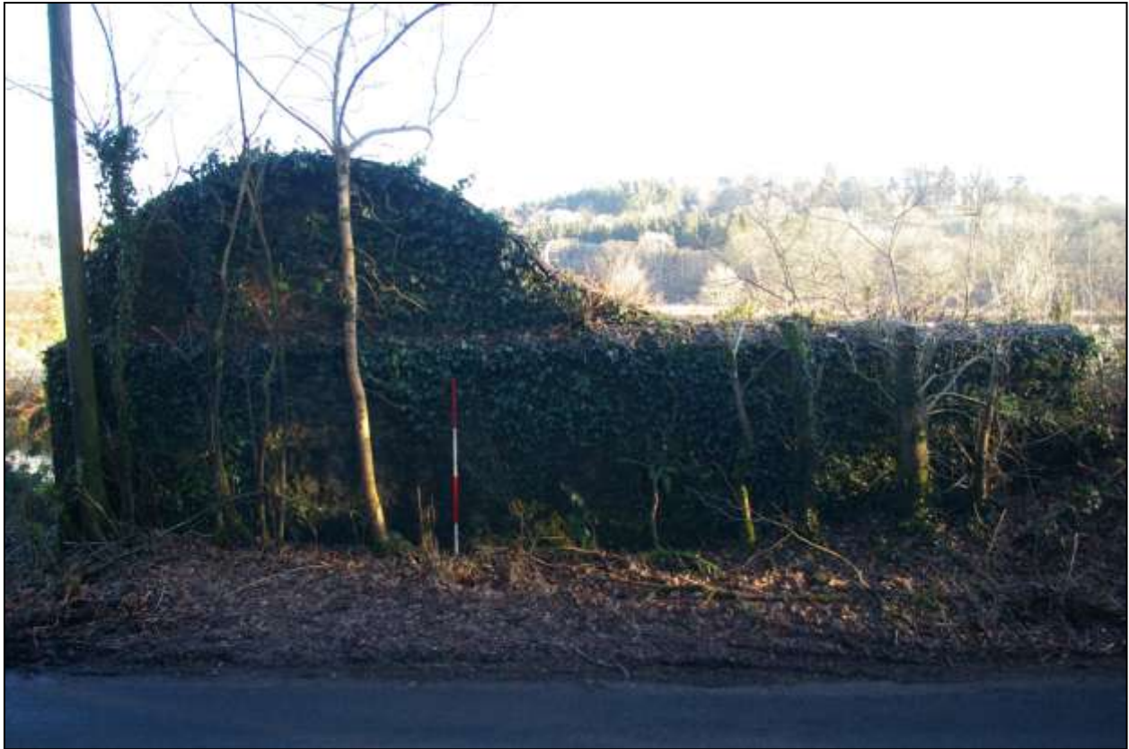
Figure 16: West elevation of B1, viewed from the west (scale 2m).
