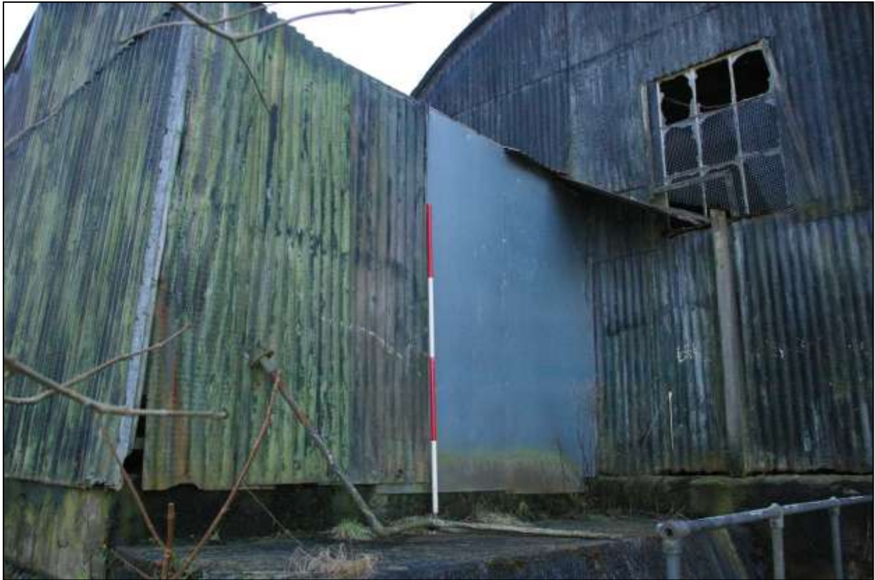
Figure 46: The north elevation of B2, viewed from the north-east (scale 2m).
