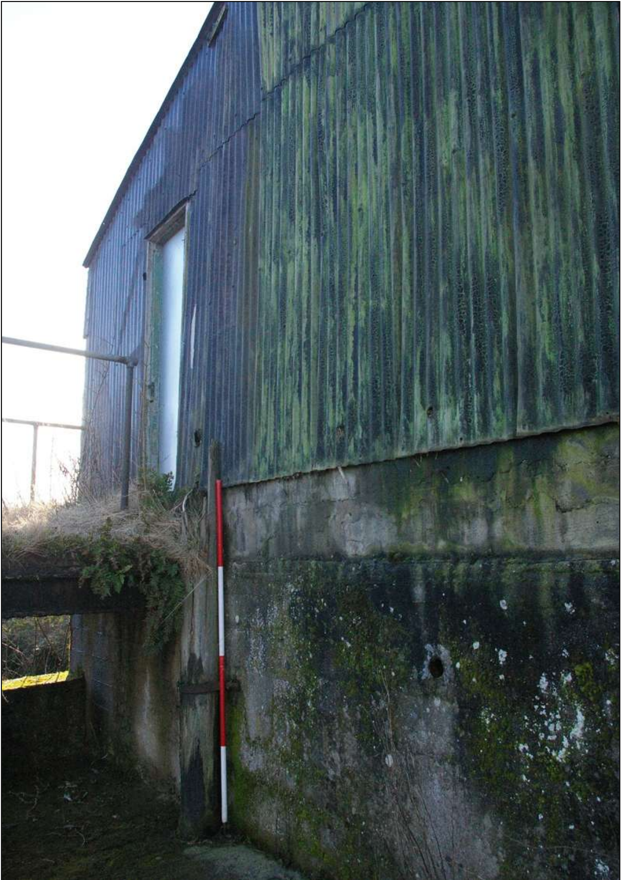
Figure 54: The east elevation of B2, viewed from the north-east (scale 2m).
