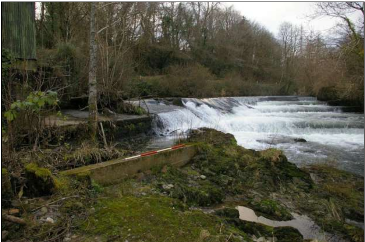
Figure 109: The wall flanking Leat 1, viewed from the south-east (scale 2m).
