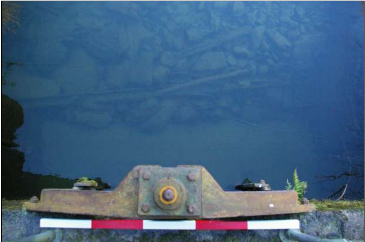
Figure 36: As above, showing an iron girder in the streambed; viewed from the south (scale 1m).
