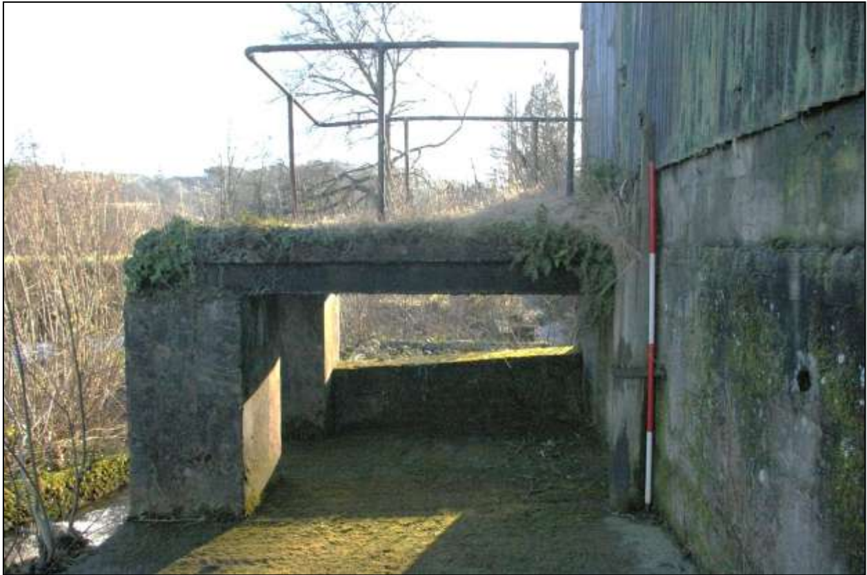
Figure 56: The platform, viewed from the north (scale 2m).
