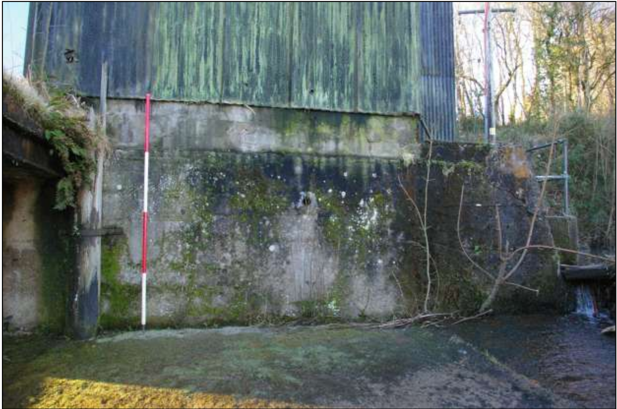
Figure 51: As above, showing more of the spillway.
