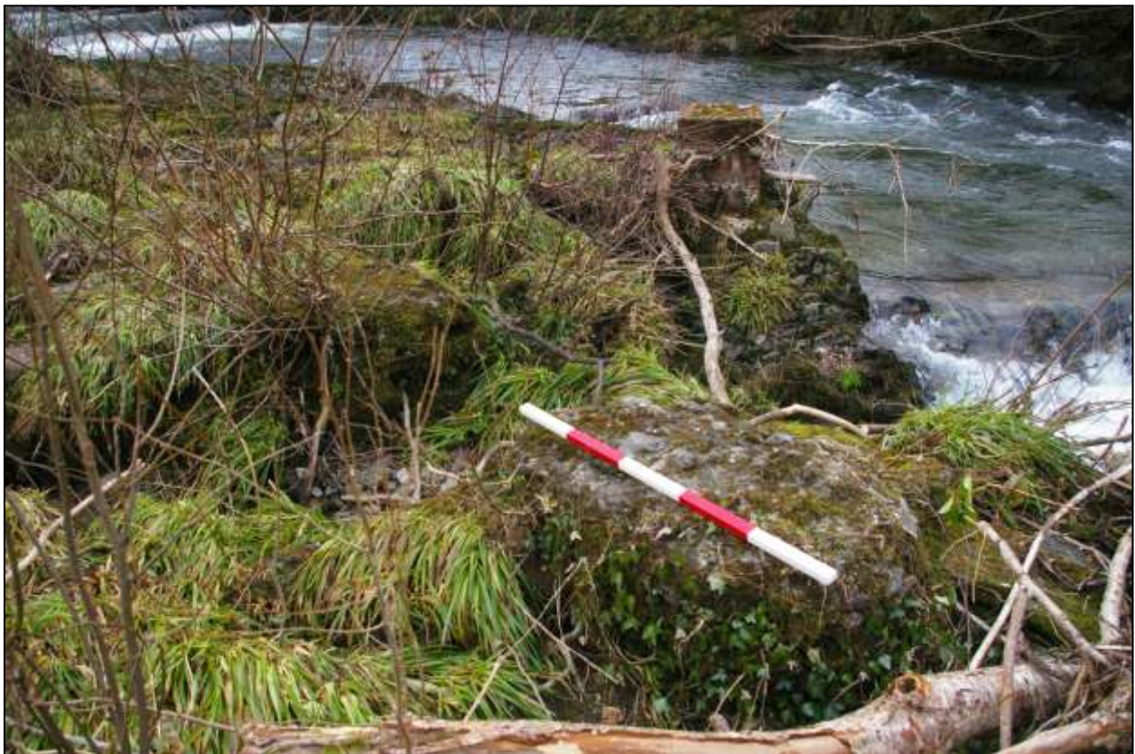
Figure 114: Block of concrete next to Wall 1, with the concrete pillar in the background; viewed from the south-west (scale 1m).
