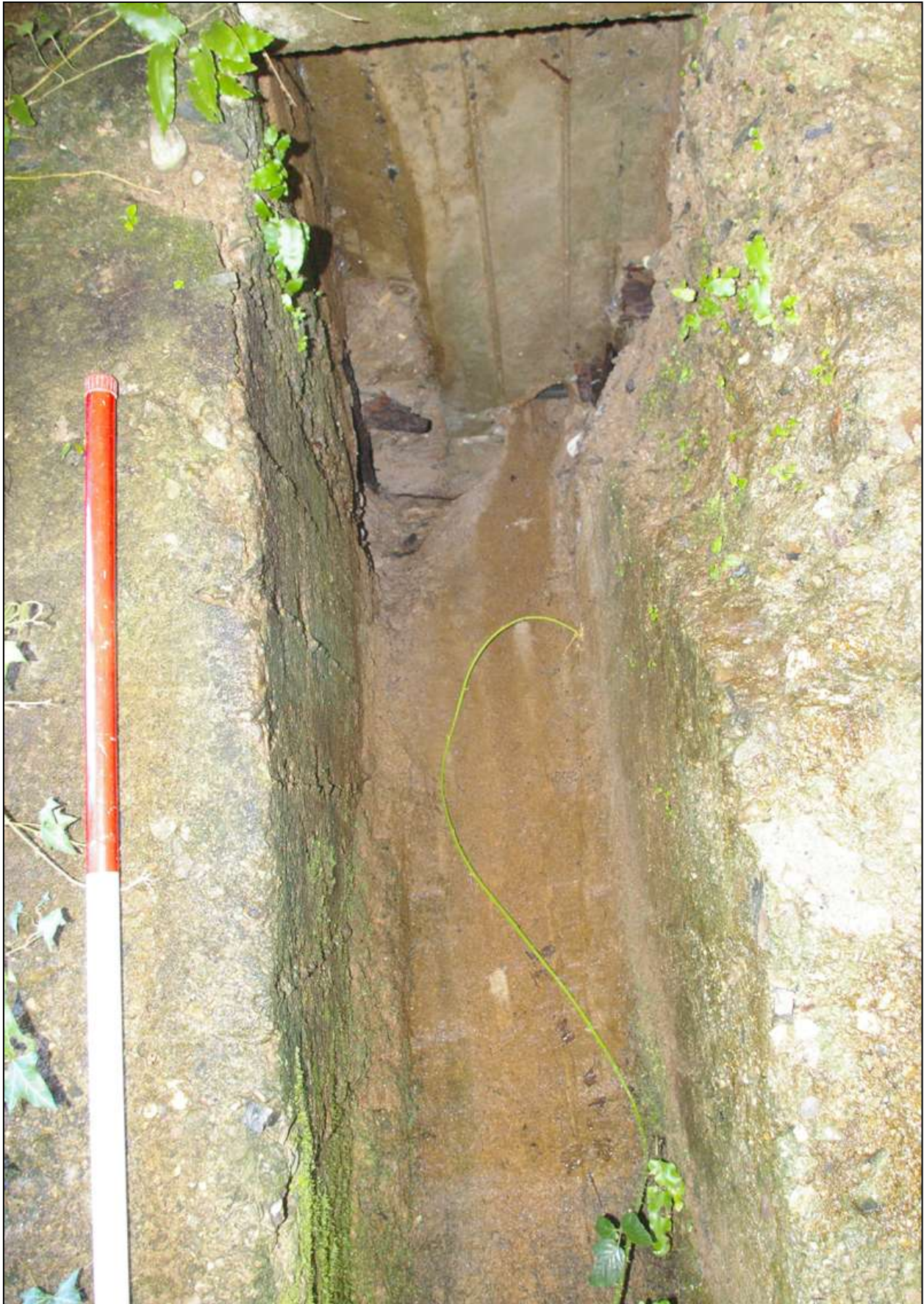
Figure 81: As above, view of the sloping cavity between the 'buttresses'; viewed from the east (scale 2m).
