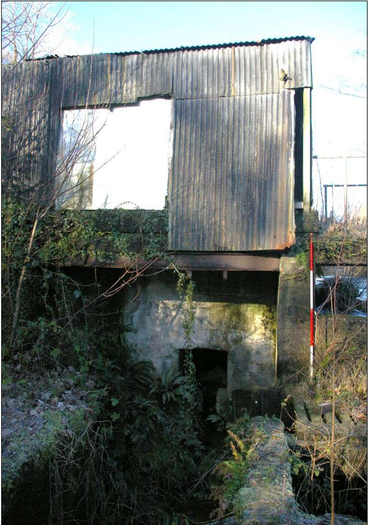
Figure 73: The south elevation of B2, viewed from the south (scale 2m).
