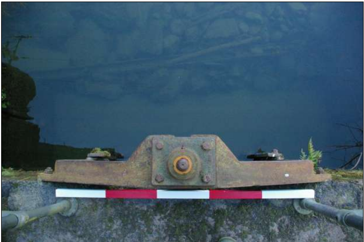
Figure 35: The current sluice gate, viewed from above (scale 1m).
