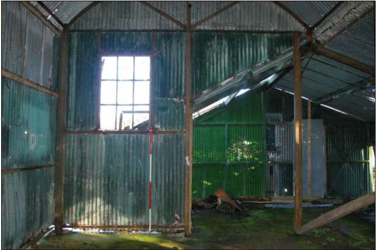
Figure 124: The east wall of B1; viewed from the west (scale 1m).
