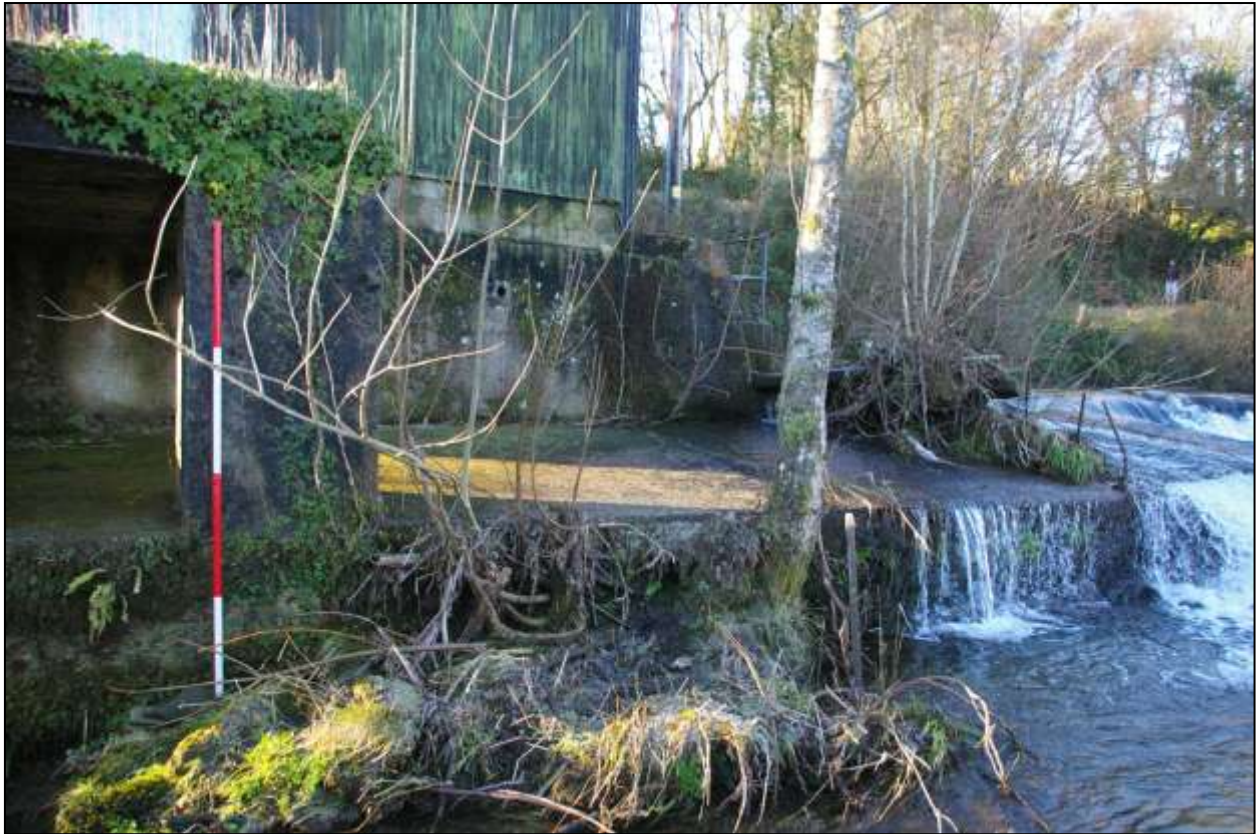
Figure 61: The spillway, viewed from the east (scale 2m).
