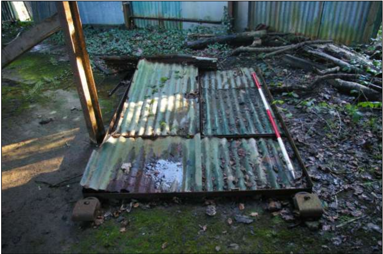
Figure 130: The former door (scale 2m).
