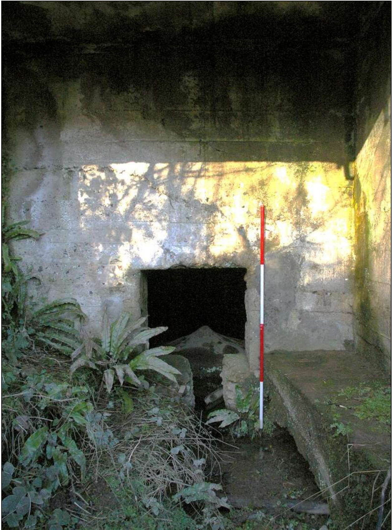
Figure 77: The south wall of the turbine chamber, showing the opening; viewed from the south (scale 2m).
