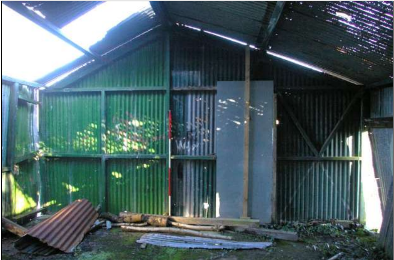
Figure 122: The east wall of B2, viewed from the west (scale 2m).
