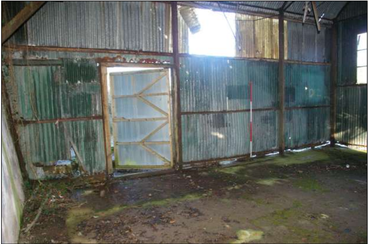
Figure 126: The north wall of B1, viewed from the south-west (scale 2m).
