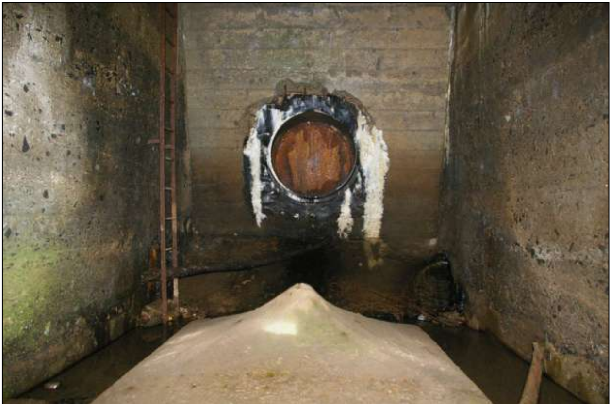
Figure 84: The interior of the turbine chamber, viewed through the opening in the south wall (no scale).
