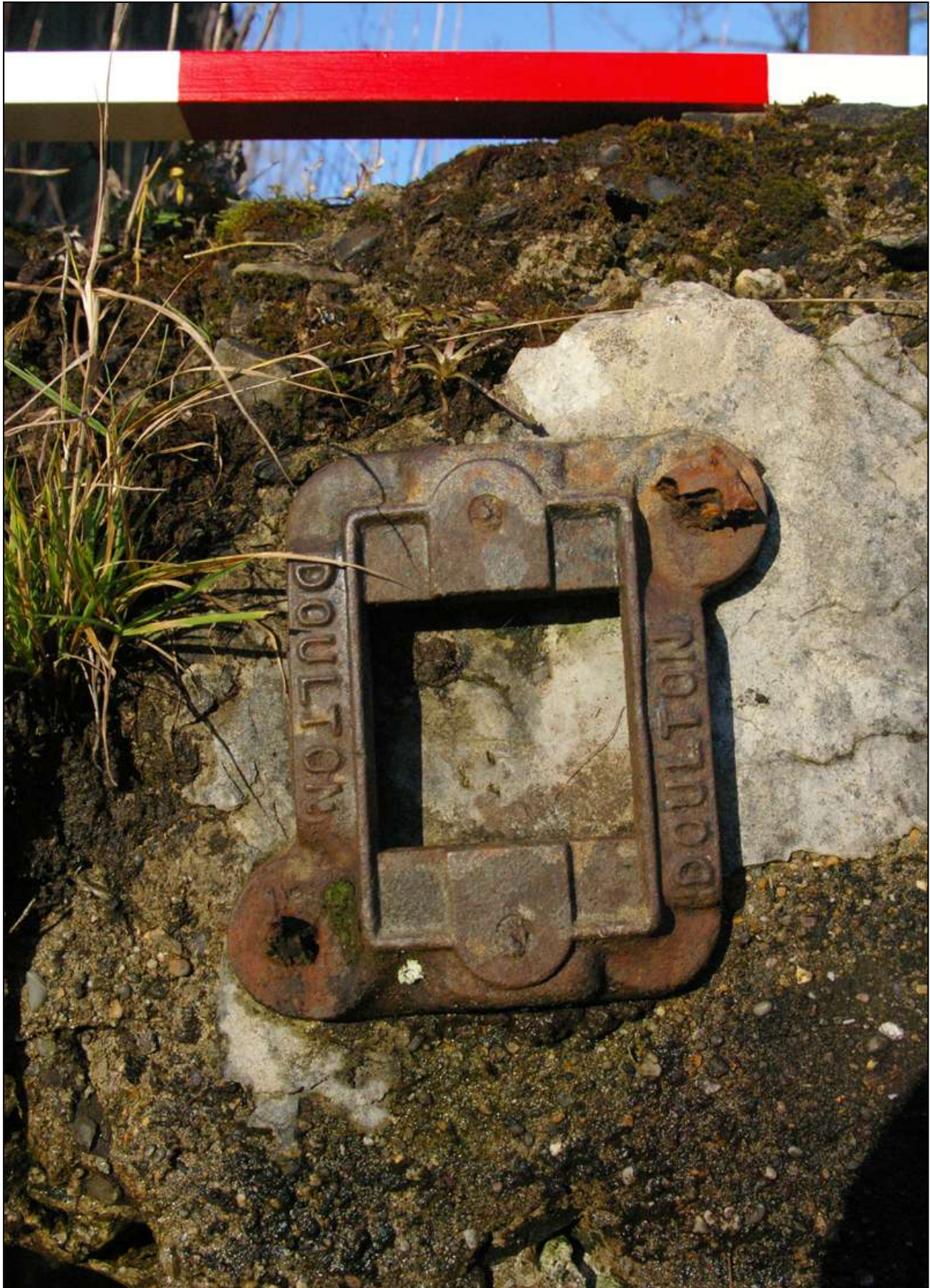
Figure 69: Detail of one of the DOULTON brackets (scale 1m).
