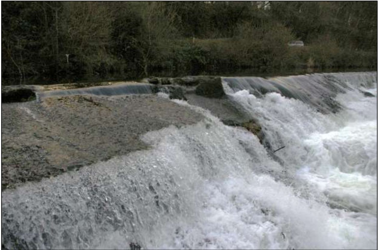
Figure 41: As above, viewed from the SSE (no scale).
