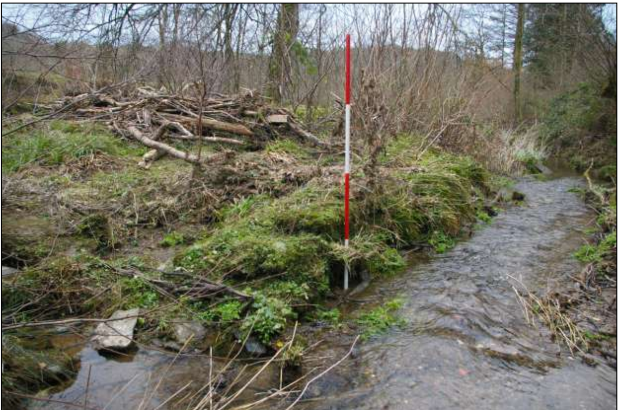
Figure 105: The ragged end of the wall flanking Leat 3, just south of the fish tanks; viewed from the NNW (scale 2m).
