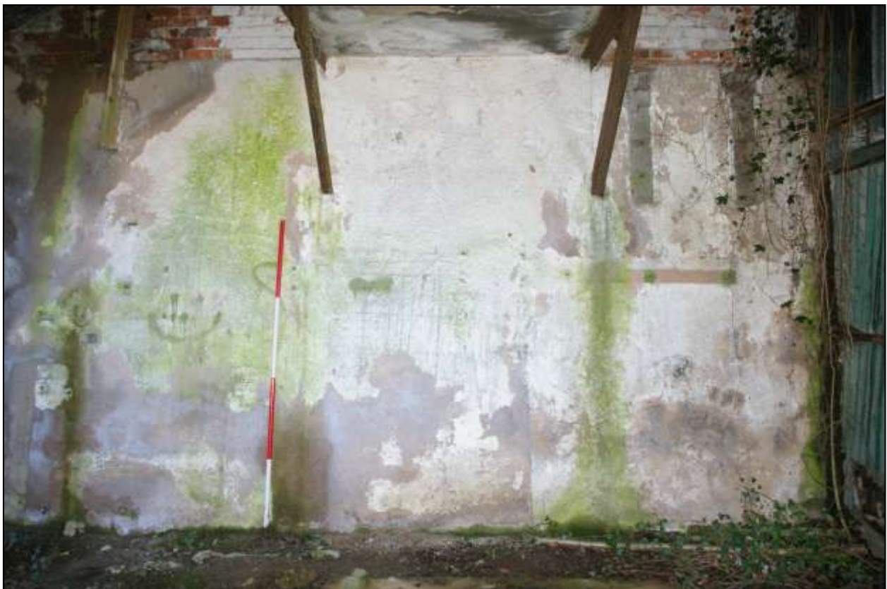
Figure 116: As above, showing detail of the west wall (scale 2m).
