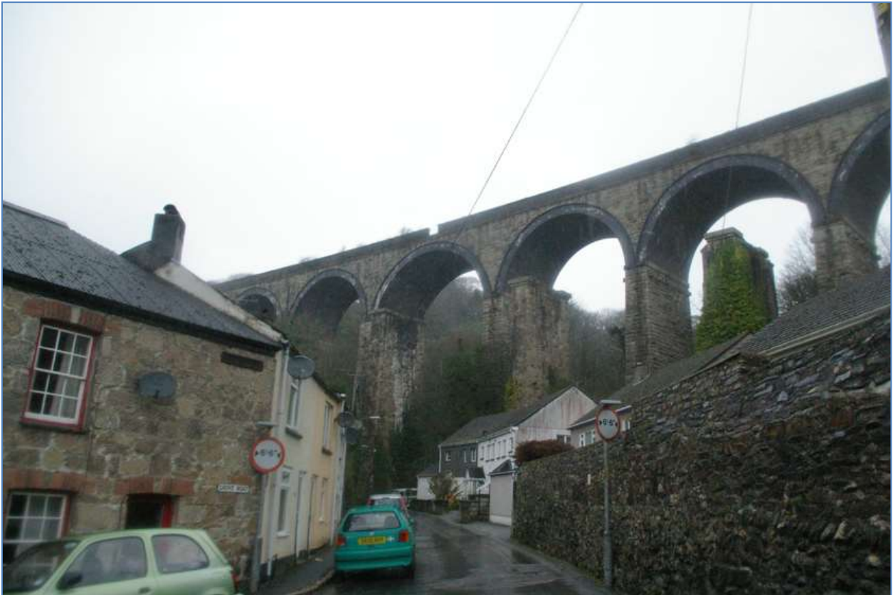
The Gover valley viaduct; from the south-east
