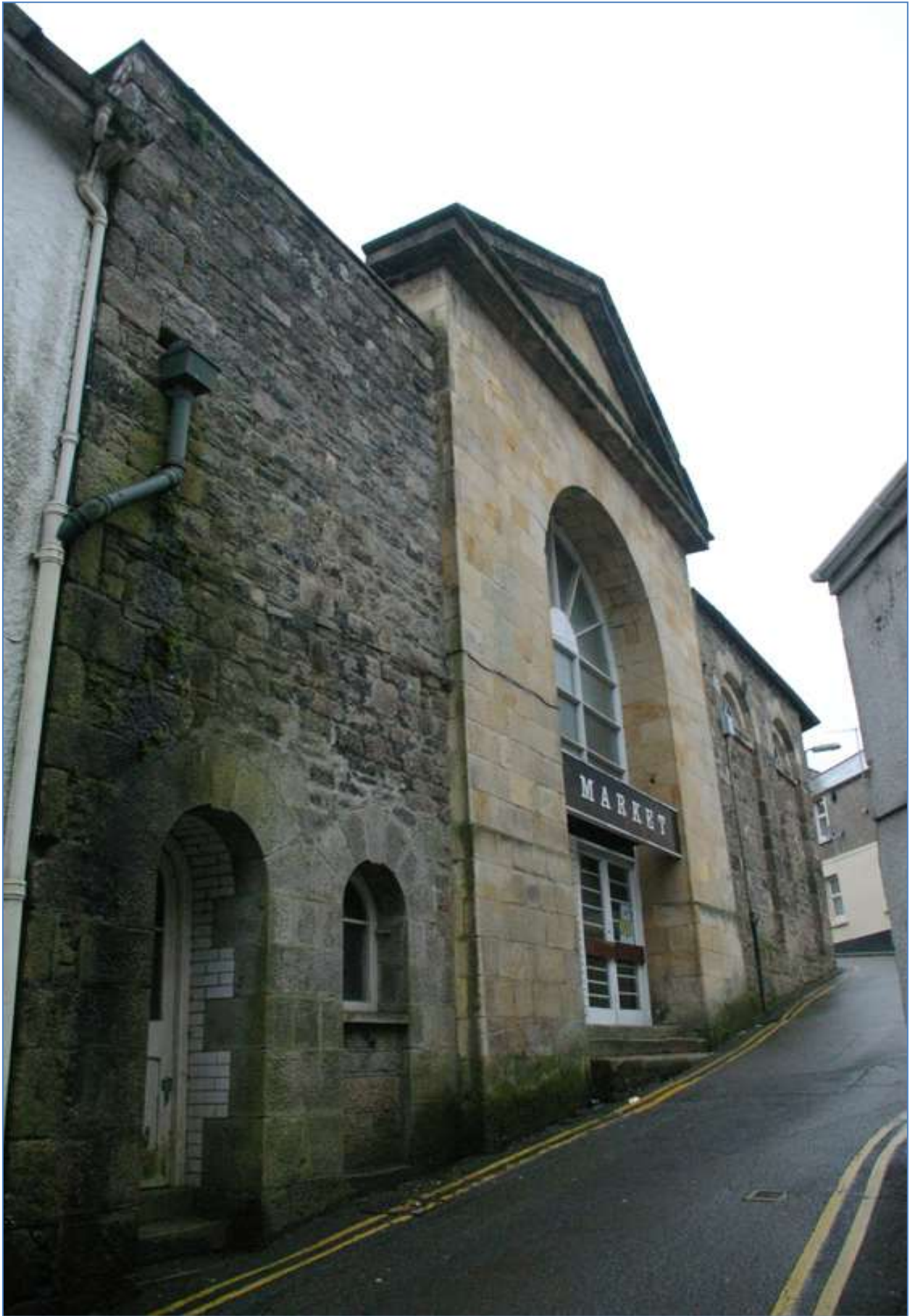
The Market House in St Austell; from the north-west.
