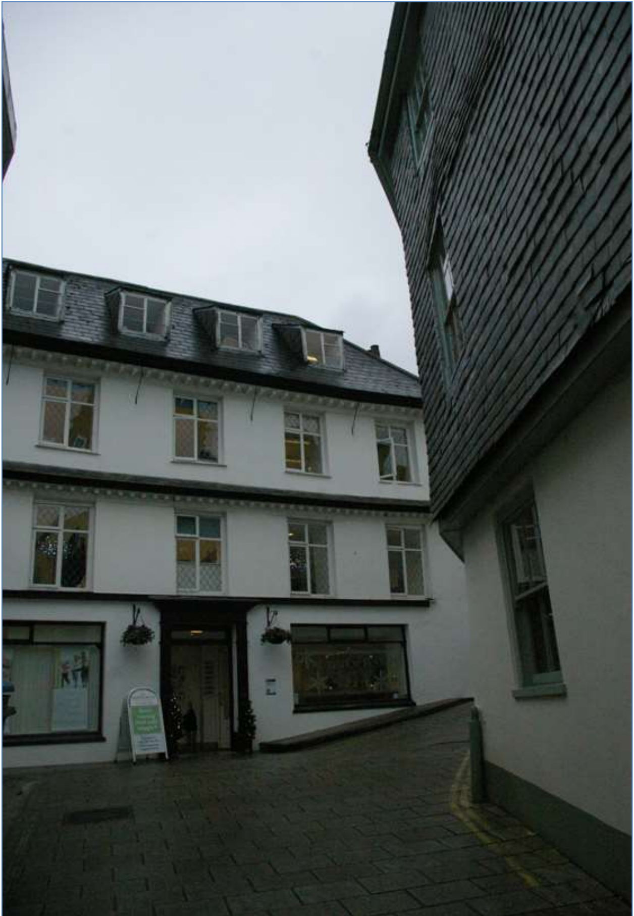
Wheal Martyn, main buildings; from the south-east.
