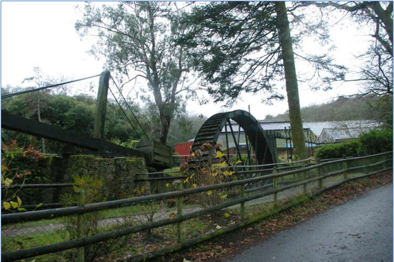
Waterwheel/beam engine at Wheal Martyn; from the east.
