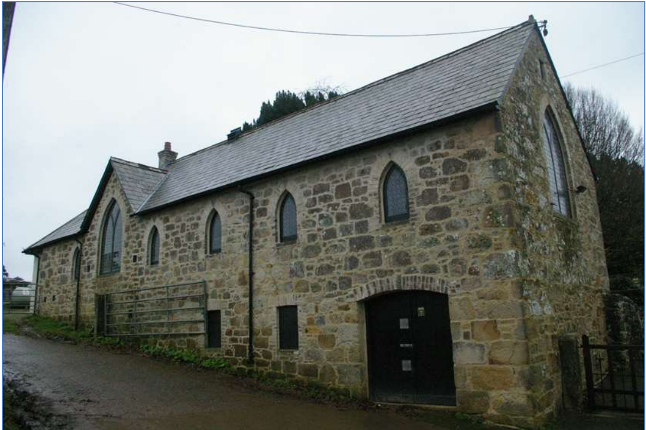
St Mewan Sunday School; from the west, north-west.
