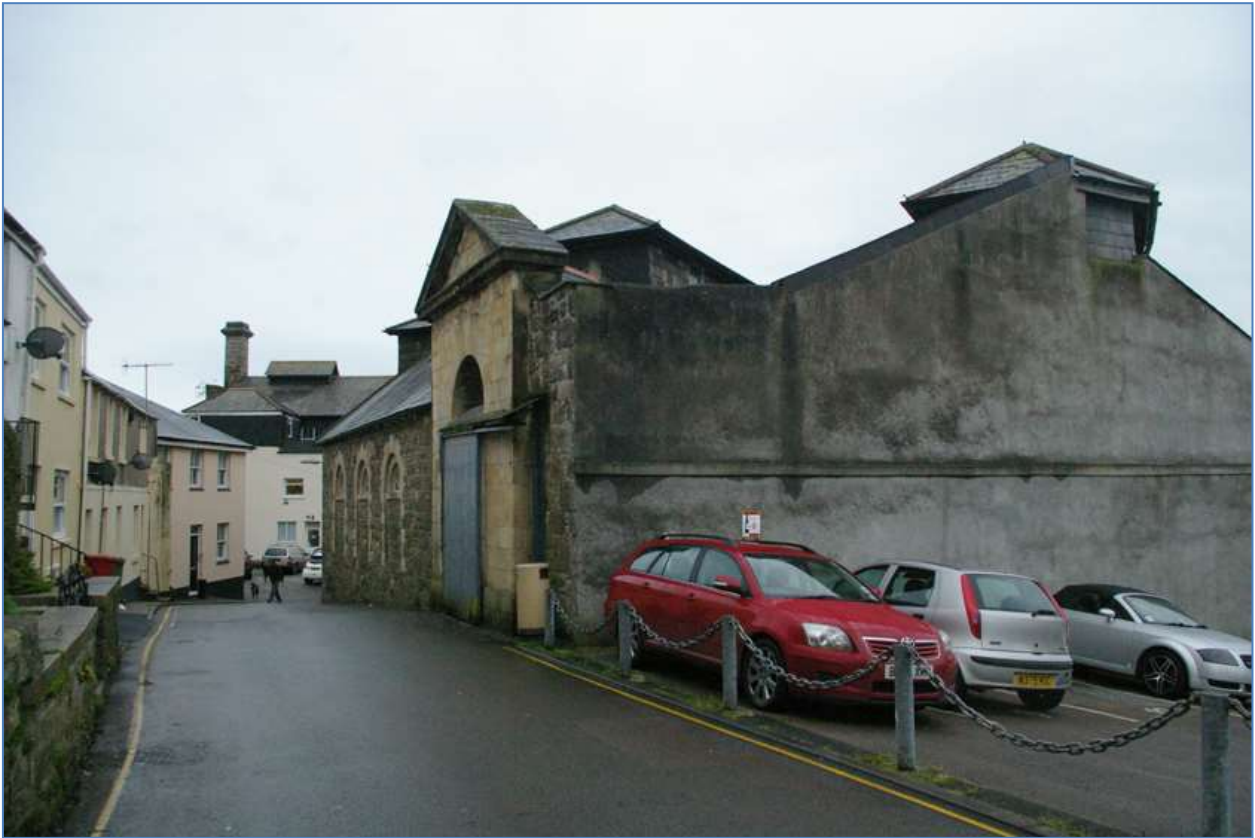
The Market House in St Austell; from the north-west.
