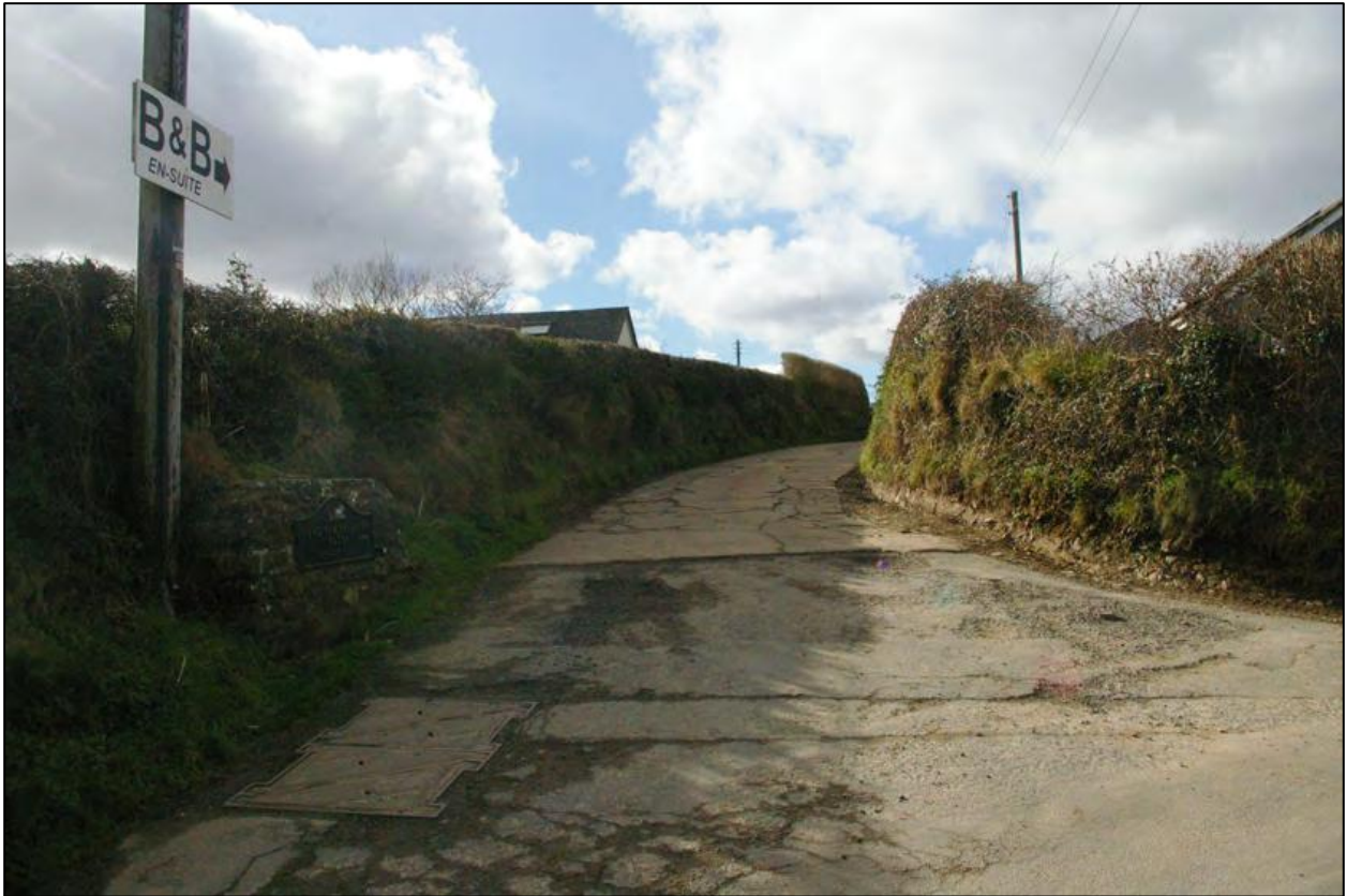
The long driveway to West Goldworthy farm; from the east.
