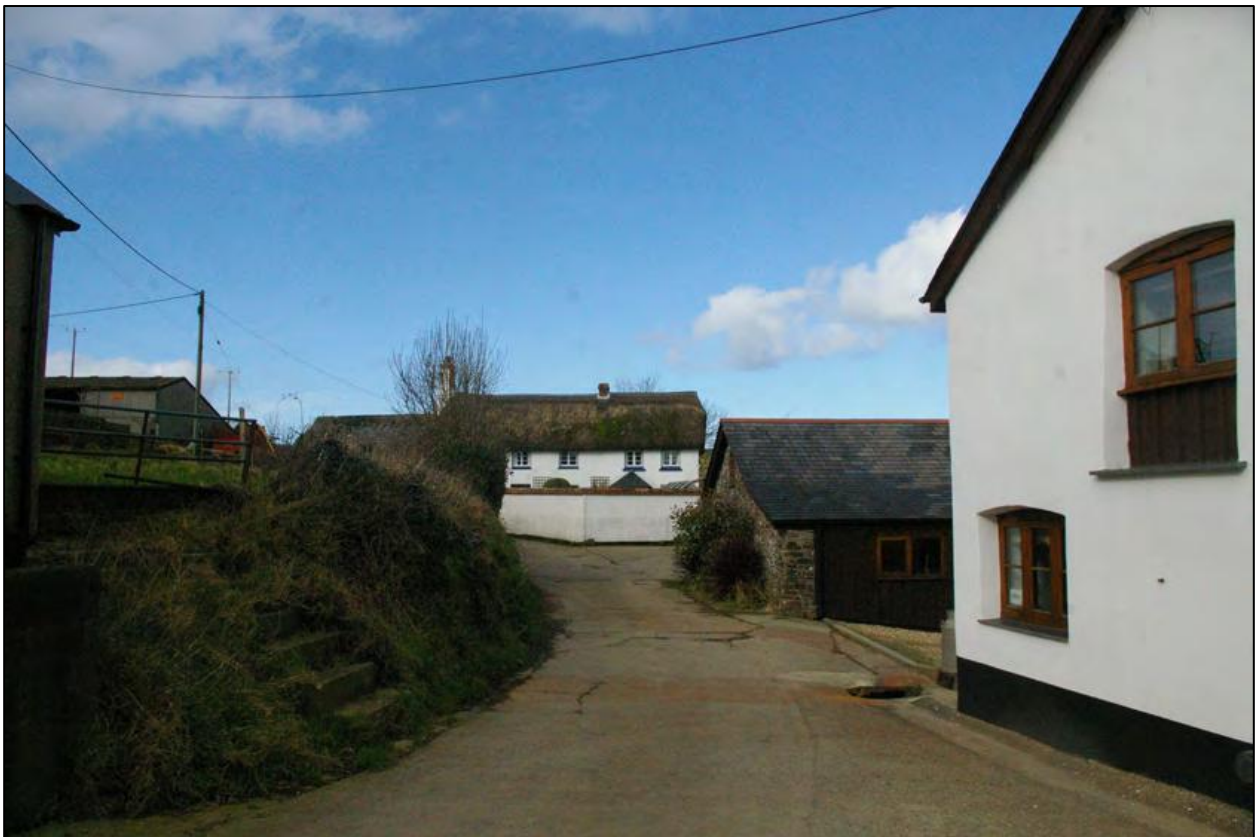
Kingsland Cottage at Goldworthy; from the south, south-west.
