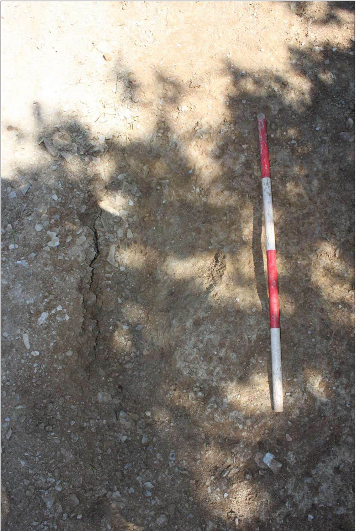
Shot of Pit [105], area to the left is the filled in service trench, viewed from the south (1m scale).
