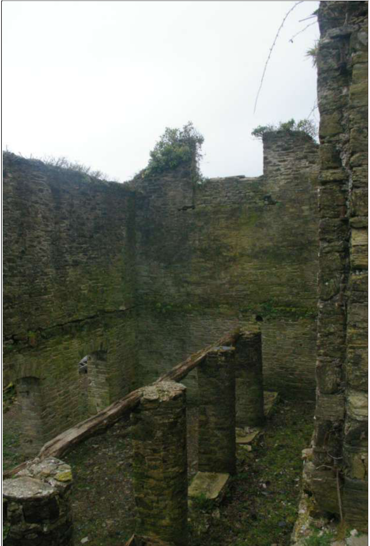
The west elevation; viewed from the north-east.
