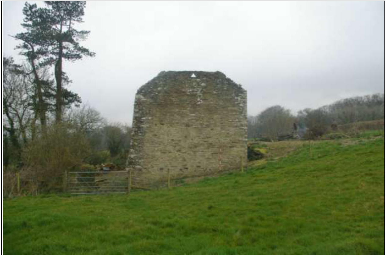
The east elevation; viewed from the east (2m scale).
