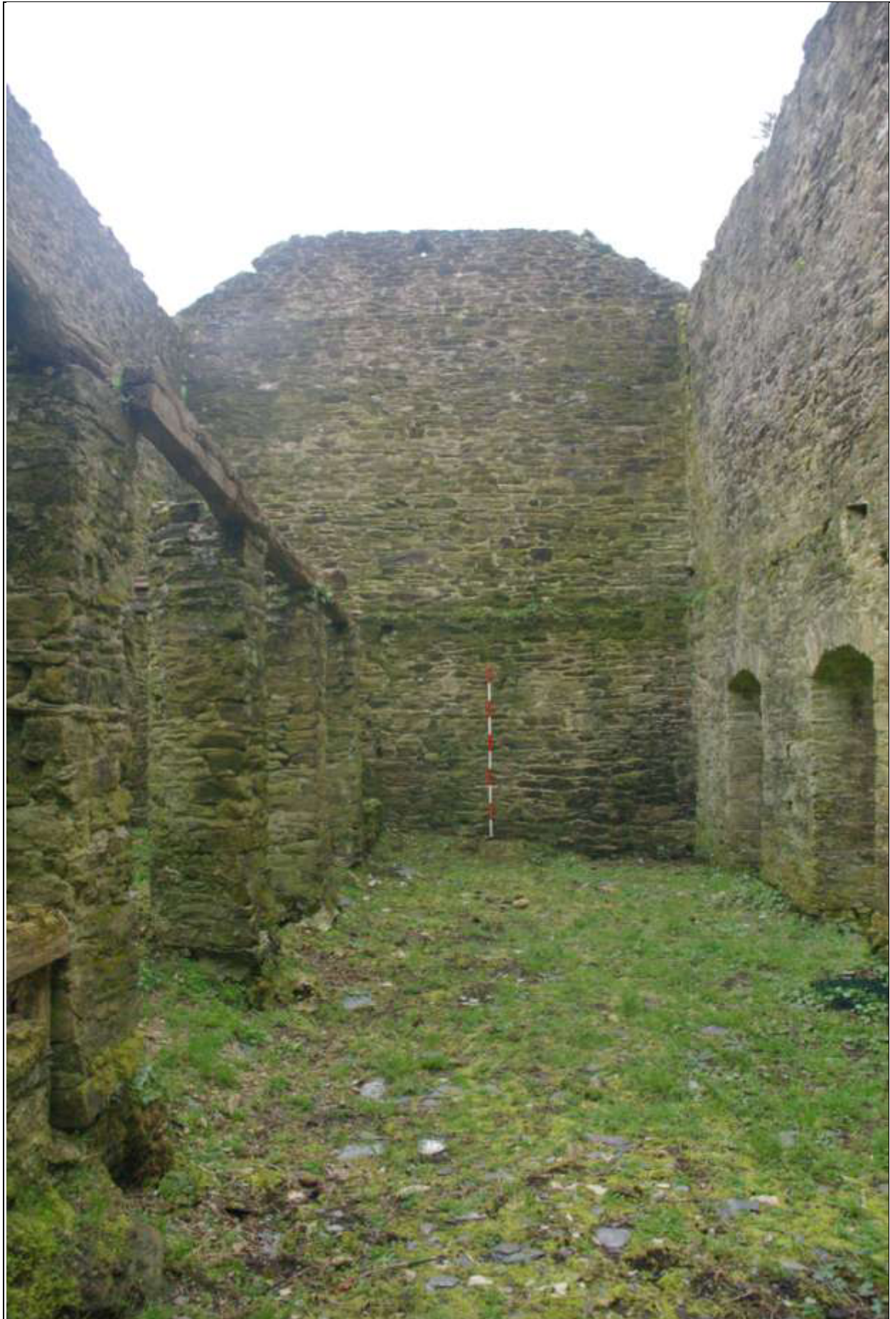
The east elevation, interior face; viewed from the west (2m scale).
