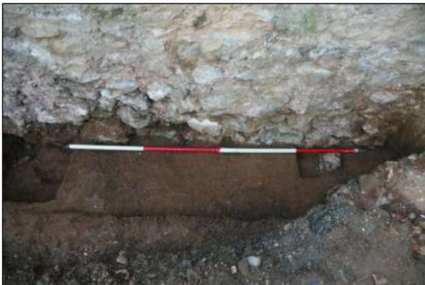
Southern foundations of north aisle and grave cuts; viewed from the west (2m scale).
