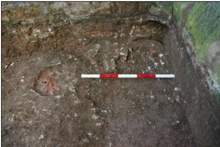
Disturbed area where the tower meets the north aisle; viewed from the west (1m scale).
