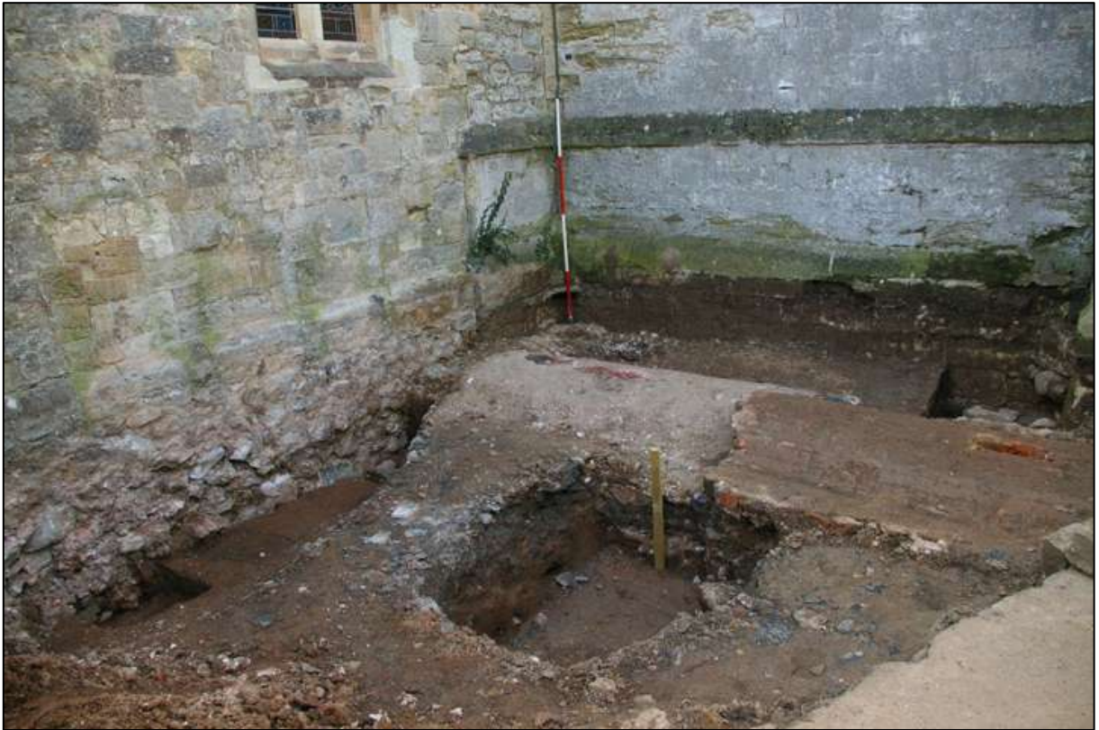
Figure 3: Site shot mid excavation; viewed from the north-west (2m scale).
