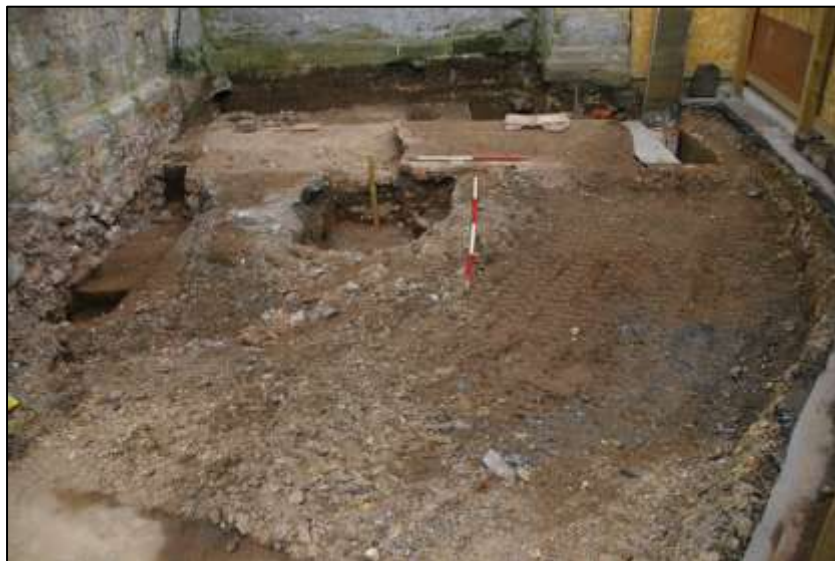
Site shot, mid-excavation; viewed from the north (1m & 2m scale).
