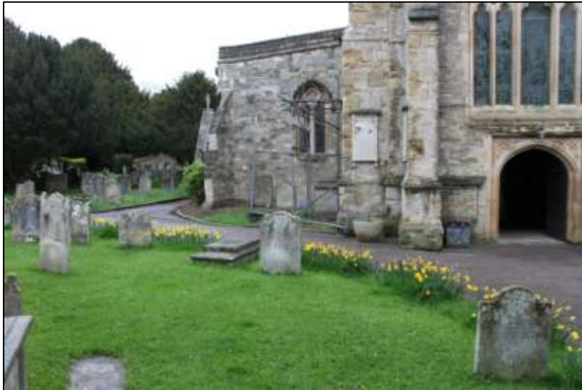
Tower and west end of north aisle, pre-excavation; viewed from the south-west (no scale).
