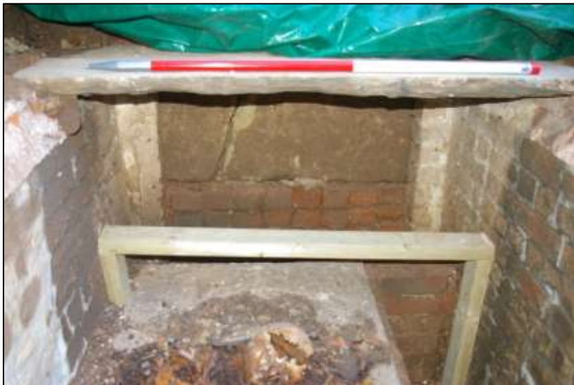
West end of Barrel tomb {107} opened; viewed from the east (1m scale).
