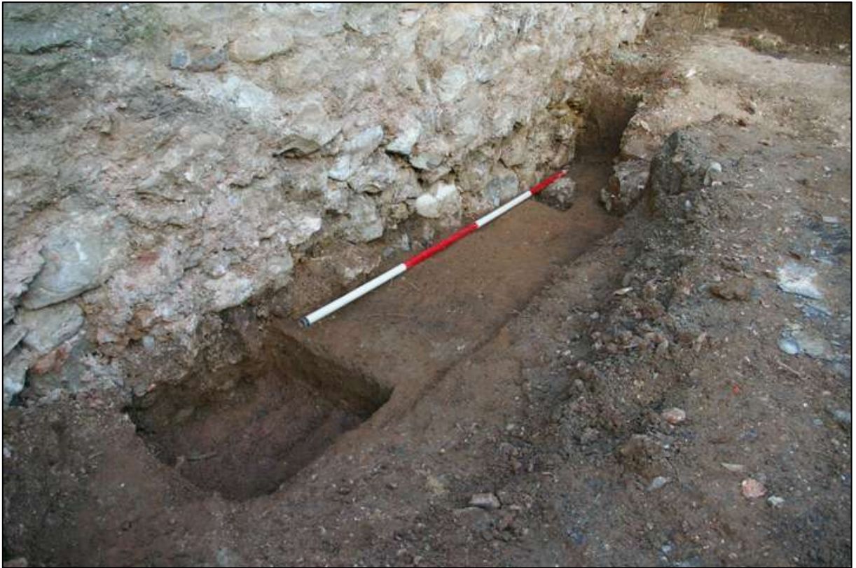
Figure 4: Southern foundations of north aisle and grave cuts; viewed from the north-west (2m scale).
