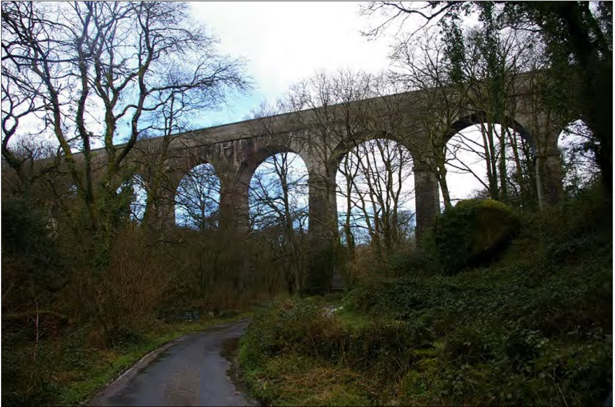
Luxulyan Valley (WHS) with the Treffry viaduct; from the south-south-east.
