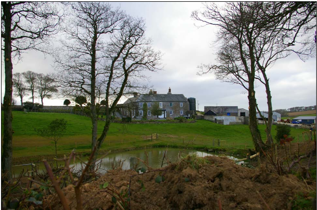
Eastleigh Manor, garden walls and associated barns and buildings; from the east.
