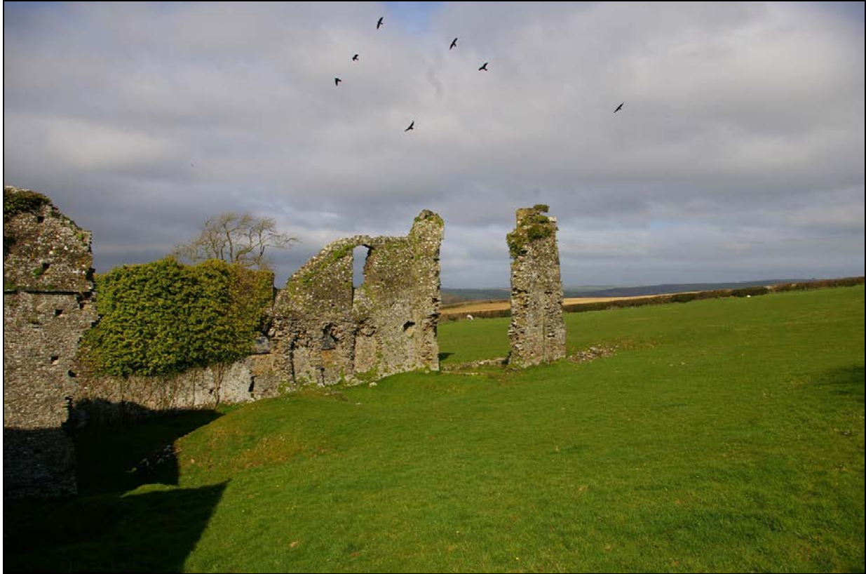
Frithelstock Priory remains, a scheduled monument, showing the wide views to the east and north-east down the valley; from the south-west.
