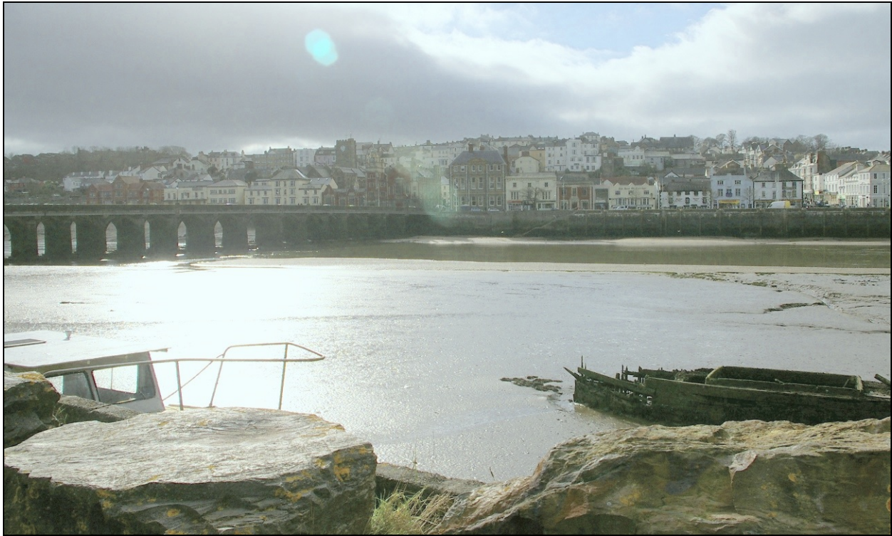
St Mary's church, Bideford medieval bridge and other listed buildings within the town, view across the river from the east side; from the north-east
