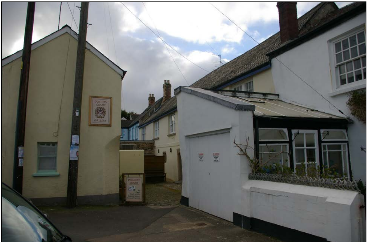
Docton Court in Appeldore, showing local blocking factors within the town; from the south-east.
