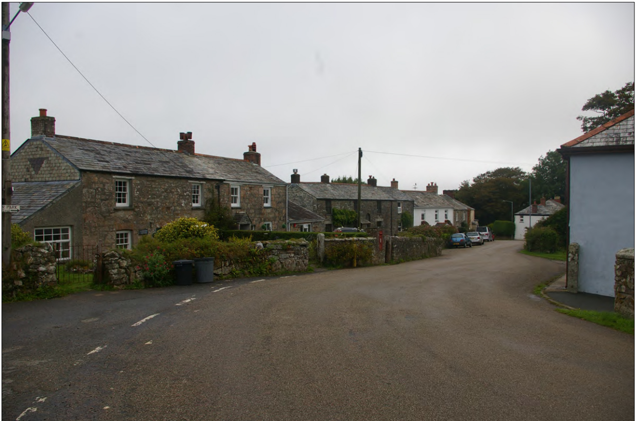
View of the north side of the main street in Withiel, with the row of Listed cottages; from the south-west.
