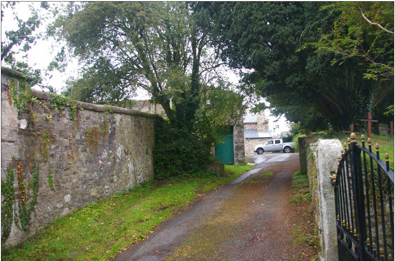
Shot of the service ranges and farm buildings to the north & north-west of Withiel House; from the east.
