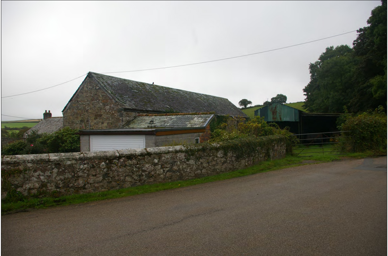
View of cottages and barns within the village of Withiel, to the east of the church; from the north-west.
