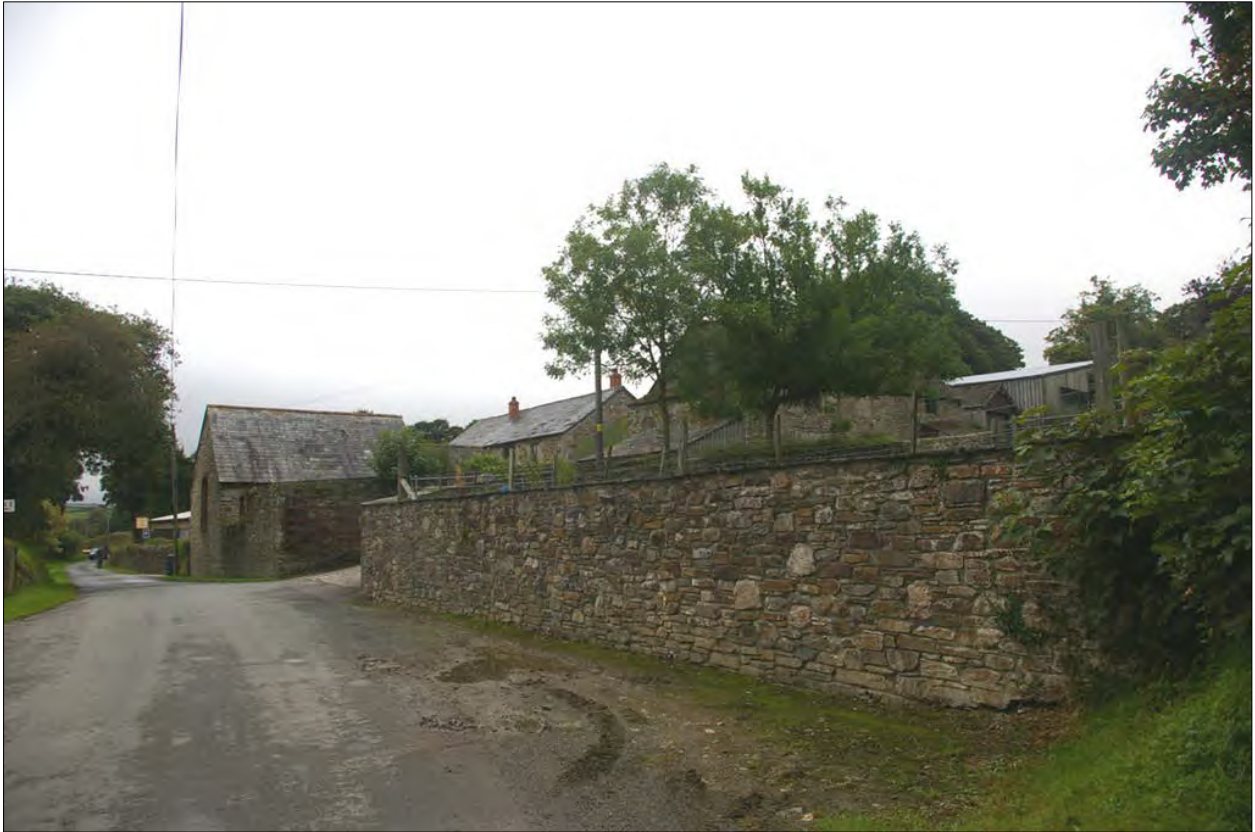
View of Tregolls Farm, with all of its buildings; from the south-east.
