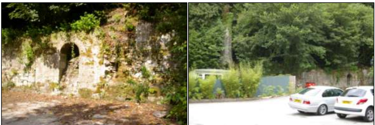
Figure 6: Remains of the Higher Blowing House; viewed from the north-east (no scale).
