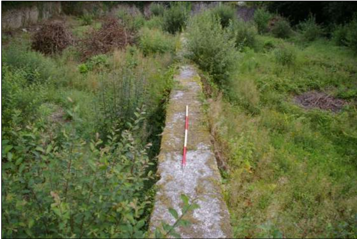
Dividing wall of settling tanks; viewed from the south (2m scale).
