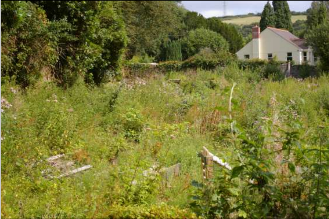
Site shot, concrete drag visible in centre with debris to the left; viewed from the south (no scale).
