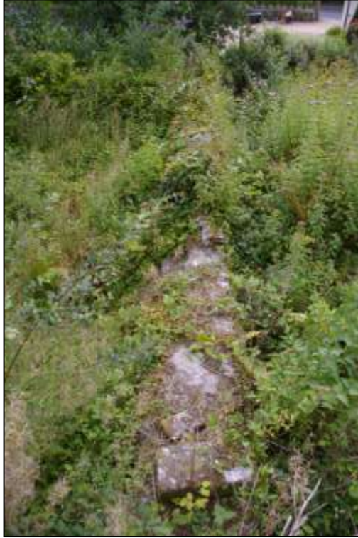
South wall of eastern settling tank; viewed from the west (no scale).
