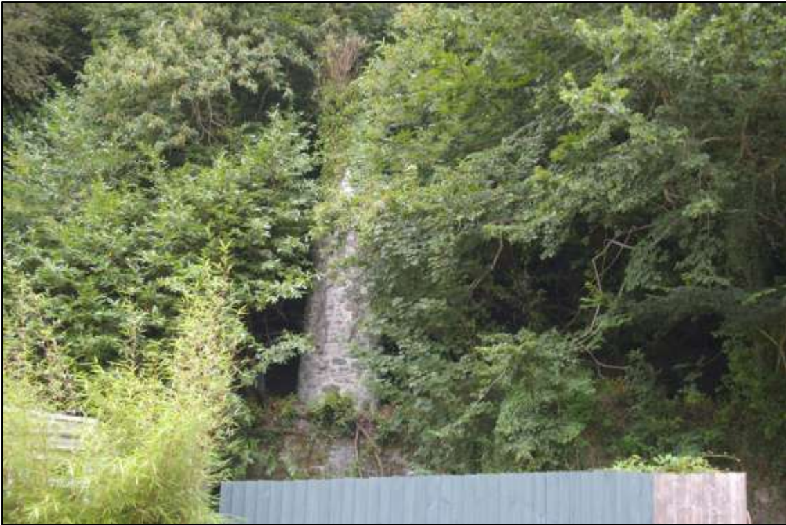
Chimney stack of demolished/infilled Higher lowing House pan kiln; viewed from the north-east (no scale).
