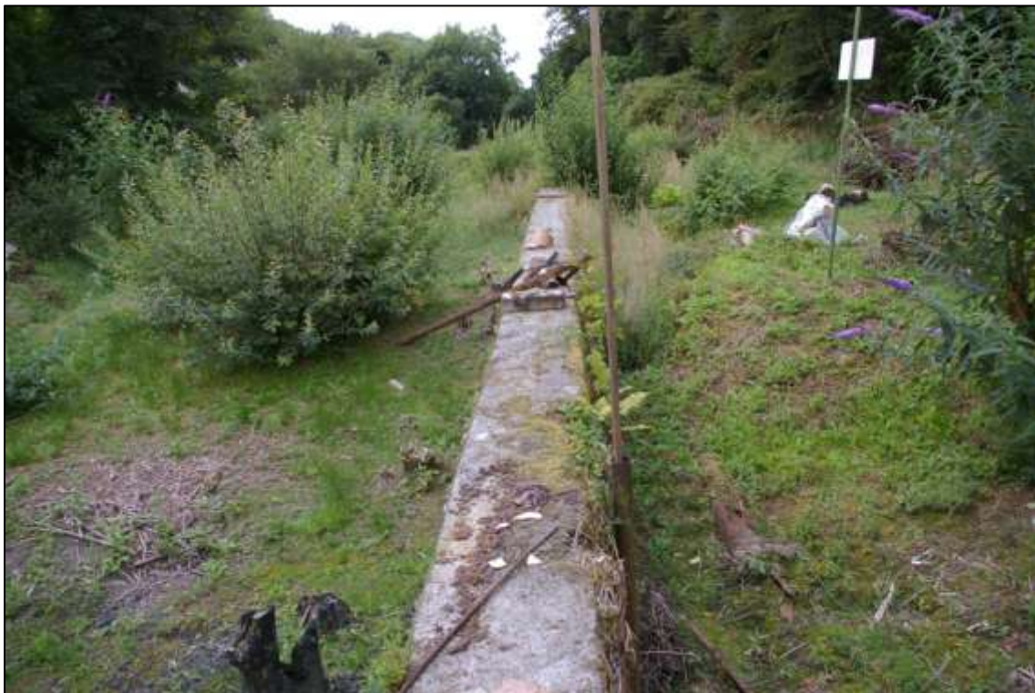
Settling tanks dividing wall; viewed from the north (no scale).
