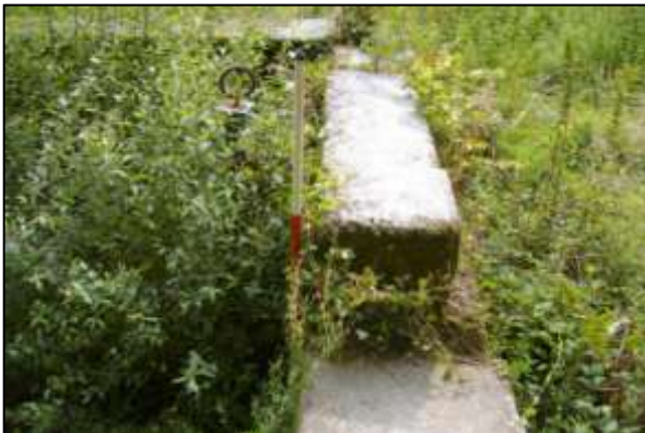
Figure 15: Shot of sluice; viewed from the west (2m scale).
