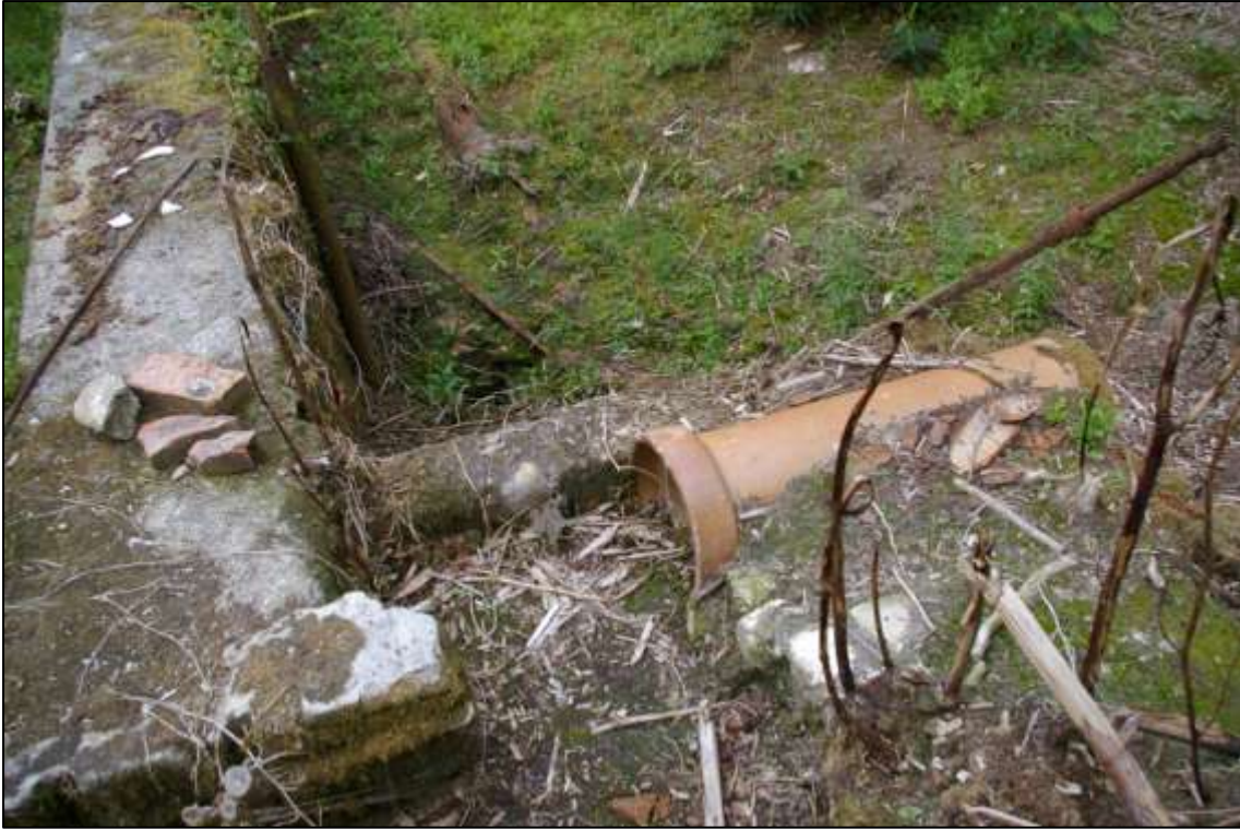
Salt glazed and Fe pipe work in north-east corner of western settling tank; viewed from the north (no scale).
