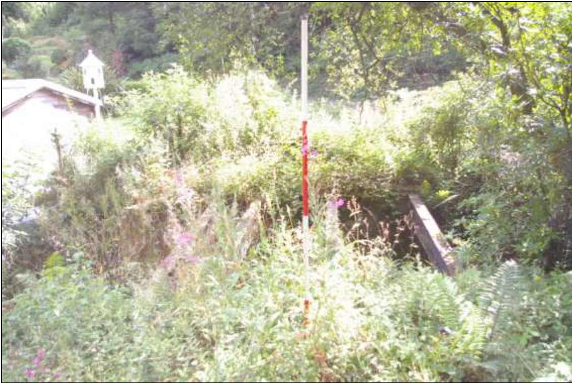
Derelict bridge; viewed from the west (2m scale).
