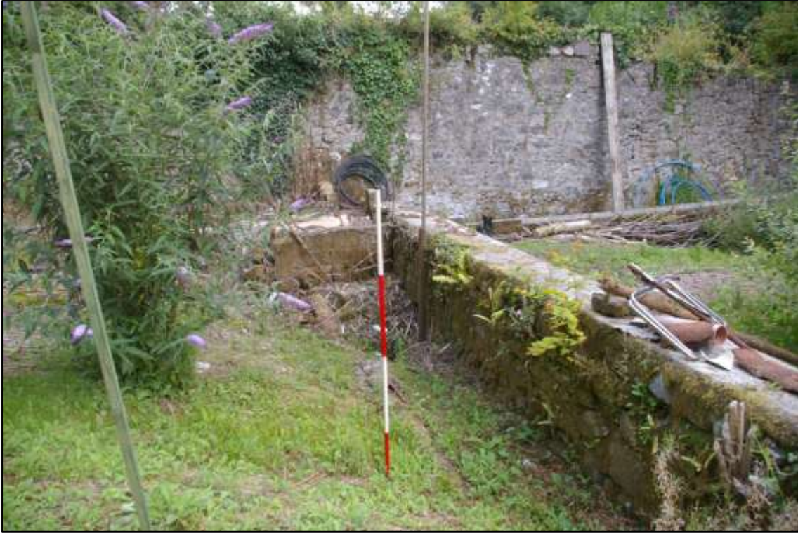
North-east corner of western settling tank, showing pipe work; viewed from the south-west (2m scale).
