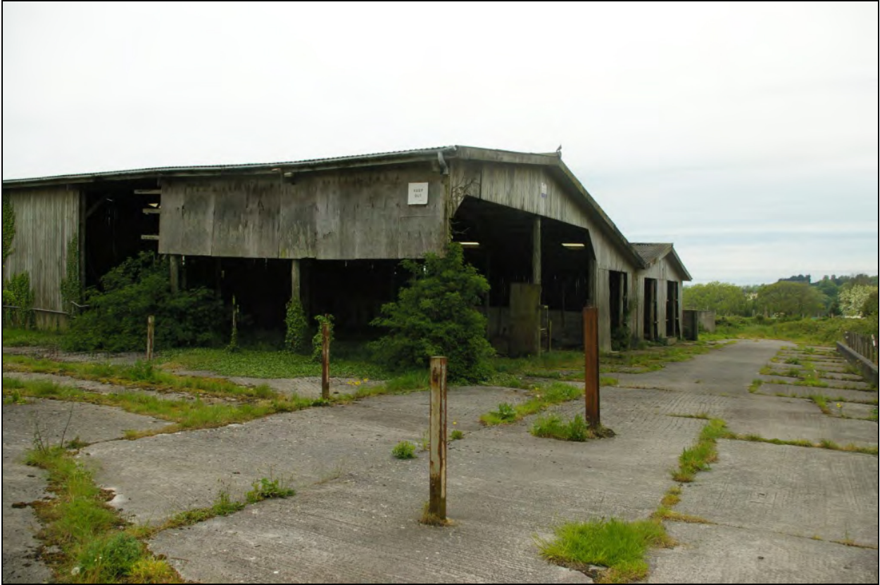
Large cow sheds within the proposal site, viewed from the east-north-east.
