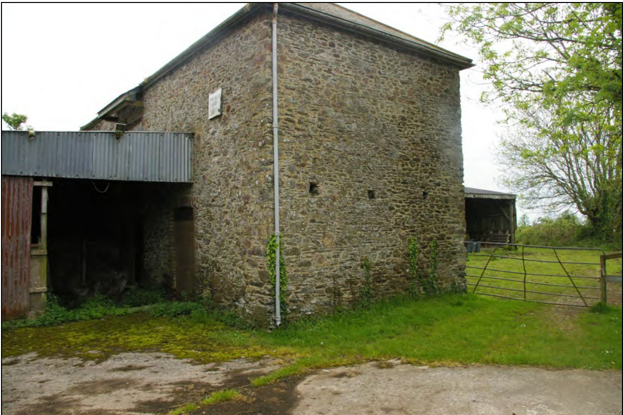
The historic barn within the proposal site, viewed from the north-east.
