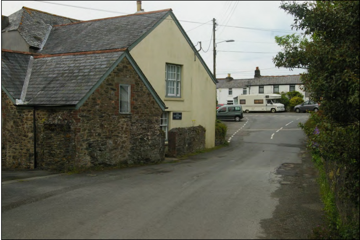
Old Churchtown Farm, at the northern end of Church Lane, viewed from the south-south-east.
