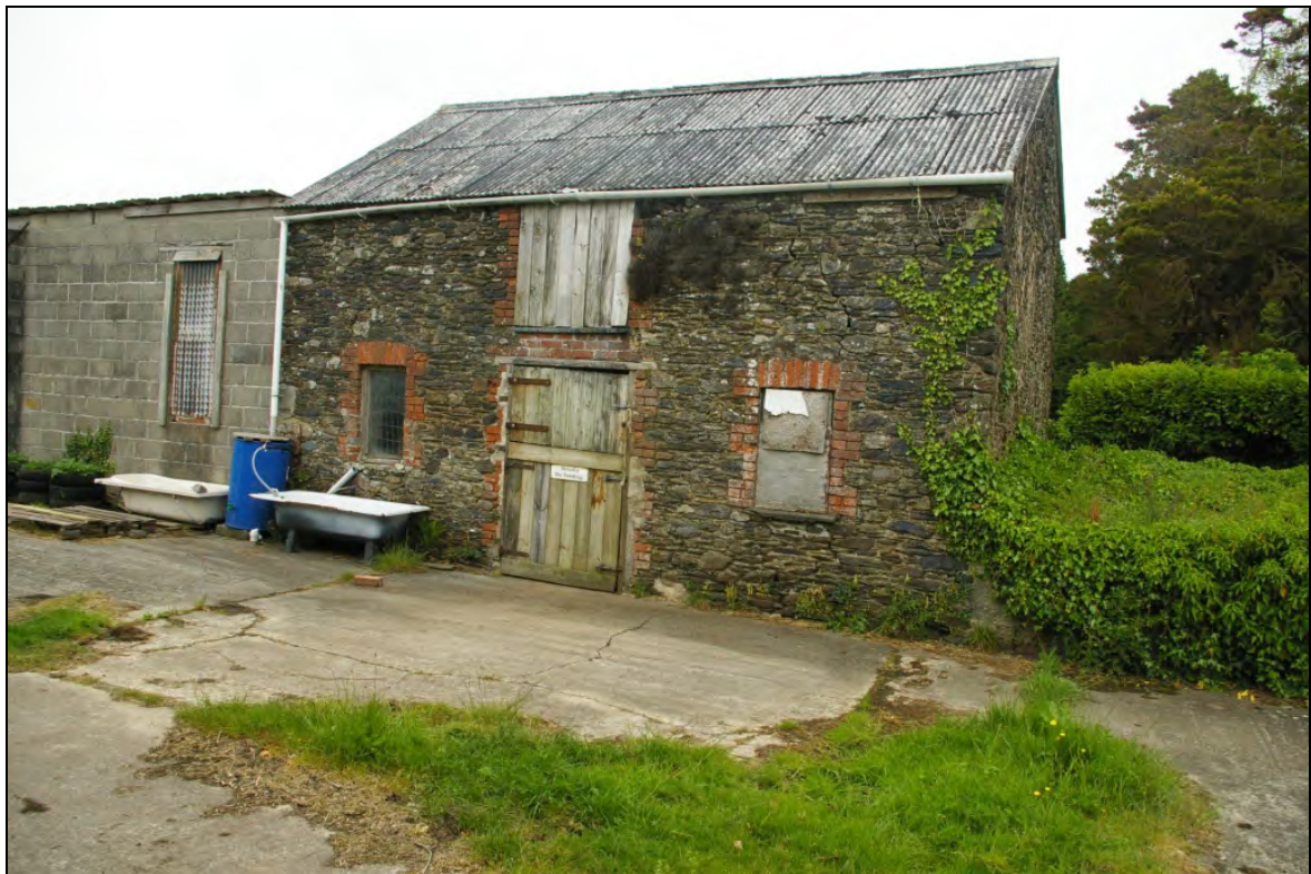
Figure 6: Shot of stable on the northern edge of the development site, viewed from the south.
