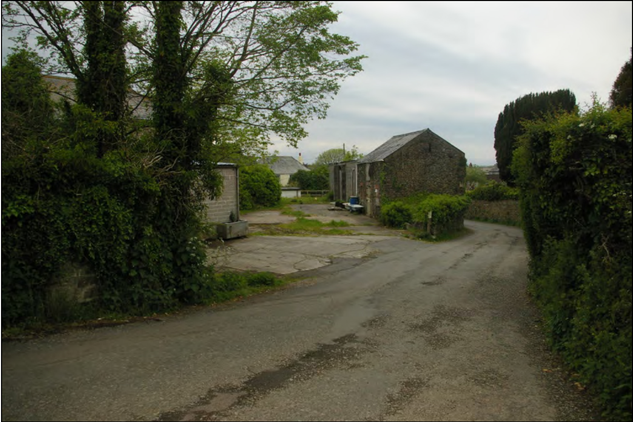
View of the main entrance to the site presently, with Hobbs Cross is visible beyond, viewed from the south-east.
