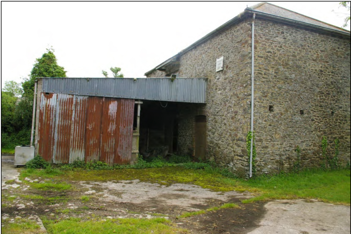
Figure 7: Shot of the barn, viewed from the north.
