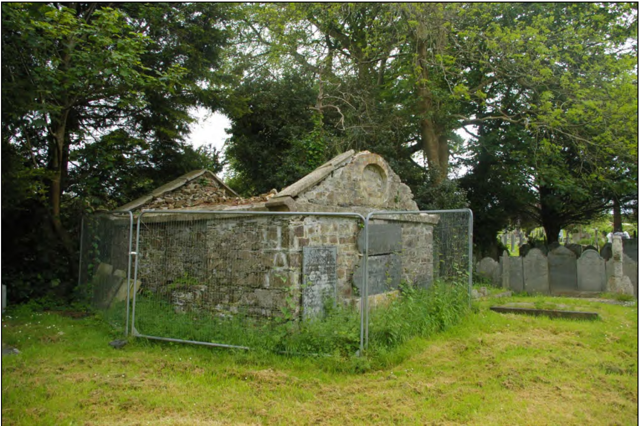
Shot of the Grade II Listed family vault in south-east of the churchyard, viewed from the north-west.
