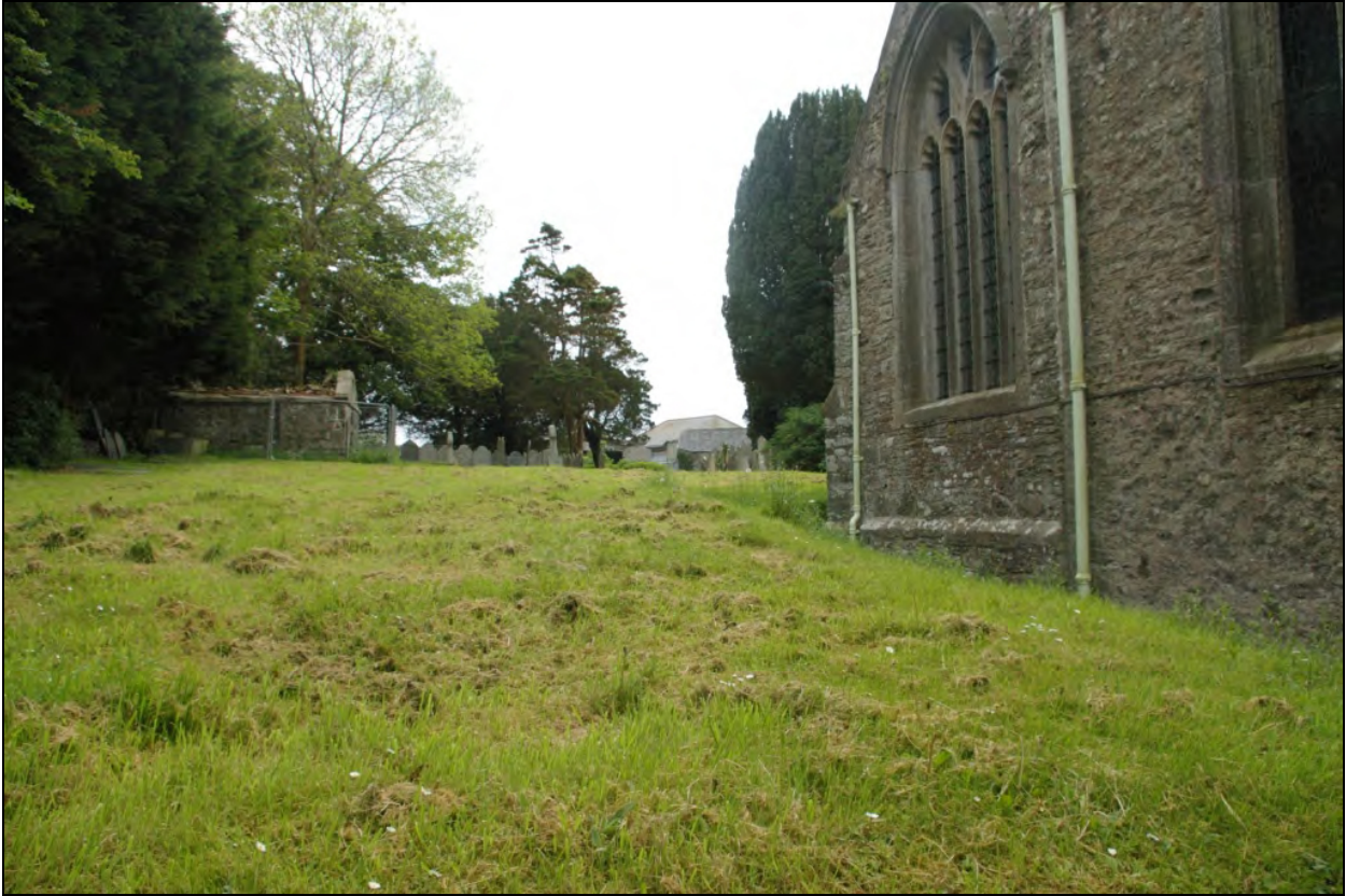
Shot of the churchyard, including the Grade II Listed family vault in south-east of the churchyard, viewed from the north.
