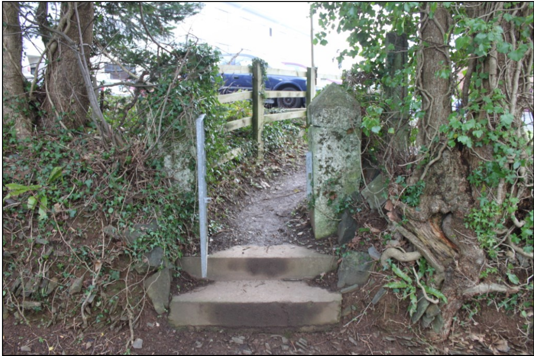
Figure 16: Gateway and steps forced into the eastern hedgebank of the footpath, viewed from the west (no scale).
