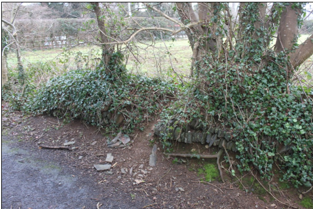
Figure 12: The only stone facing surviving in the western boundary, viewed from west (no scale).
