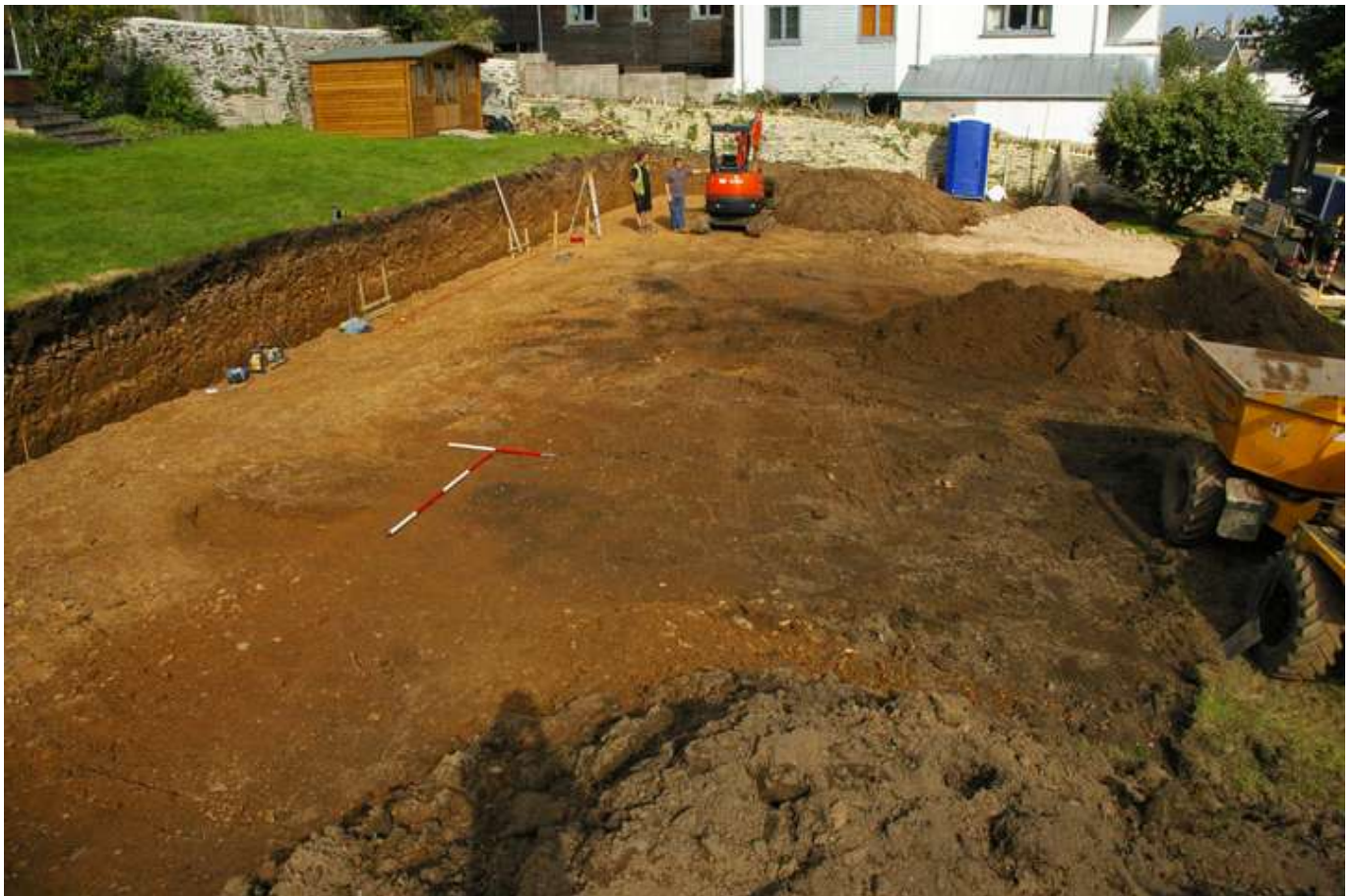
Figure 1: Site shot post-excavation; looking north-west (1m & 2m scale).
