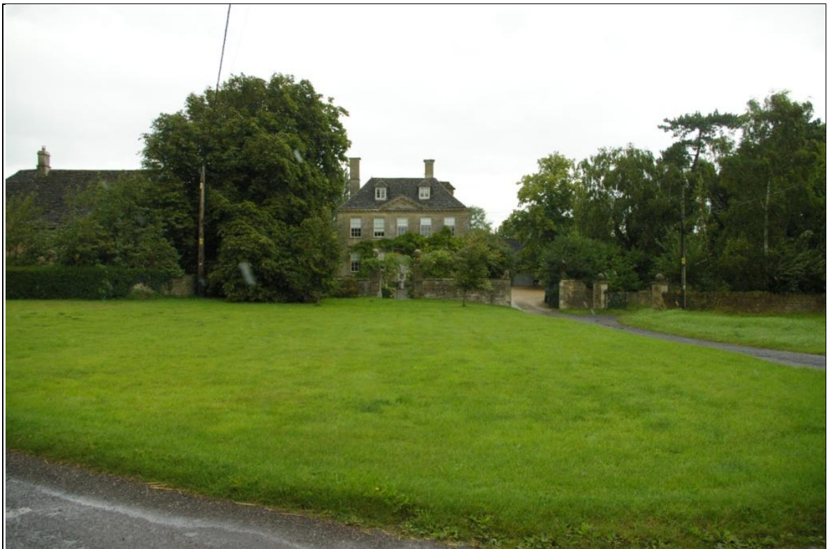
Figure 3: The primary, southern, elevation of Gifford Hall, viewed from the south.
