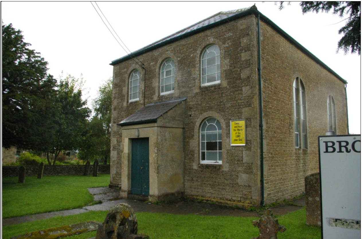
Broughton Gifford Baptist Chapel, viewed from the south-west.
