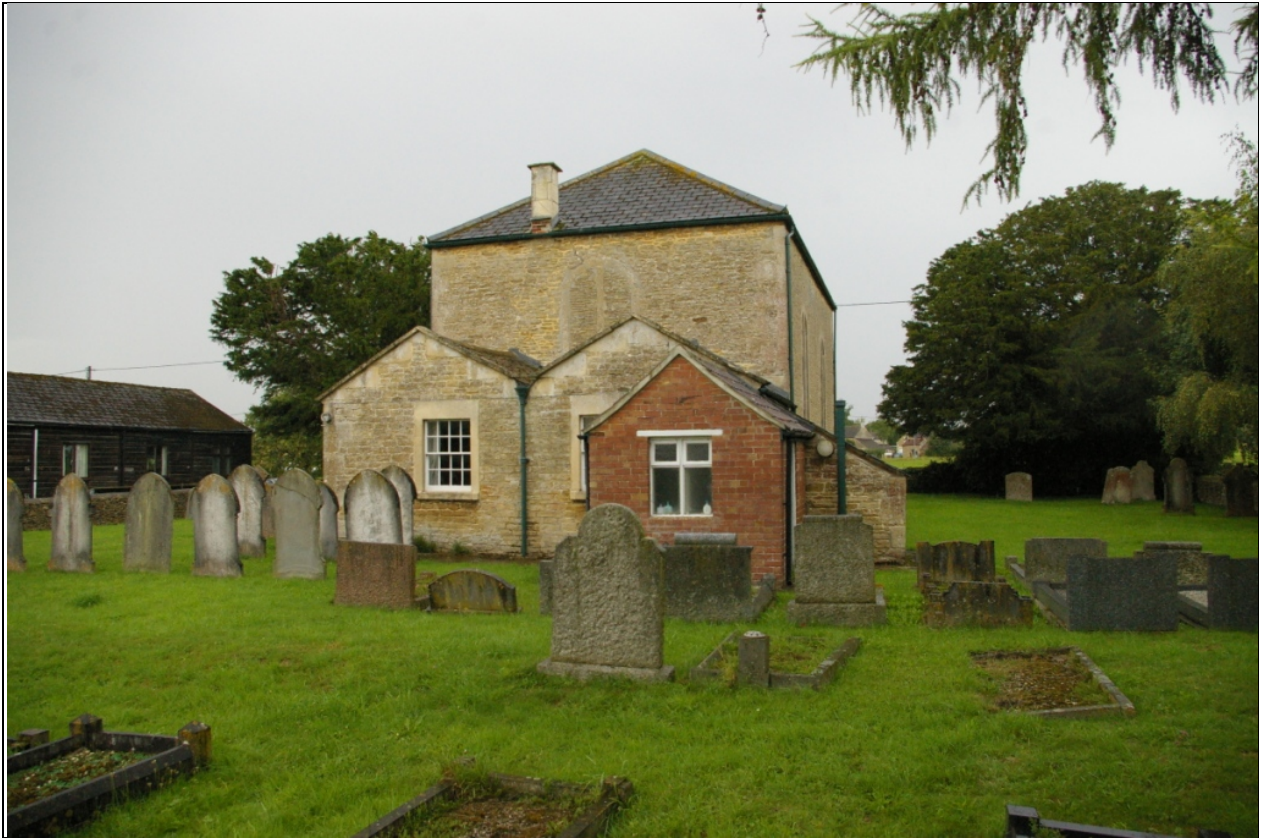
Broughton Gifford Baptist Chapel's 19 th and 20 th century additions, viewed from the east.
