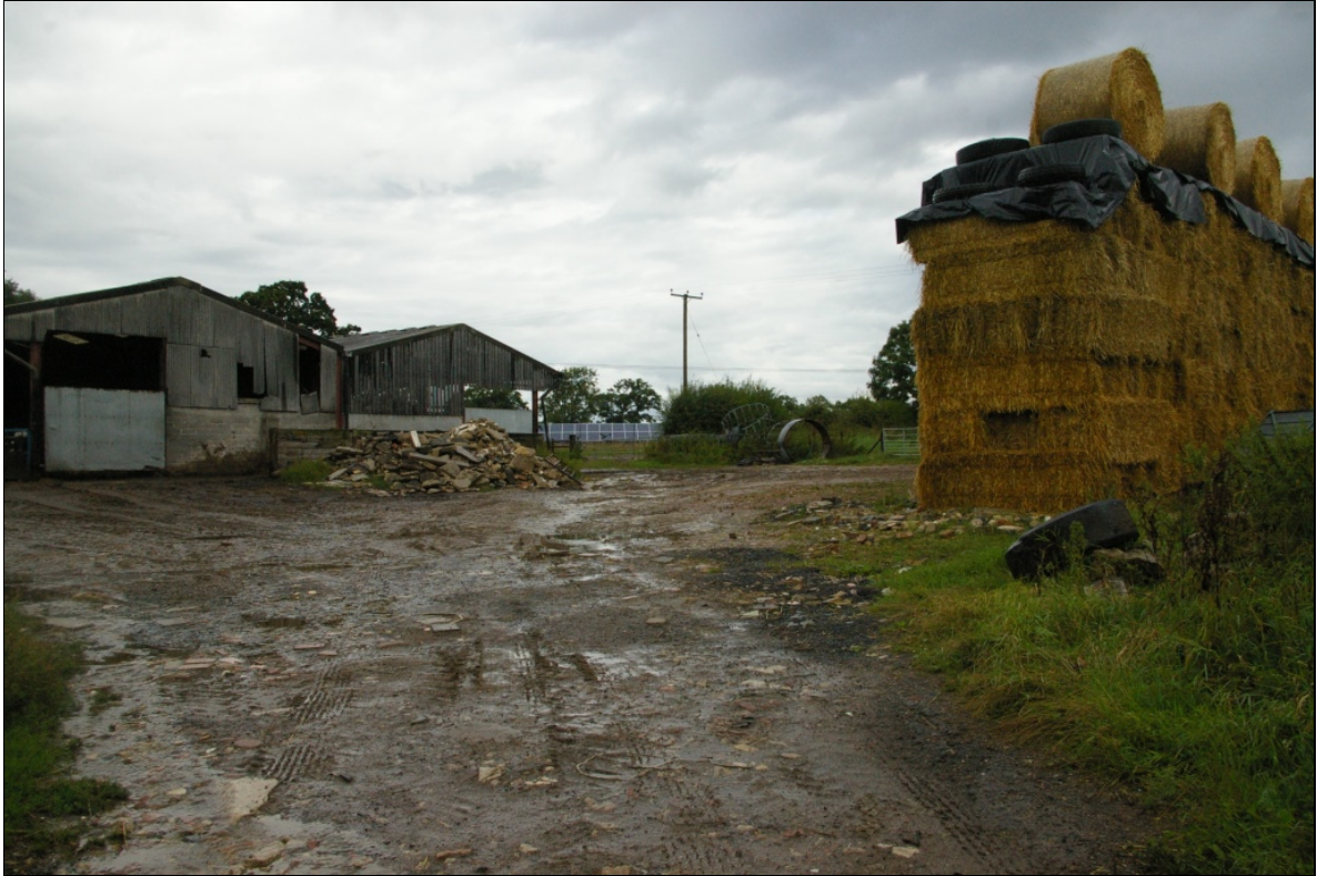
Figure 4: View towards the existing solar site from the public footpath located at the northern end of the conservation area, viewed from the south.
