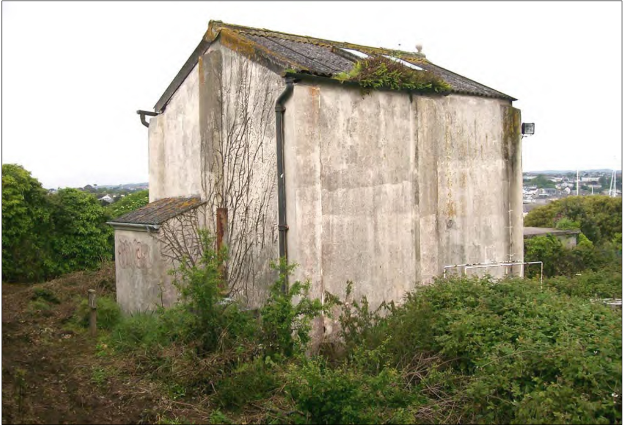
The pump house; viewed from the east.
