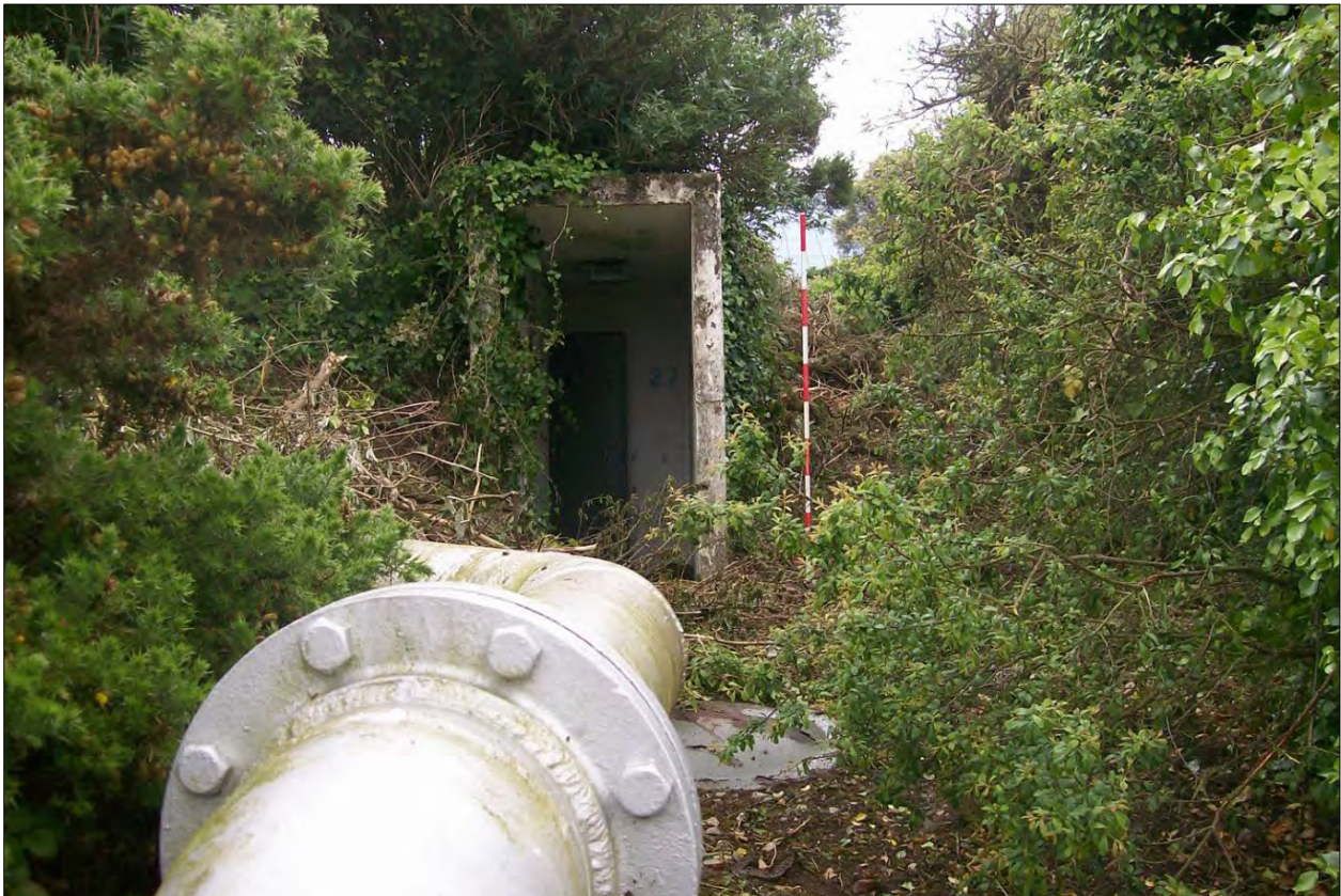
The entrance to the west tank, south side of fuel depot; viewed from the north-west (scale 2m).
