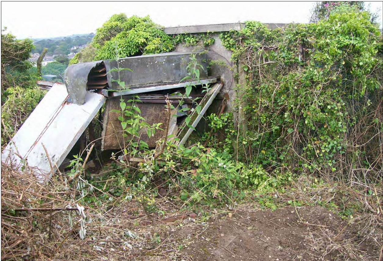
Ancillary building; viewed from the north-east.
