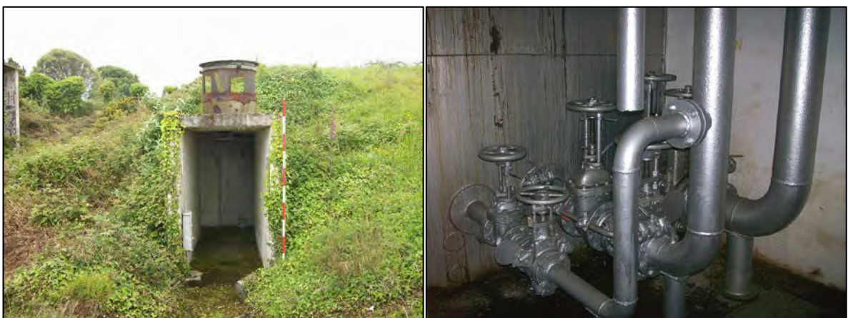
Figure 18: Entrance to the western tank; viewed from the north (2m scale). Figure 19: Inside the western tank; viewed from the north-east.
