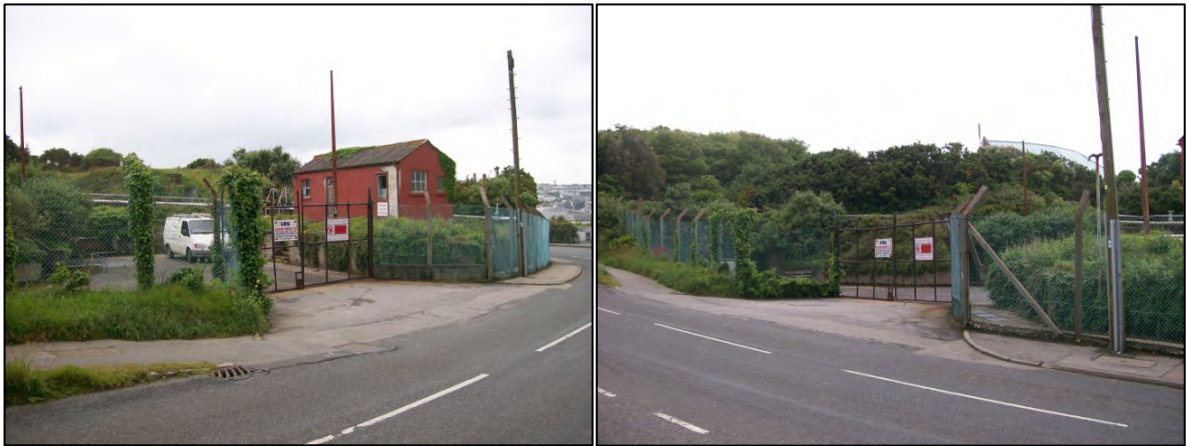
Figure 10: Current entrance to fuel depot/eastern field (viewed from north-east).
