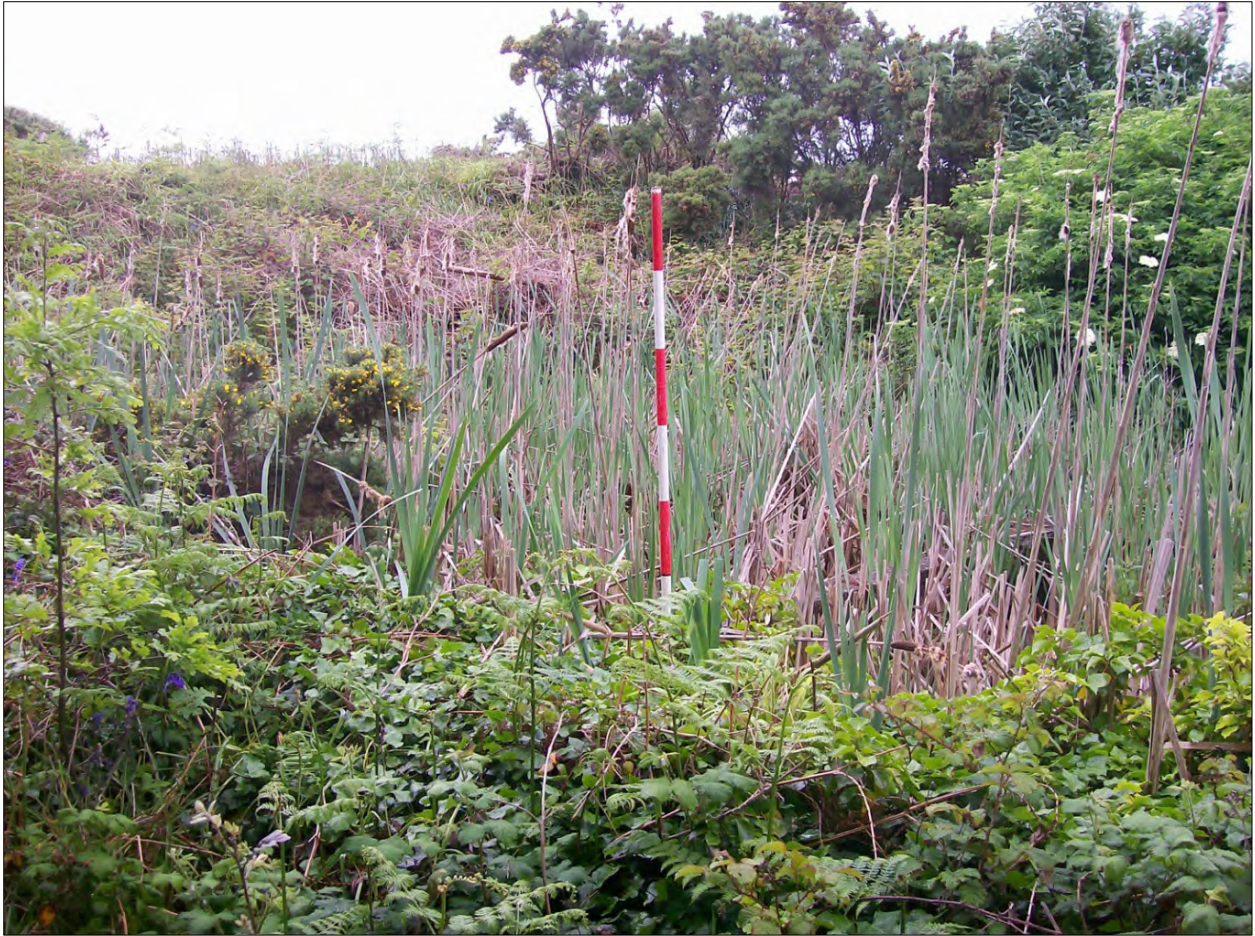
'Grid-shaped' tanks at the eastern end of the fuel depot; viewed from the north-east (scale 2m).
