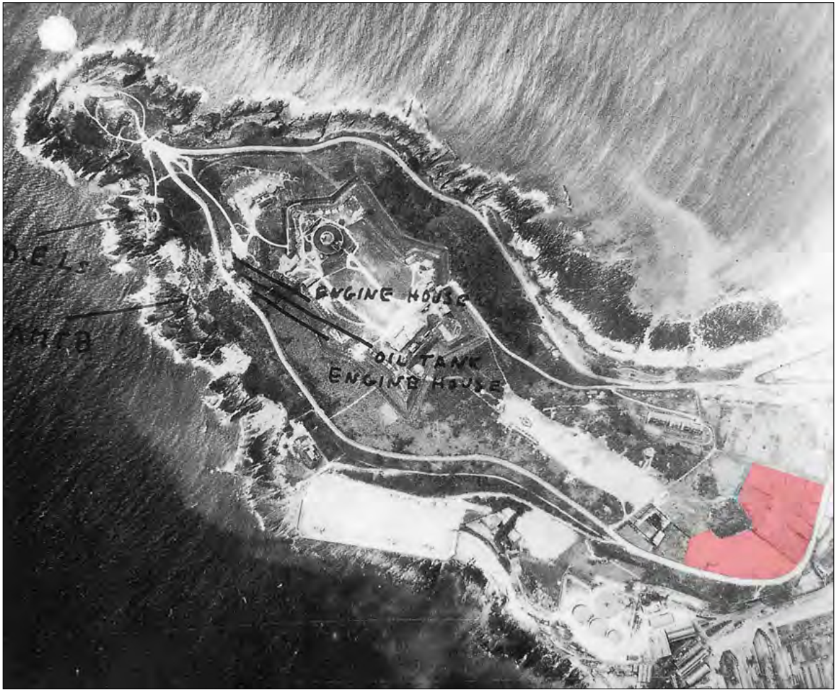
Figure 9: camouflage determination reconnaissance photo from April 1941. The site is indicated.
