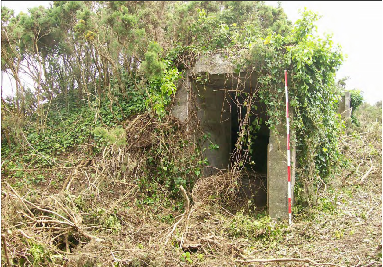
Entrances to the southern tanks; viewed from the west (scale 2m).
