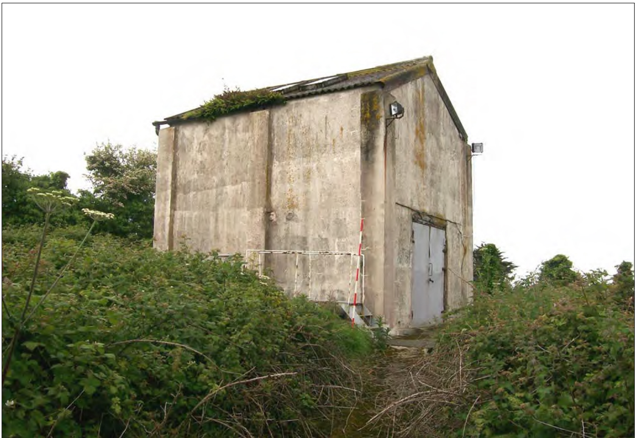
The pump house; viewed from the north.
