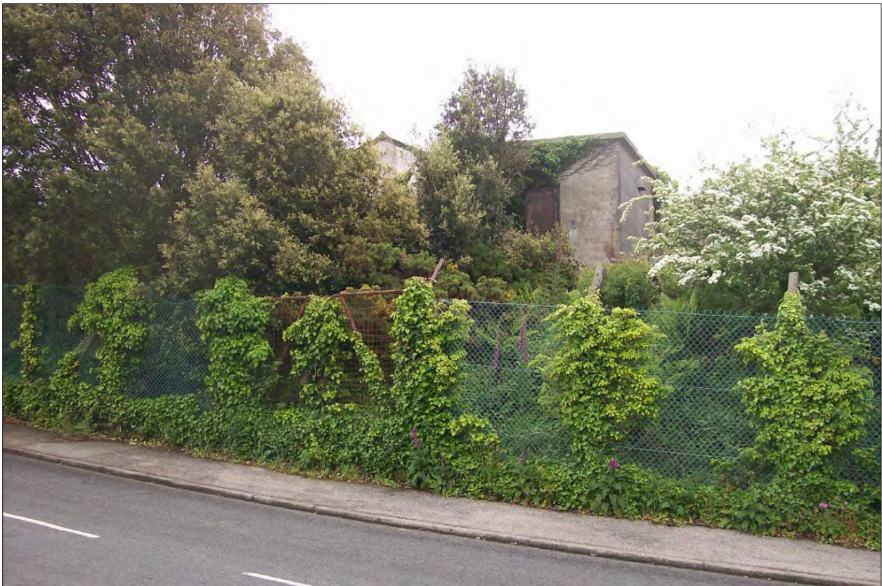
Ancillary building and alternative entrance to fuel depot from Castle Drive, at the western end of the depot; viewed from the north-west.
