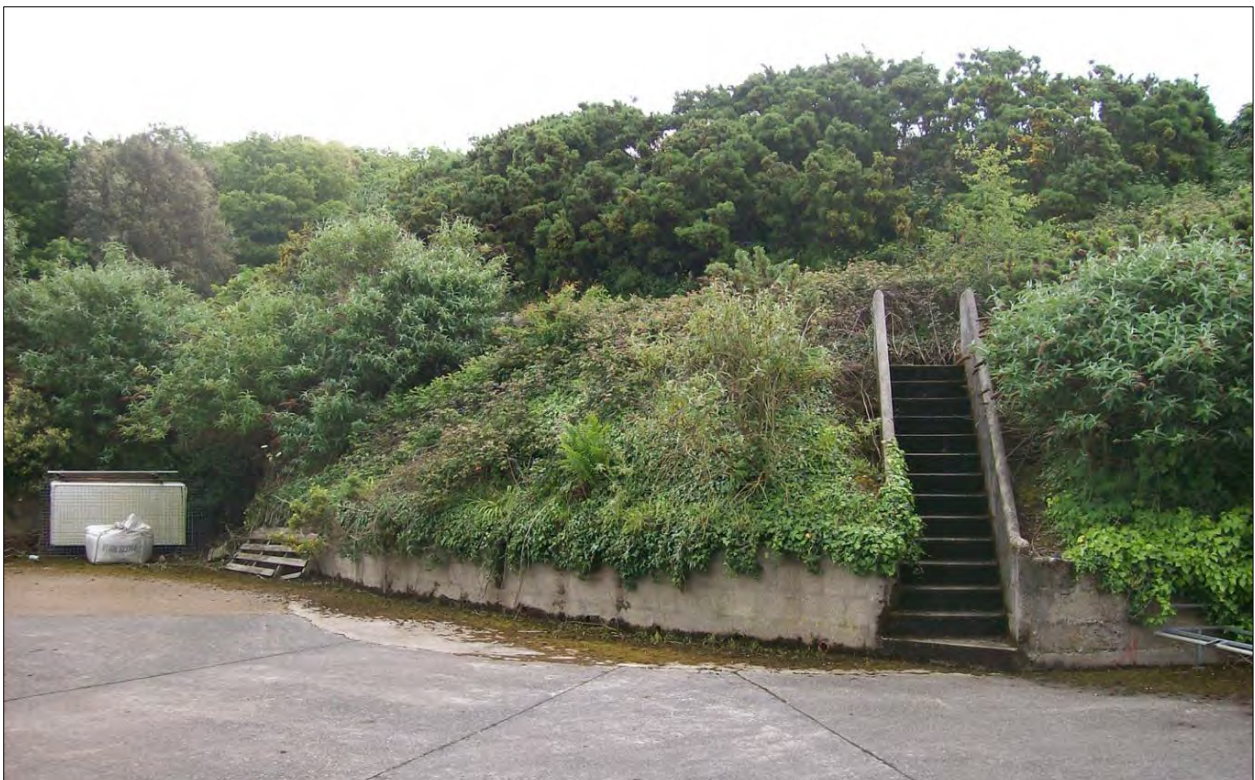
East side of car park; viewed from the west.
