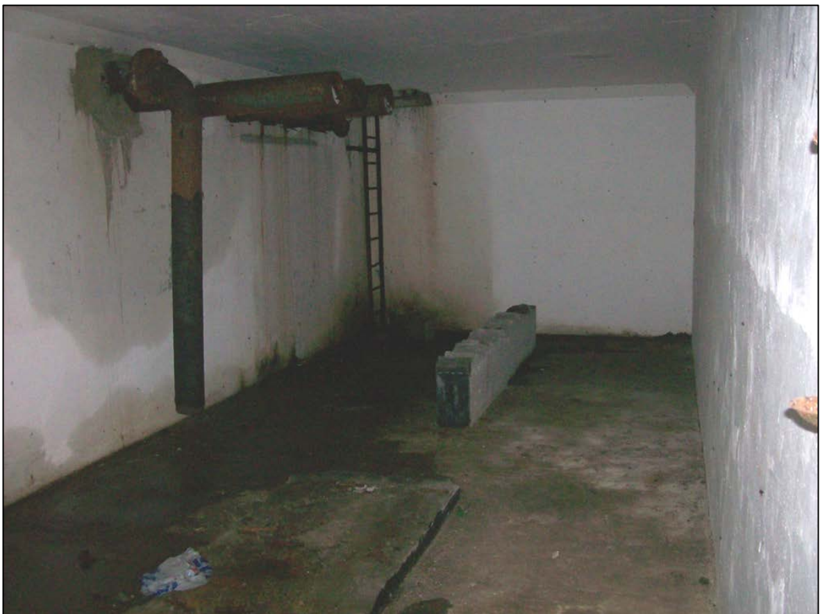
Figure 26: Inside the air-raid shelter; viewed from the south-west.
