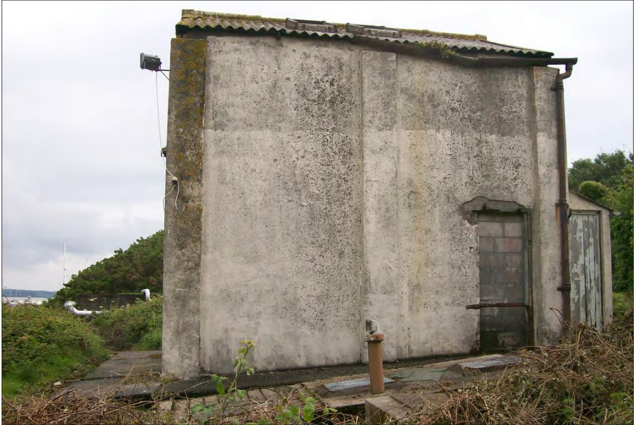
Pump house (viewed from south-west).
