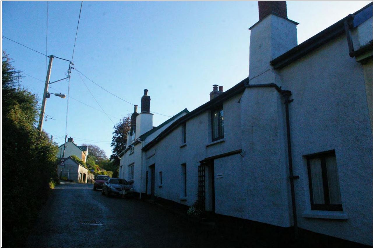
View of medieval or late medieval cob cottages, with later lateral stacks alongside the road, within the main street of Goodleigh, of a typical local North Devon vernacular, a character of the conservation area; from the west-north-west.
