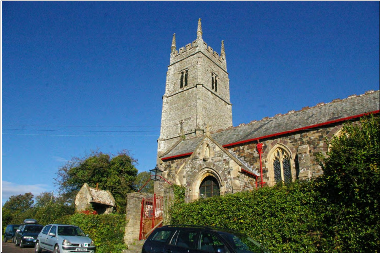
The church in Goodleigh, with tall stone tower, with wide views across and along the valley, from its position on the north slopes of the valley, facing south; from the south-east.
