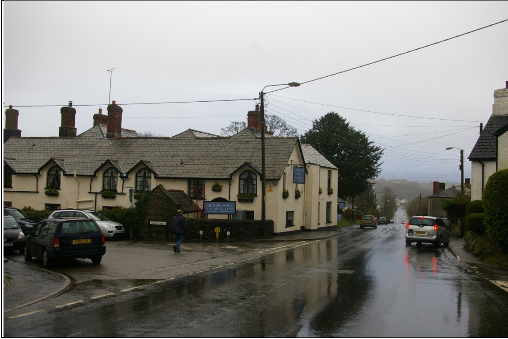
Lifton Hall Hotel, with views to the east, down Fore Street, showing some views across the houses to the south-east; from the south-west.
