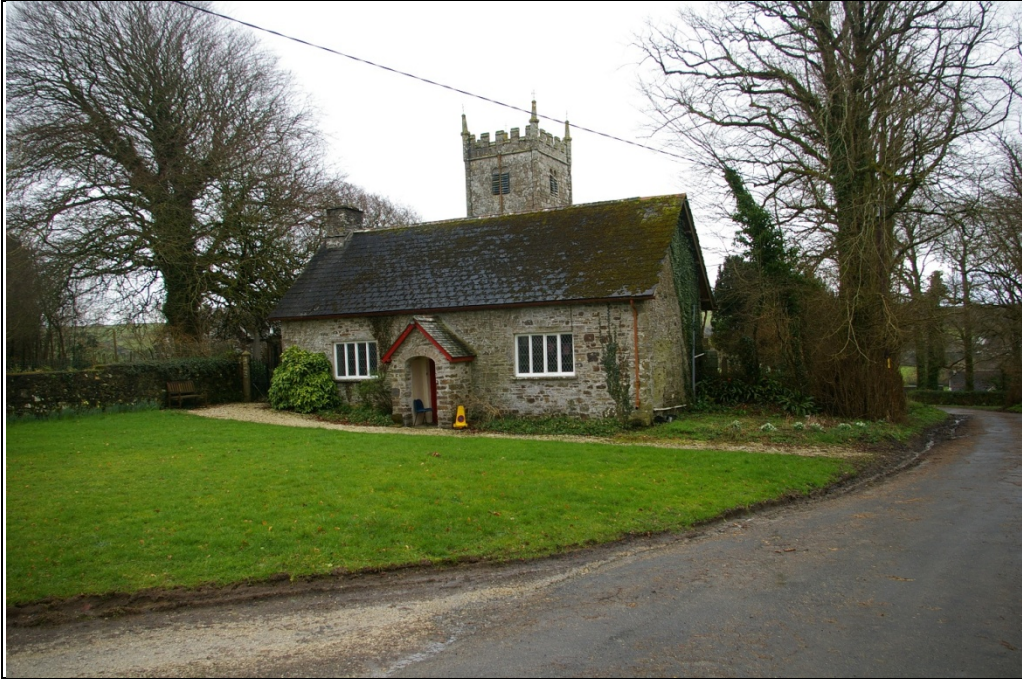
The Sunday school in Marystowe, locally blocked by trees and hedges; from the north-west
