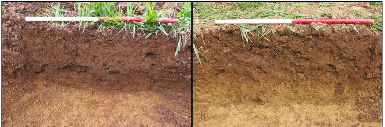
Figure 9: Section, north end Trench 1, viewed from east (1m scale).
