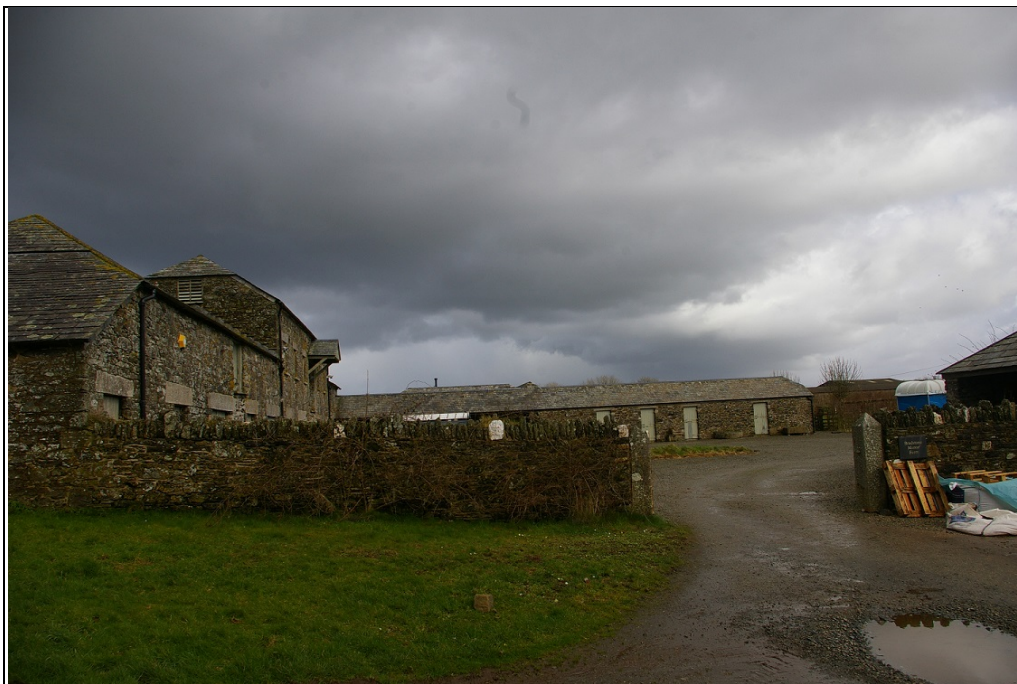
The large courtyard of barns and buildings which sit to the north and north-east of the main house, blocking views to the turbine; from the west.
