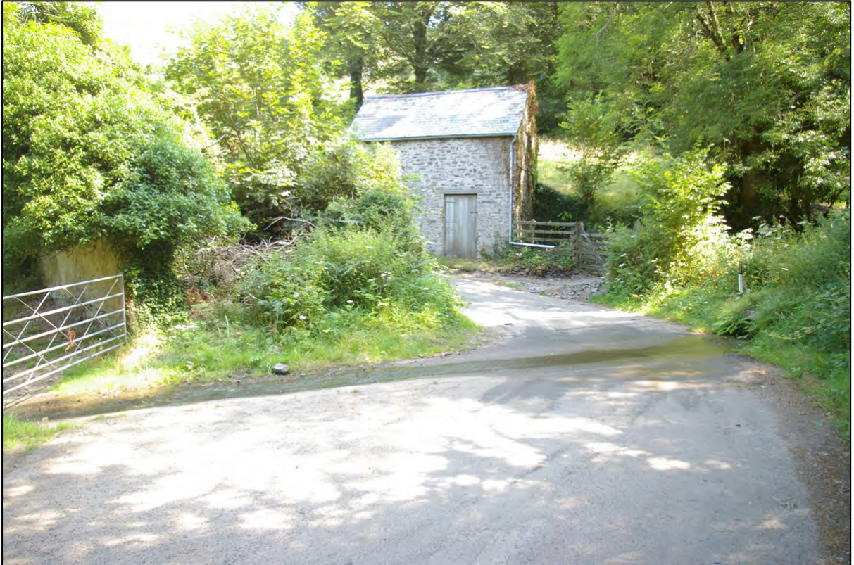
Figure 14: Building on north side of Cherryford across the ford; viewed from the south (no scale).
