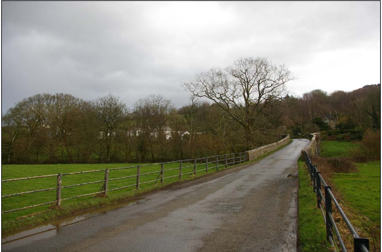
The horsebridge in Horsebridge, which crosses the Tamar, showing the local blocking factors; from the south-east.
