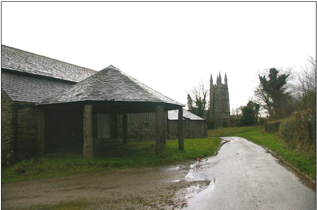
View between the extensive farm buildings at Bradstone, most of which are Listed, and the church; showing the visual links within the settlement; from the north-east.
