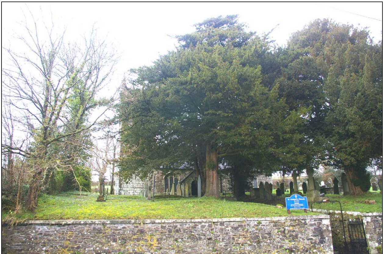
St Andrews in Coryton shielded by the large Yew trees in its churchyard and further blocked by woodland in the area; from the south.
