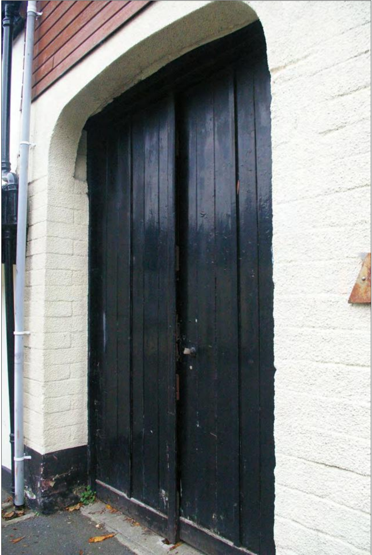
The double doors serving Area 5; from the south-west.
