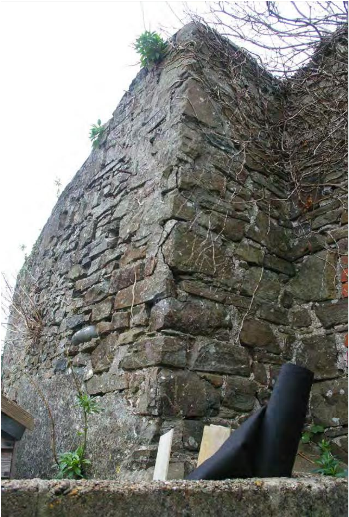
The wall between Areas 3 & 4, the stone quoin, from within Area 4; from the south, south-west.
