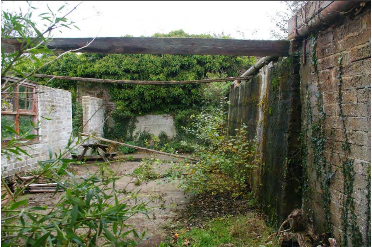
Area 3, from the doorway between Areas 3 & 4; from the west.
