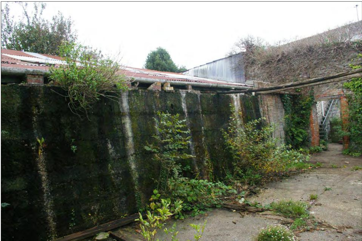
The concrete block party wall between Areas 3 & 6; from the north-east.
