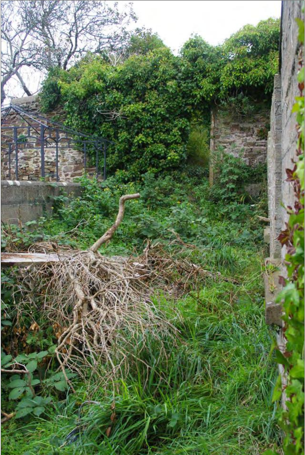
More detailed view of the rubble and overgrowth in Area 2; from the south, south-west.
