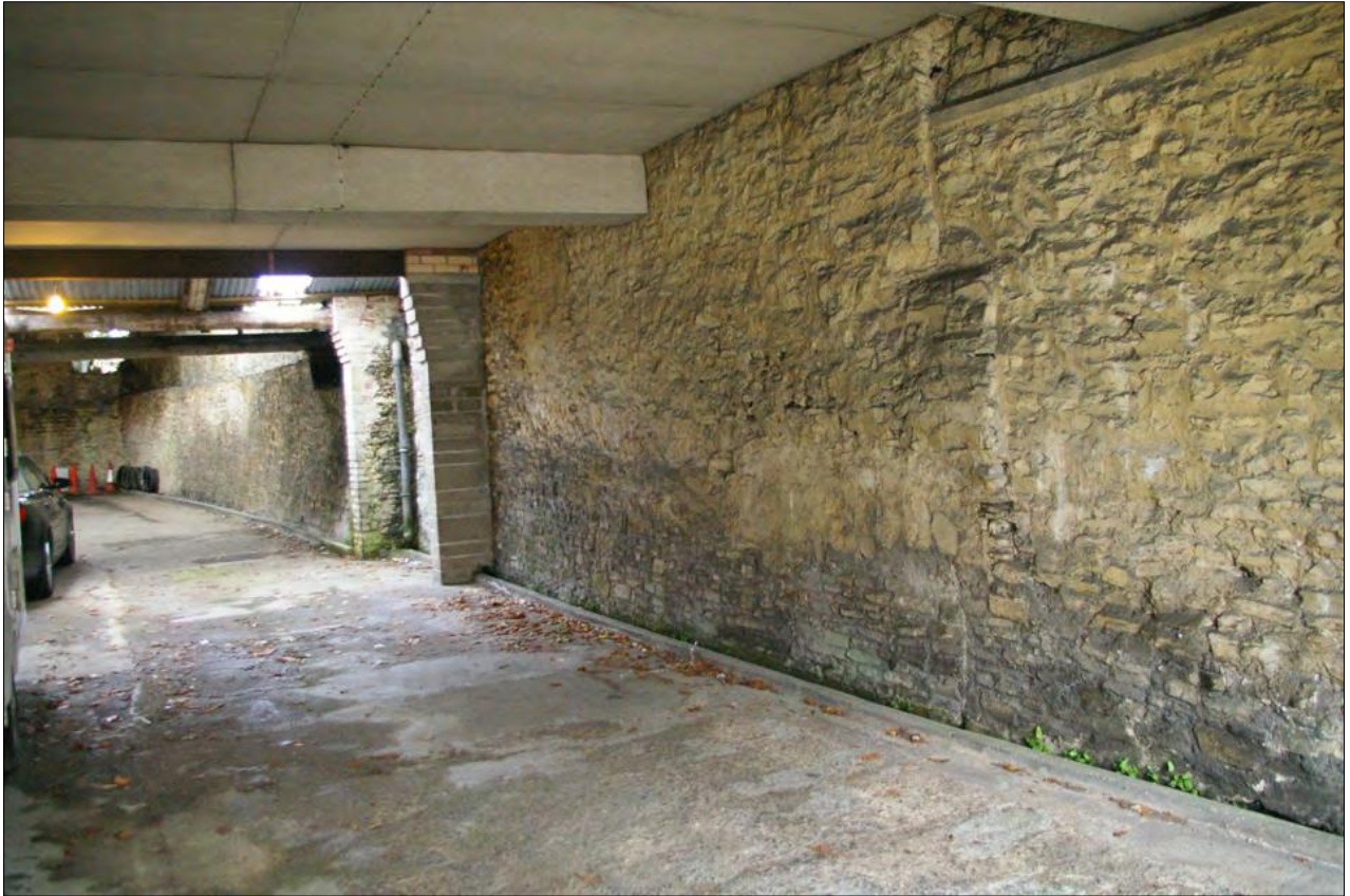
The south wall in Area 6; from the west, north-west.
