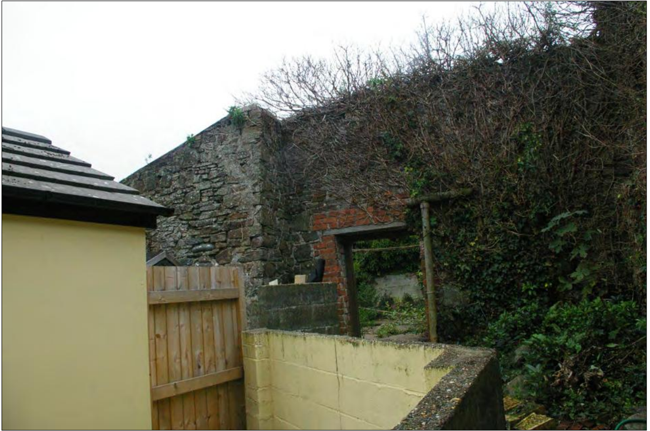
The stone wall between Areas 3 & 4, from Area 4; from the west-south-west.
