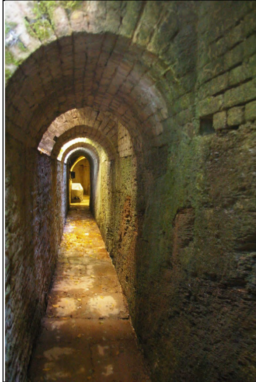
View down the drainage/air vent tunnel in Area 4; from the east.
