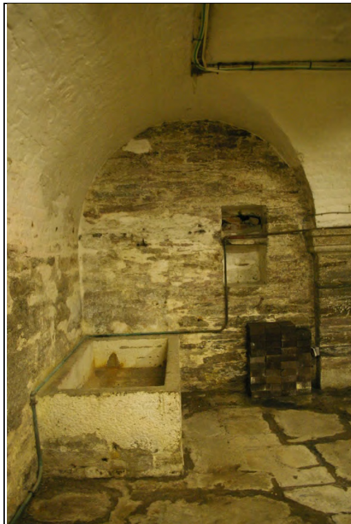
The east wall of the wine cellar, with keeping place and stone trough; from the west.
