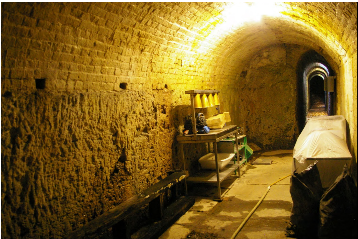
View of the south wall, cut out of the bedrock, within the vault in Area 4; from the north-east.
