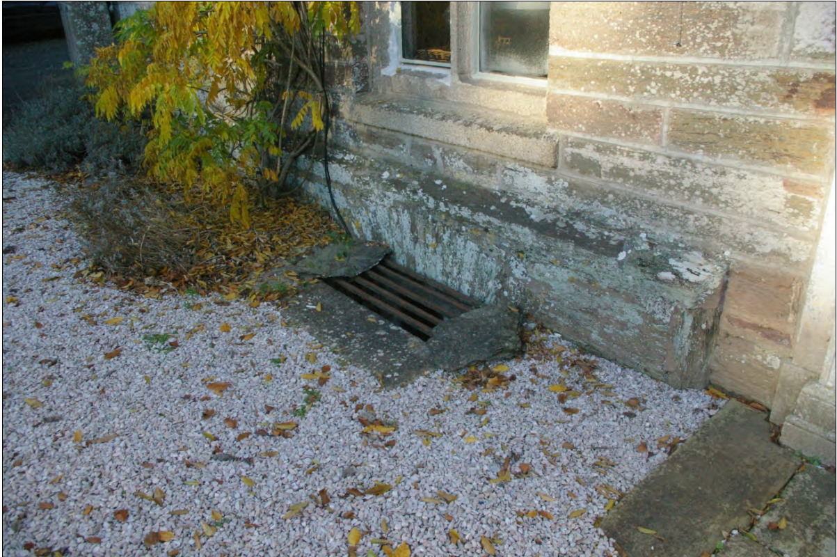
Detail of one of the light wells, with the segmental arch within the plinth; from the south-east.
