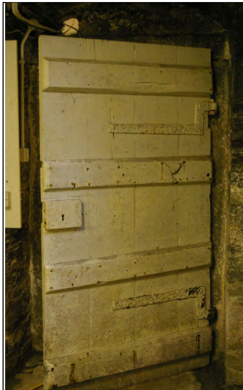
Detail of the secure 19 th century plank door; from the west.
