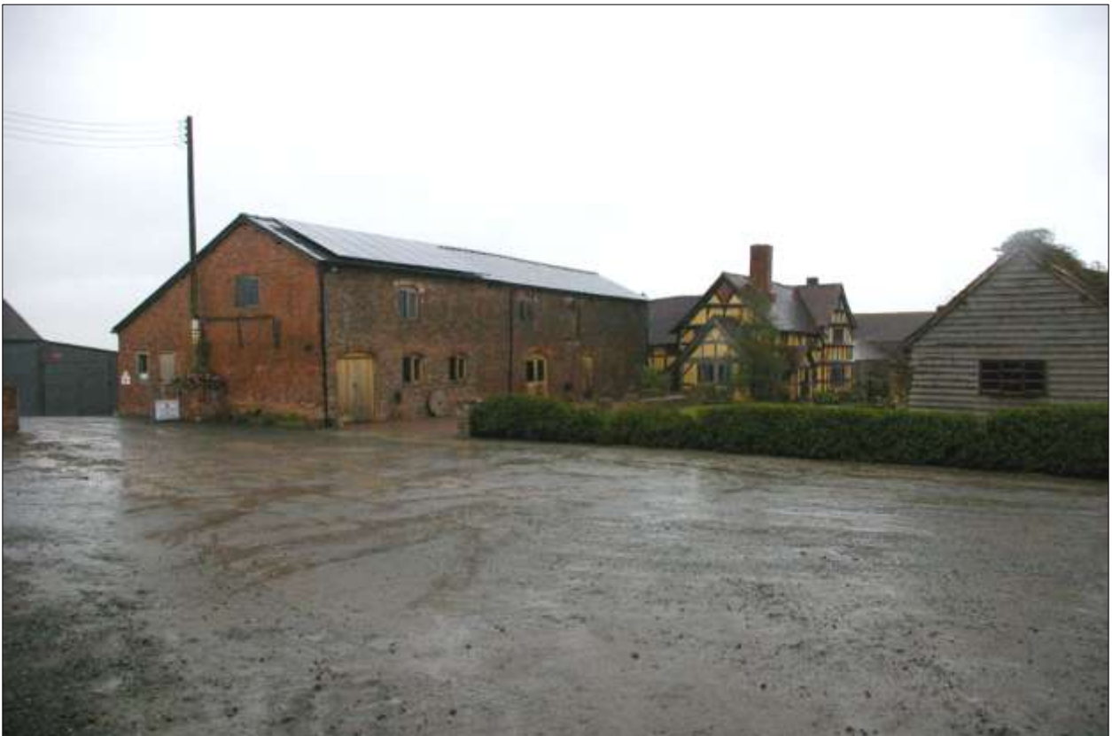
Newton Farm, viewed from the south-west, looking north-east.
