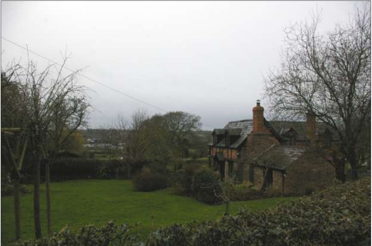
View over Providence Cottage, viewed from the east, looking west.
