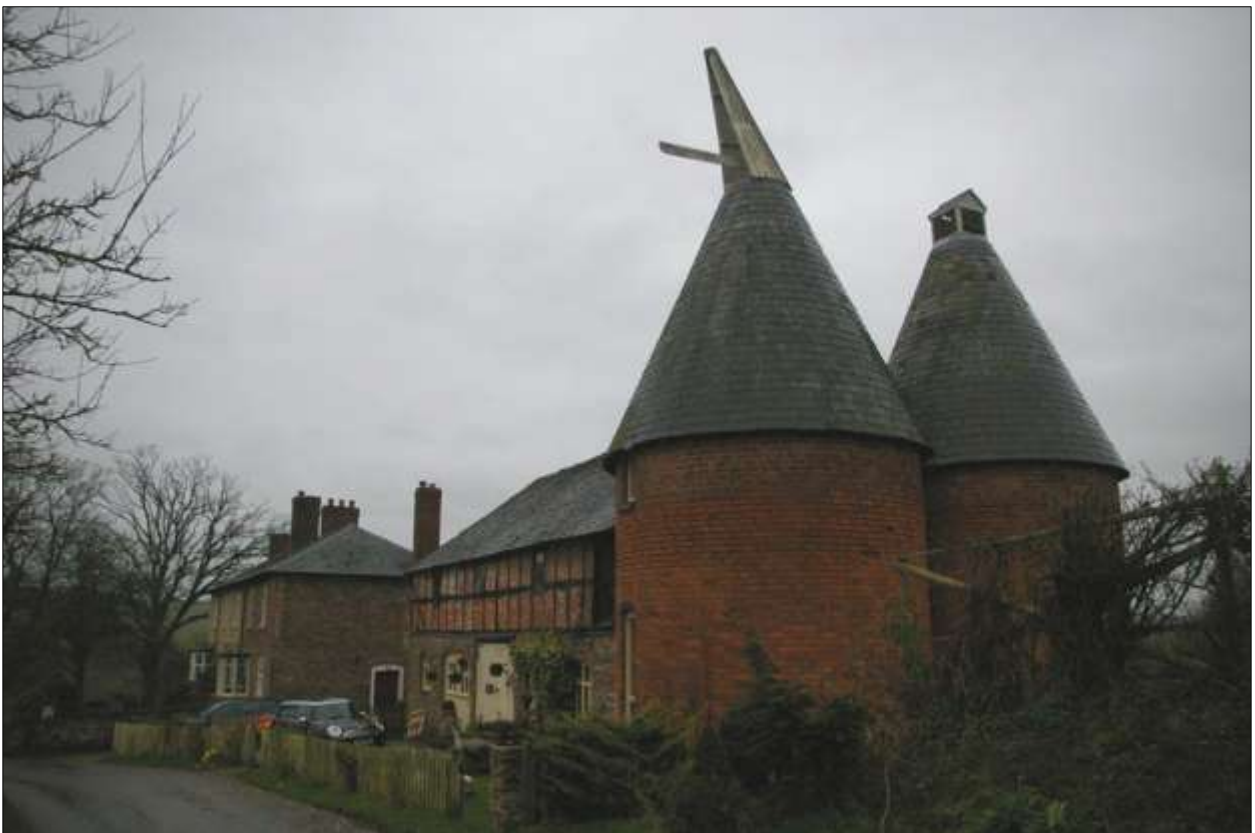
Avenbury Court, Barn and Hopkilns; viewed from the south-west, looking north-east.
