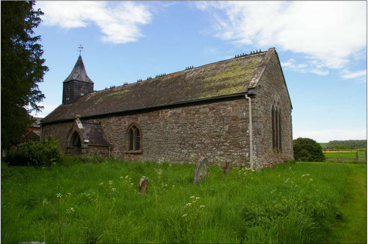
As above, from the south-east.
