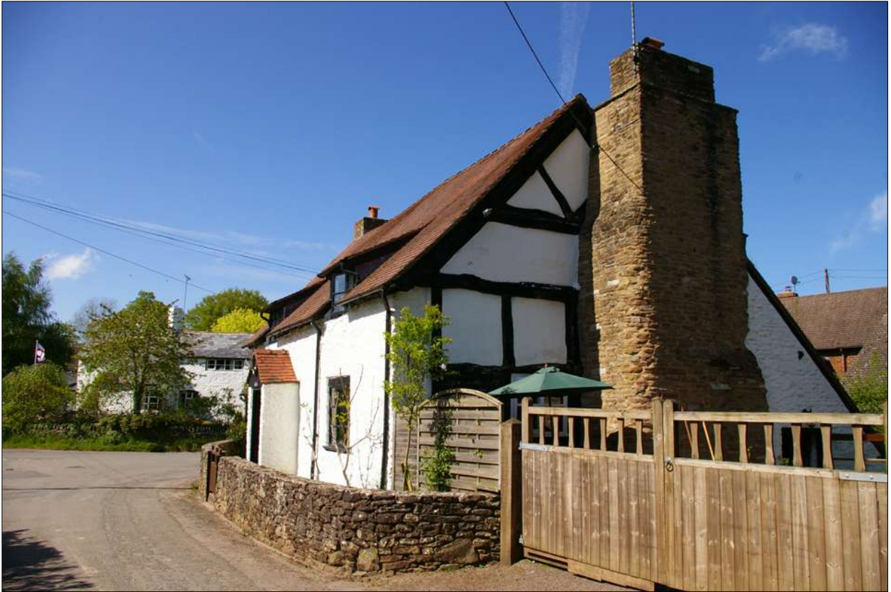
Tally Ho Cottage; viewed from the south-east, looking north-west.
