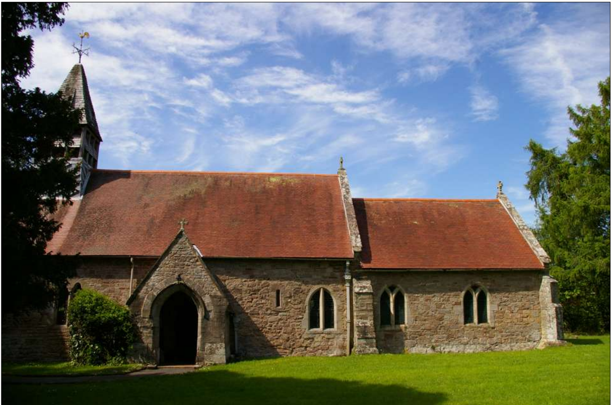
The church at Ullingswick; viewed from the south, looking north.
