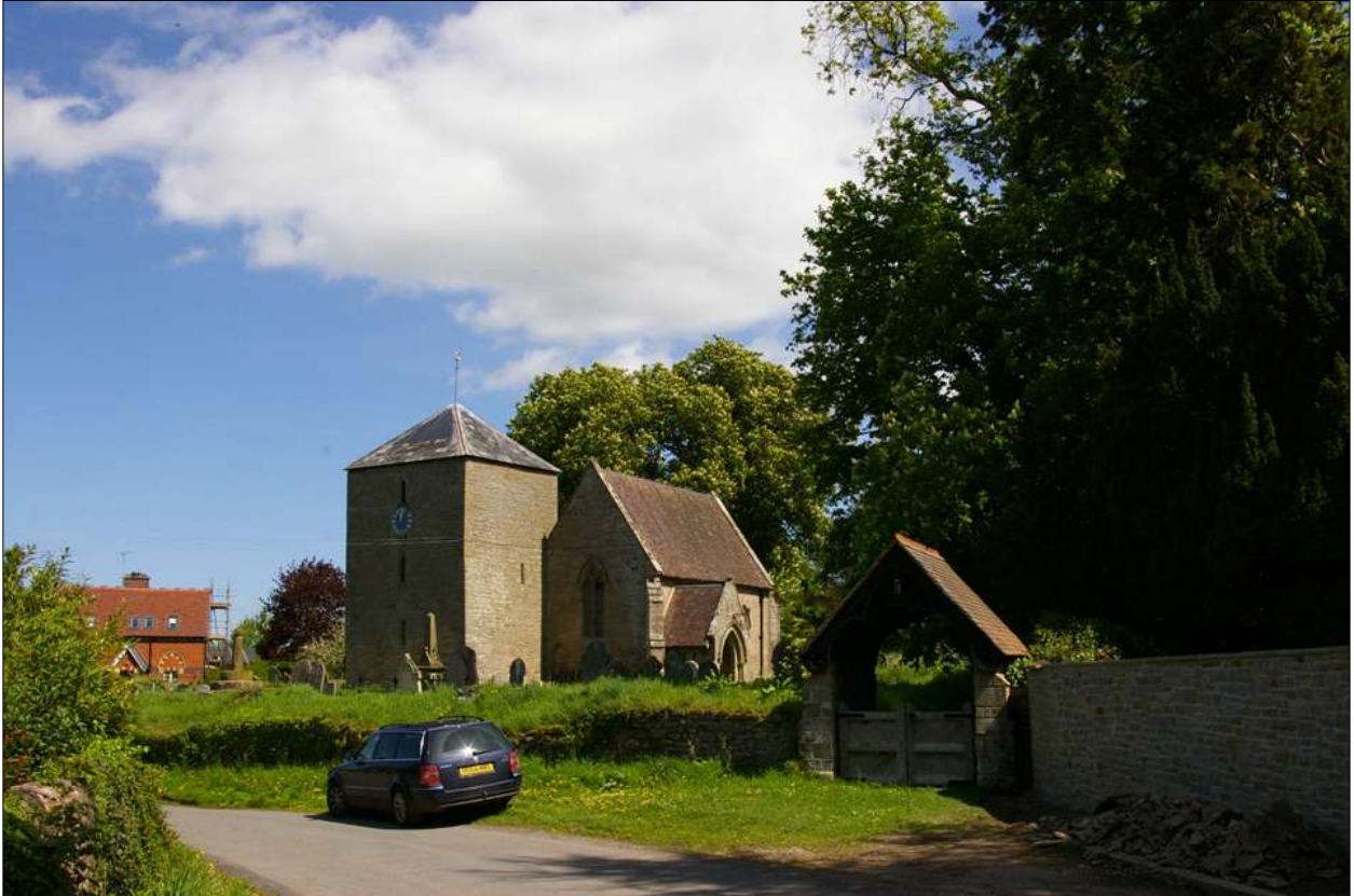
The church at Westhide; viewed from the south-west, looking north-east.
