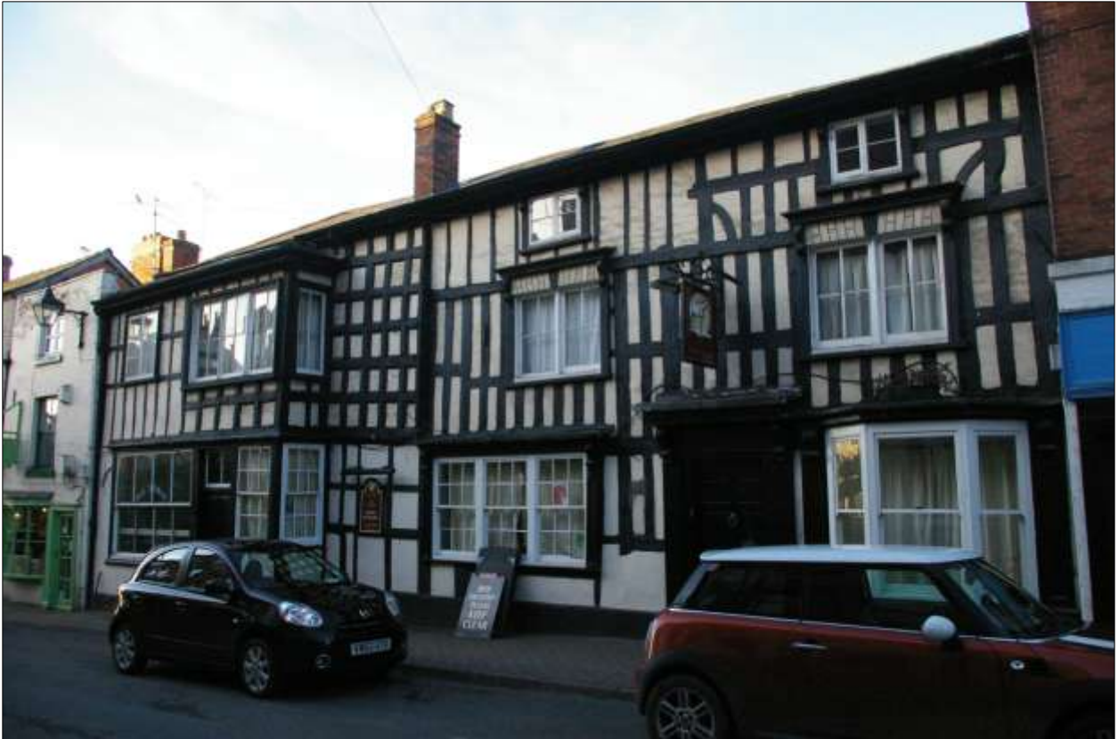
Bromyard, the exterior of the Bay Horse PH GII*, viewed from the north-east.
