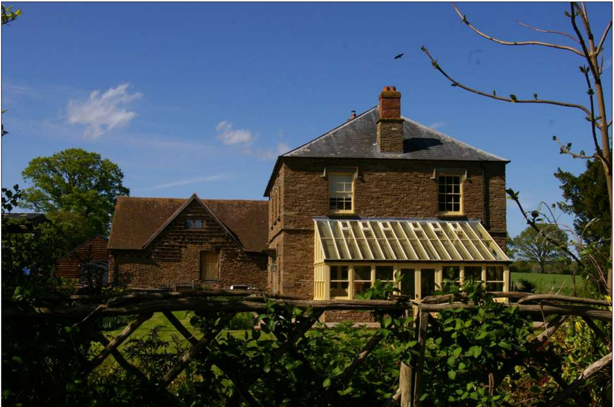
Pencombe Court, with the Listed barn to the left; viewed from the churchyard (south), looking north.
