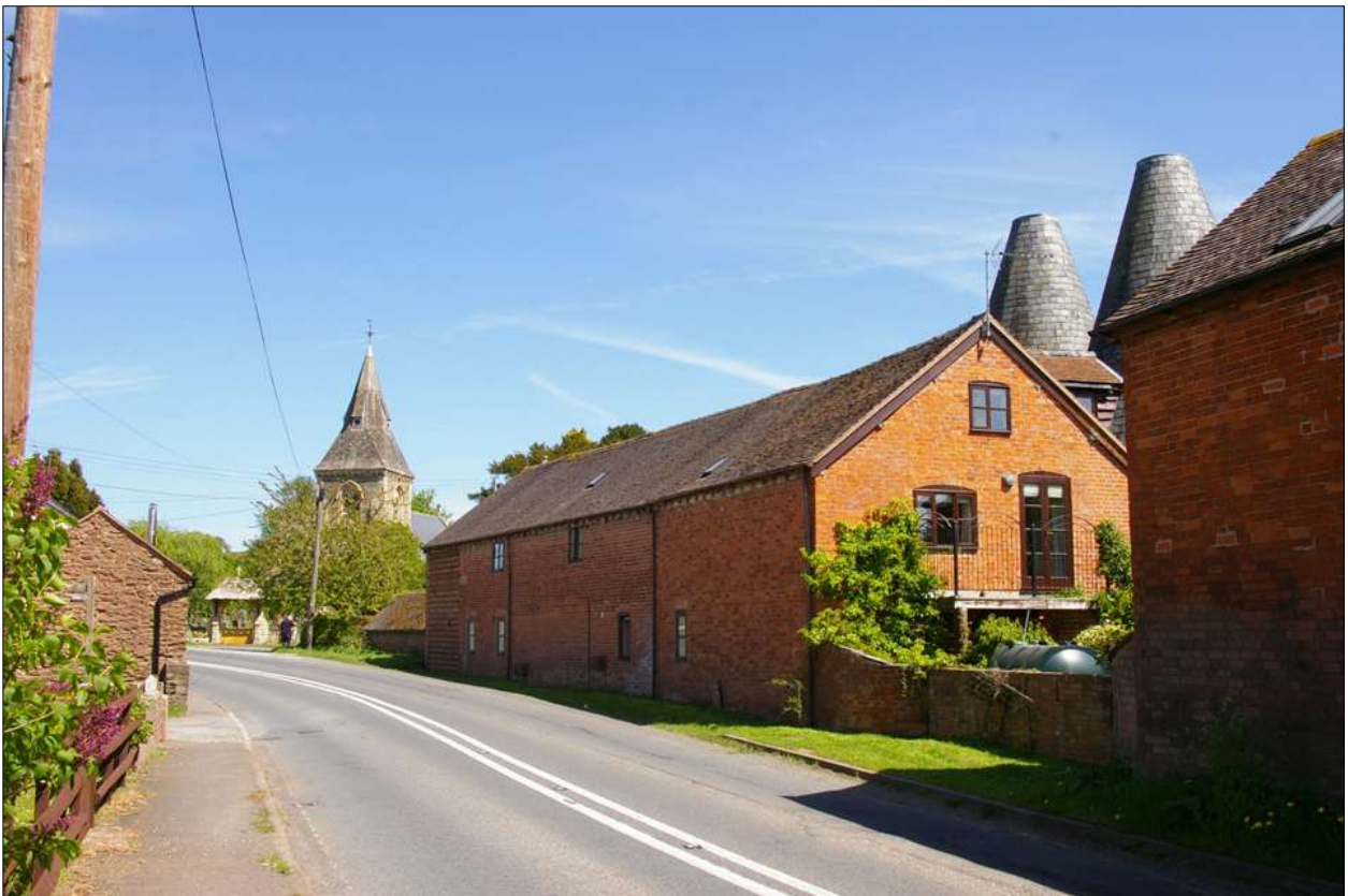
View past the converted farm buildings at Nether Court to the church at Stoke Lacy; viewed from the south-west, looking north-east.
