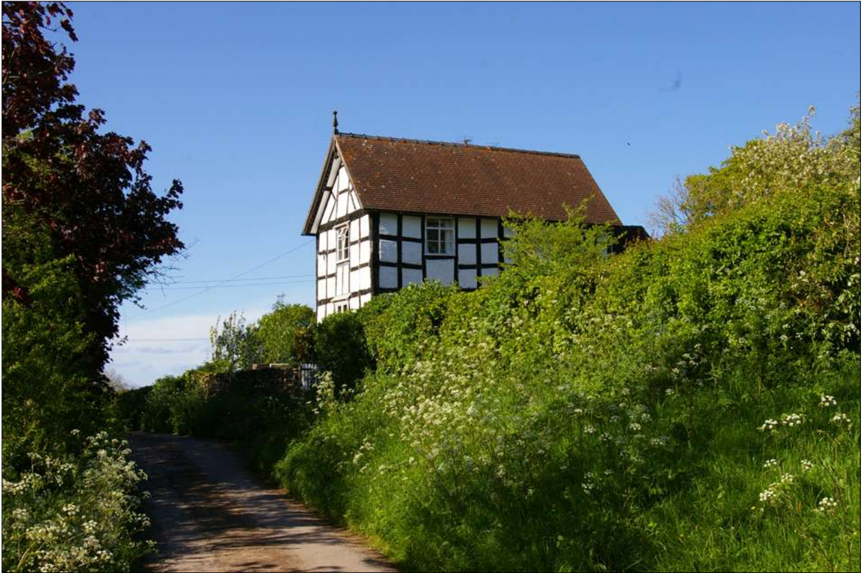
The Folly; viewed from the south, looking north.
