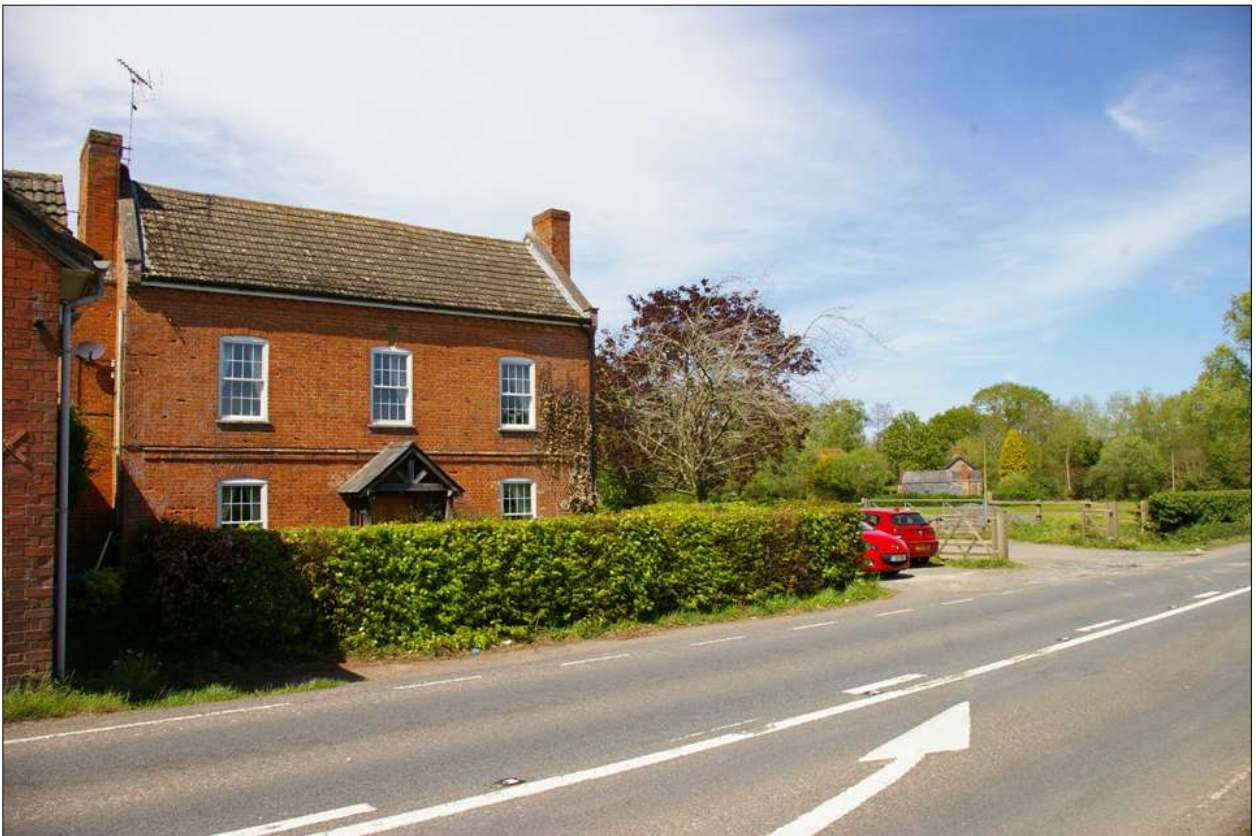
The Brick House, viewed from the roadside, with Stoke Lacy Mill in the background (right); viewed from the south, looking north.
