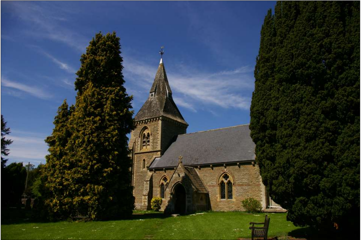
The church at Stoke Lacy; viewed from the south-east, looking north-west.
