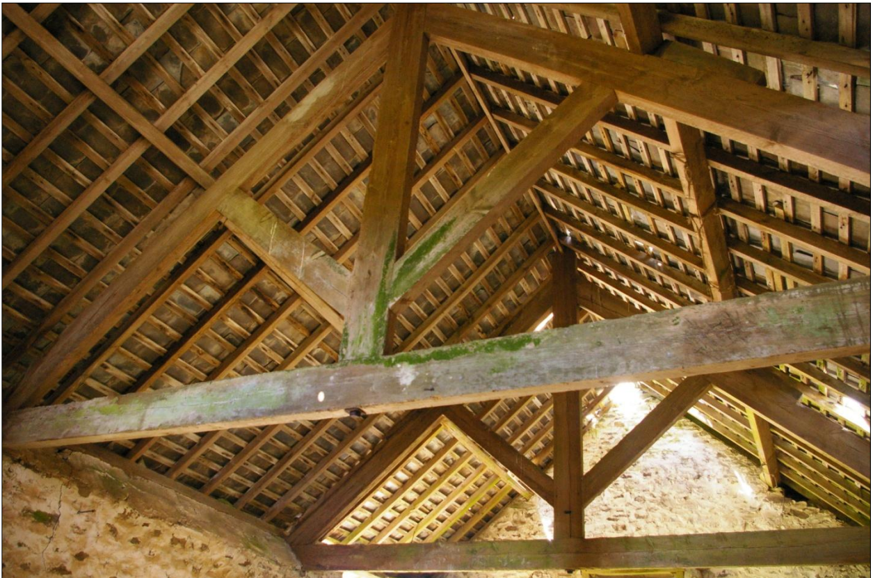
The king-post roof in Building 1; viewed from the north-east.
