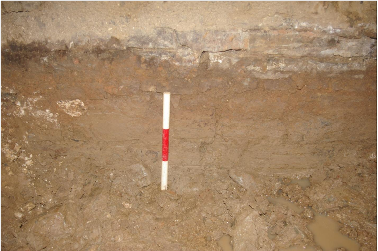
Detail of lower wall foundations of north wall, building B1, Area #5; viewed from the south (0.3m scale).
