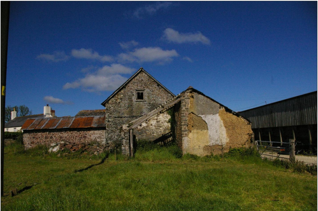
The east elevation of the barn complex; viewed from the east.
