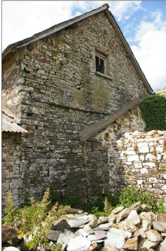
The east gable wall of Building 1; viewed from the south-east.
