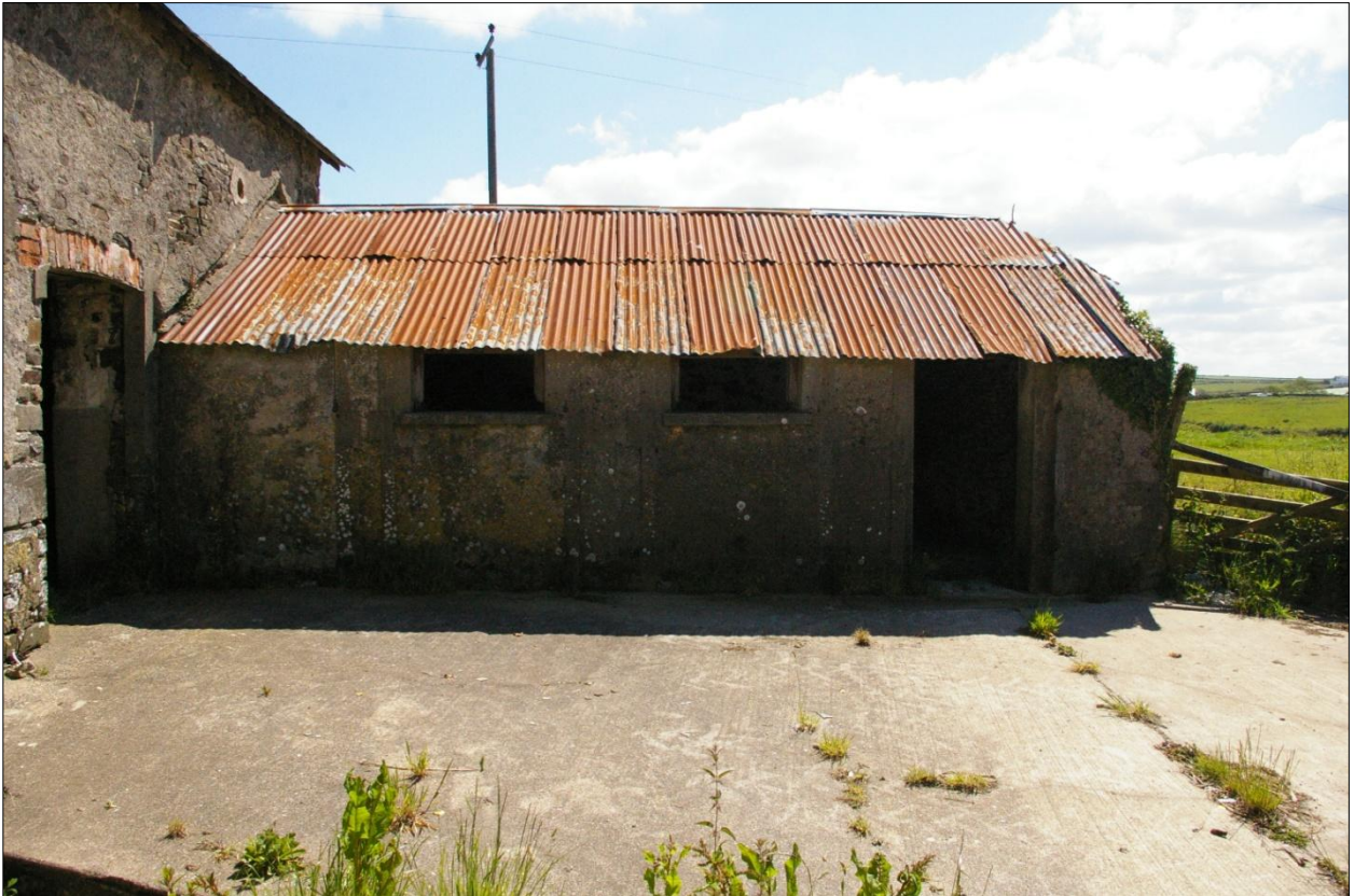
The west elevation of Building 4; viewed from the west.
