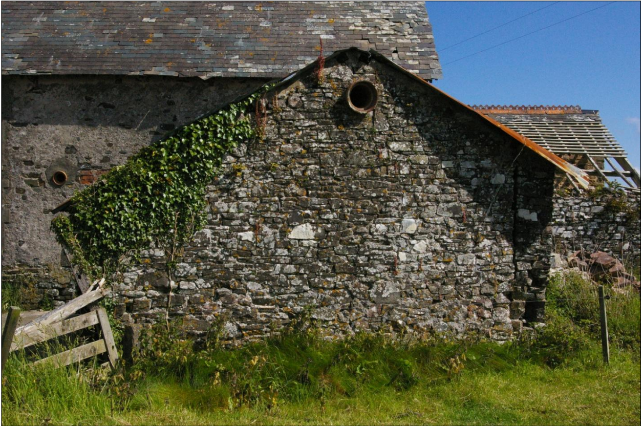
South elevation of Building 4; viewed from the south.
