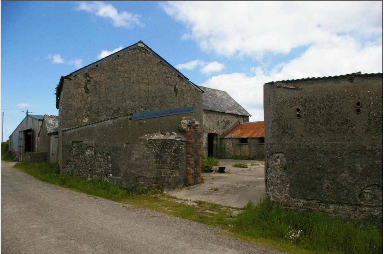
The yard and barn complex looking through the entrance gateway; viewed from the south-west.
