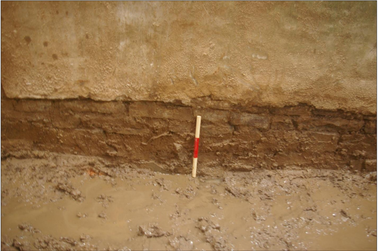
Detail of lower wall foundations of south wall building B1, Area #5; viewed from the north (0.3m scale).
