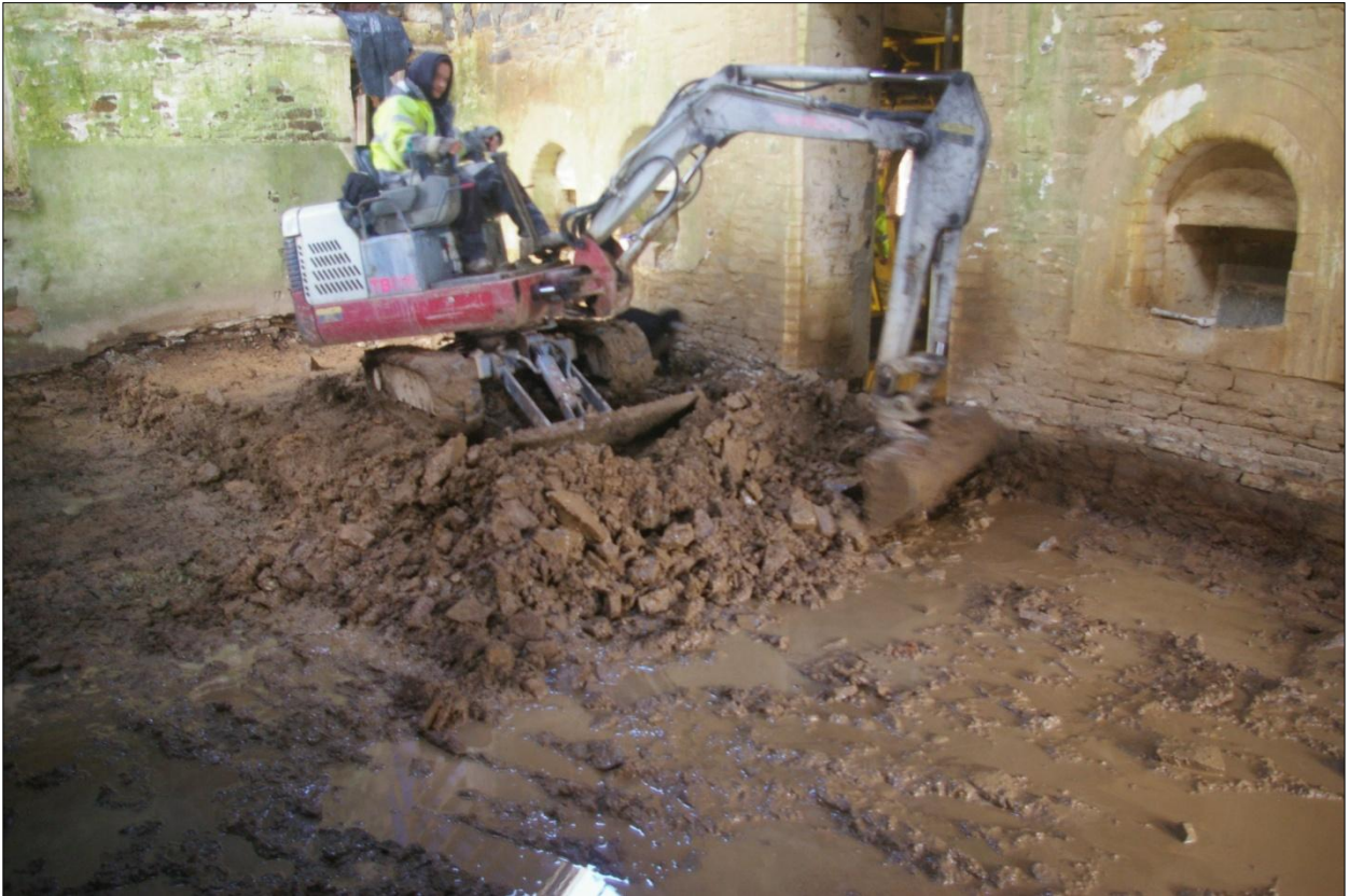
Working shot during ground-works, Area #5; viewed from the south-east (no scale).
