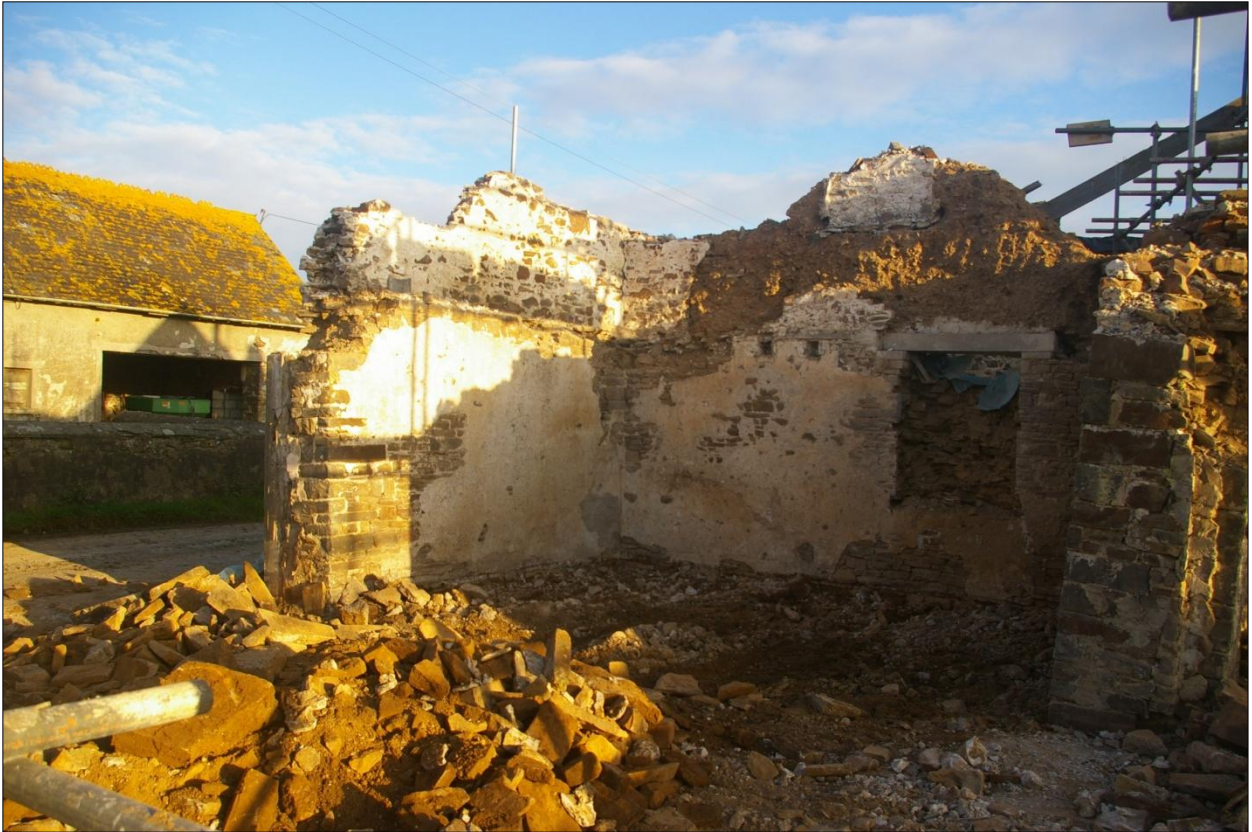
Pre-excitation view of Area #7; viewed from the south-east (no scale).
