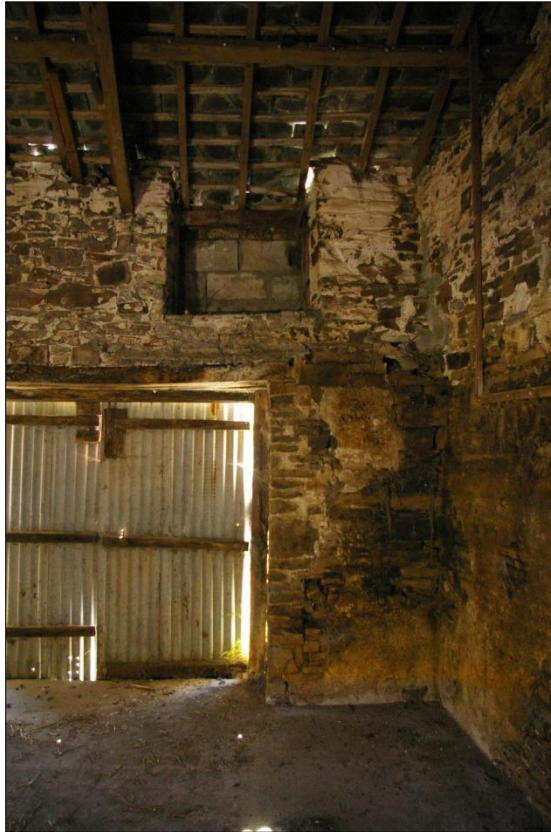
The east wall of Building 2, internal face, showing the southerly of the two windows at eaves height and the large forced ground floor double doorway; viewed from the west.
