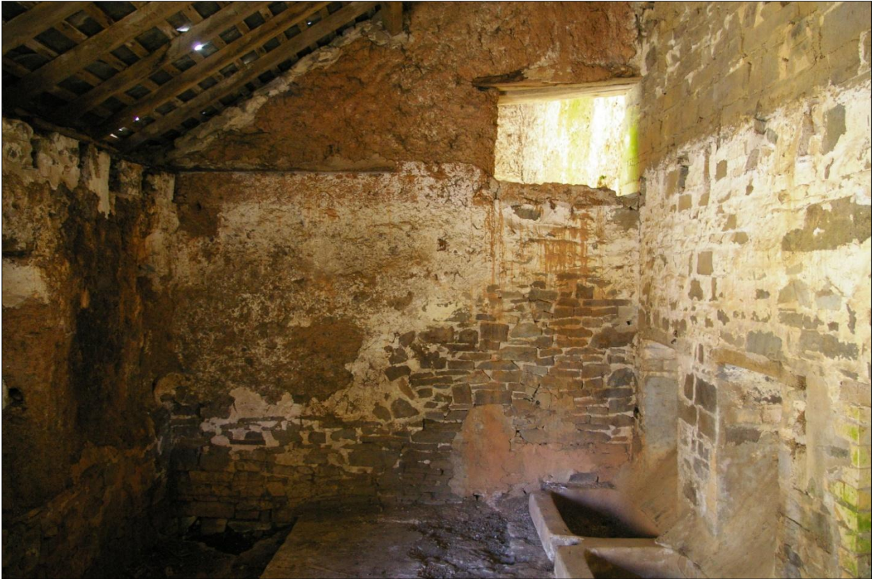
The east wall of Building 3, internal face; viewed from the west.
