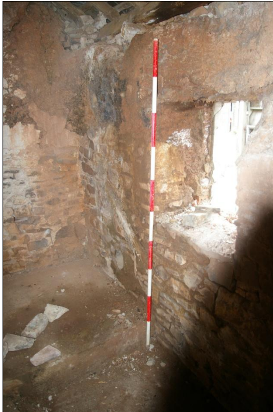
The north wall of Building 3, internal face, showing detail of the stone footings and cob upper; viewed from the south-east (2m scale).
