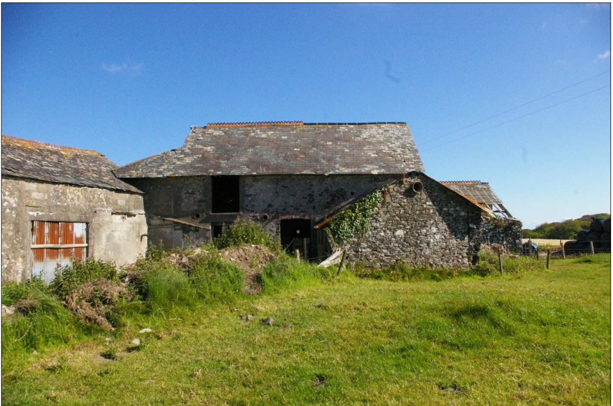
The barn complex; viewed from the south.
