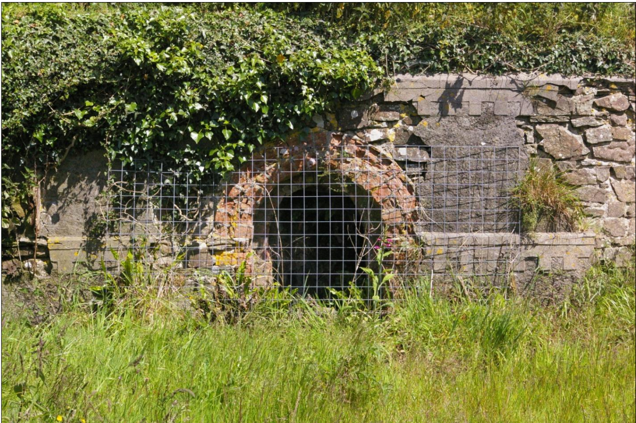
The well just to the north-west of the complex, with brick arch to stone-built well-house; viewed from the south.
