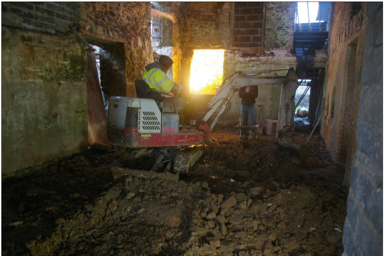
Working shot during ground-works, Area #5; viewed from the east (no scale).
