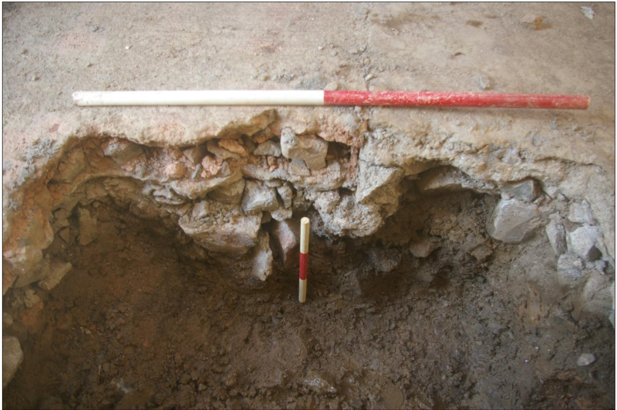
East facing section of under-pinning trench), Area #5; viewed from the east (0.3m and 1m scales).
