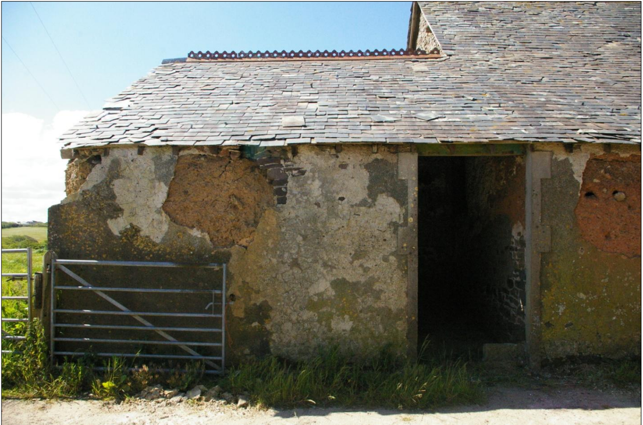
The north wall of Building 5; viewed from the north.
