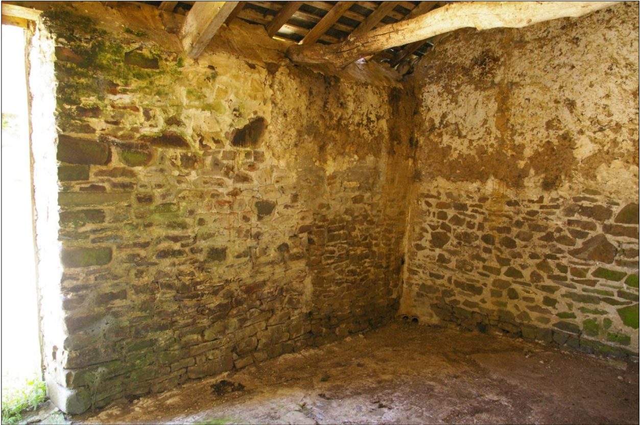
The north wall of Building 5, internal face; viewed from the south-west.
