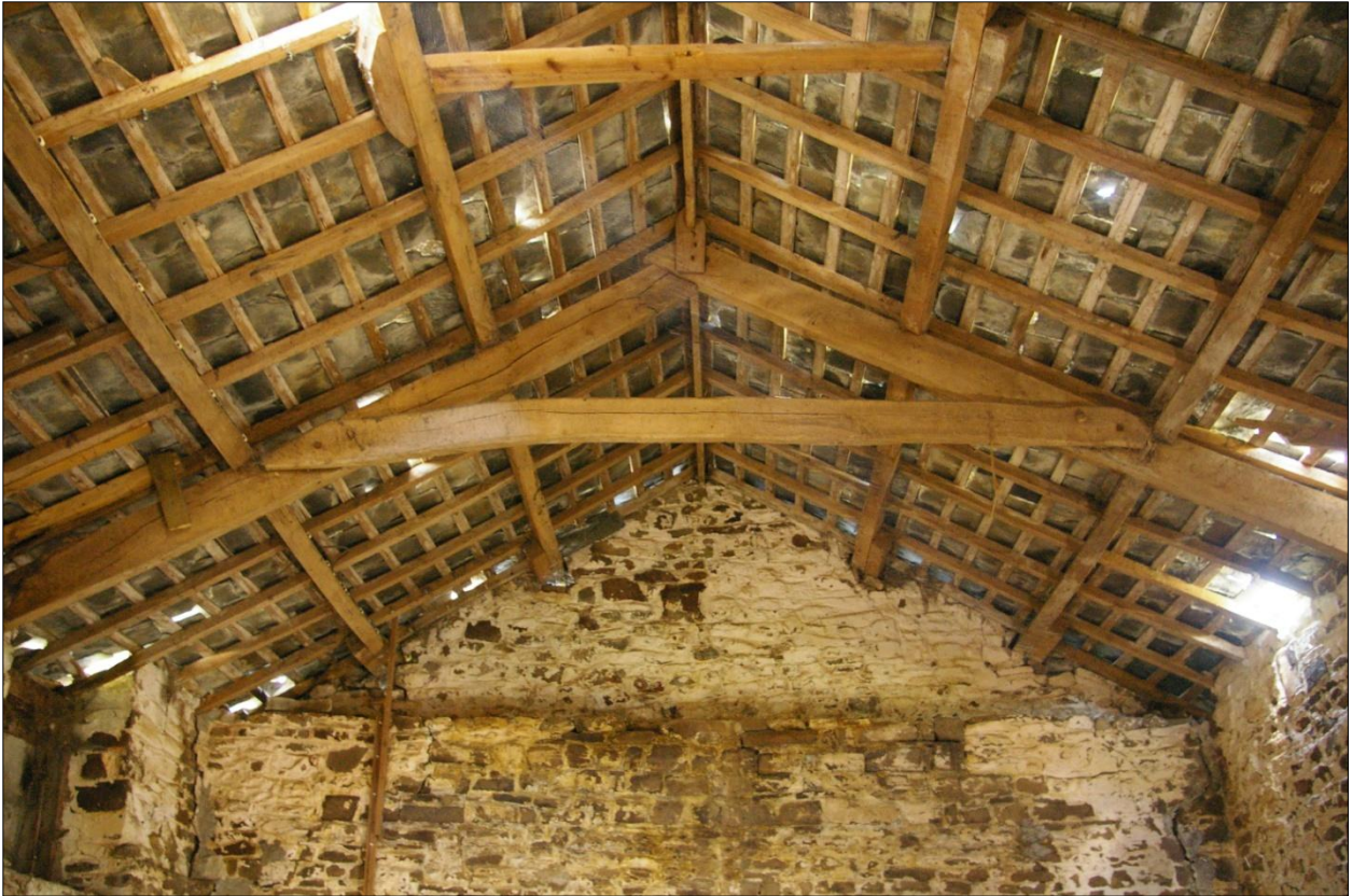
The pegged and bolted A-frames within Building 2; viewed from the north.
