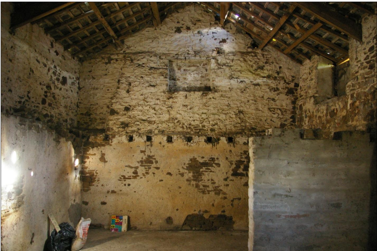
The north wall of Building 2, internal face, showing the remains of a stack and a window forced into that stack; viewed from the south.
