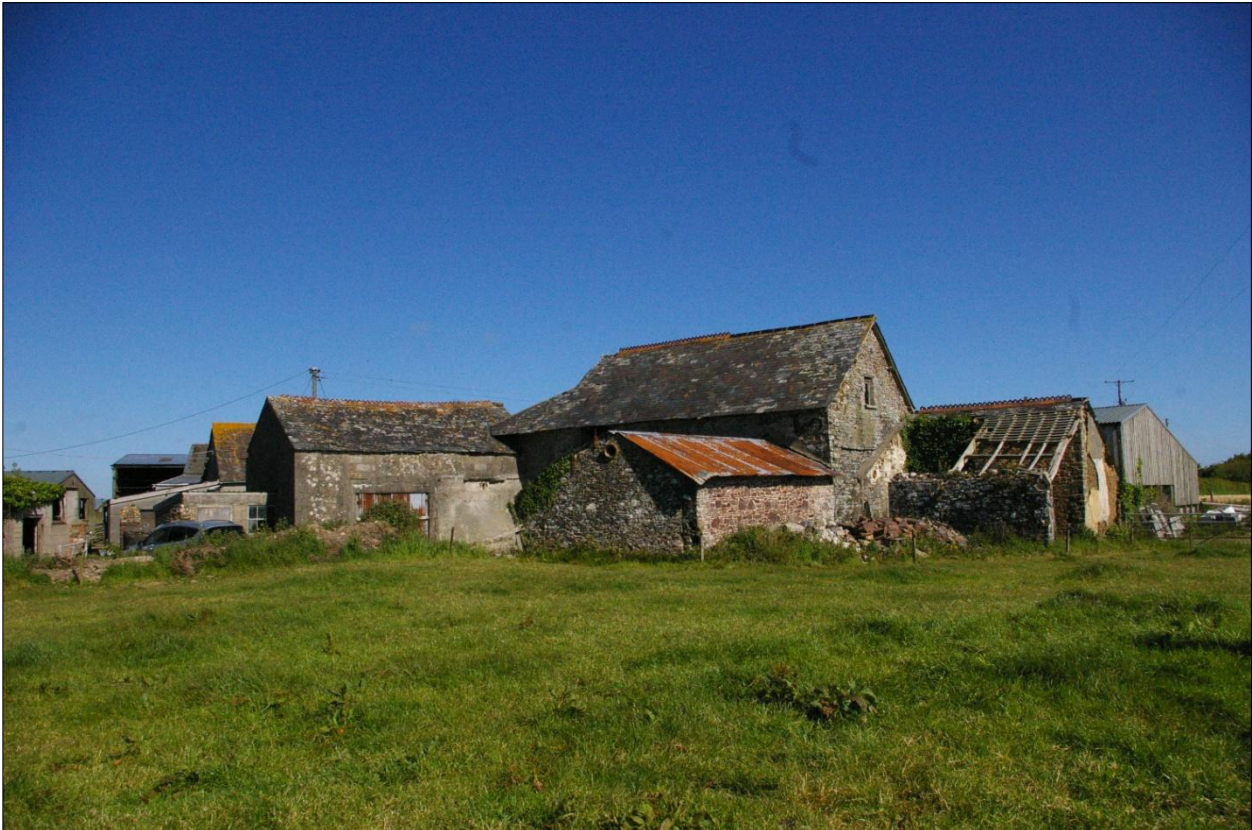
The barn complex; viewed from the south-east.
