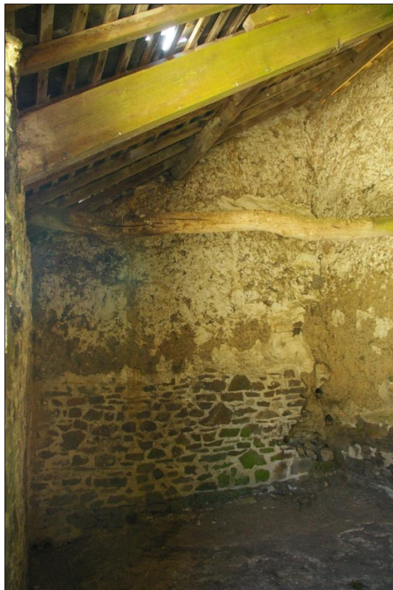
The east wall of Building 5, internal face; viewed from the north-west.
