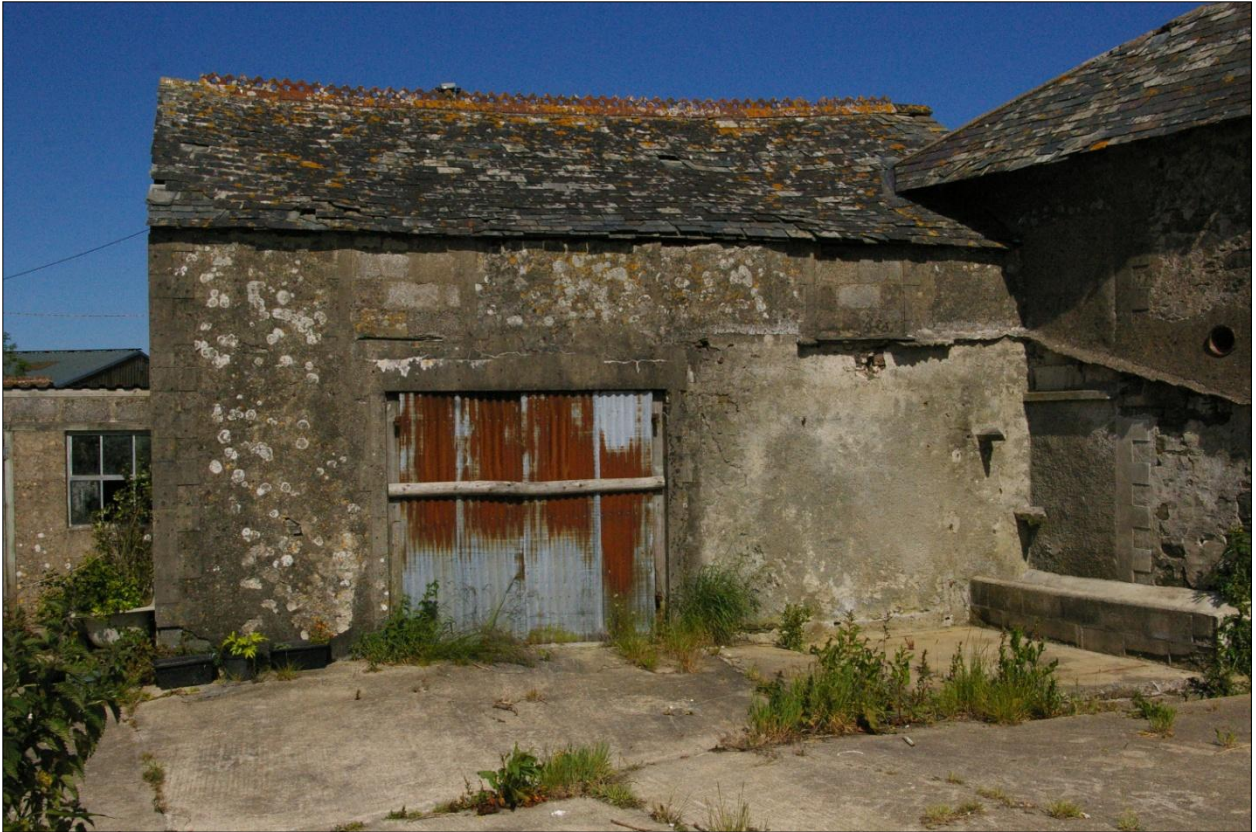
East elevation of Building 2; viewed from the east.
