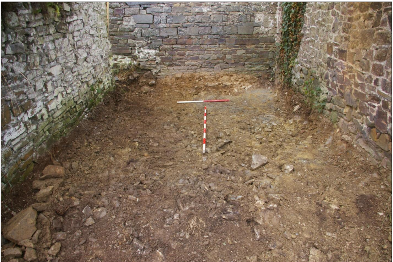
Post excavation plan view of Area #2; viewed from the east (1m and 2m scales).
