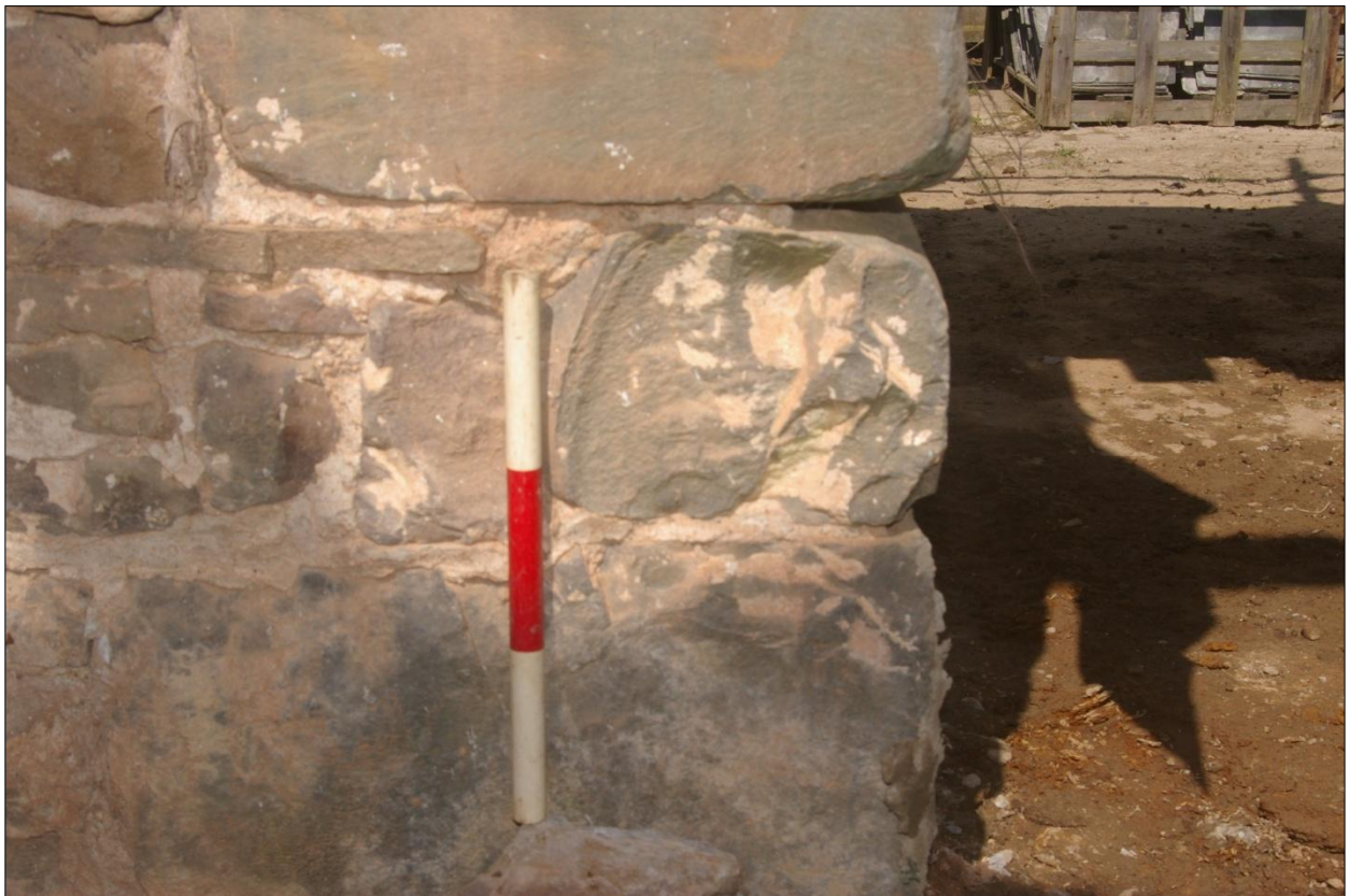
Detail of possible ecclesiastical stone set within north doorway of building 3; viewed from the south (0.3m scale).
