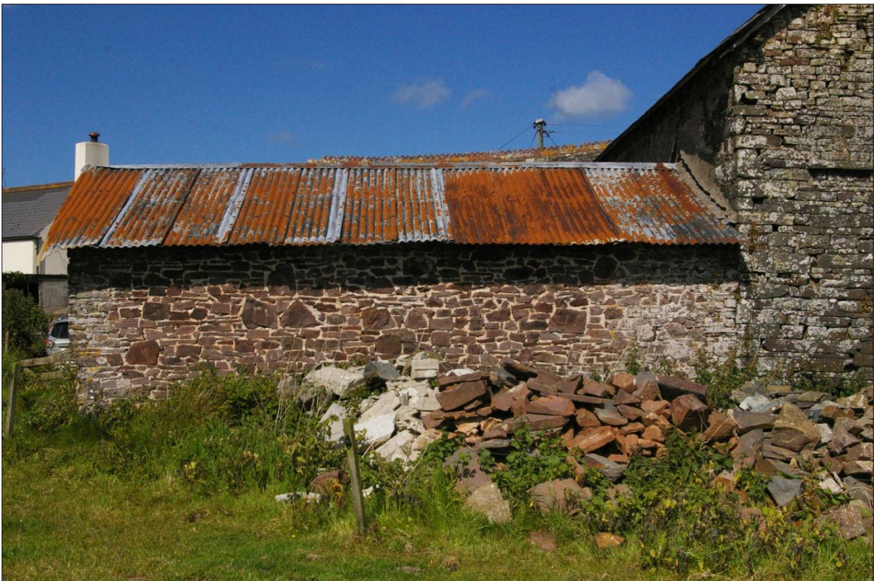
East elevation of Building 4; viewed from the east.
