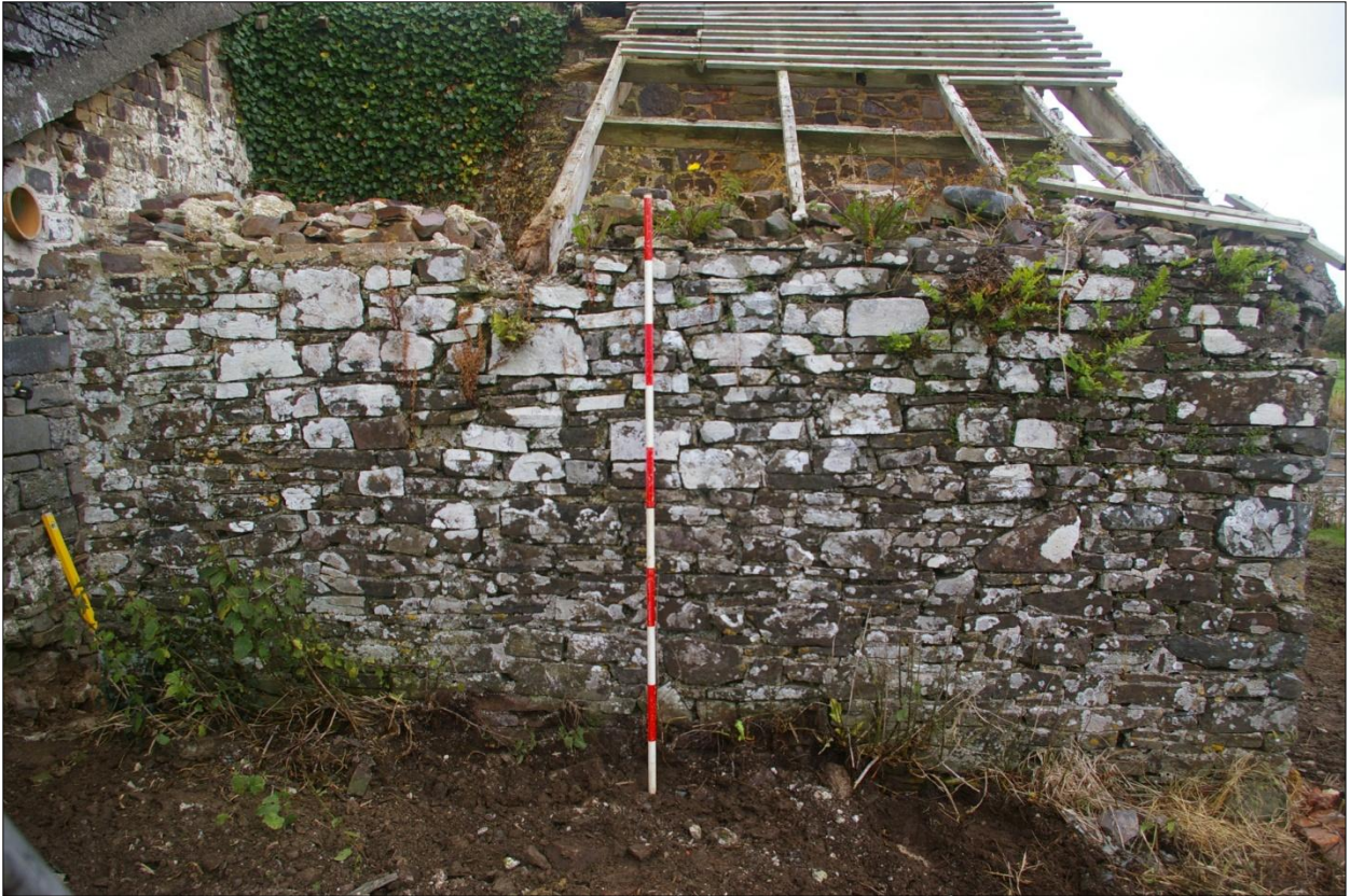
The south wall of Building 6; viewed from the west (2m scale).
