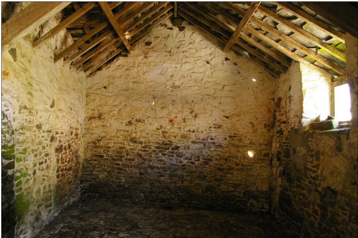
The west wall of Building 7, internal face; viewed from the east.
