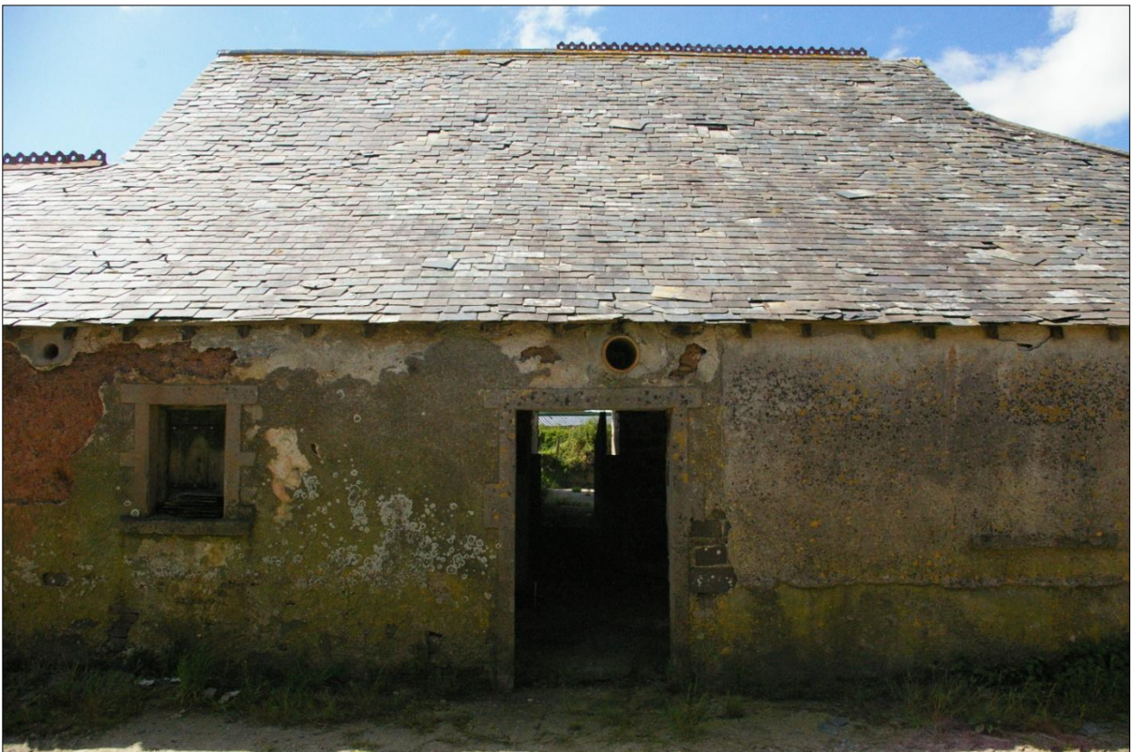
North elevation of Building 3; viewed from the north.
