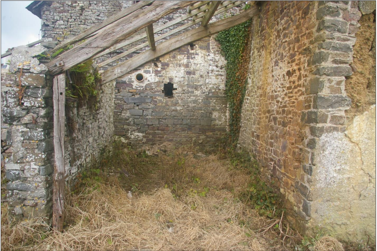
Pre excavation plan view of Area #2; viewed from the east.
