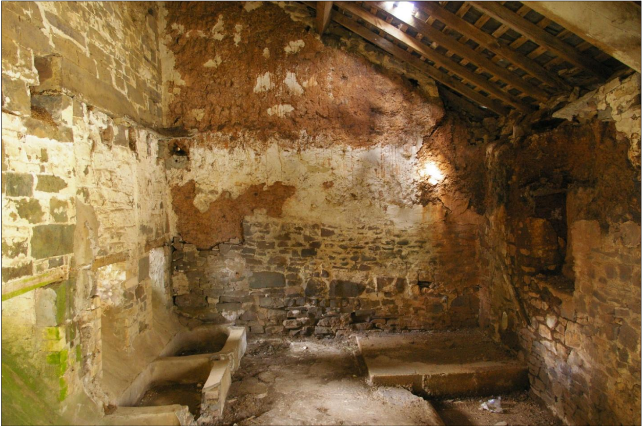
The west wall of Building 3, internal face; viewed from the east.
