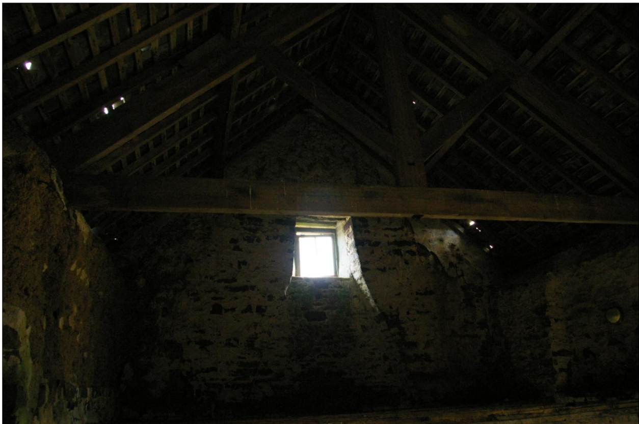
The east gable wall of building 1, internal face at first floor level, showing detail of the window forced into the chimney stack; viewed from the north-west.
