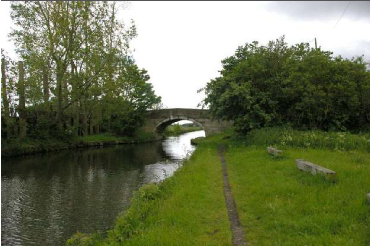
Harkers Bridge, over the Leeds and Liverpool Canal, near Halsall; from the north-north-west.
