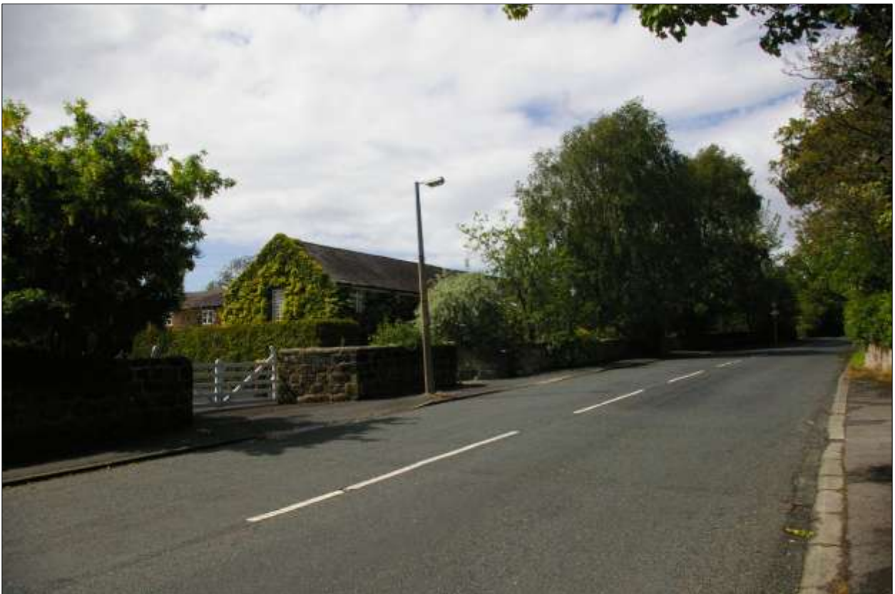
Old Hall, Aughton; from the south-east.
