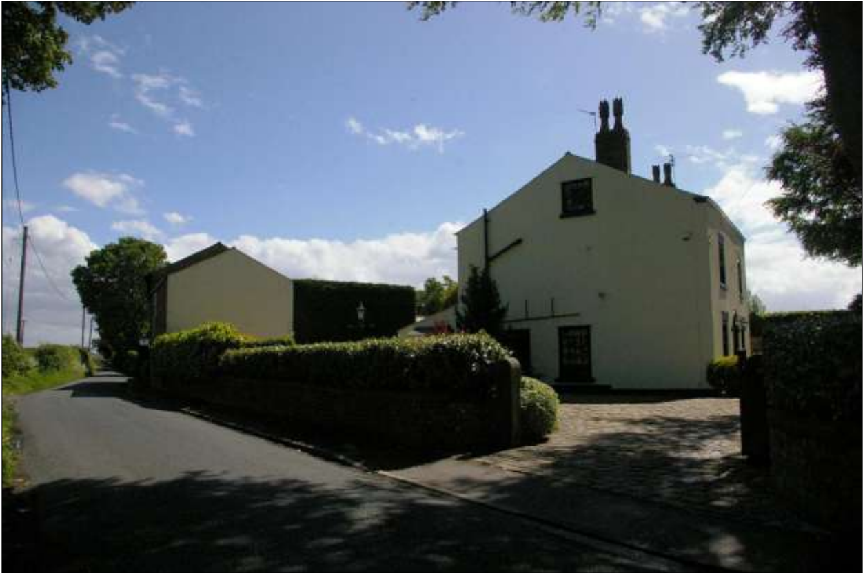
Aughton House, south-east of the rest of the village; from the west-north-west.
