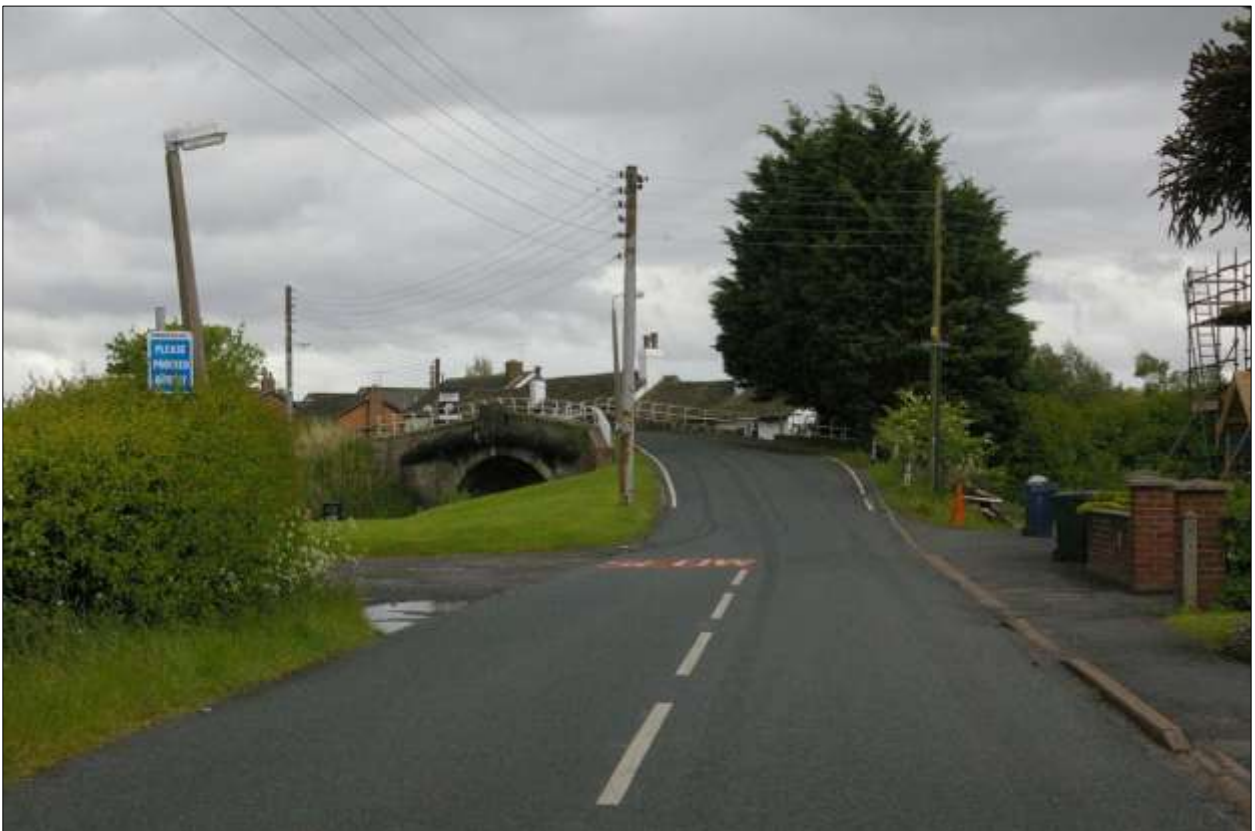
Bridge No.24 over the Leeds and Liverpool Canal, near Halsall; from the west, north-west.
