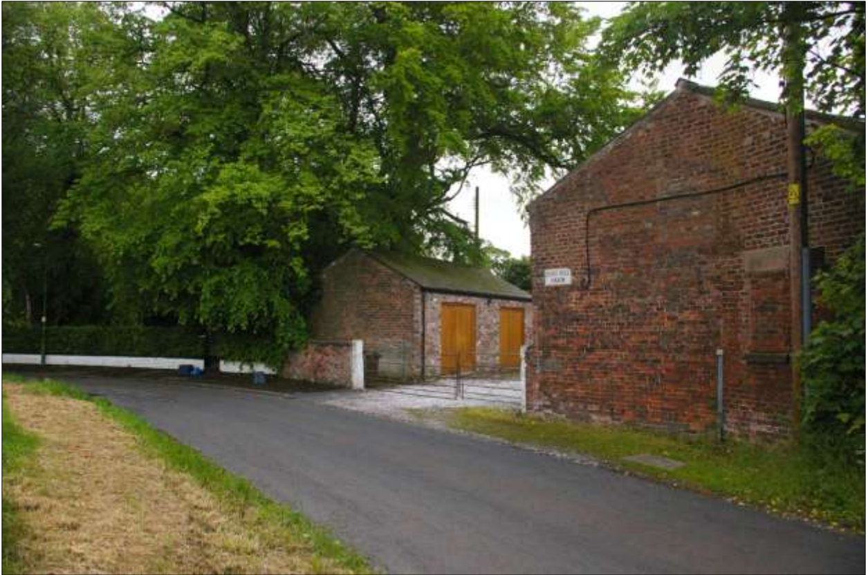
The stables and barns at Rose Hill House; from the north.
