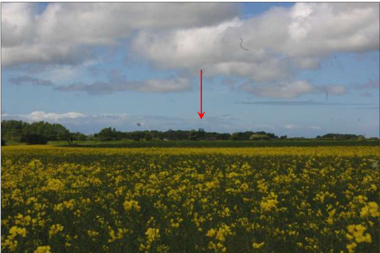
View to the tower, parapet and finials of the Catholic Church of Our Lady, Lydiate (indicated), across the fields; from the east.
