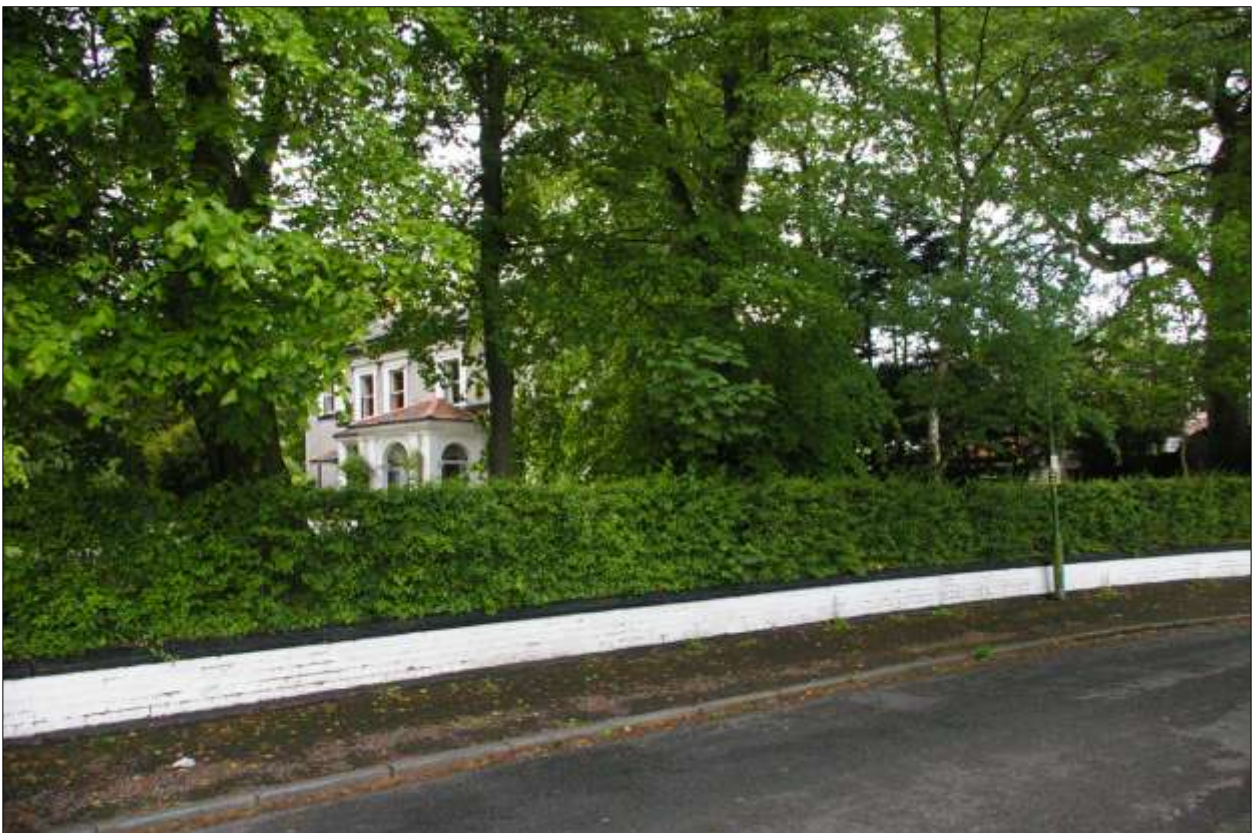
Rose Hill House within its landscaped wooded gardens; from the north-east.
