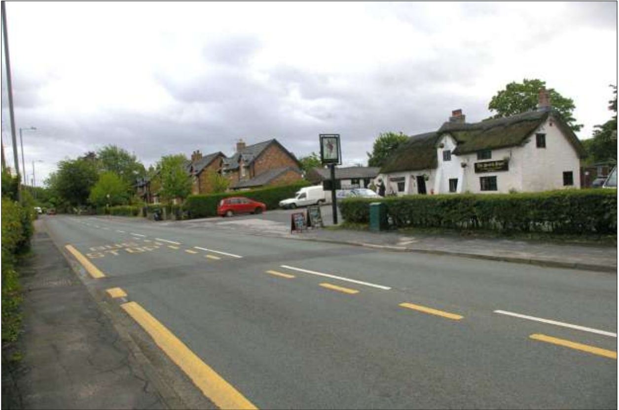
The Scotch Piper public house in Lydiate; from the north-east.
