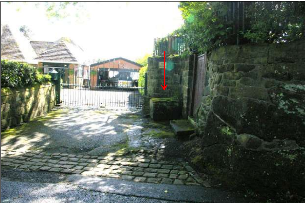
The cross base with socket (indicated) on Mill Lane, Aughton; from the north.
