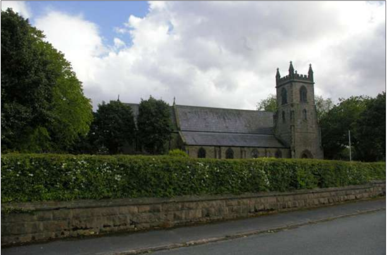
The Church of Our Lady, the Catholic church at Lydiate; from the north-east.
