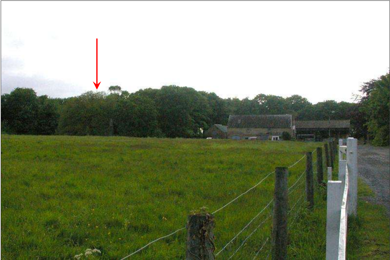
The ruins of Lydiate Hall (indicated) set amongst the trees; from the north-east.
