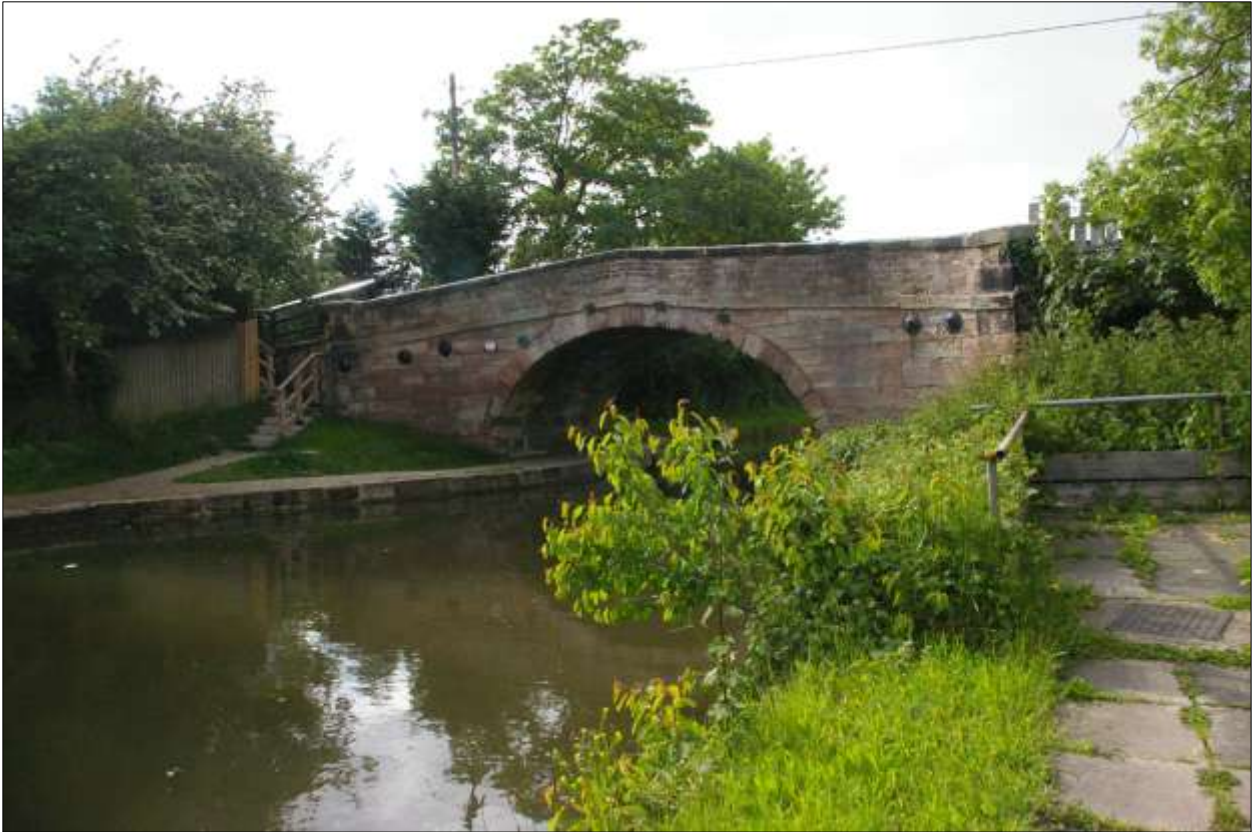
Lydiate Bridge, across the Leeds and Liverpool Canal; from the south-east.
