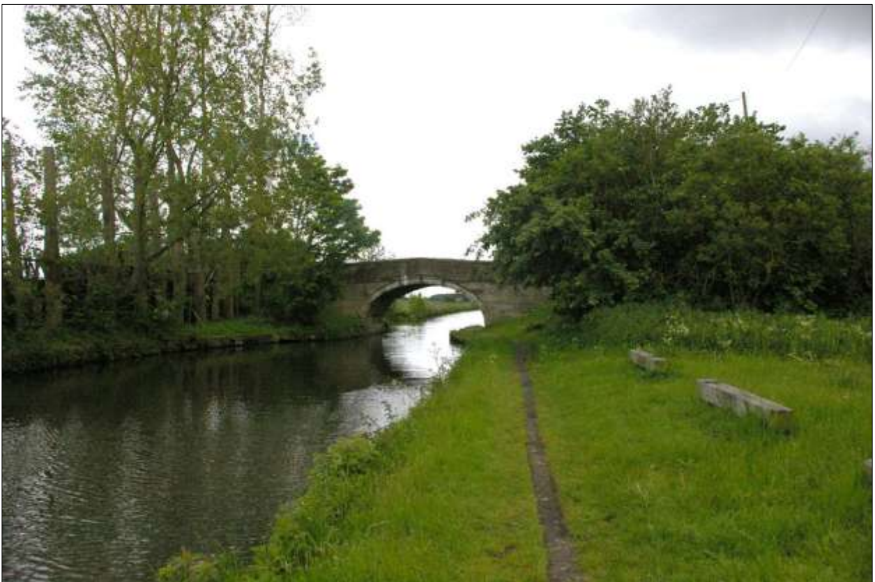
Harkers Bridge, over the Leeds and Liverpool Canal, near Halsall; from the north-north-west.
