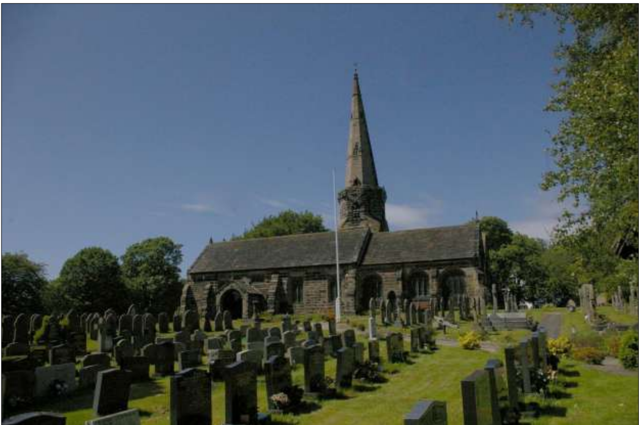
Aughton Church in its large open churchyard; from the south-east.
