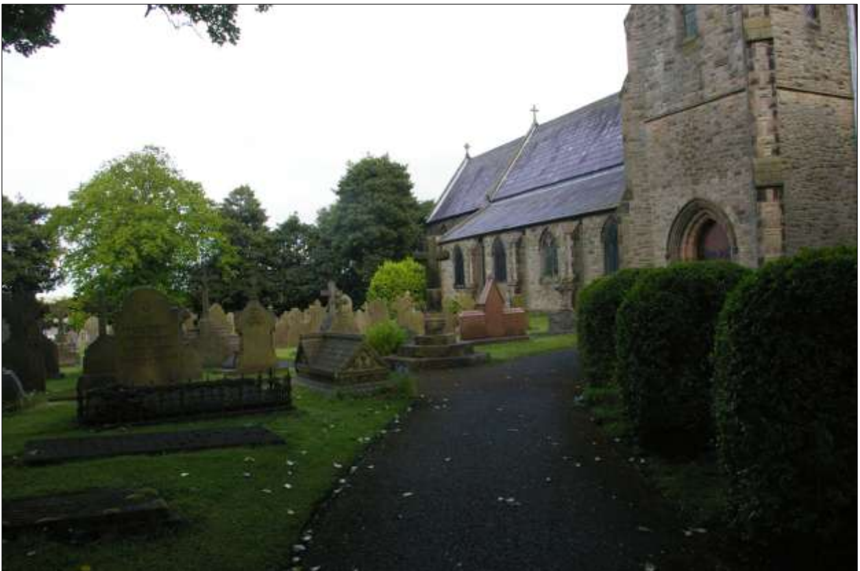
The cross in the churchyard from the west-north-west.
